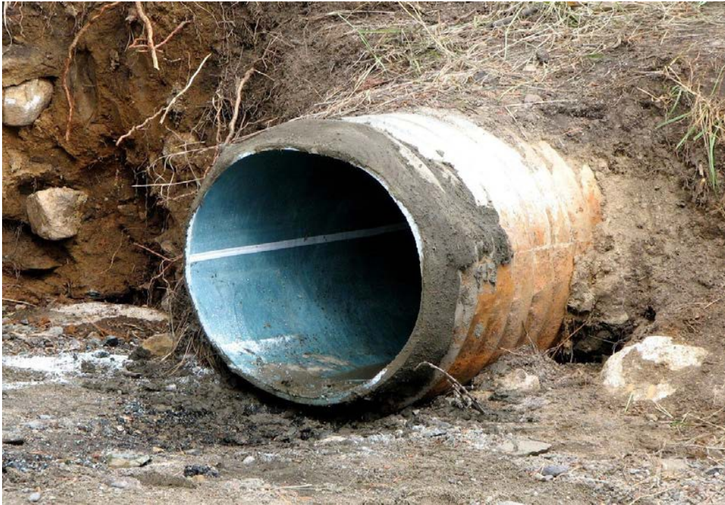
Figure 21. View of a fully installed CIPP liner ( Note intimate contact of the liner with the pipe).
