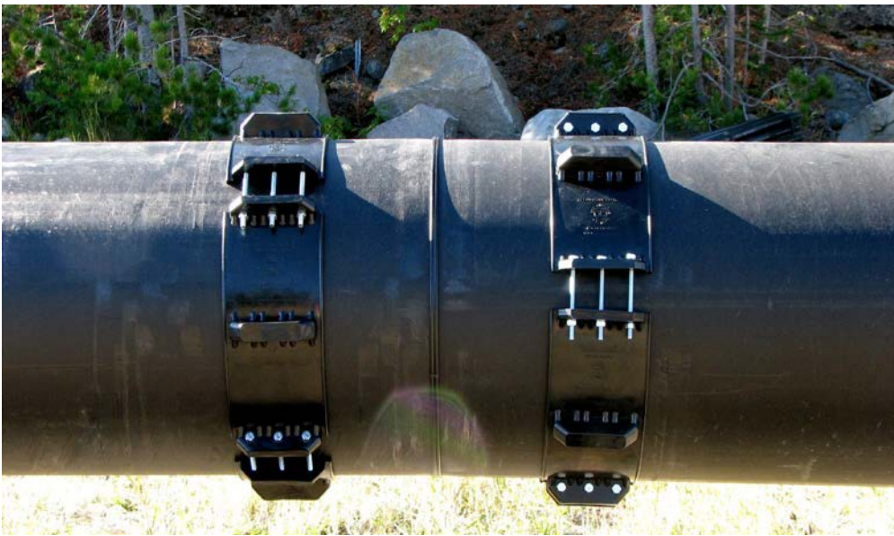
Figure 6. View of the welded pipes and spacers.
