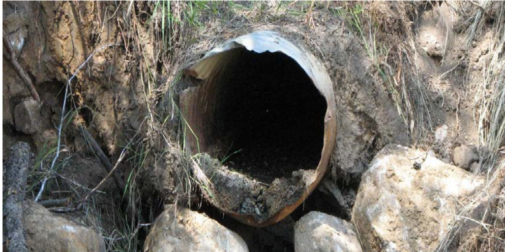
Figure 2. Existing condition of a typical culvert at the project site.
