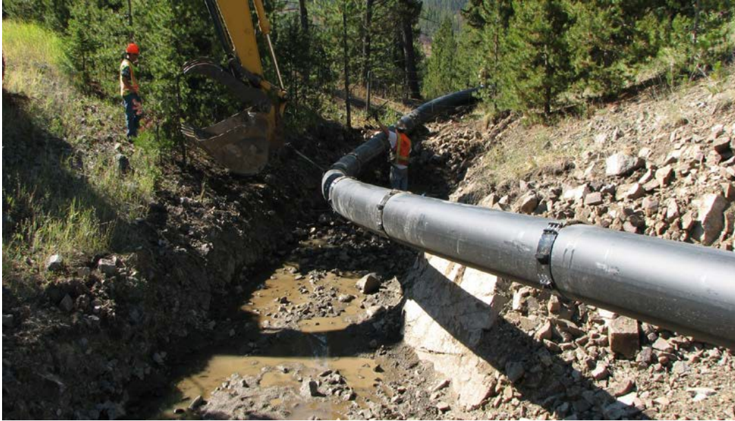
Figure 7. View of the welded HDPE liner ready for installation.
