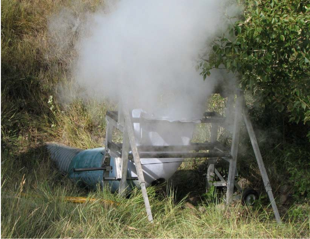
Figure 19. View of steam exiting at the intake end of the culvert.
