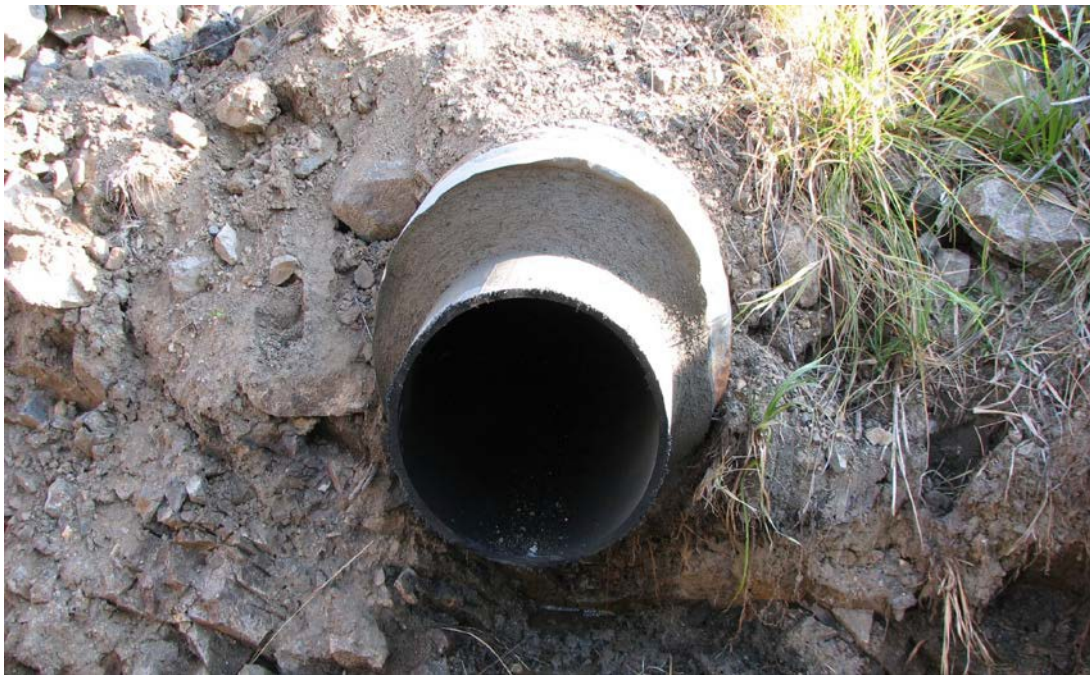
Figure 10. Fully installed HDPEP and the cementitious materials.
