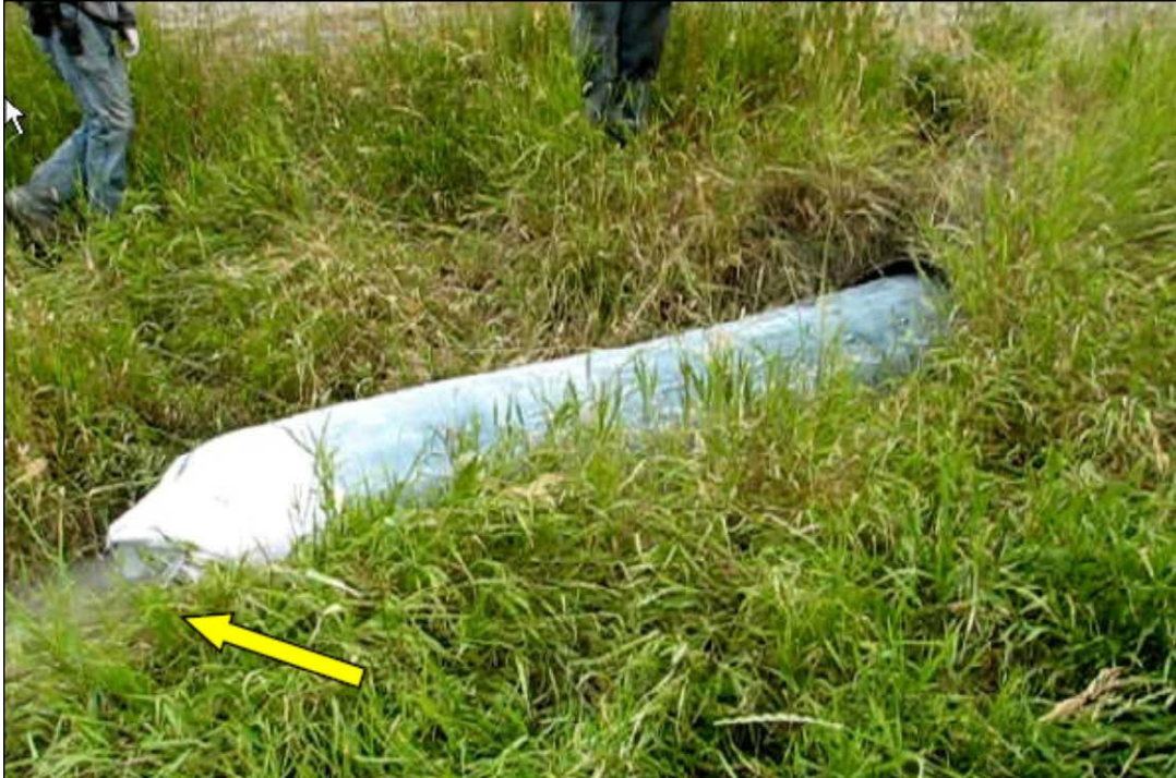
Figure 16. Fully exited liner at the outlet end.
