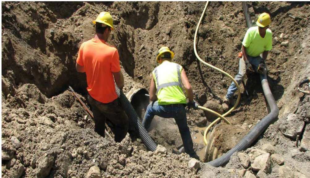
Figure 3. Cleaning and removal of debris from the existing CSP.
