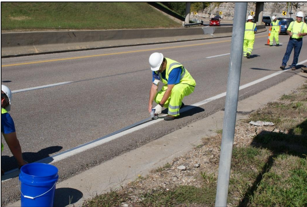
Figure 5. Photo. Workers cover existing lane markings before application of HFST.
