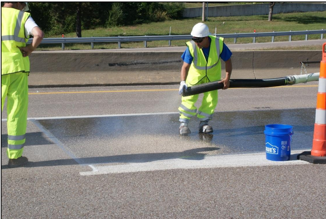
Figure 9. Photo. Surface material blown onto recently placed epoxy binder.
