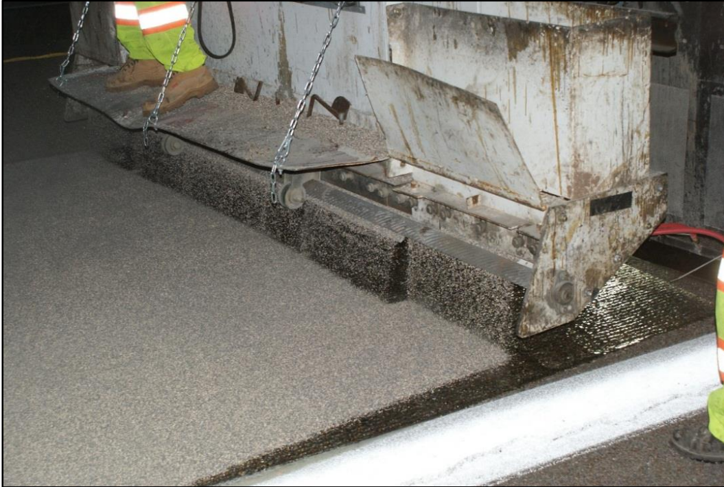
Figure 19. Photo. Bauxite chips dropped onto surface following application of epoxy resin.
