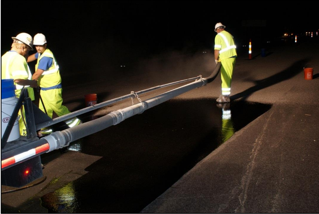
Figure 23. Photo. Bauxite material blown onto surface of previously installed epoxy binder.
