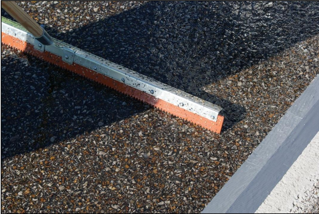
Figure 7. Photo. Epoxy spread using notched squeegee.
