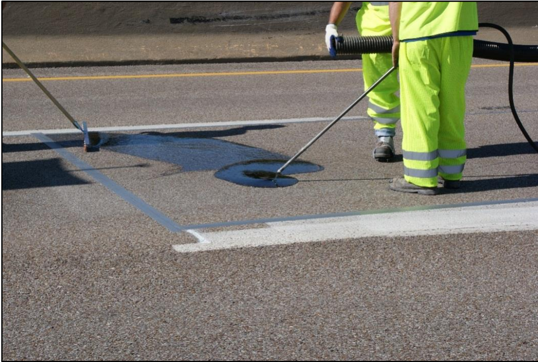
Figure 6. Photo. Application of epoxy to road surface.
