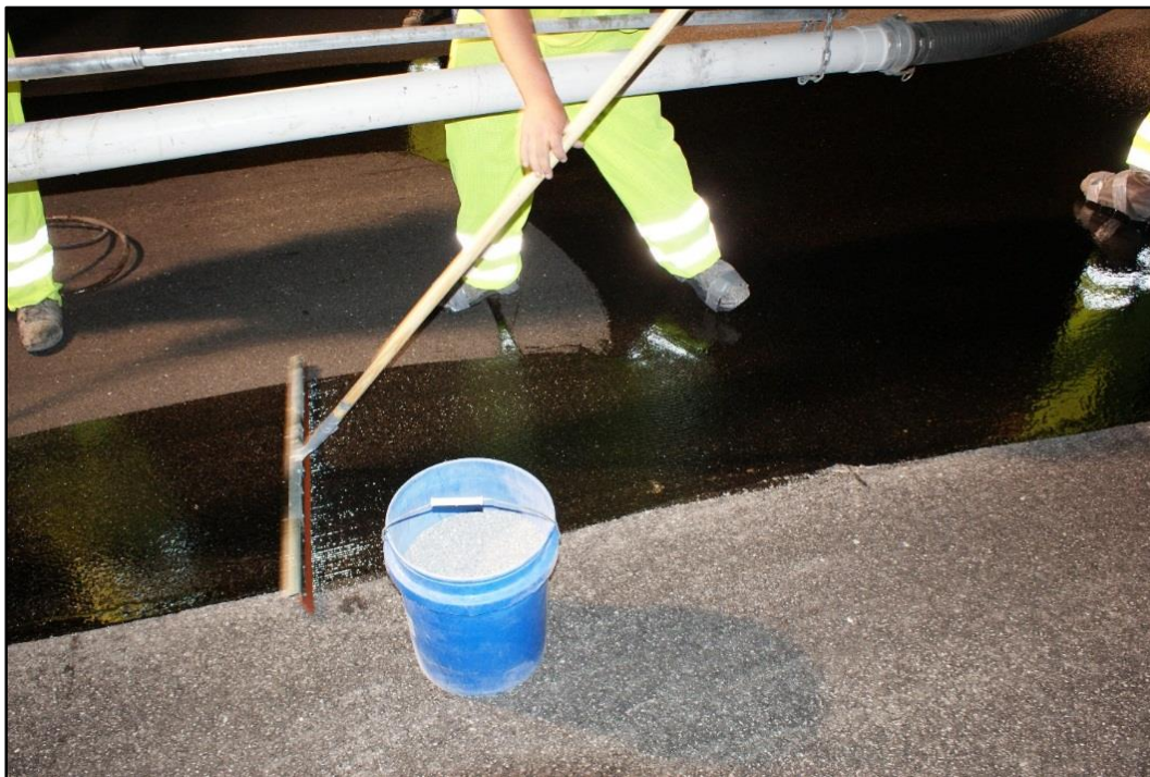
Figure 22. Photo. Epoxy material spread using notched squeegee.
