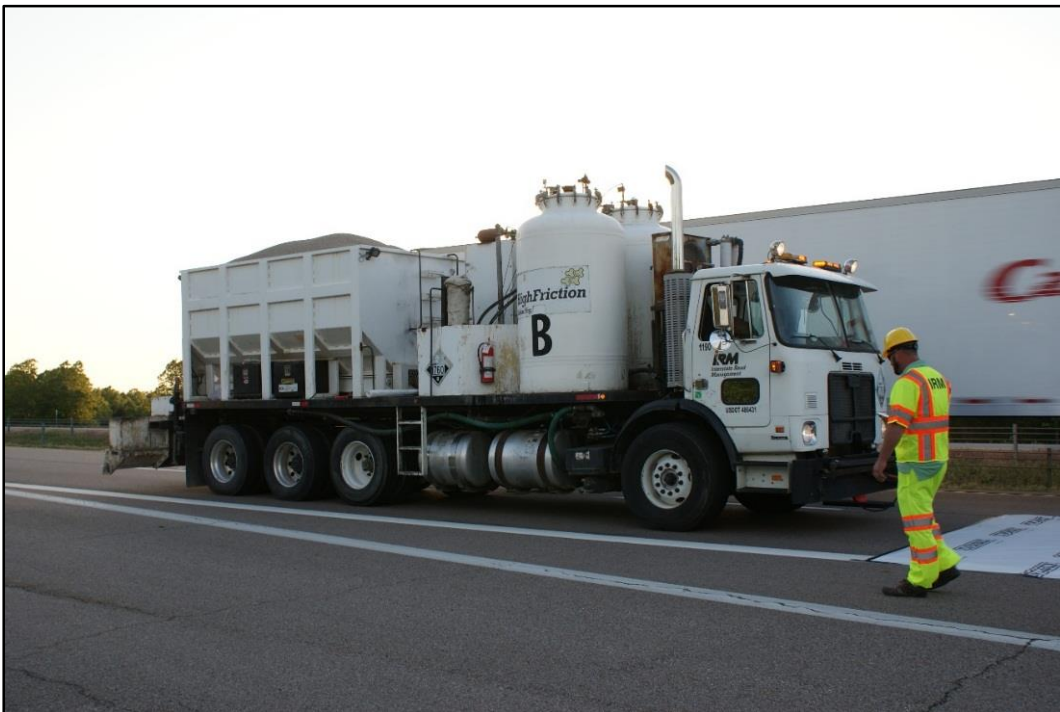
Figure 18. Photo. Machine used to place HFST.
