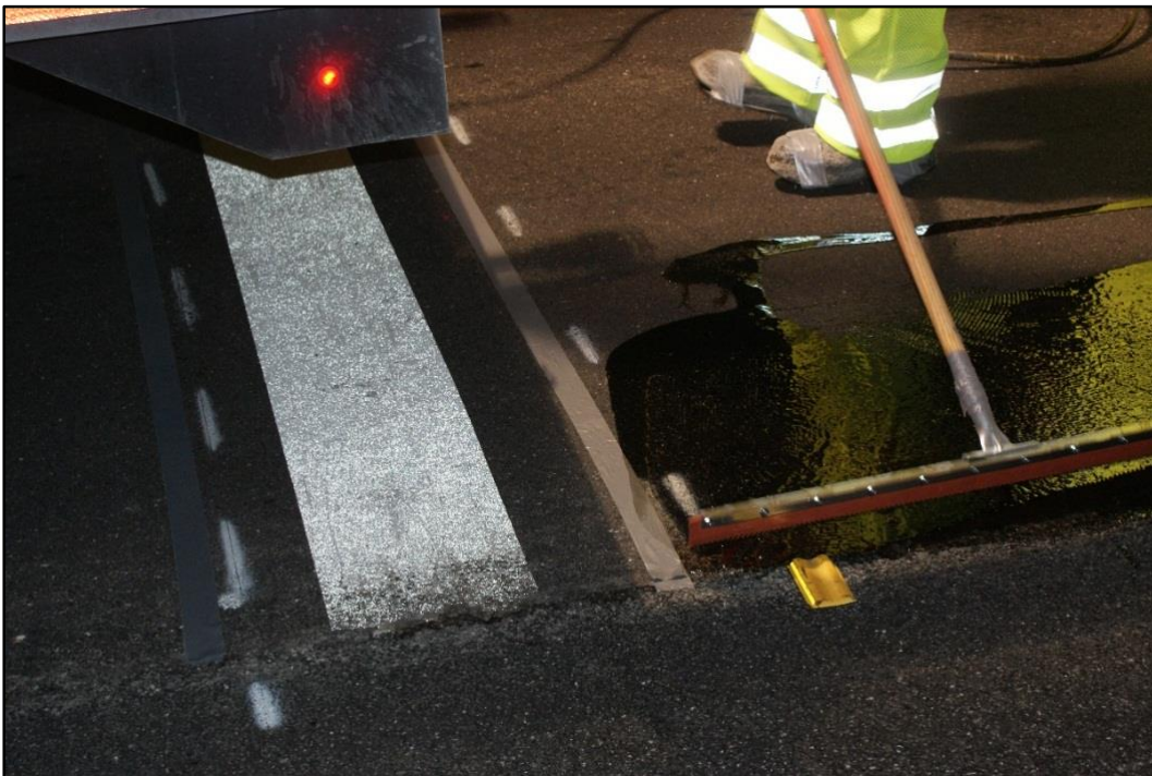
Figure 24. Photo. Workers apply epoxy material near previously installed pavement markings.
