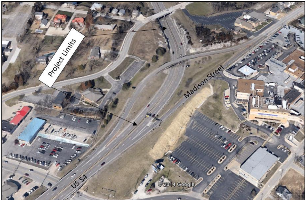
Figure 2. Photo. US 54, Jefferson City, Missouri near Madison Street Exit (courtesy: Google Earth).
