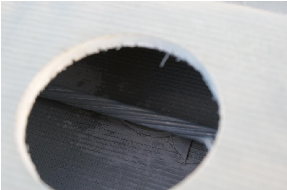
Figure 9. Filler openings located at one-quarter points along the beam top with steel reinforcing strand visible.
