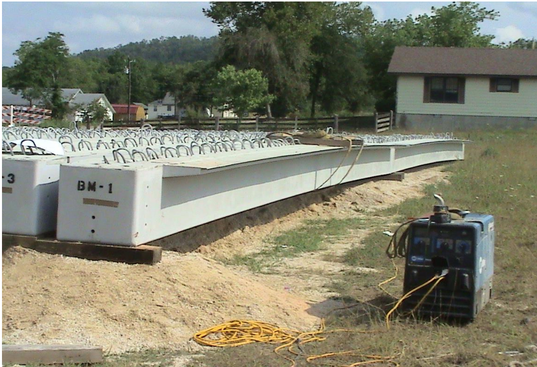
Figure 29. Beams at staging location after insertion of shear steel.
