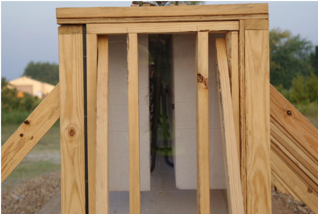
Figure 5. End view of mockup showing location and density of web reinforcement.
