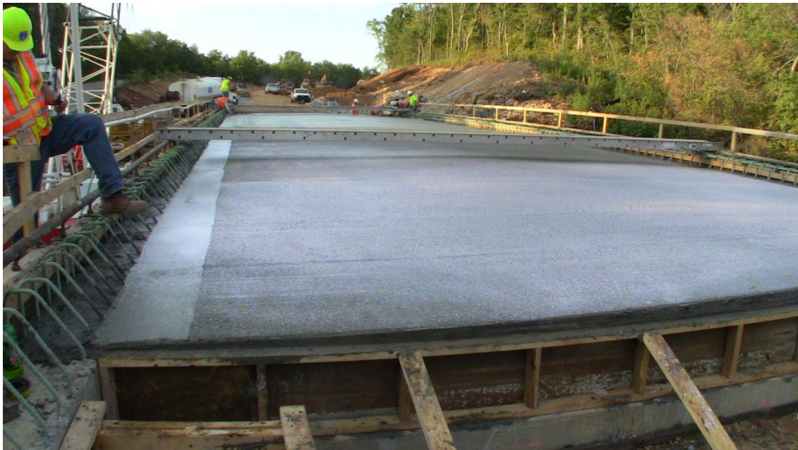
Figure 47. Completed deck on MO 97, Dade County.
