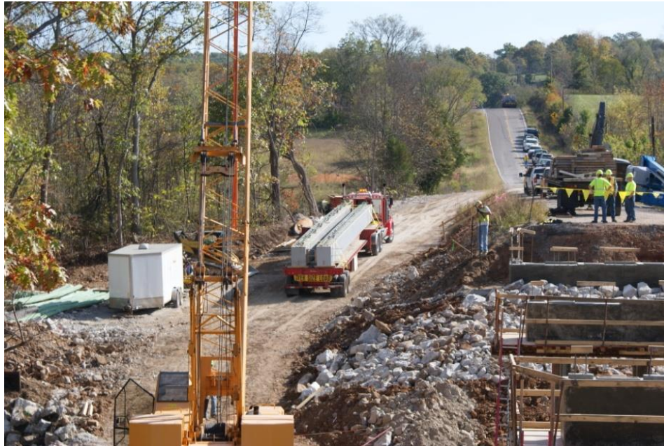
Figure 16. Delivery of beams to Douglas County project.
