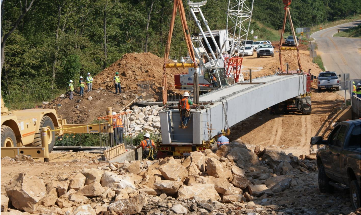
Figure 44. First beam attached to cranes for placement.
