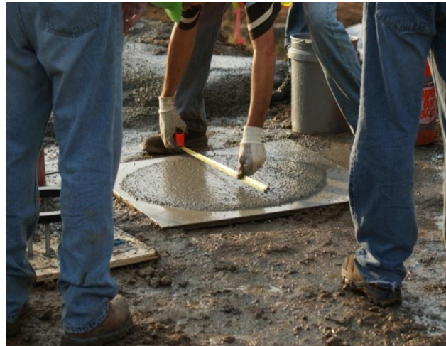
Figure 27. Modified slump test.
