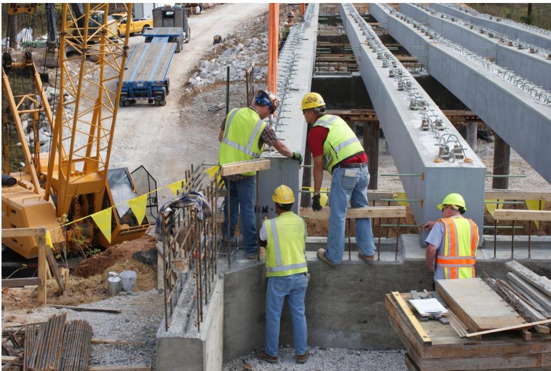
Figure 20. Final beam set in place.
