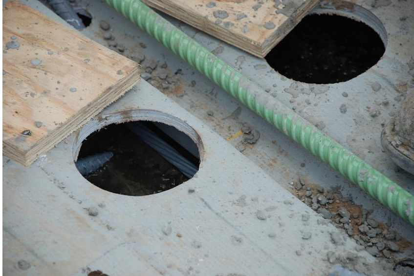
Figure 33. Original 4-in access holes for concrete introduction.
