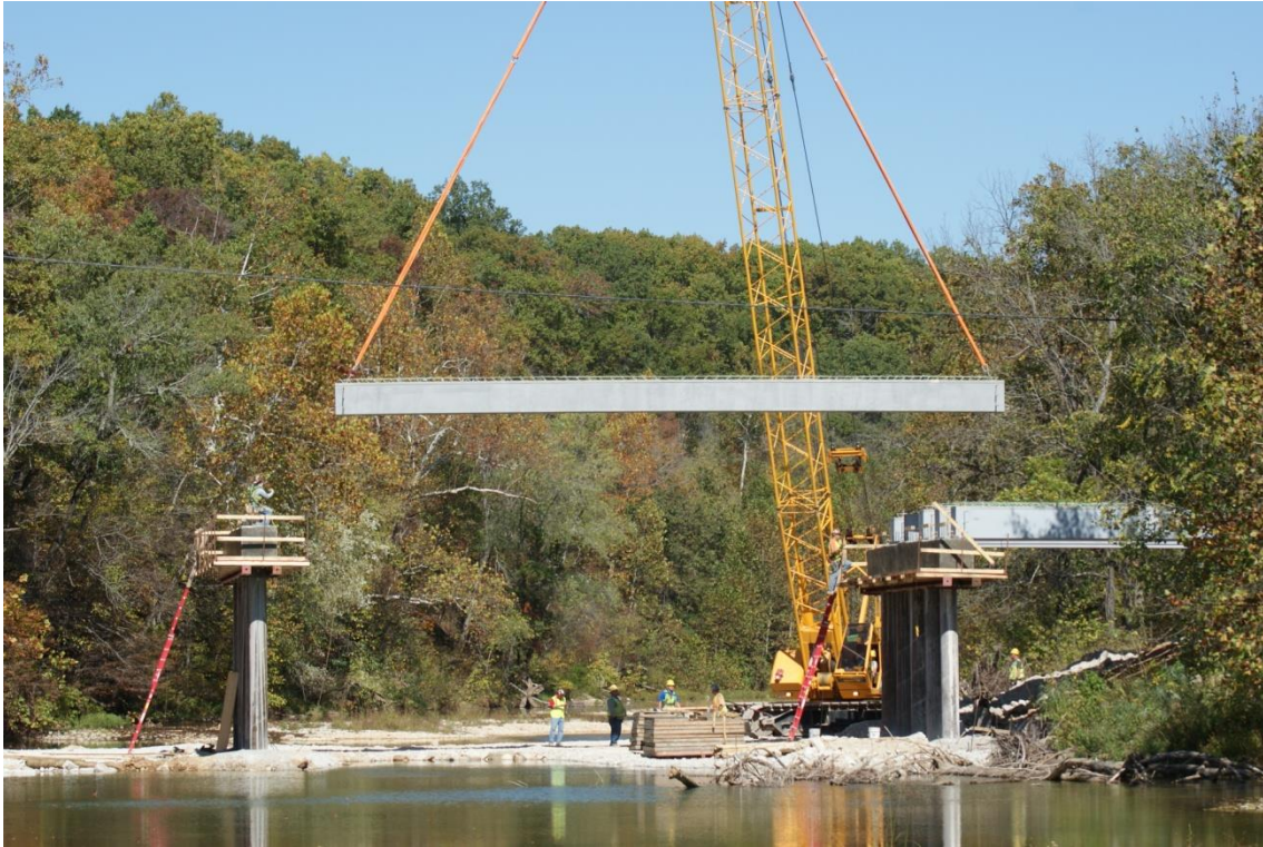
Figure 19. First center span beam lifted into position.
