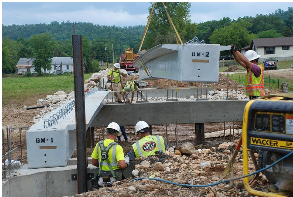
Figure 31. First beams lifted into place over Ottery Creek Overflow. (Photo courtesy of MoDOT)
