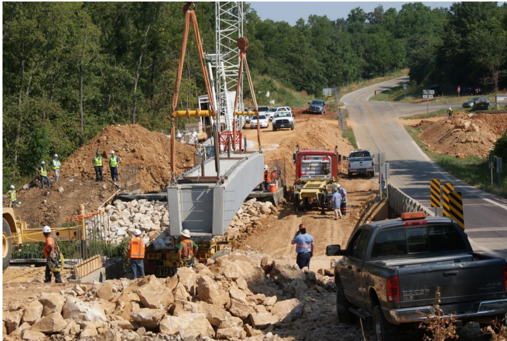
Figure 45. First beam moved into place.
