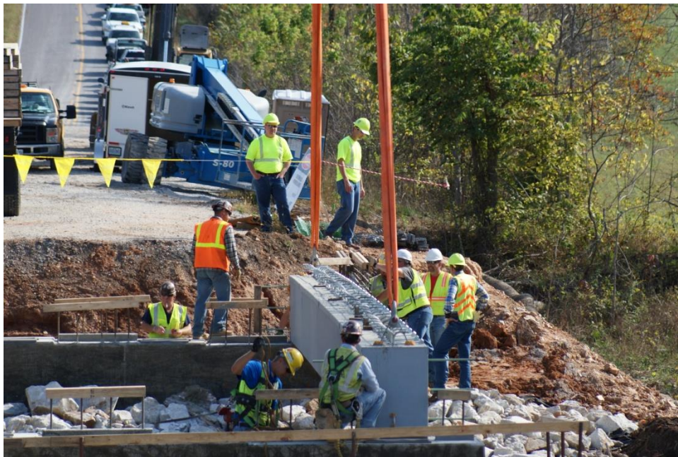
Figure 18. First beams lifted from truck and set in place.
