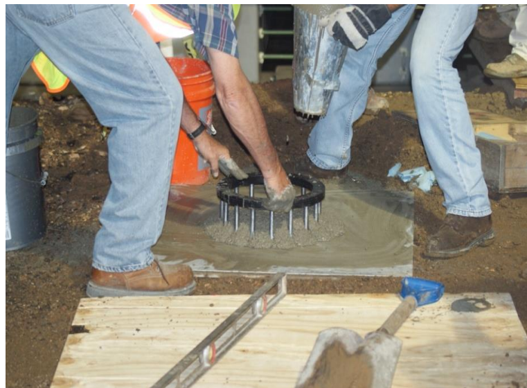
Figure 28. Cage test performed at the Reynolds County site.
