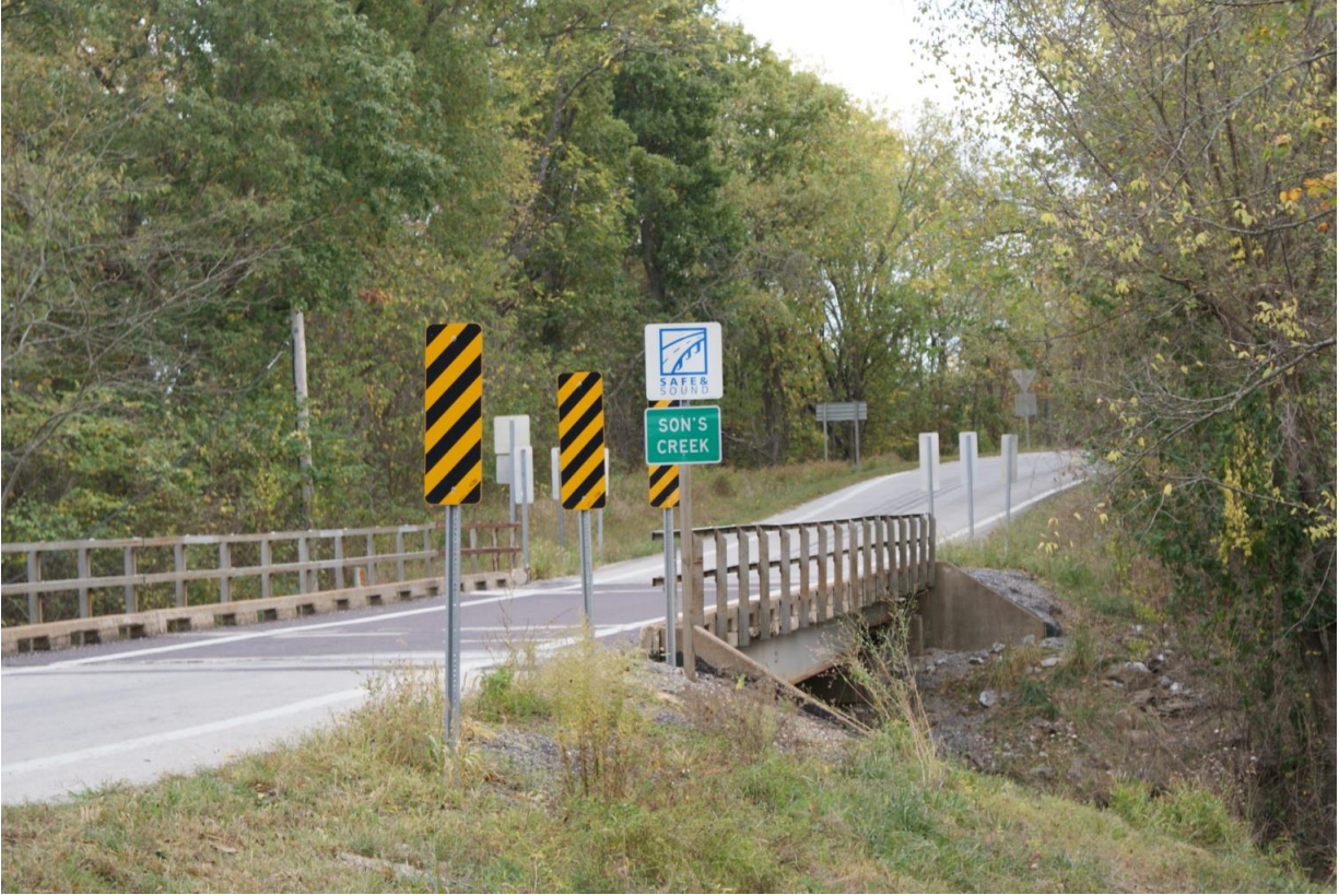
Figure 37. Existing structure on MO 97 over Sons Creek in Dade County.
