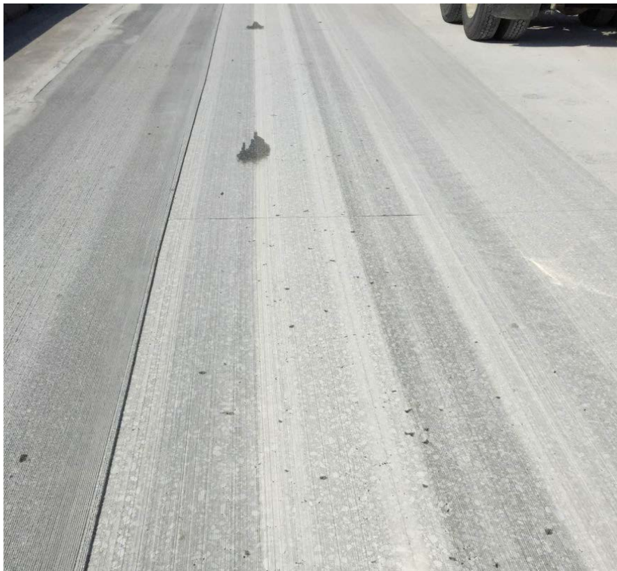
Figure 11. Photo. Flush ground surface created by first pass of NGCS.
