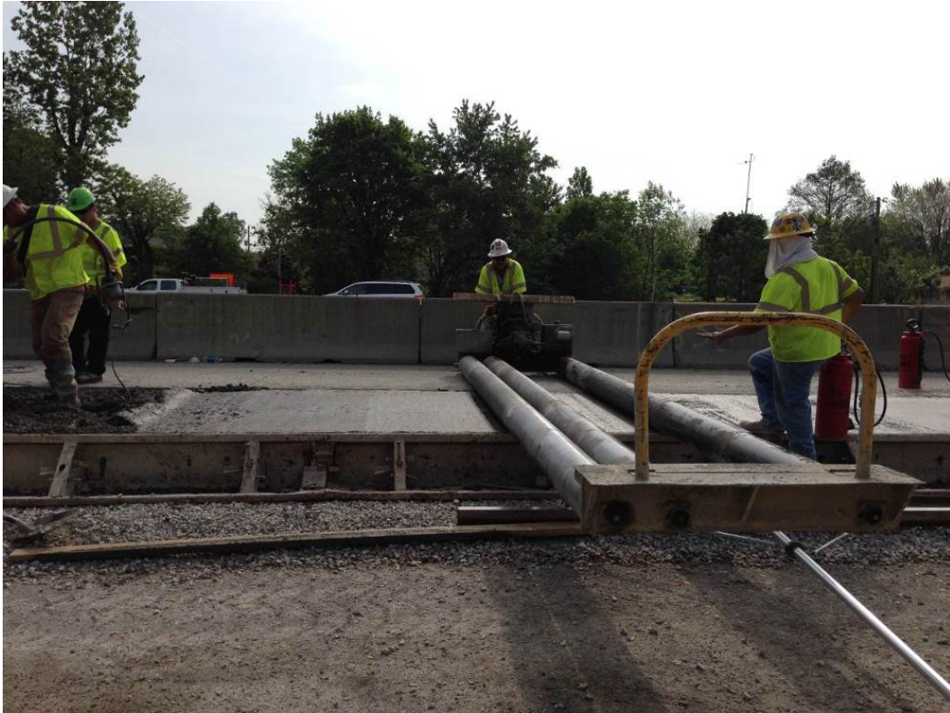
Figure 9. Photo. Tube rolling of concrete material.
