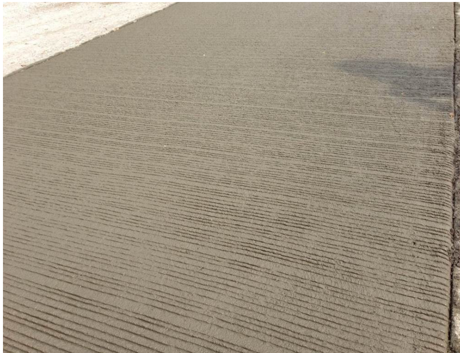
Figure 14. Photo. Concrete surface with INDOT's traditional transverse tining finish.
