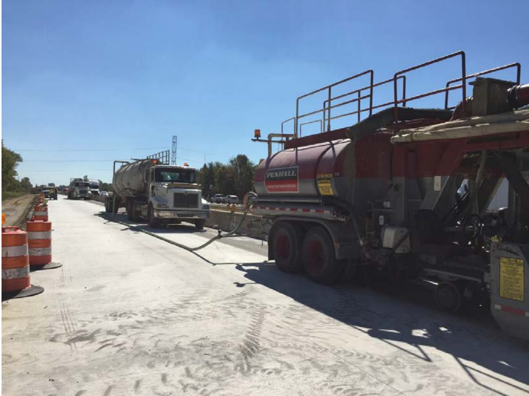
Figure 10. Photo. Application of NGCS – first pass.
