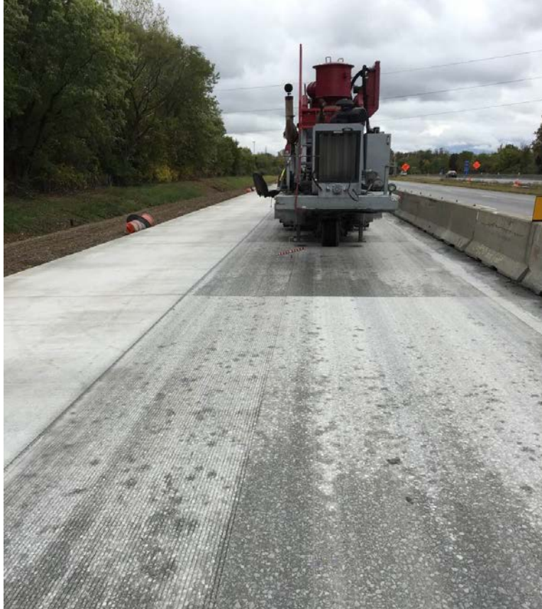
Figure 12. Photo. Application of NGCS – second pass.
