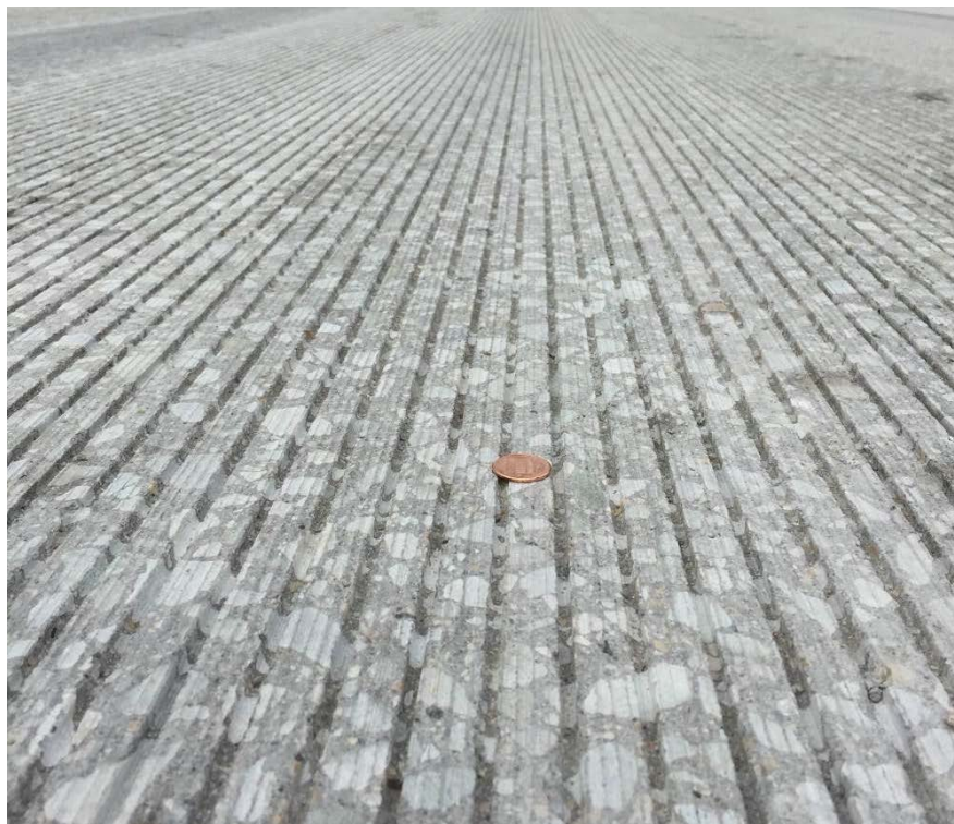
Figure 13. Photo. Concrete surface with double pass NGCS.
