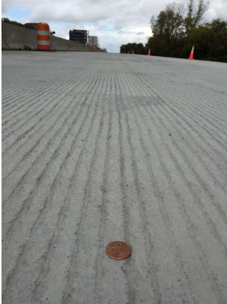
Figure 15. Photo. Concrete surface with longitudinal tining finish.
