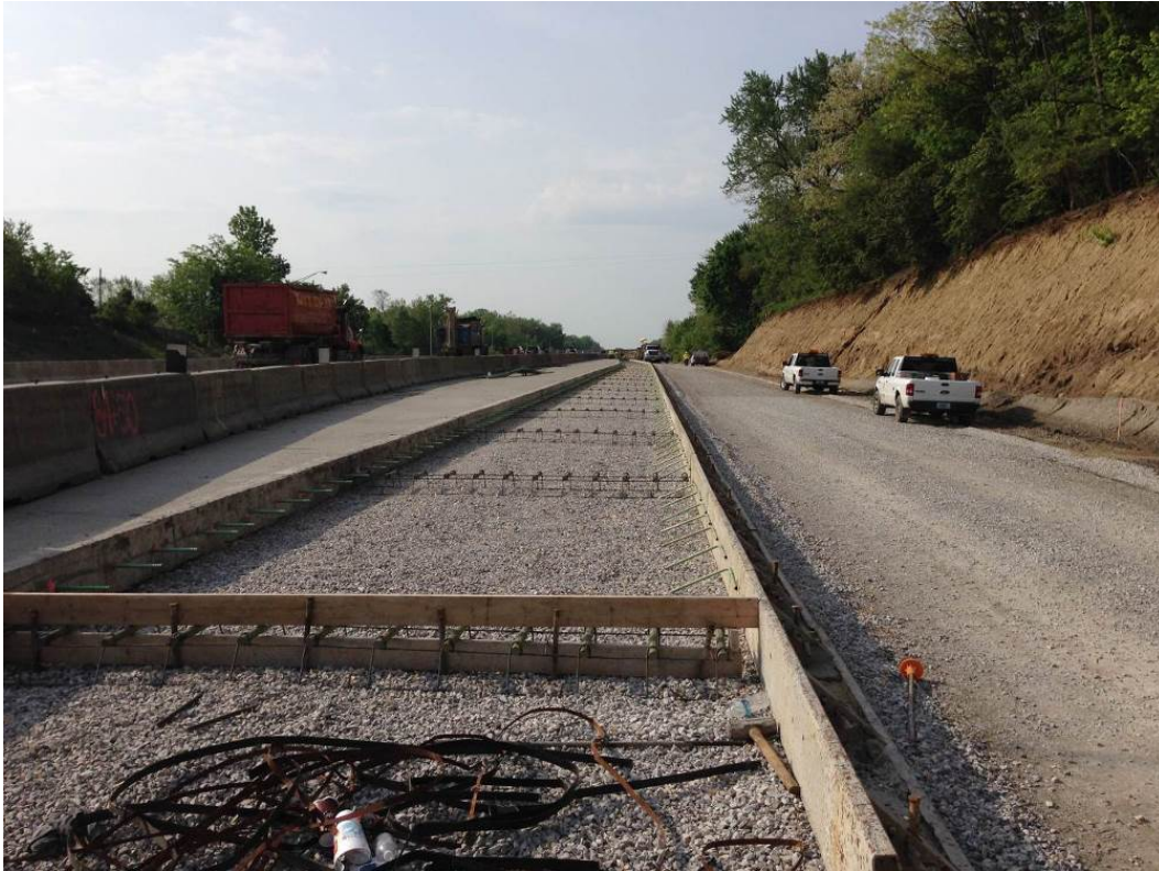
Figure 7. Photo. Dowel bar placement and tie bar retrofit.
