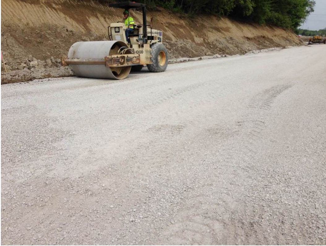
Figure 6. Photo. Subbase preparation for concrete paving.
