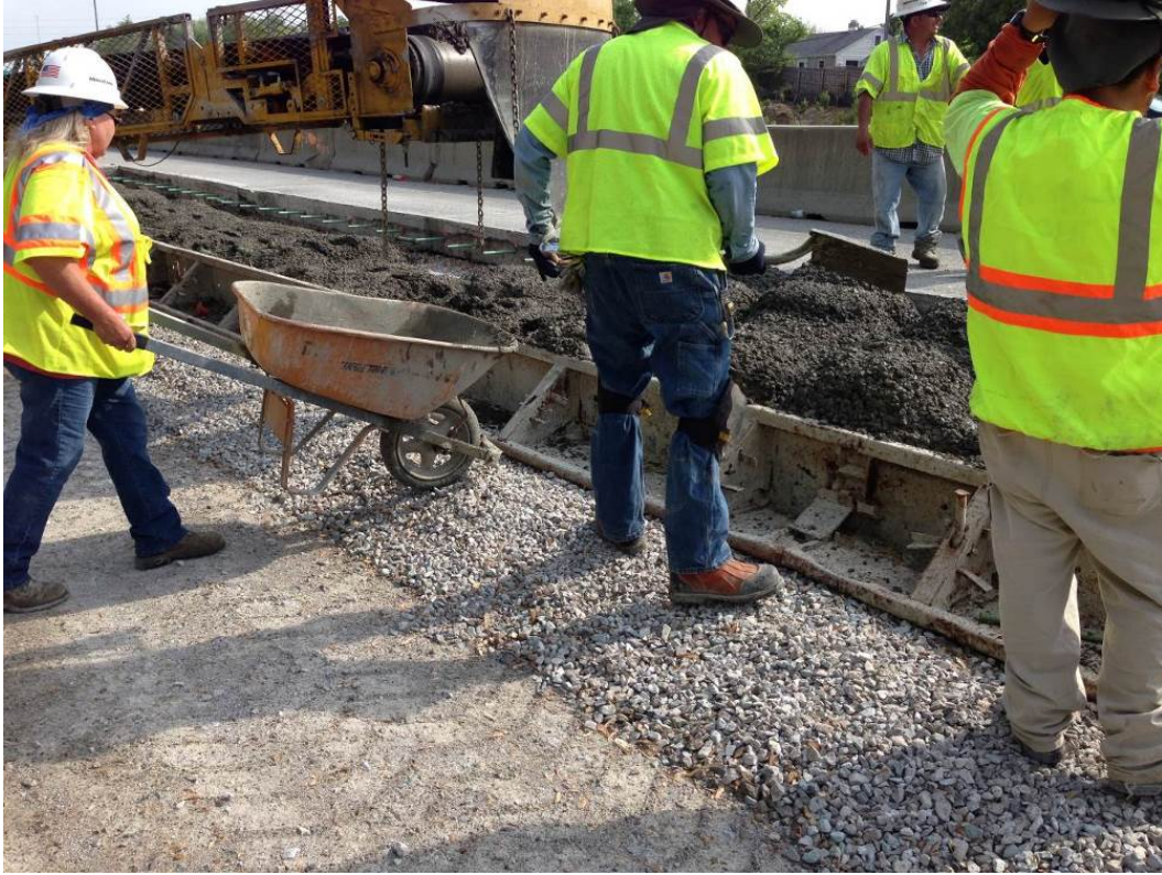
Figure 8. Photo. Placement of fresh concrete.
