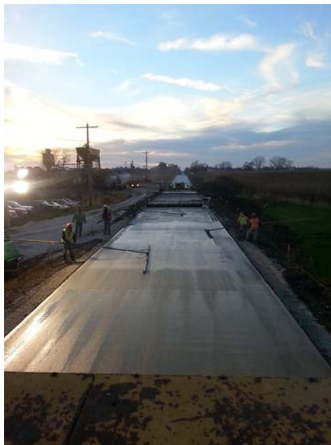
Figure 13. Photo. Concrete finishing. (courtesy: Knox County Highway Department)
