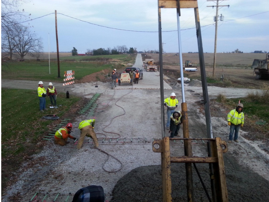
Figure 10. Photo. Aggregate base and dirt fill being carried out. (courtesy: Knox County Highway Department)
