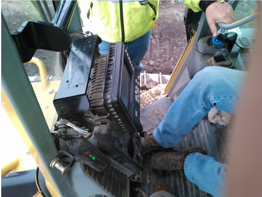
Figure 5. Photo. Operator using the on-board computer on the bulldozer.
