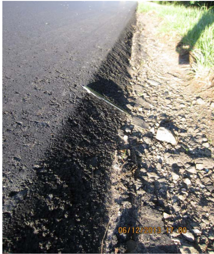
Figure 11. Photo. Close-up of the Safety Edge pavement.
