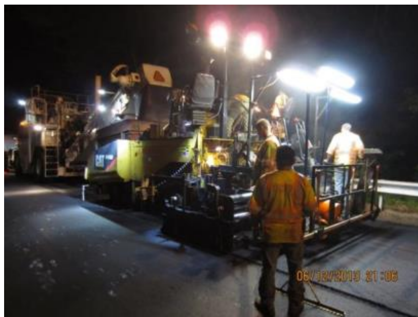
Figure 5. Photo. Paving of I-95.
