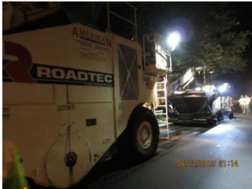
Figure 6. Photo. Roadtec material transfer device.
