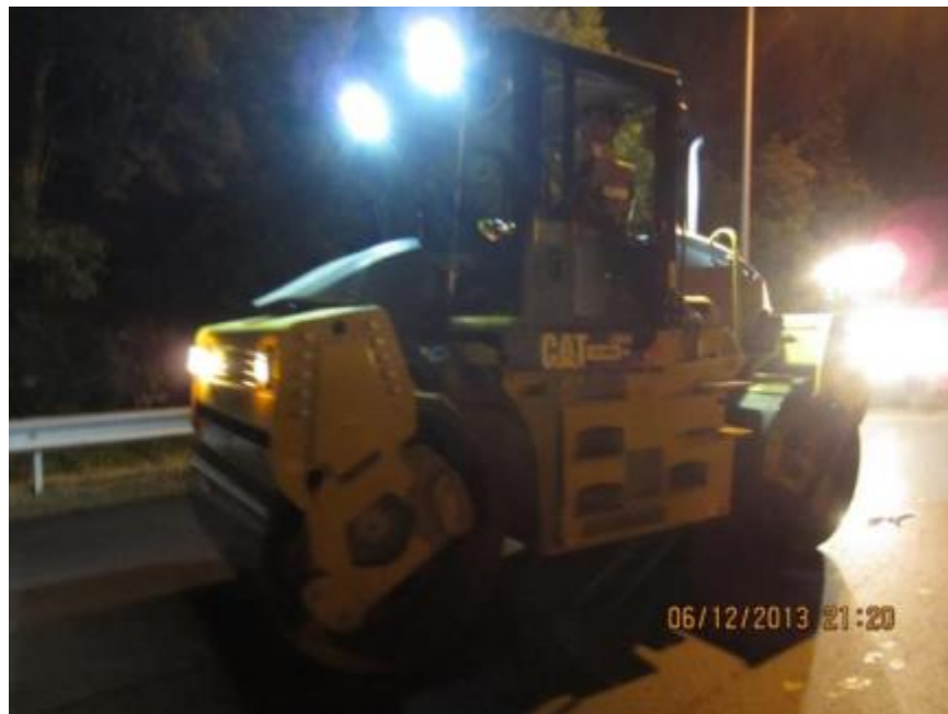
Figure 7. Photo. Compaction roller.
