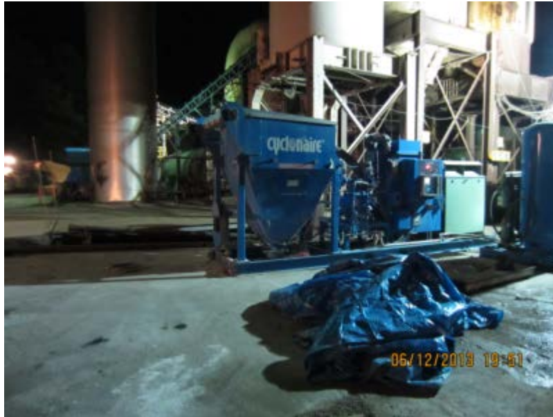
Figure 4. Photo. Cyclonaire injector system for the Advera WMA additive.
