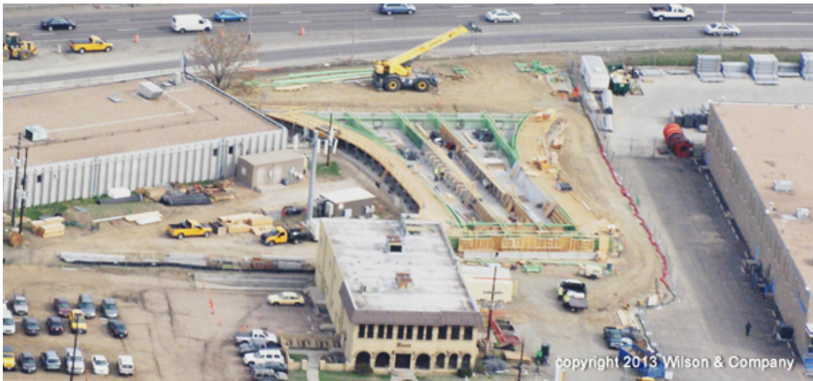
Figure 14. Photo. Overhead view of bridge staging area (courtesy: Colorado DOT).
