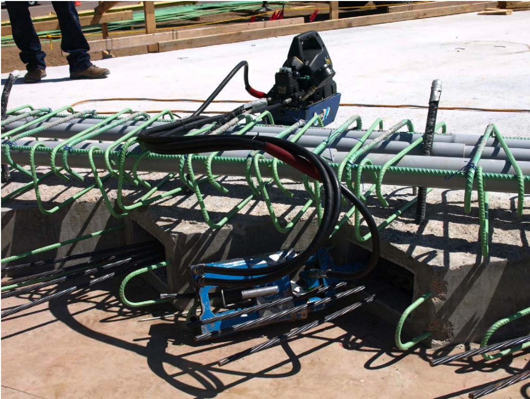
Figure 20. Photo. Transverse deck tendons (courtesy: Colorado DOT).
