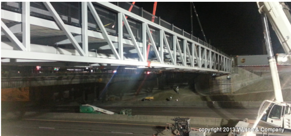
Figure 16. Photo. Placement of pedestrian bridge (courtesy: Colorado DOT).
