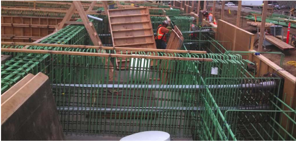
Figure 17. Photo. Longitudinal internal tendons (courtesy: Colorado DOT).
