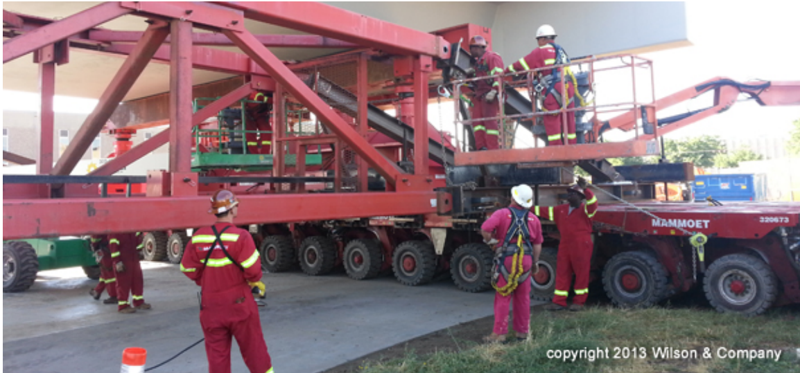
Figure 26. Photo. Workers connecting frame (courtesy: Colorado DOT).
