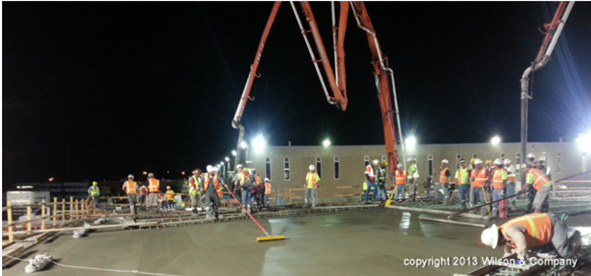
Figure 15. Photo. Deck finishing operation (courtesy: Colorado DOT).
