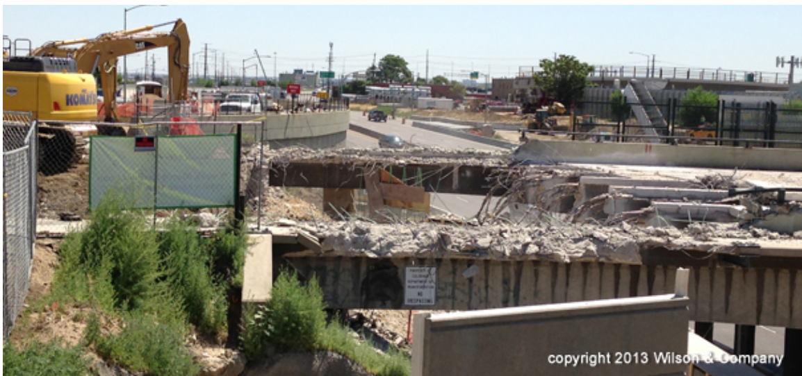
Figure 29. Photo. Daylight view of partially demolished structure (courtesy: Colorado DOT).
