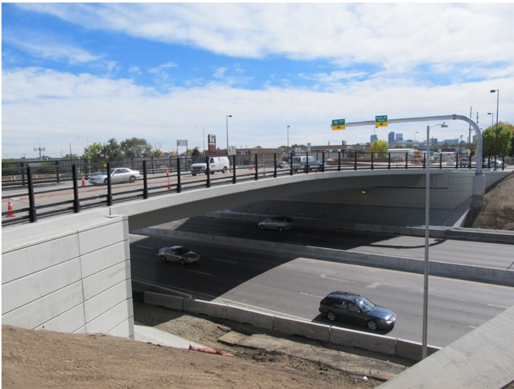
Figure 36. Photo. Profile view of Pecos Street Bridge over I-70 (courtesy: Colorado DOT).
