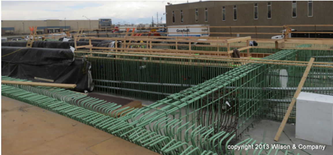
Figure 13. Photo. Epoxy-coated reinforcement for diaphragm (courtesy: Colorado DOT).
