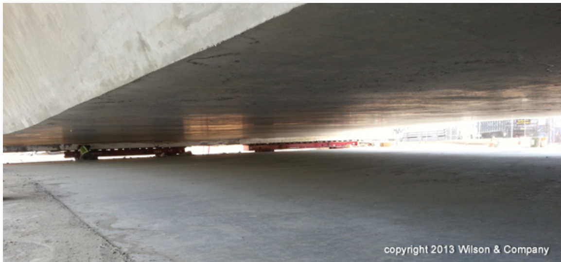
Figure 21. Photo. Completed superstructure on temporary supports (courtesy: Colorado DOT).
