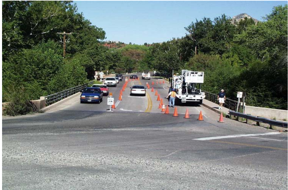
Figure 3.3.1 Traffic Control Operation
