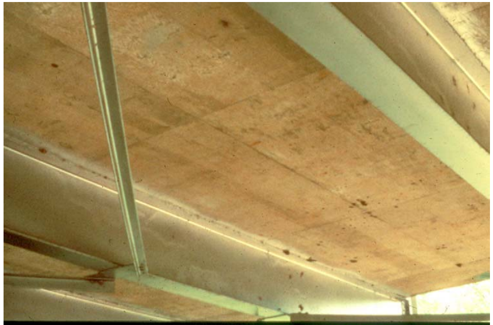
Figure P.2.30 Concrete Deck
