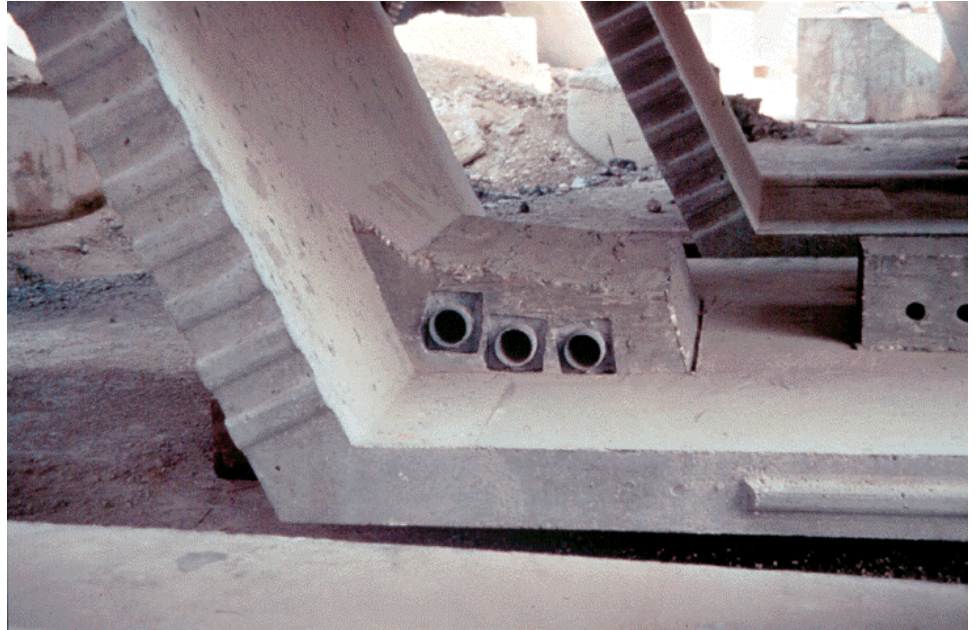
Figure 7.11.40 View of Box Girder Joint and Anchorage Block
