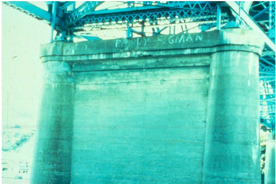
Figure P.2.72 Column Pier with Web Wall
