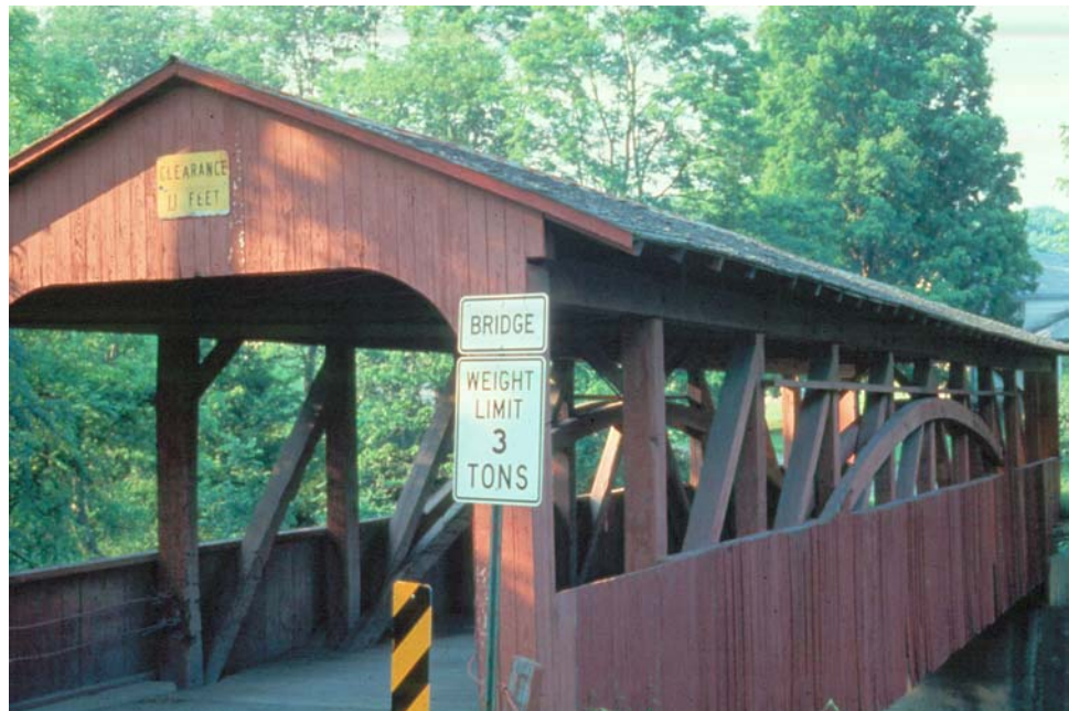
Figure 6.1.8 Burr Arch-truss Covered Bridge
