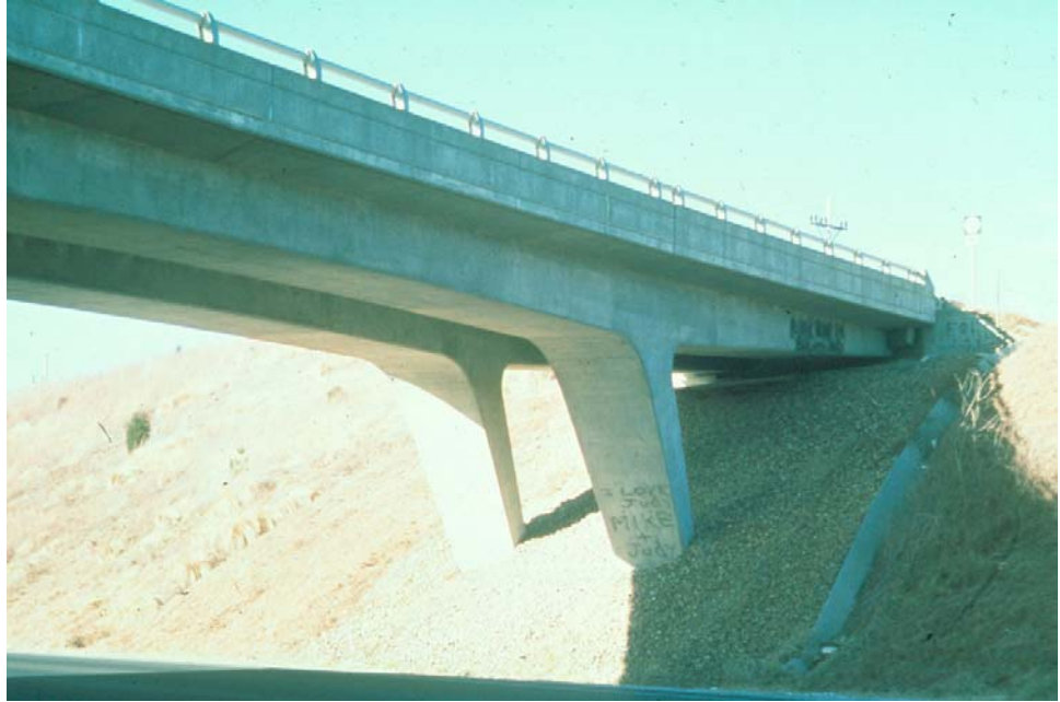
Figure 7.6.14 K-frame Leg
