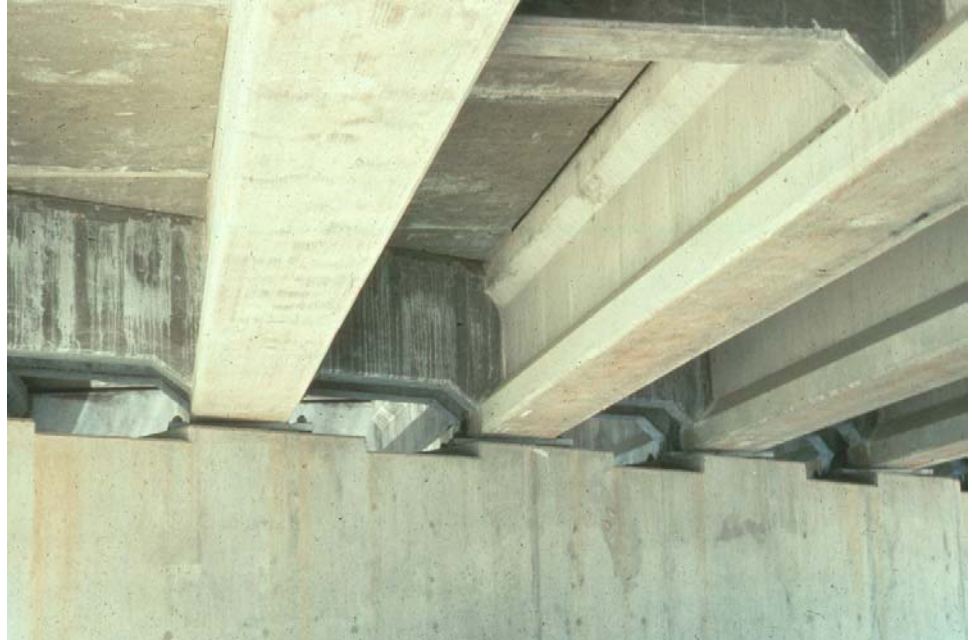
Figure 7.9.6 Concrete End Diaphragm
