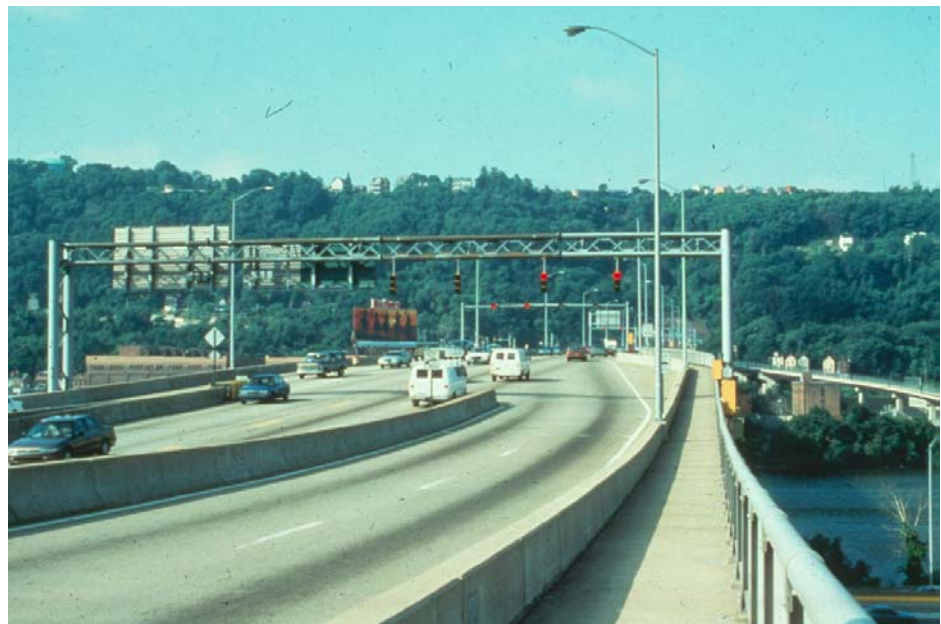
Figure P.2.38 Bridge Lighting
