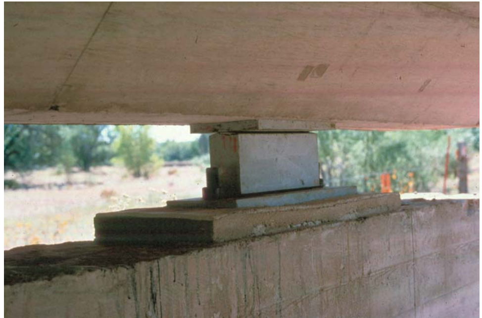
Figure 7.1.4 Steel Rocker Bearing Supporting Haunched Slab at Pier
