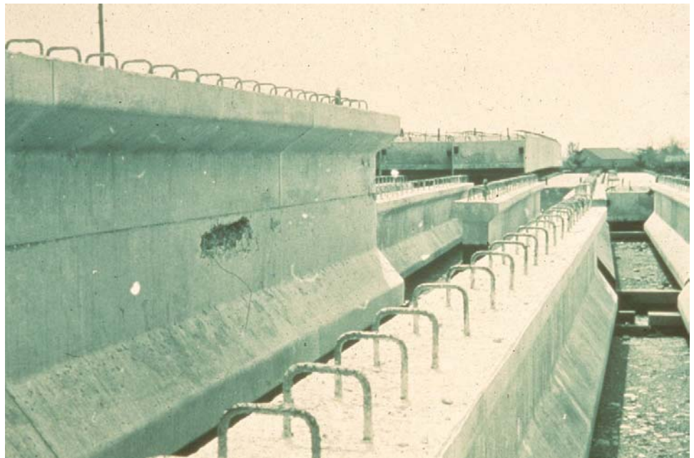
Figure 5.2.4 Prestressed Concrete Beam with Shear Connectors Protruding
