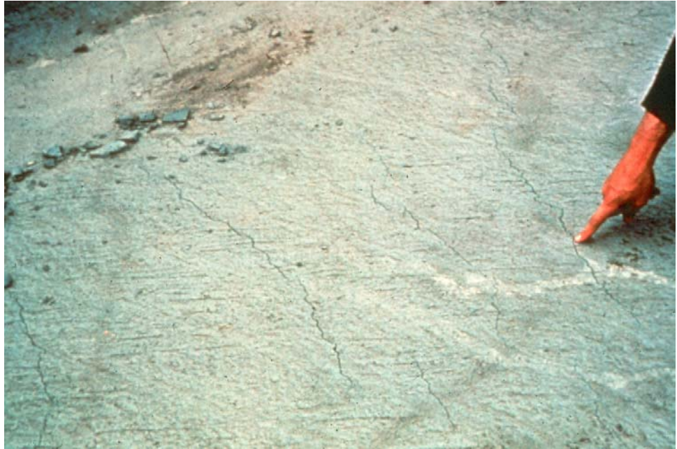
Figure 2.2.11 Temperature Cracks
