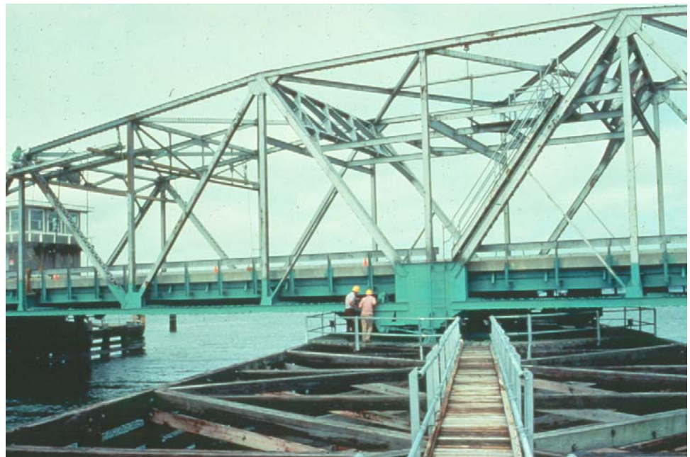
Figure P.2.60 Swing Bridge
