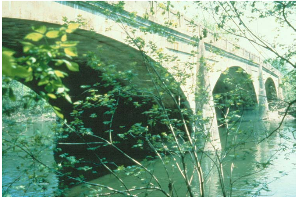
Figure 7.5.2 Multi-span Closed Spandrel Arch Bridge
