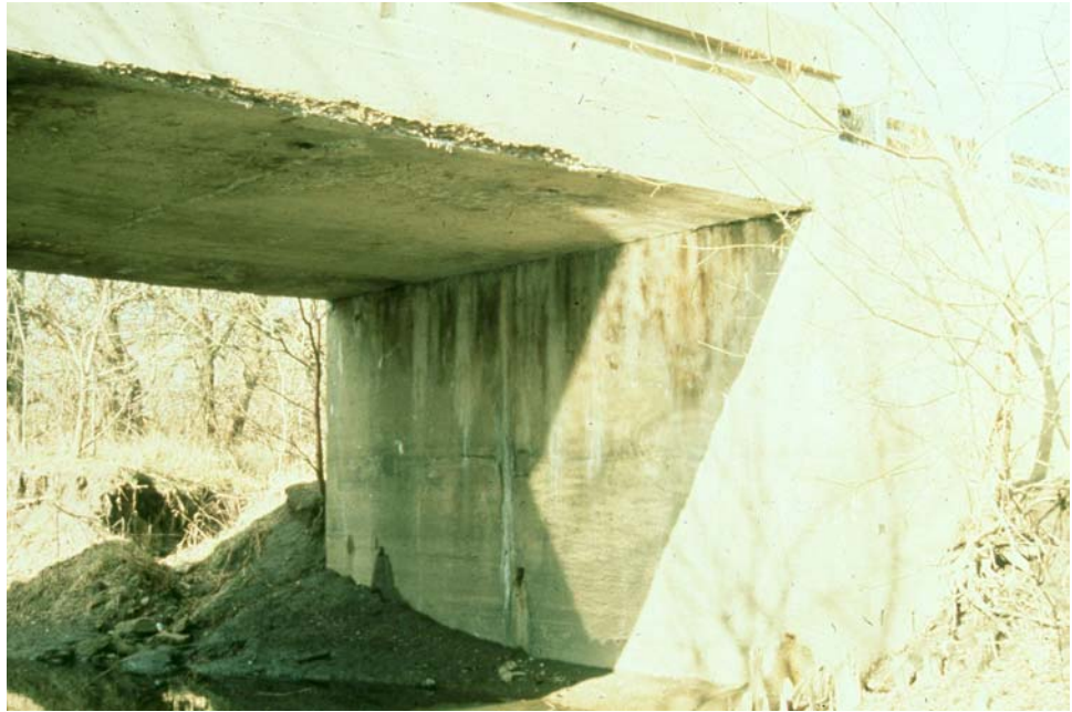
Figure 7.3.6 Bearing Area of a Through Girder Bridge
