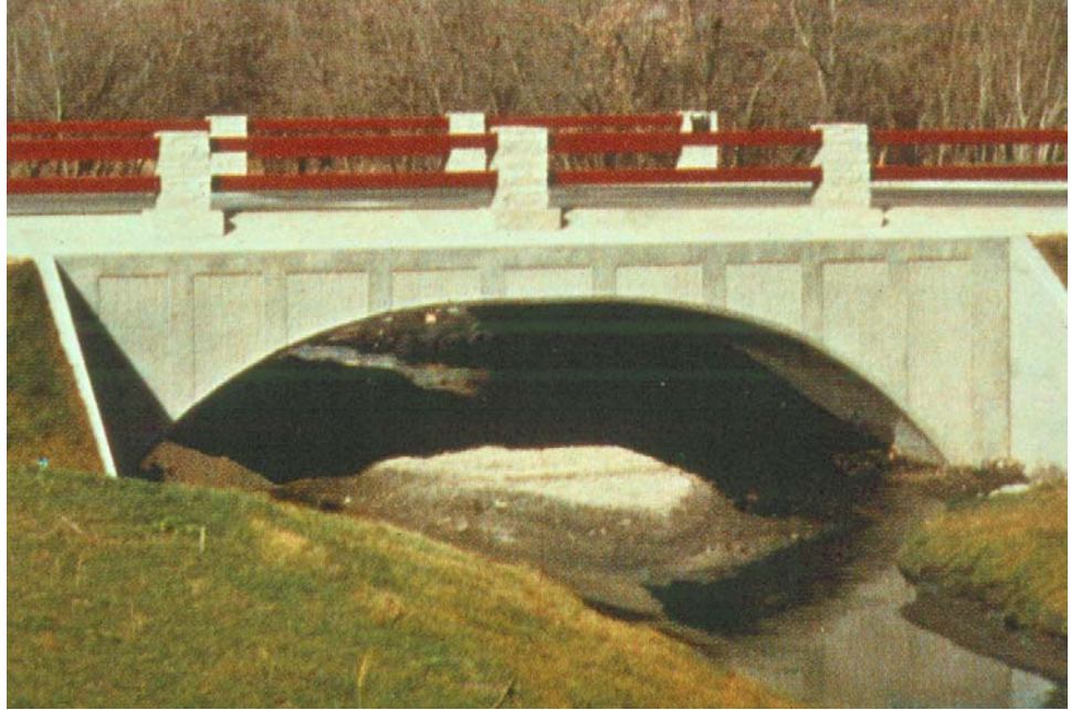
Figure 7.5.7 Concrete Arch Culvert
