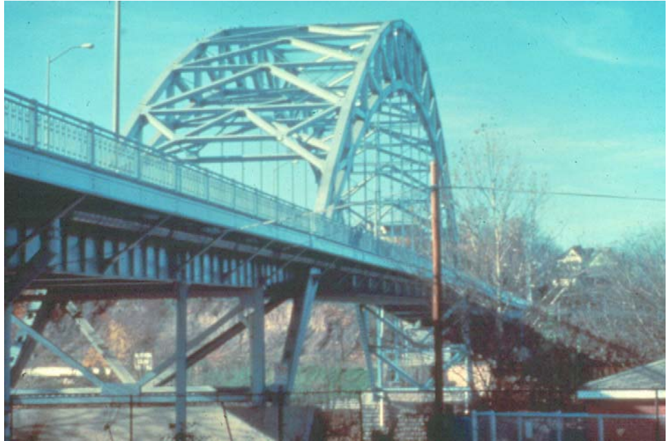
Figure P.2.56 Through Arch Bridge
