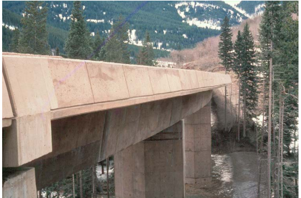
Figure 7.11.4 Typical Cast-in-place Concrete Box Girder Bridge
