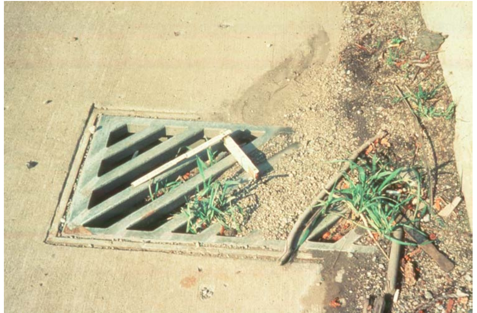
Figure 5.4.13 Bridge Deck Inlet
