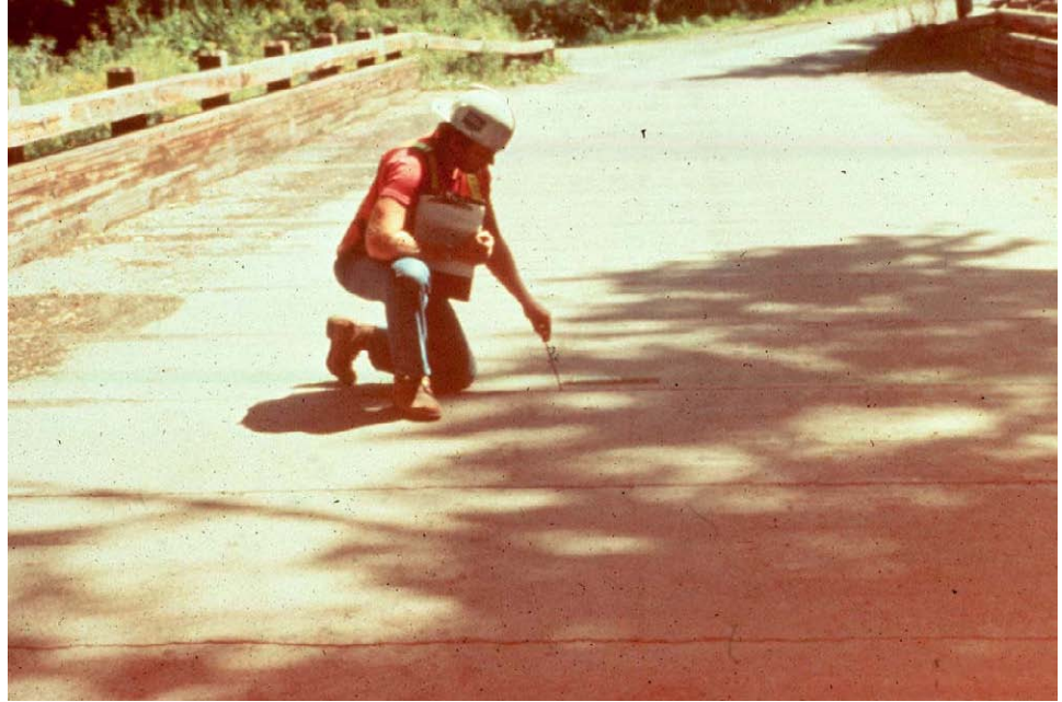
Figure 2.1.27 Inspector Probing Timber
