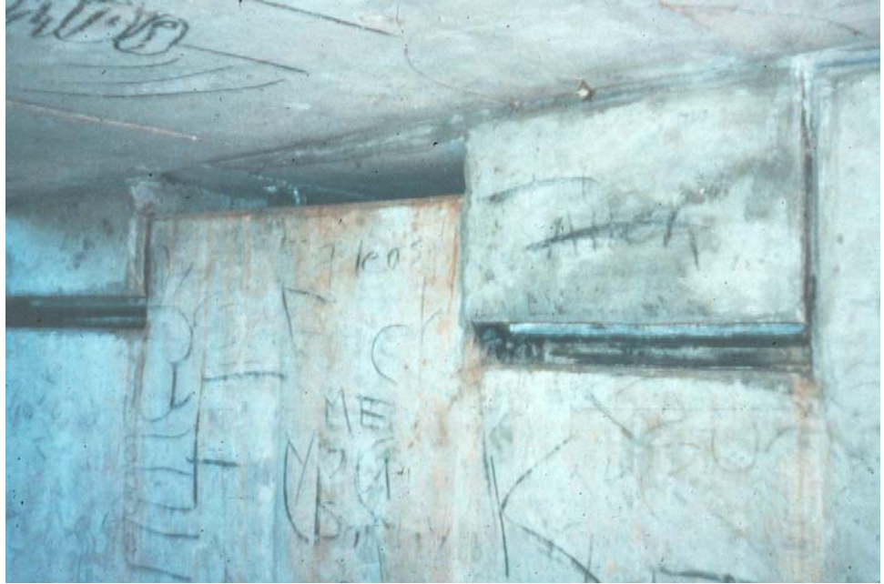
Figure 7.11.25 Bearing Area of a Cast-in-place Box Girder Bridge
