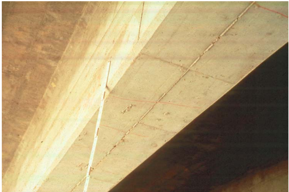
Figure 7.2.2 Typical Tee Beam with Fillet
