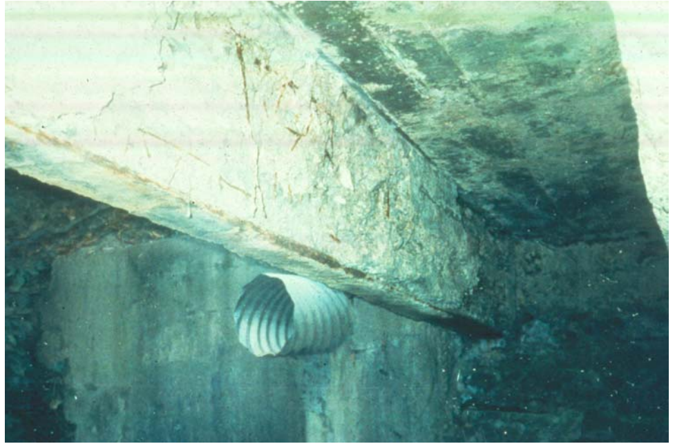
Figure 7.2.3 Concrete Encased Steel I-beam
