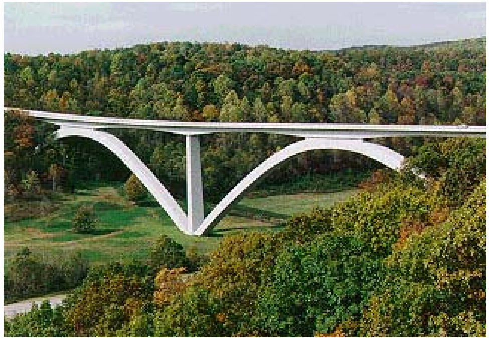
Figure 7.5.6 Precast Post-tensioned Concrete Arch without Spandrel Columns
