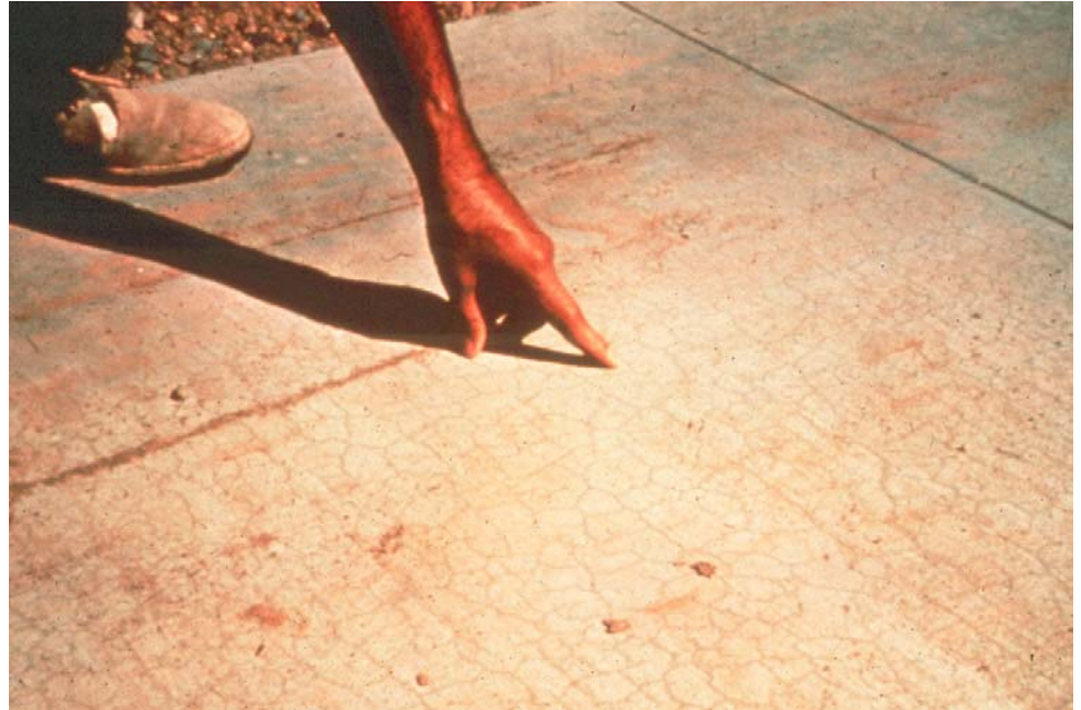
Figure 2.2.15 Pattern or Map Cracks
