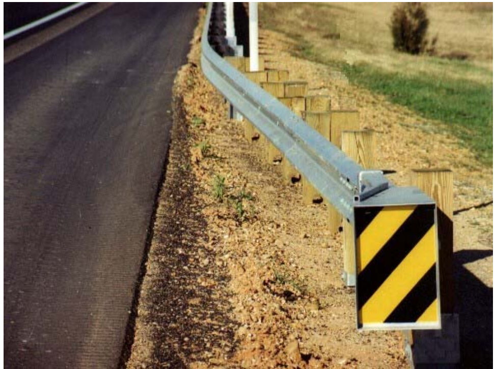
Figure 5.5.10 FLEAT-350 - FLared Energy-Absorbing Terminal
