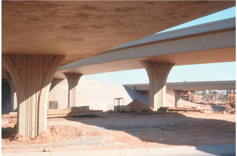
Figure 7.11.7 Box Girder Bridge Construction Using At-grade Forming
