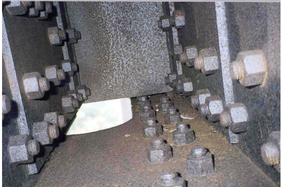
Figure 2.3.26 Black – Non-protective Oxide
