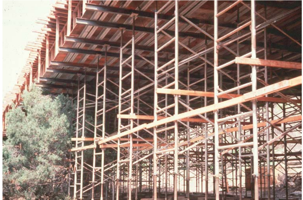
Figure 7.11.5 High Level Formwork Support Scaffolding
