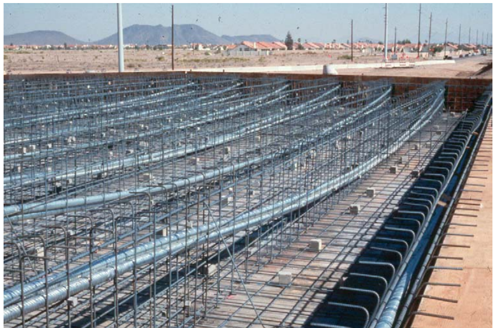
Figure 7.11.6 At-grade Formwork with Post-tensioning Ducts
