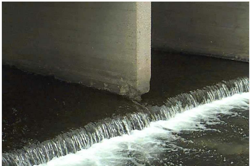
Figure P.3.20 Energy Dissipator
