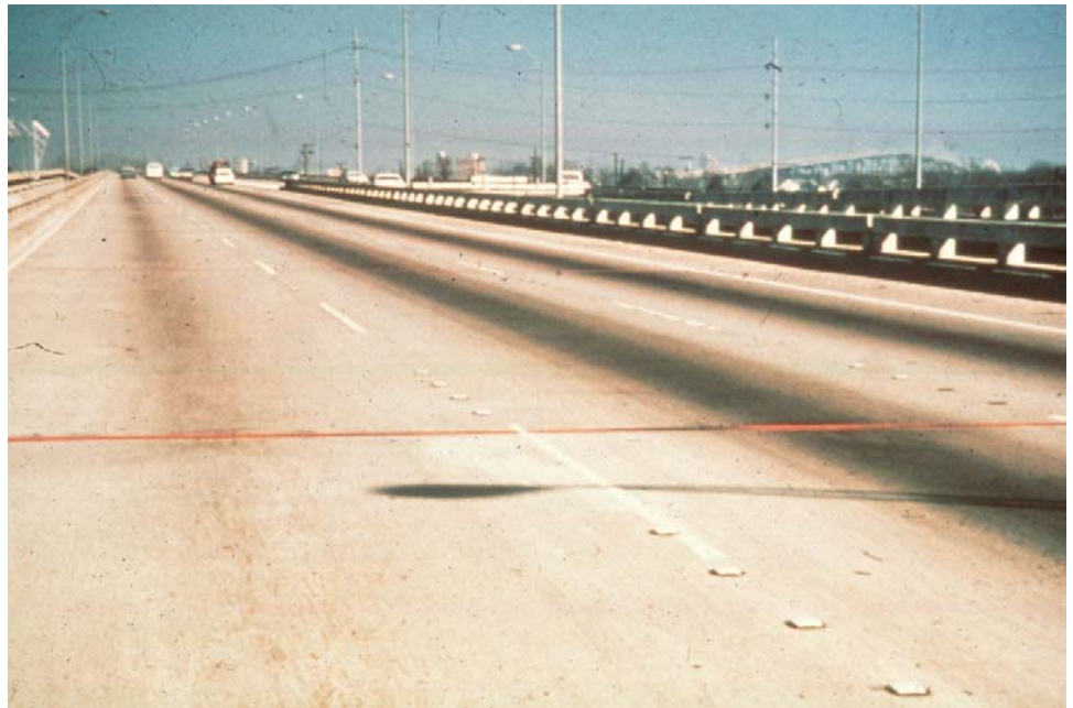
Figure P.2.25 Bridge Deck with a Smooth Riding Surface
