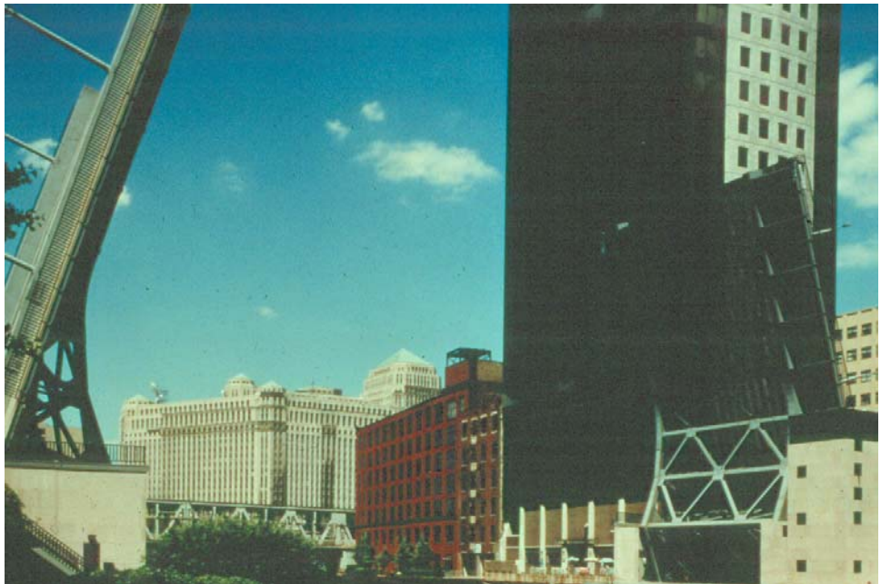
Figure P.2.59 Bascule Bridge
