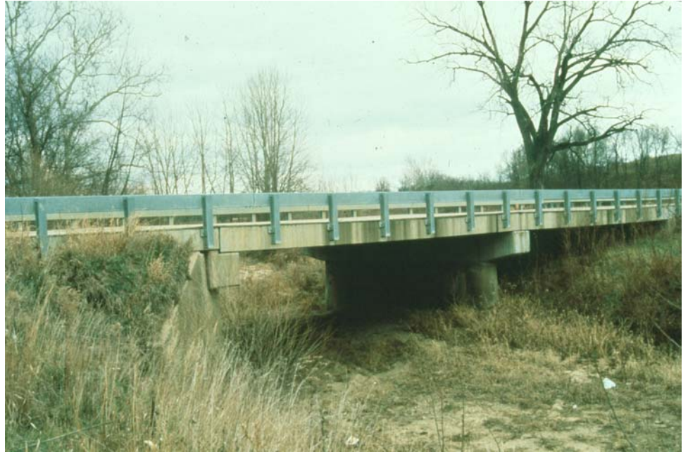
Figure 7.4.3 General View of a Precast Channel Beam Bridge
