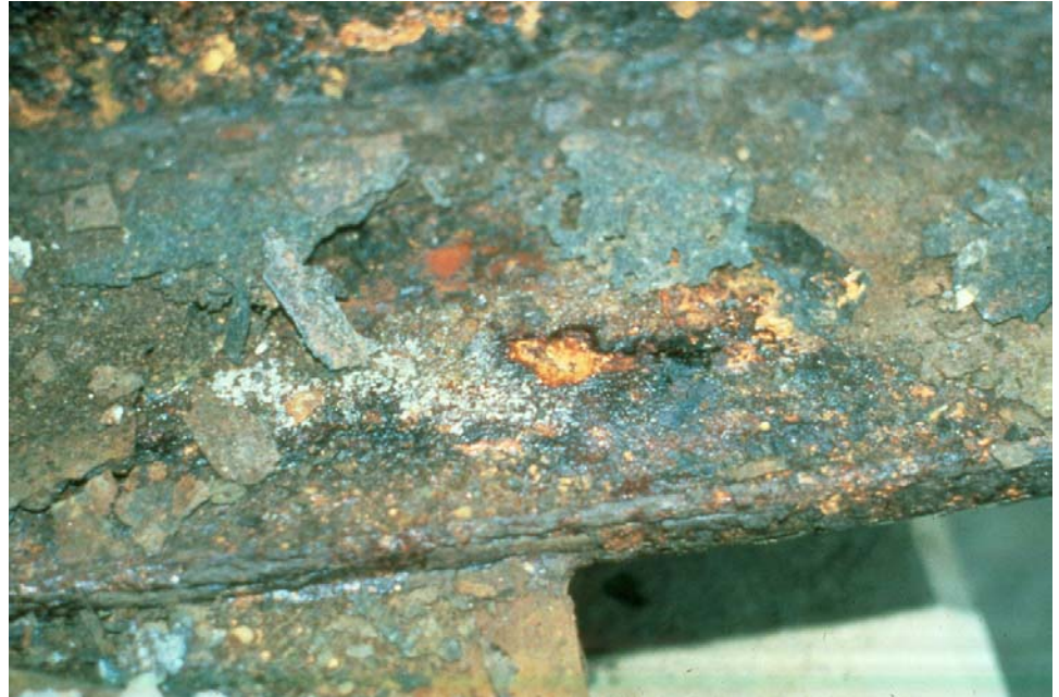
Figure 2.3.22 Color of Oxide Film is Critical in the Inspection of Weathering Steel; Dark Black Color in an Indication of Non-protective Oxide
