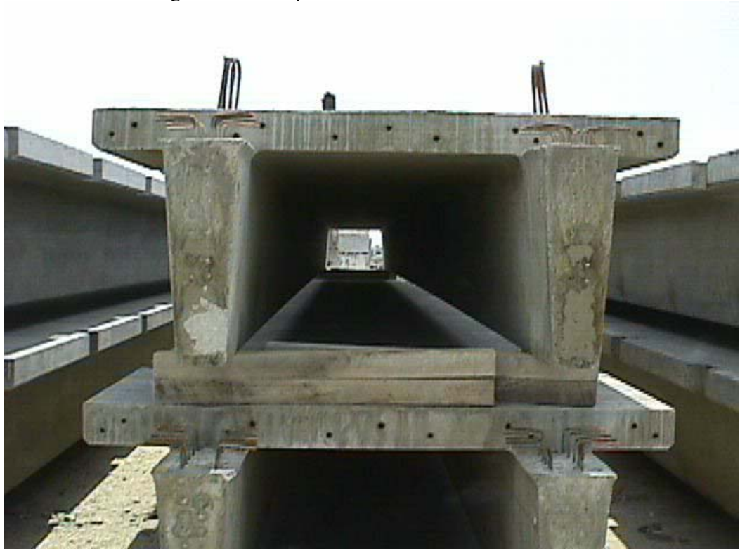
Figure 7.8.1 Typical Prestressed Double Tee Beam
