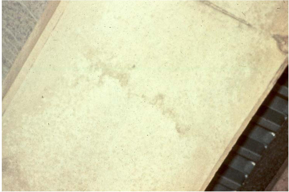
Figure 7.9.10 Flexure Crack
