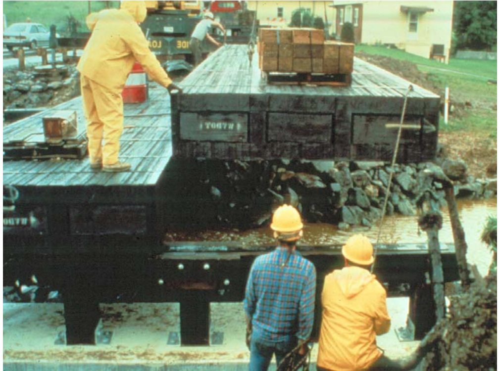
Figure 5.1.5 Structural Composite Lumber Deck Using Box Sections
