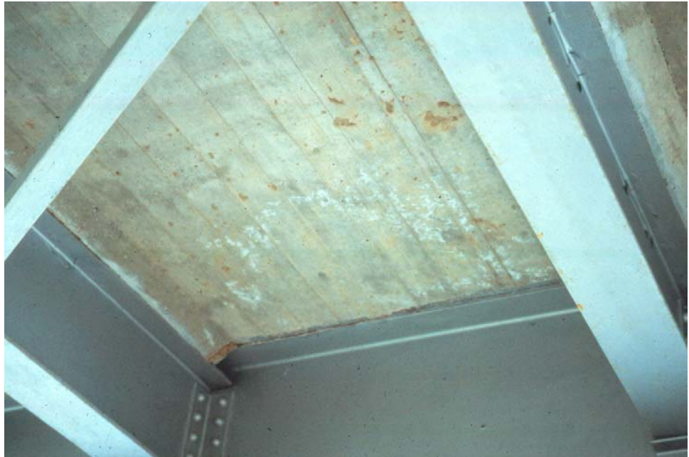
Figure P.2.26 Underside View of a Bridge Deck
