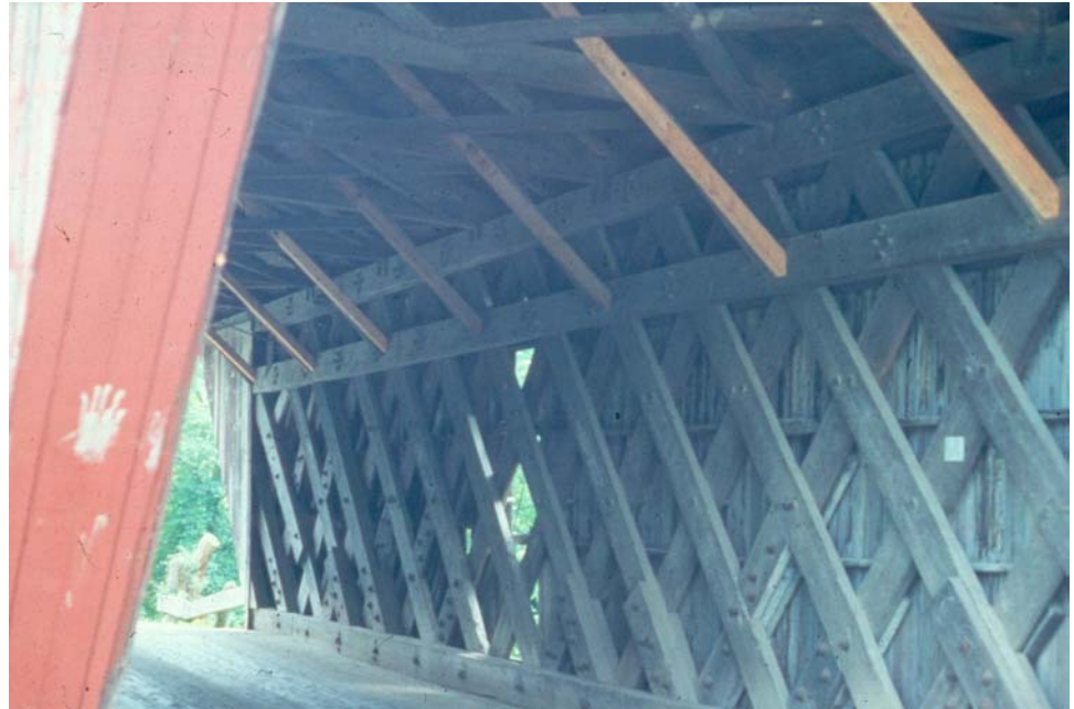
Figure 6.1.10 Town Truss Design
