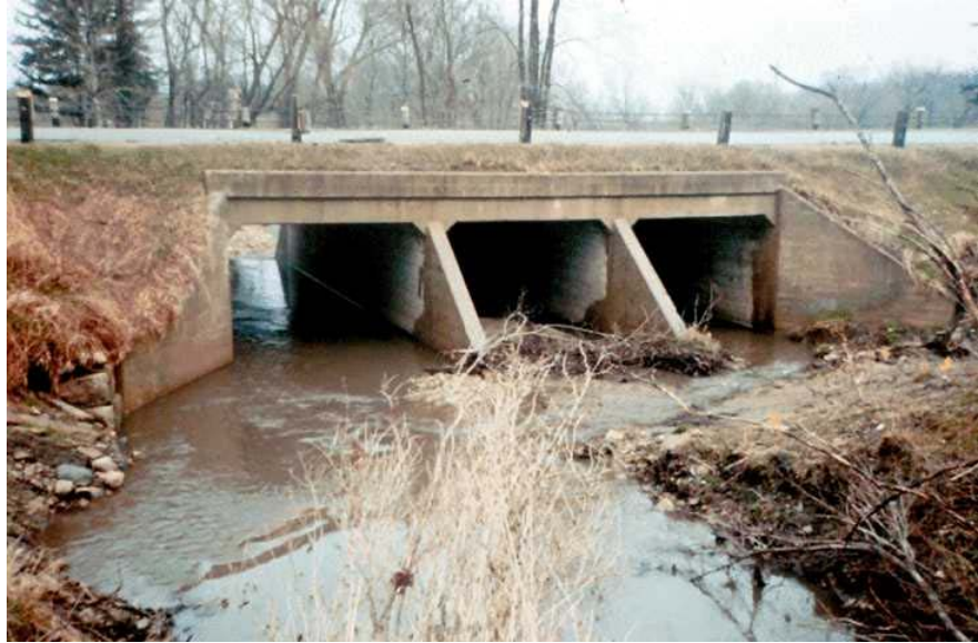
Figure P.3.11 Frame Culvert
