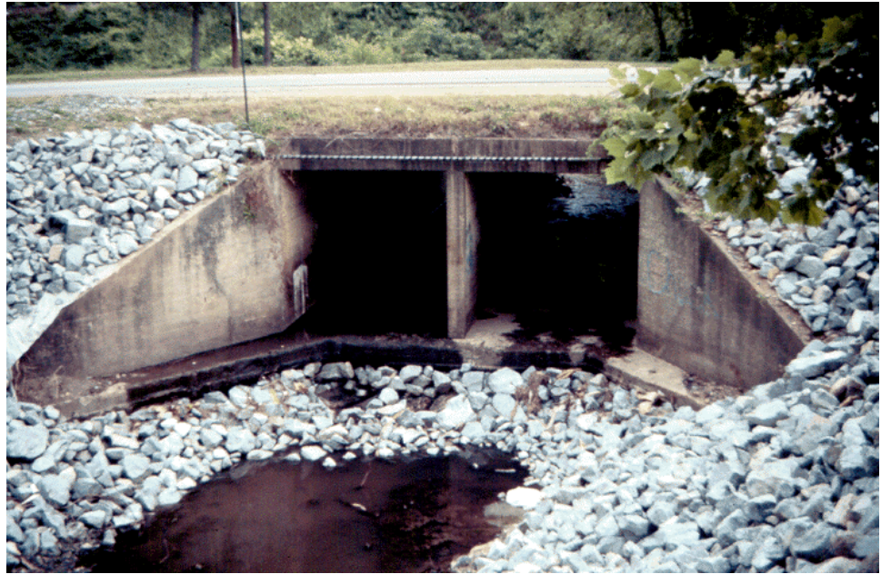
Figure 7.12.2 Multicell Concrete Box Culvert
