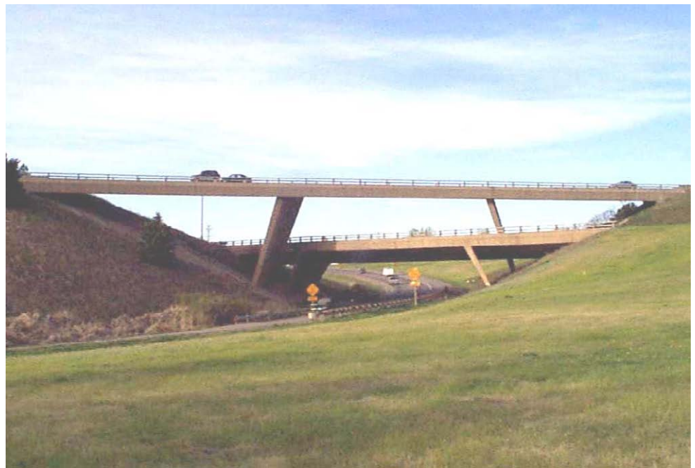
Figure 7.6.1 Three Span Concrete Rigid Frame Bridge
