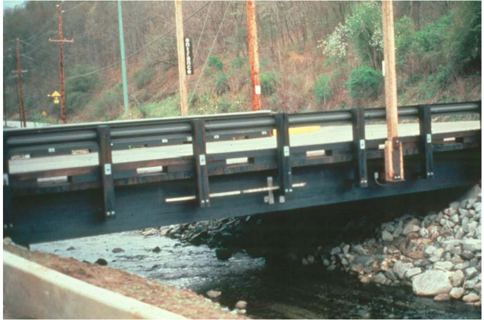
Figure 6.2.3 Elevation View of Typical Glulam Multi-beam Bridge
