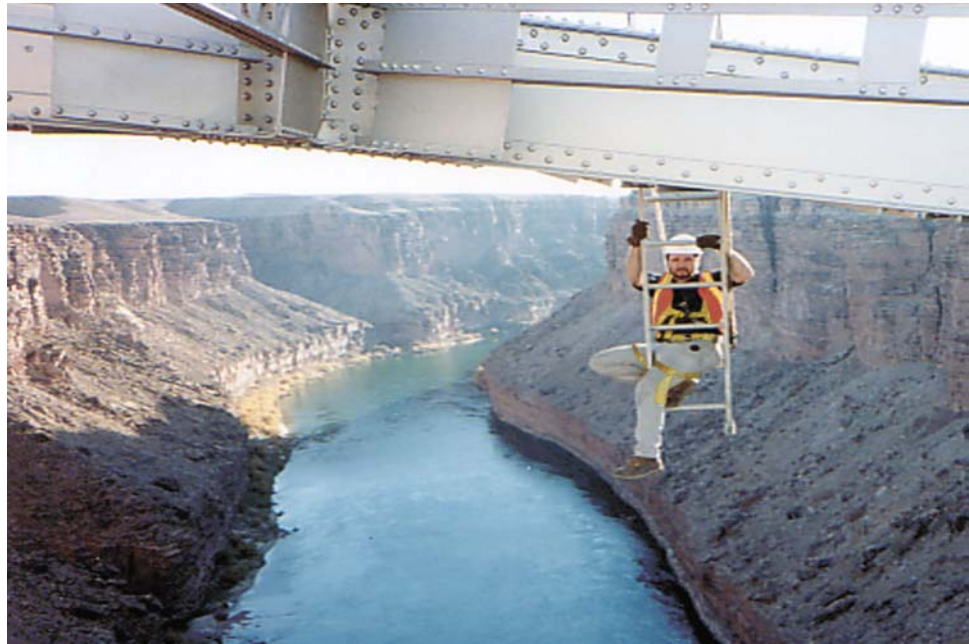
Figure 3.5.2 Use of a Hook-ladder
