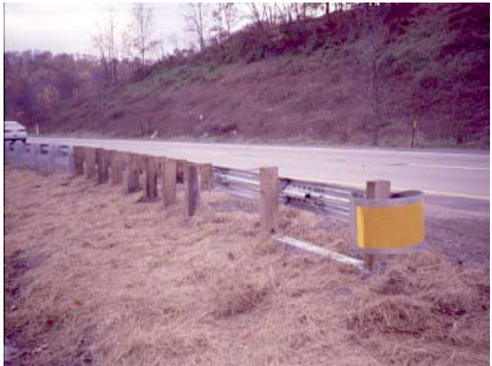
Figure 5.5.11 SRT-350 - Slotted Rail Terminal
