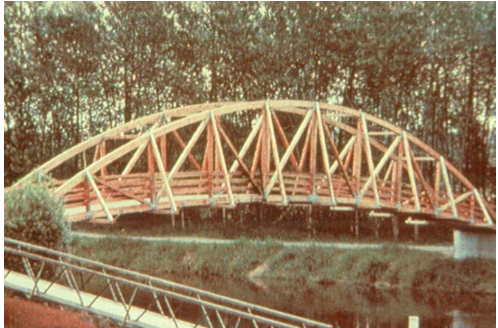
Figure 6.2.6 Bowstring Truss Pedestrian Bridge
