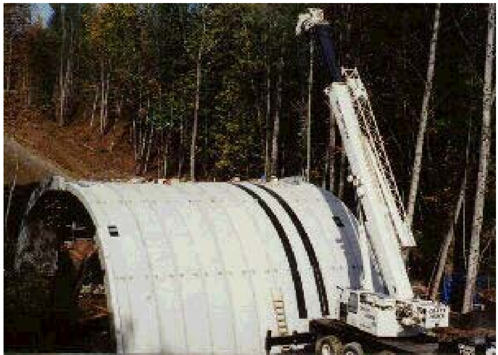
Figure 7.5.5 Precast Segmental Concrete Arch
