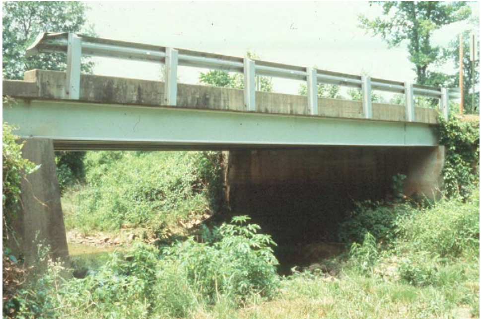
Figure 2.3.4 Rolled Shapes
