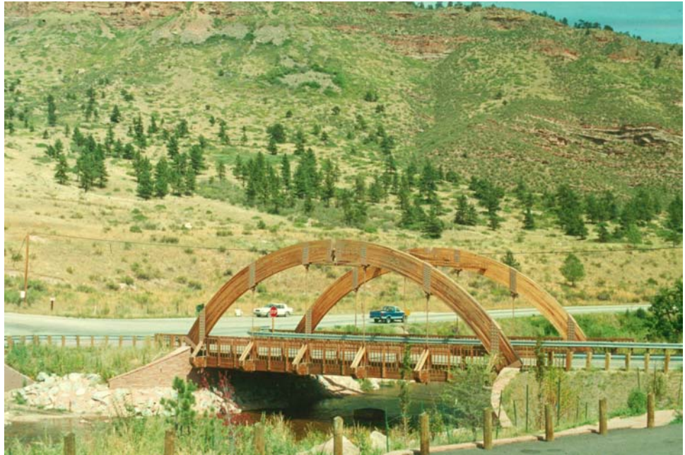
Figure 6.2.9 Glulam Arch Bridge (Colorado)
