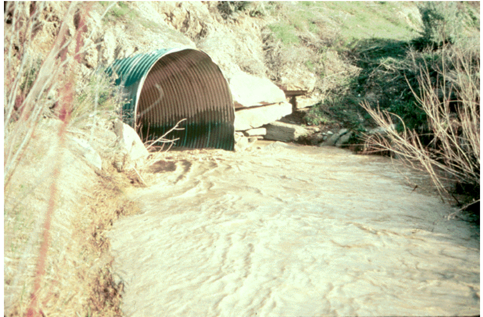
Figure P.3.15 Culvert End Projection
