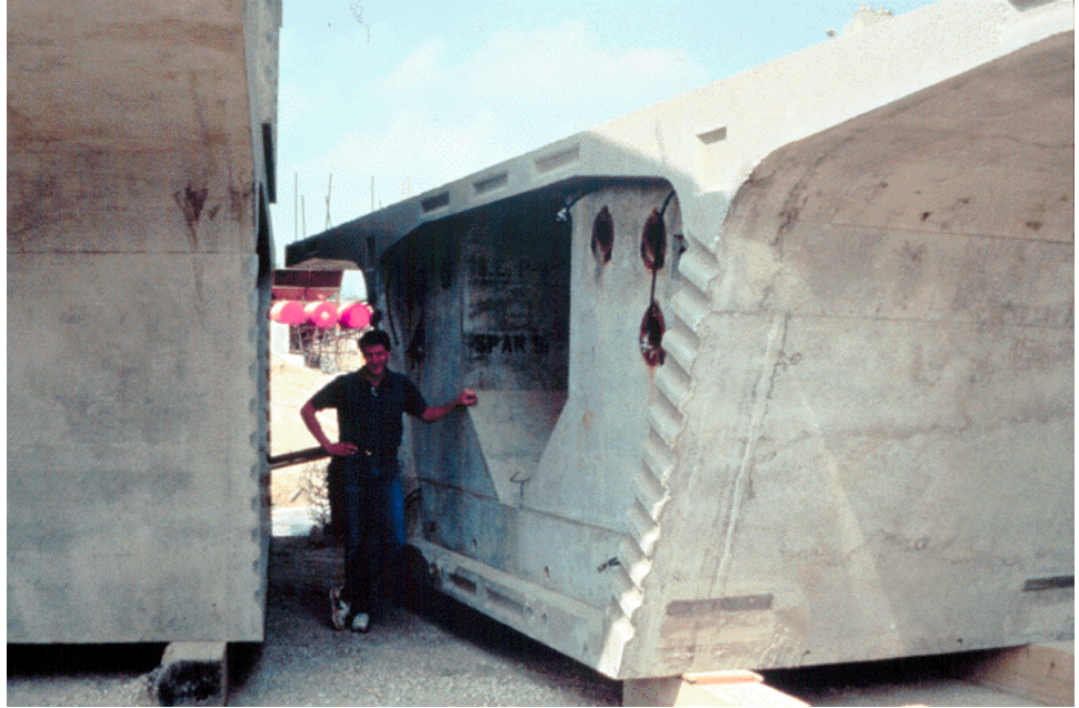
Figure 7.11.41 Box Girder Interior Diaphragm
