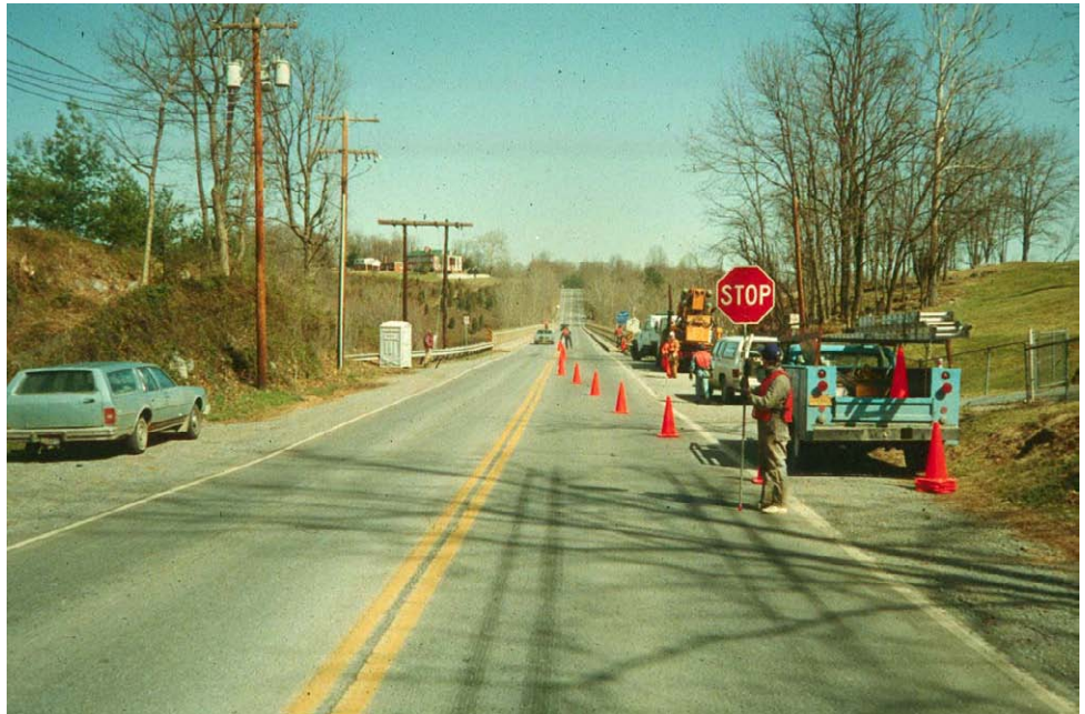
Figure 3.1.4 Traffic Control Operation
