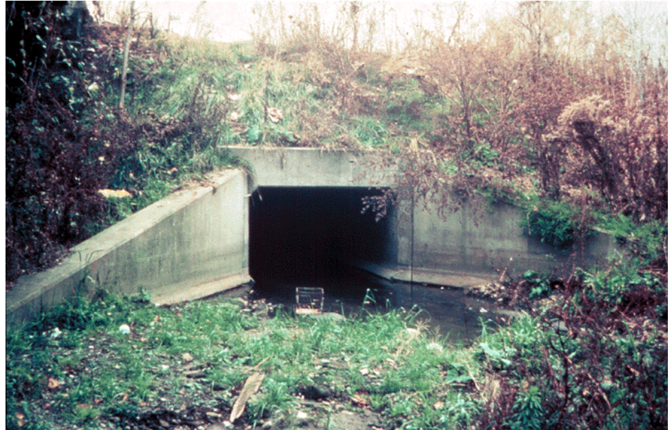
Figure P.3.9 Concrete Box Culvert
