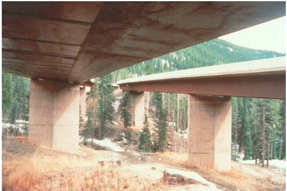
Figure P.2.52 Steel Box Girder Bridge
