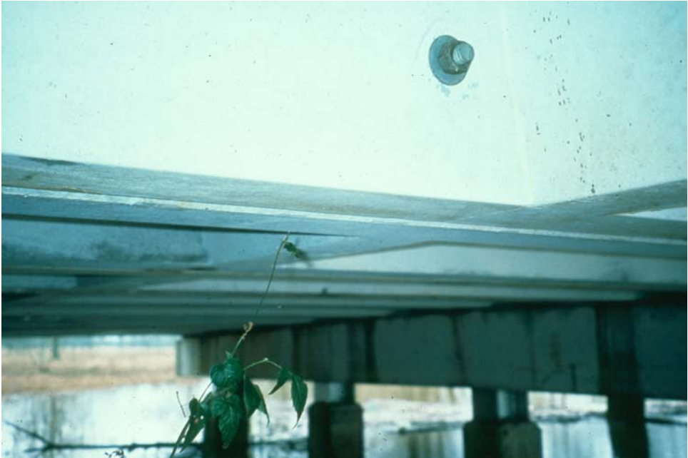
Figure 7.4.9 Stem Tie-bolts
