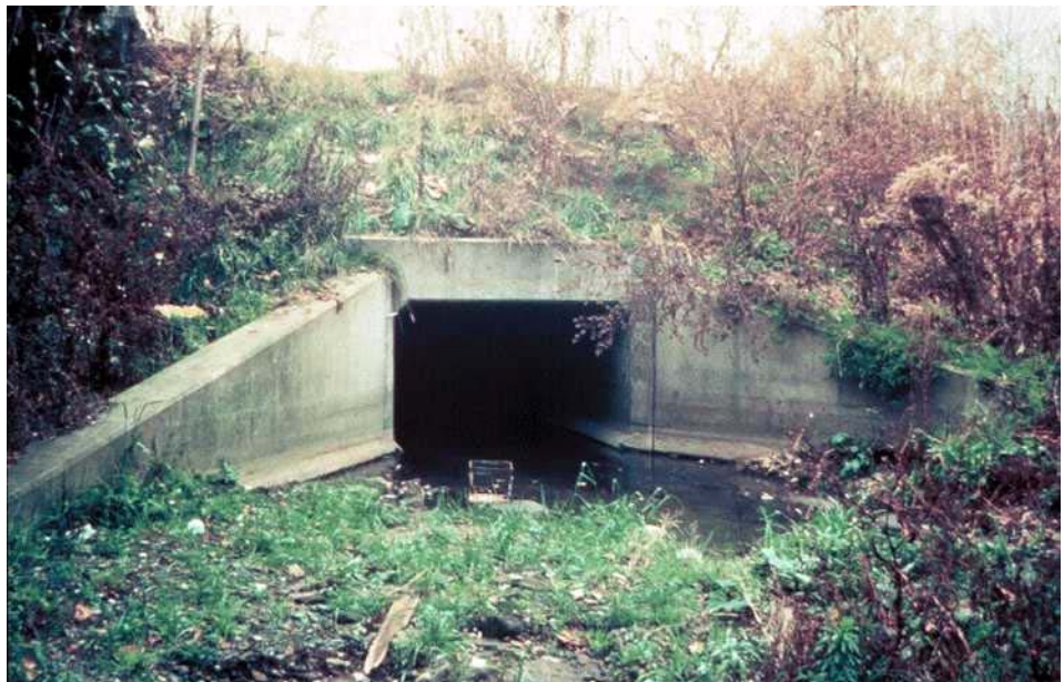
Figure P.3.18 Culvert Headwall
