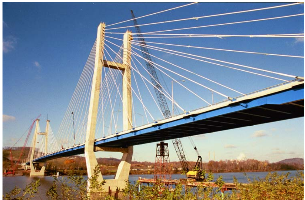
Figure P.2.17 Cable-Supported Bridge
