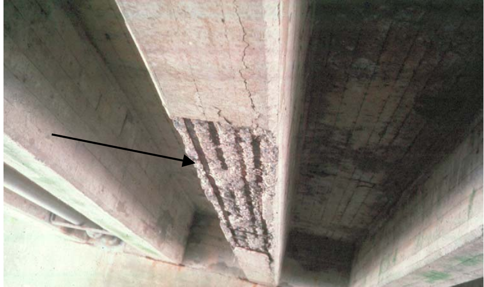
Figure 2.2.1 Concrete Member with Tensile Steel Reinforcement Showing
