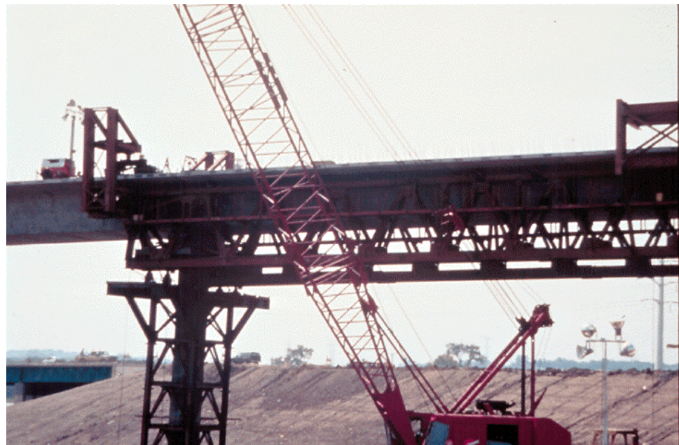
Figure 7.11.20 Span-by-span Close-up (with Erection Truss)
