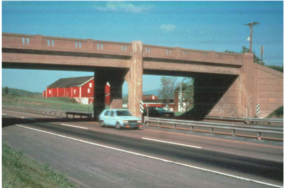
Figure 7.2.20 Tee Beam Bridge Over a Highway
