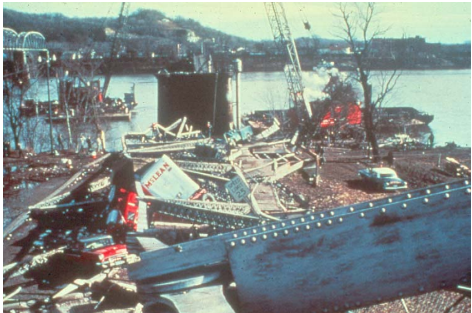
Figure 1.1.1 Collapse of the Silver Bridge
