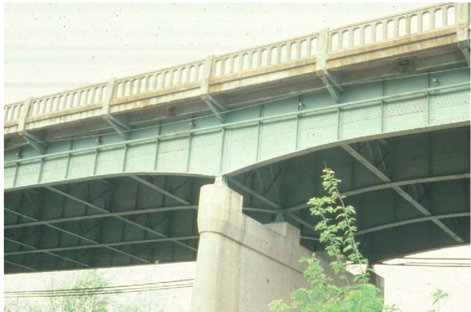
Figure 2.3.5 Built-up Shapes
