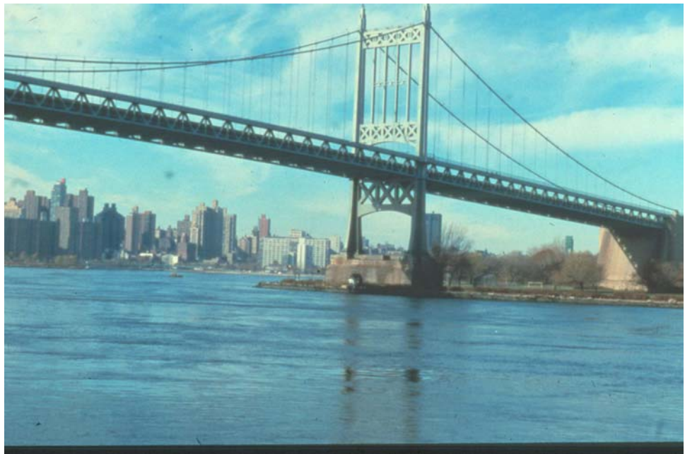
Figure P.2.57 Steel Suspension Bridge
