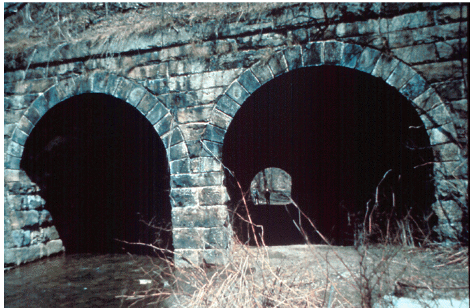
Figure P.3.13 Typical Stone Masonry Arch Culvert
