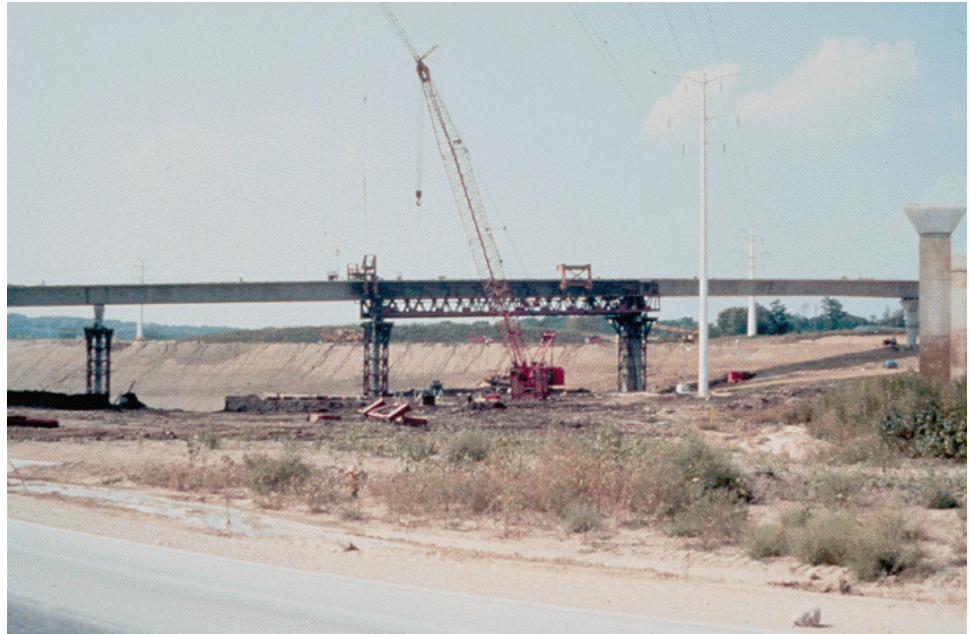
Figure 7.11.19 Span-by-Span Construction (with Erection Truss)
