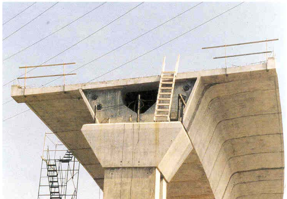
Figure 2.2.5 Post-tensioned Concrete Box Girder
