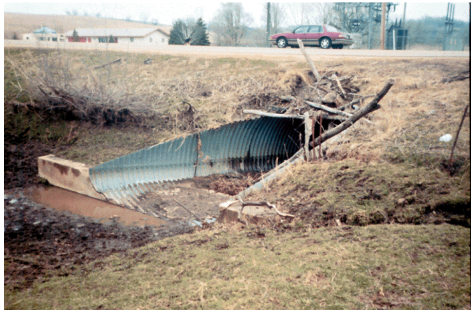
Figure P.3.16 Culvert Mitered End
