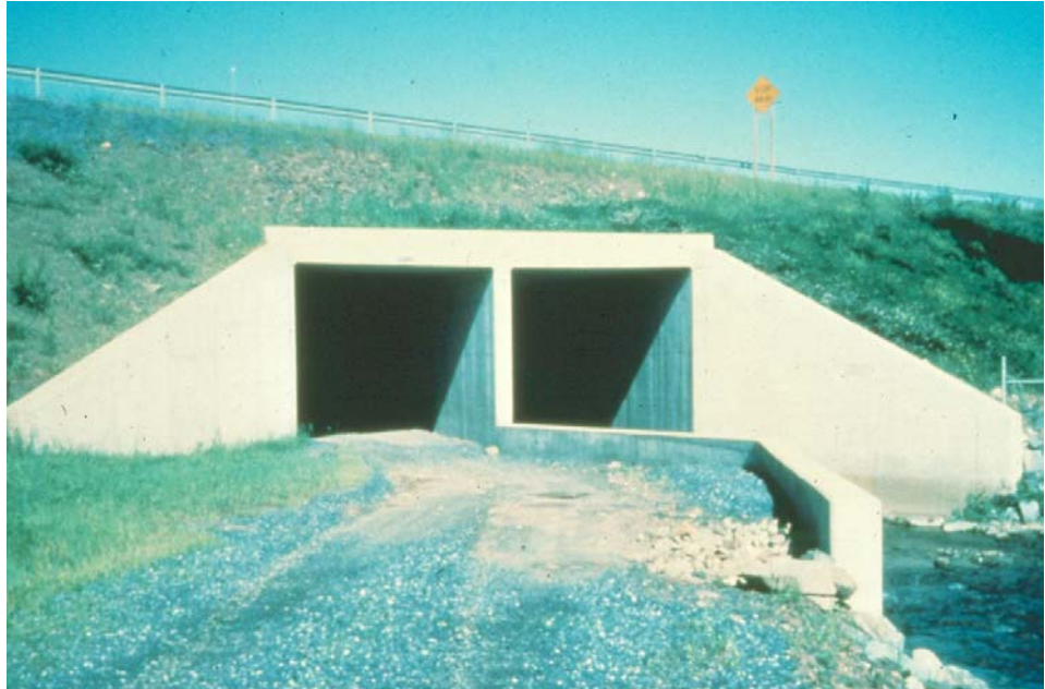
Figure P.3.17 Culvert Skewed End
