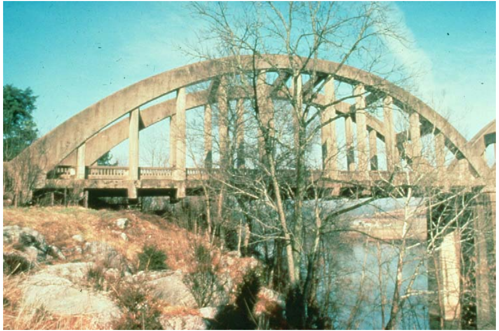
Figure 7.5.3 Concrete Through Arch Bridge
