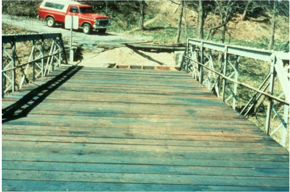
Figure P.2.29 Plank Deck
