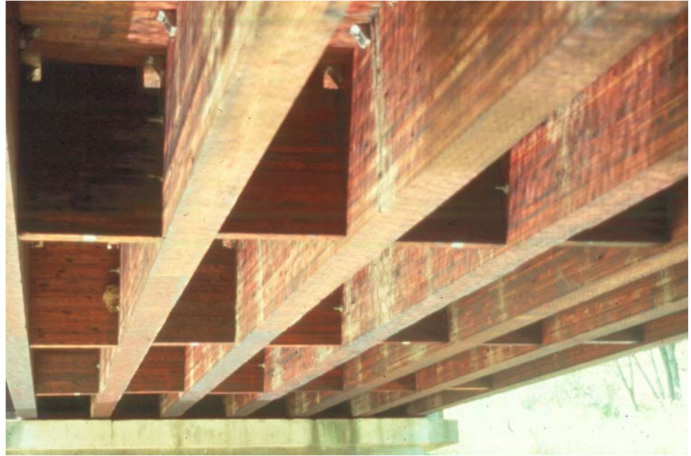
Figure 6.2.2 Underside View of a Glulam Multi-beam Bridge
