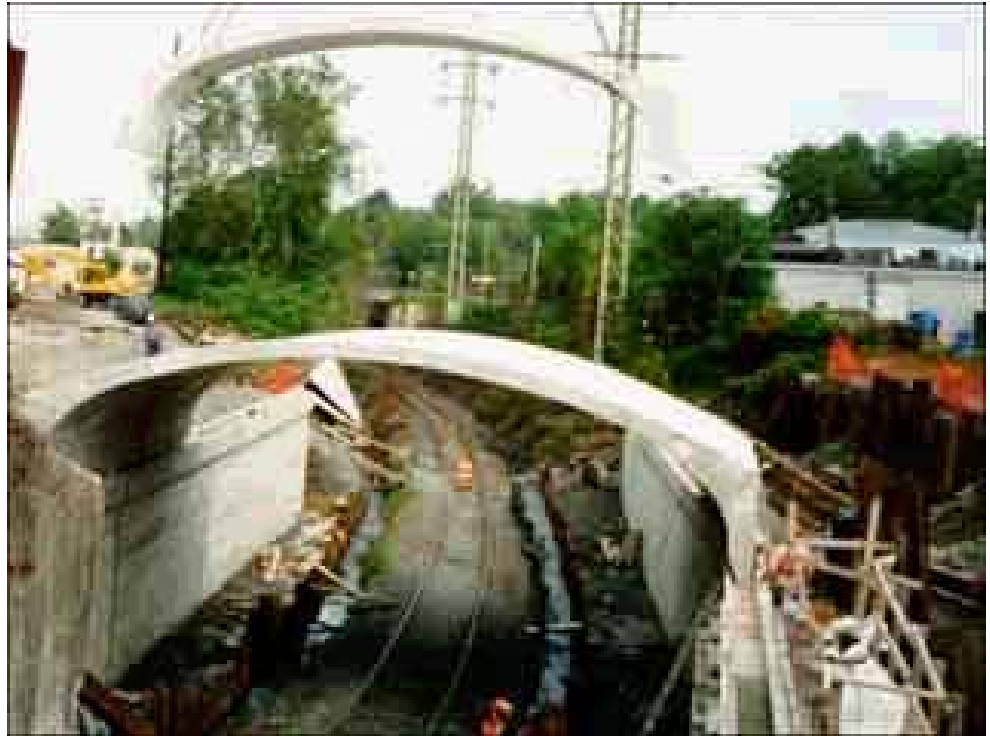
Figure 7.5.4 Precast Concrete Arch with Integral Vertical Legs
