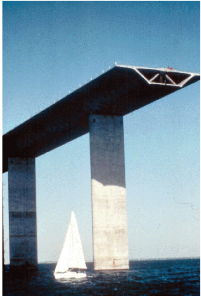
Figure 7.11.22 Progressive Placement Construction
