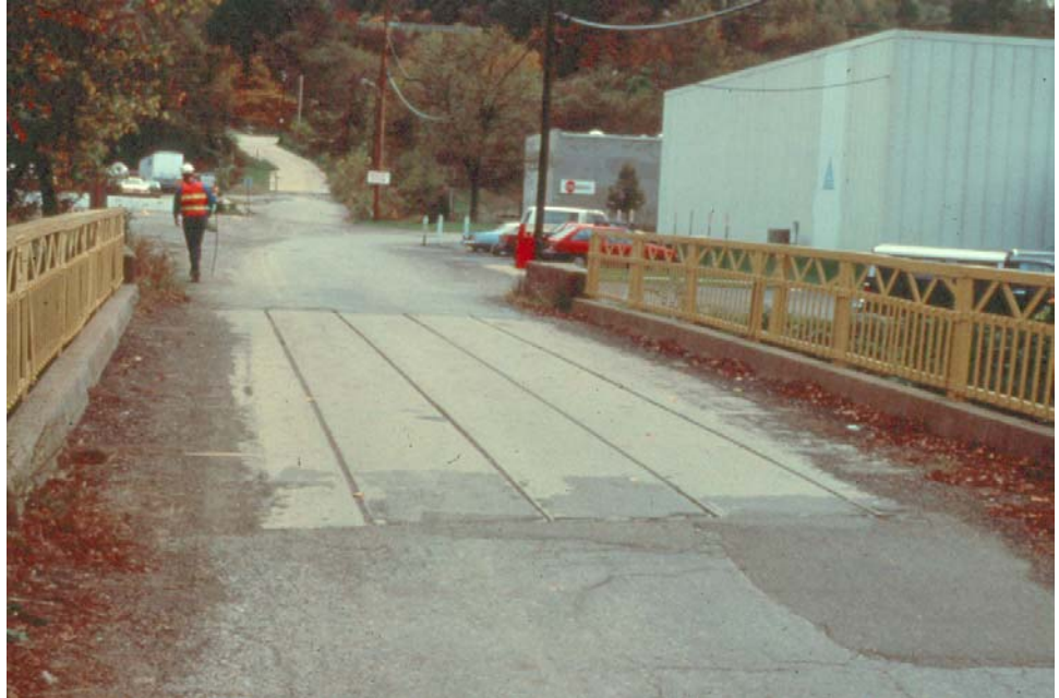
Figure 7.10.5 Adjacent Box Beams Acting as the Deck
