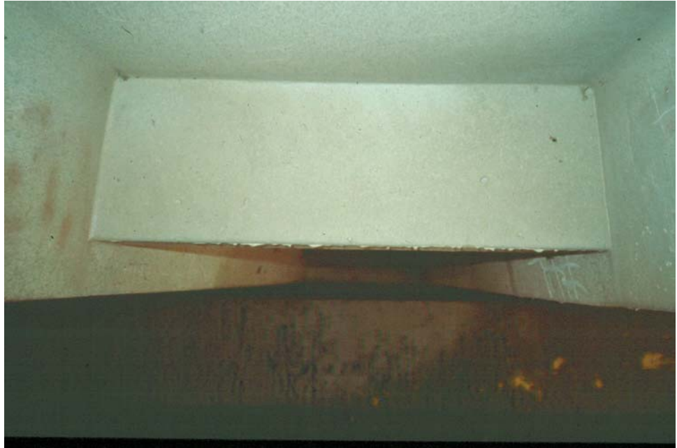
Figure 7.4.11 Close-up of Diaphragm
