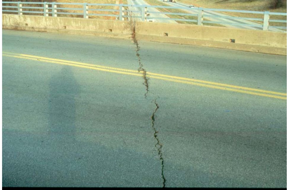
Figure 5.4.19 Asphalt Wearing Surface over an Expansion Joint
