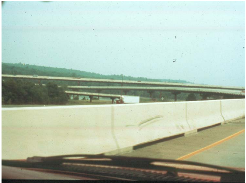
Figure 5.5.4 New Jersey Barrier
