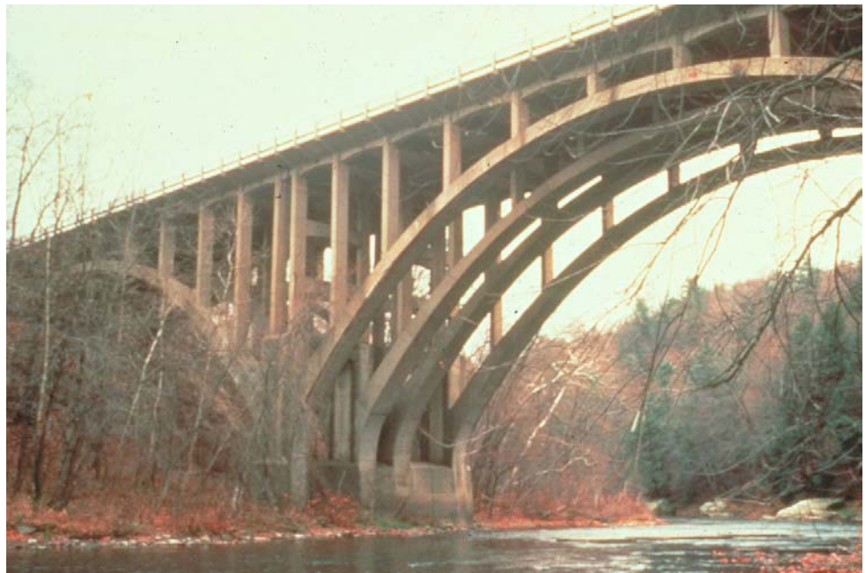
Figure P.2.55 Deck Arch Bridge
