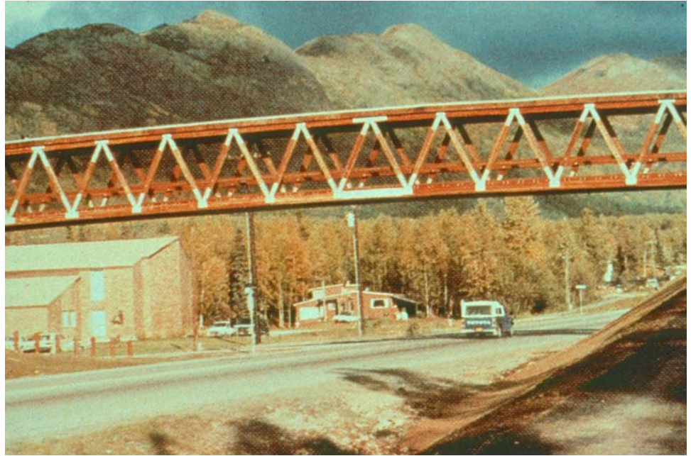
Figure 6.2.7 Parallel Chord Truss Pedestrian Bridge (Eagle River, Alaska)
