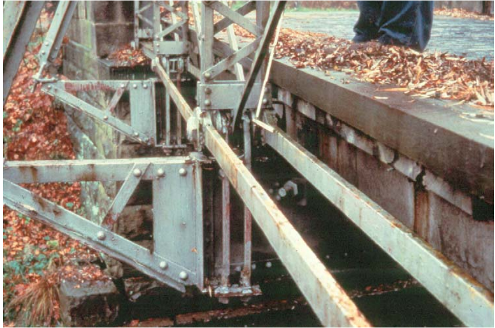
Figure P.2.19 Pin-Connected Truss Members
