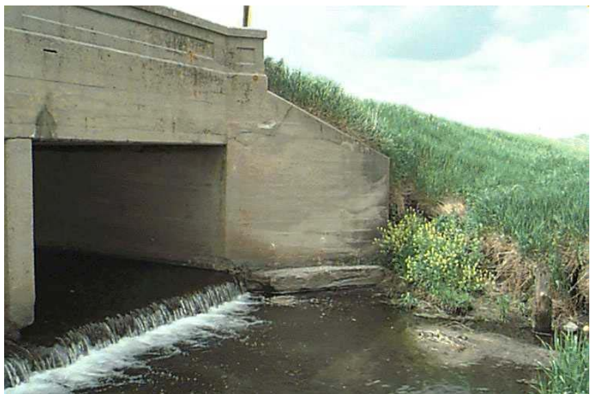
Figure 7.12.9 Cast in Place Concrete Box Culvert Outlet
