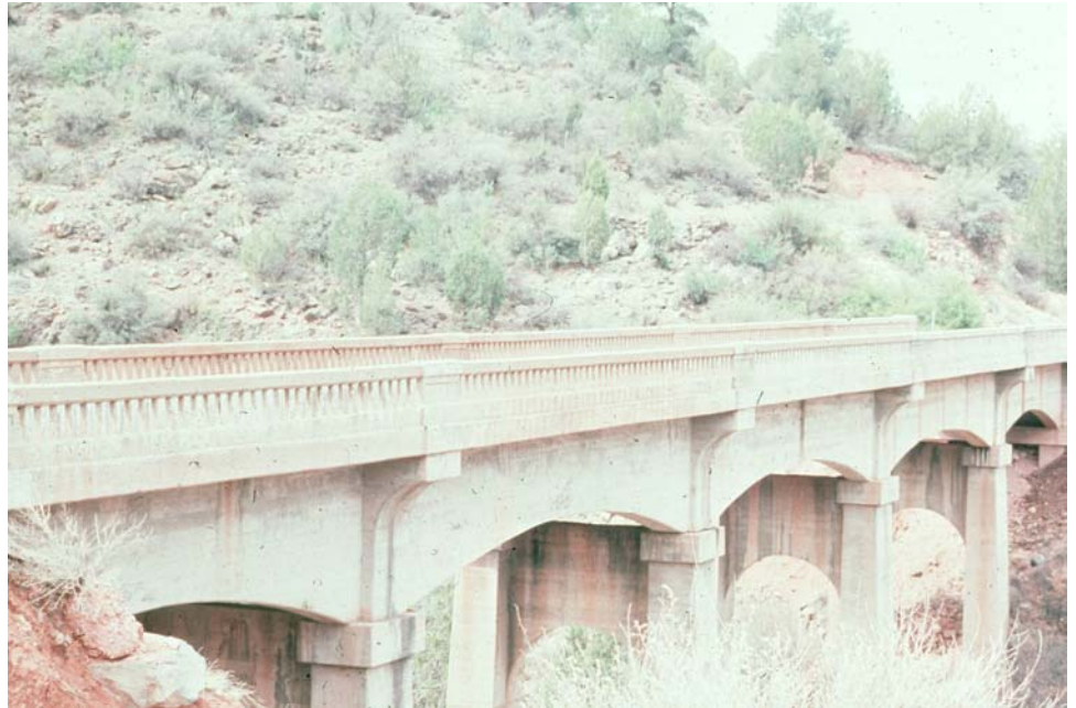
Figure 7.3.1 Concrete Deck Girder Bridge
