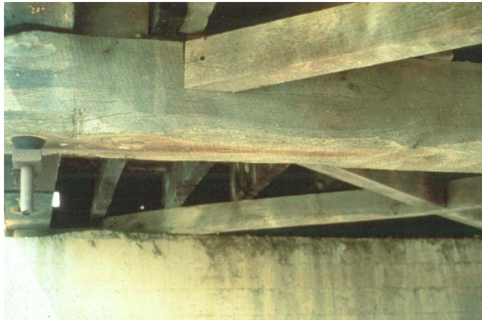
Figure 2.1.17 Hanger Connection on a Timber Floorbeam
