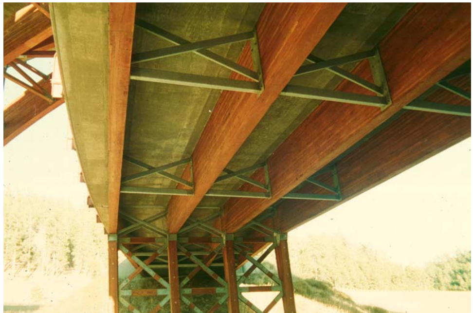
Figure 6.2.17 Glulam Beams with Numerous Fastener Locations
