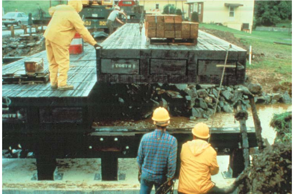
Figure 6.3.8 Stress-Laminated Timber Box Beam Bridge Being Erected
