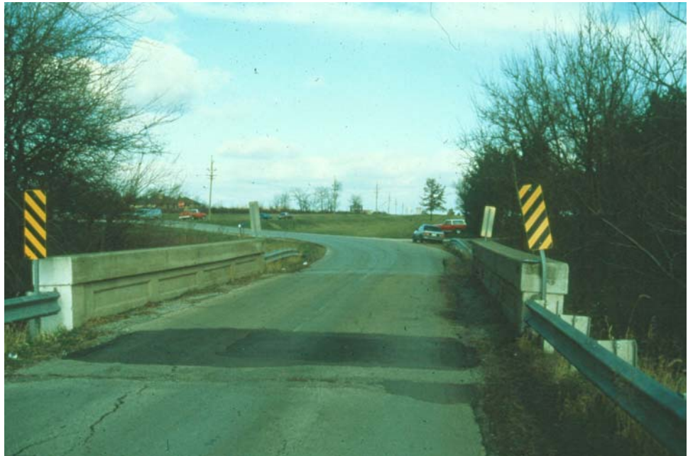
Figure 7.3.2 Concrete Through Girder Bridge
