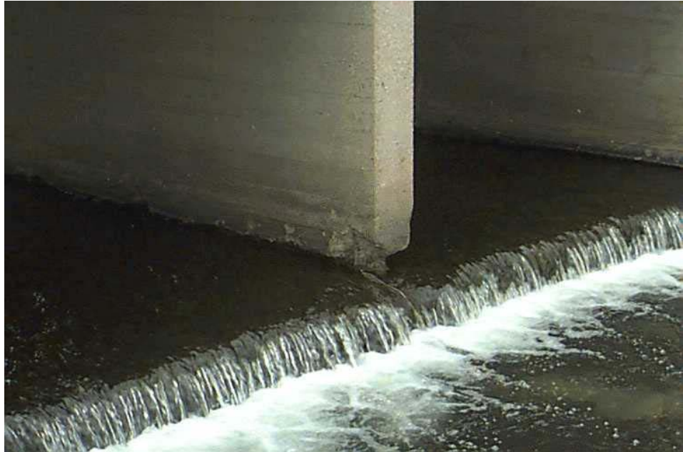
Figure P.3.34 Energy Dissipater
