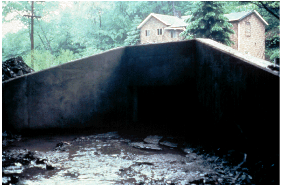
Figure P.3.32 Culvert Headwall
