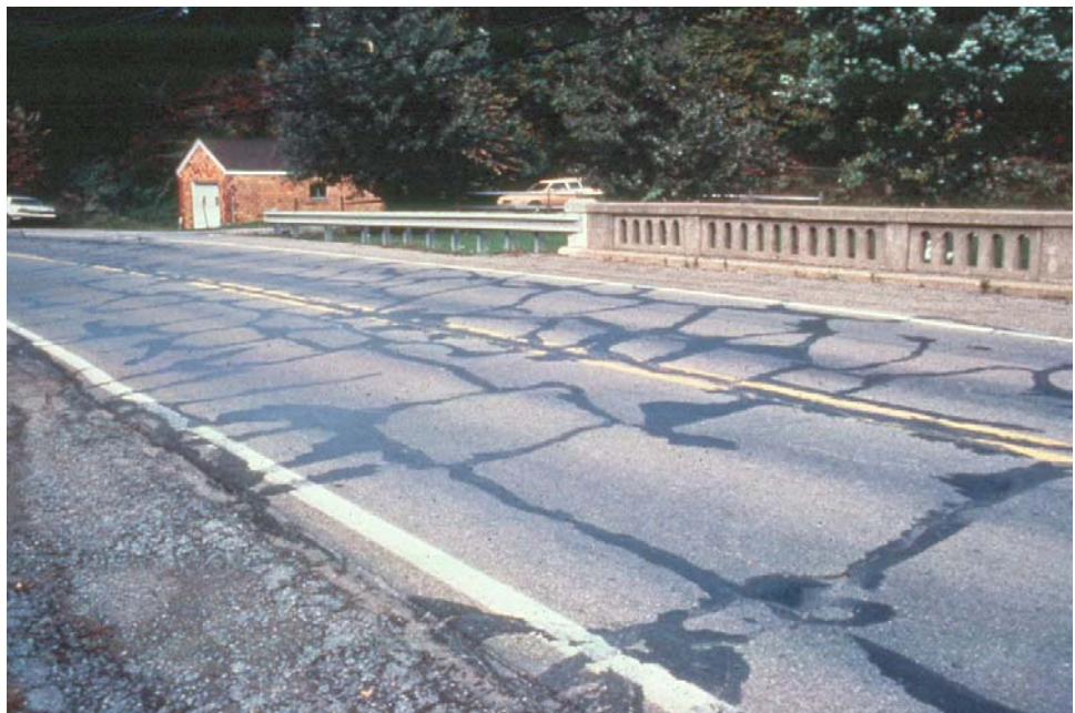
Figure 7.2.17 Asphalt Covered Tee Beam Slab
