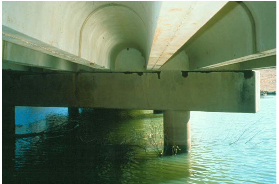
Figure 7.4.4 Underside View of a Cast-in-Place Channel Beam Bridge
