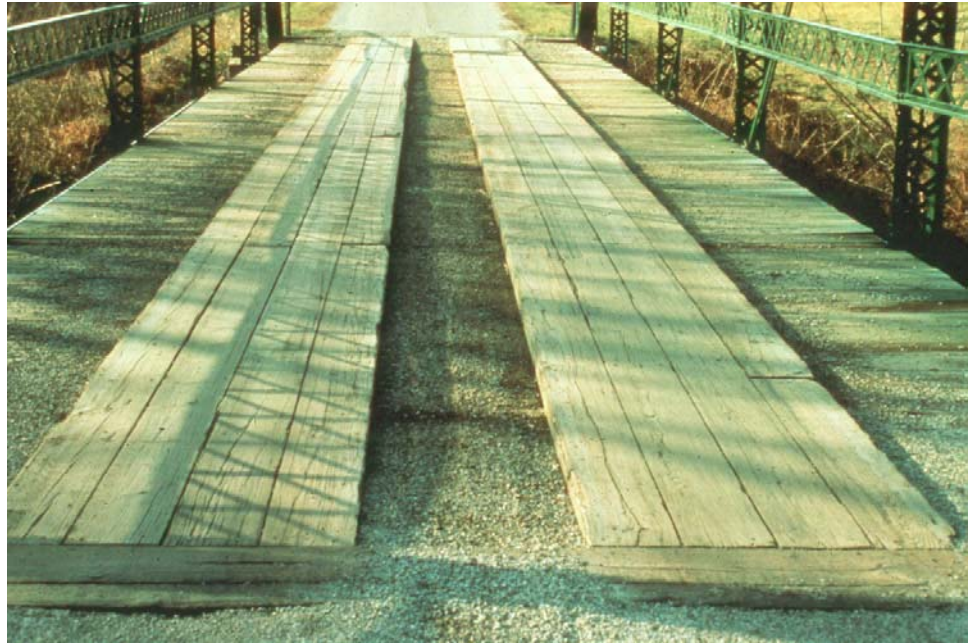
Figure 5.1.6 Timber Wearing Surface on a Timber Deck
