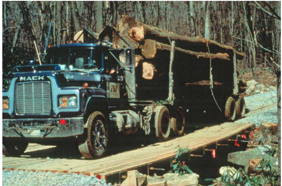
Figure 6.3.1 Stressed-Laminated Timber Deck Bridge Carrying a 90,000-Pound Logging Truck (Source: Barry Dickson, West Virginia University)
