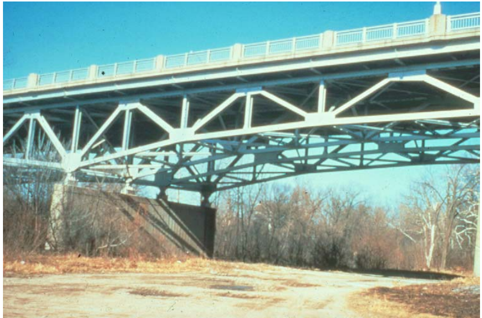
Figure P.2.53 Deck Truss Bridge
