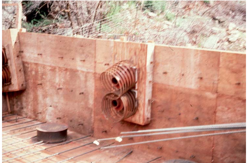
Figure 7.11.11 Formwork with Post-tensioning Duct End Fittings and Spiral Anchorage Reinforcement
