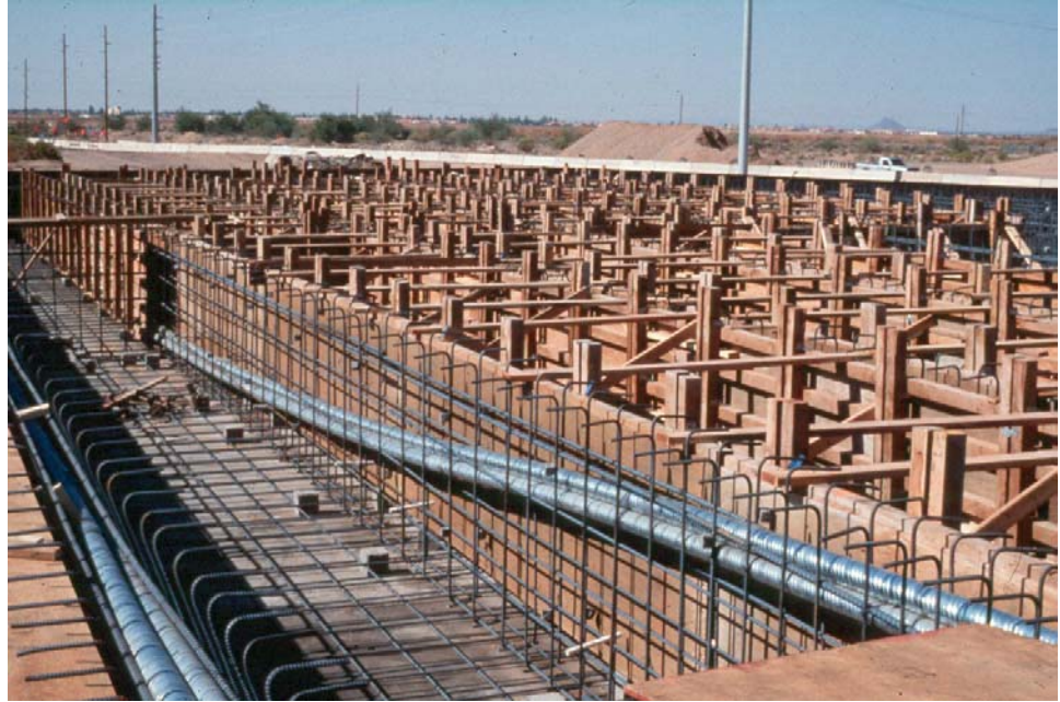
Figure 7.11.29 Post-tensioning Tendon Duct
