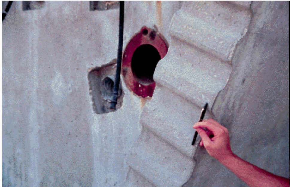
Figure 7.11.39 Close-up View of Box Girder Shear Keys
