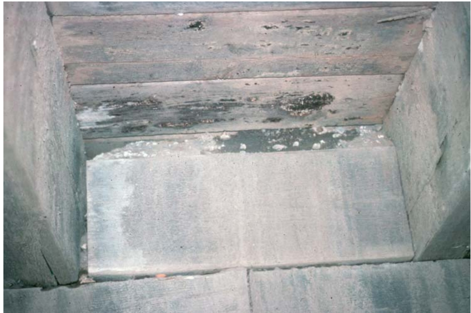
Figure 6.1.14 Typical Timber End Diaphragm
