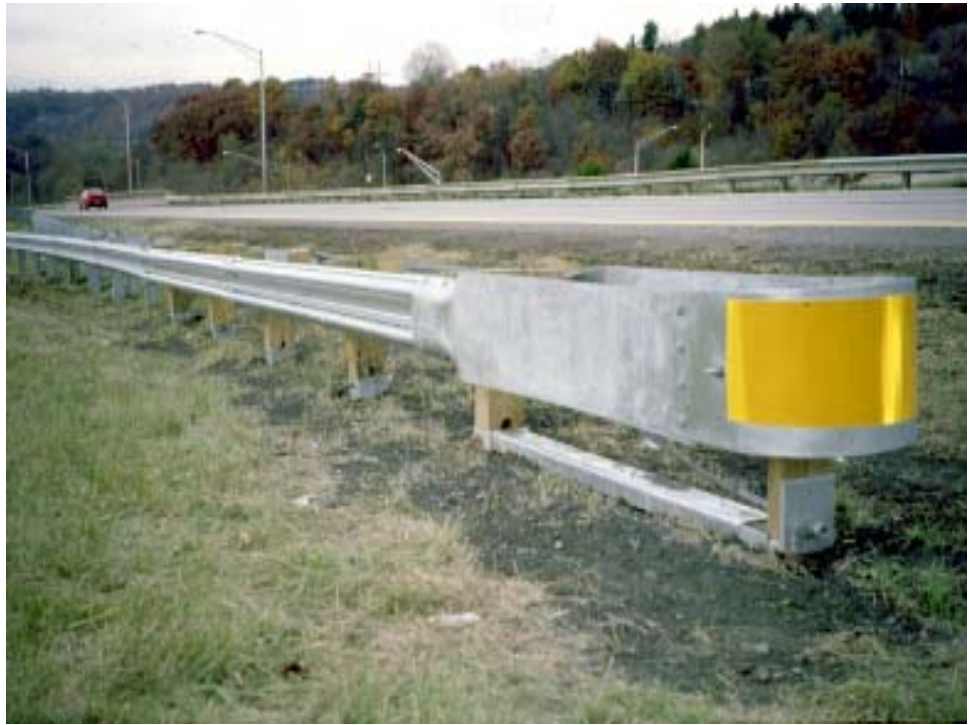
Figure 5.5.15 CAT – Crash-cushion Attenuating Terminal
