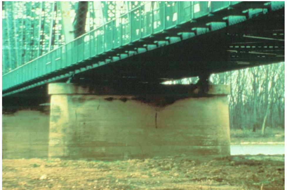
Figure P.2.70 Solid Shaft Pier
