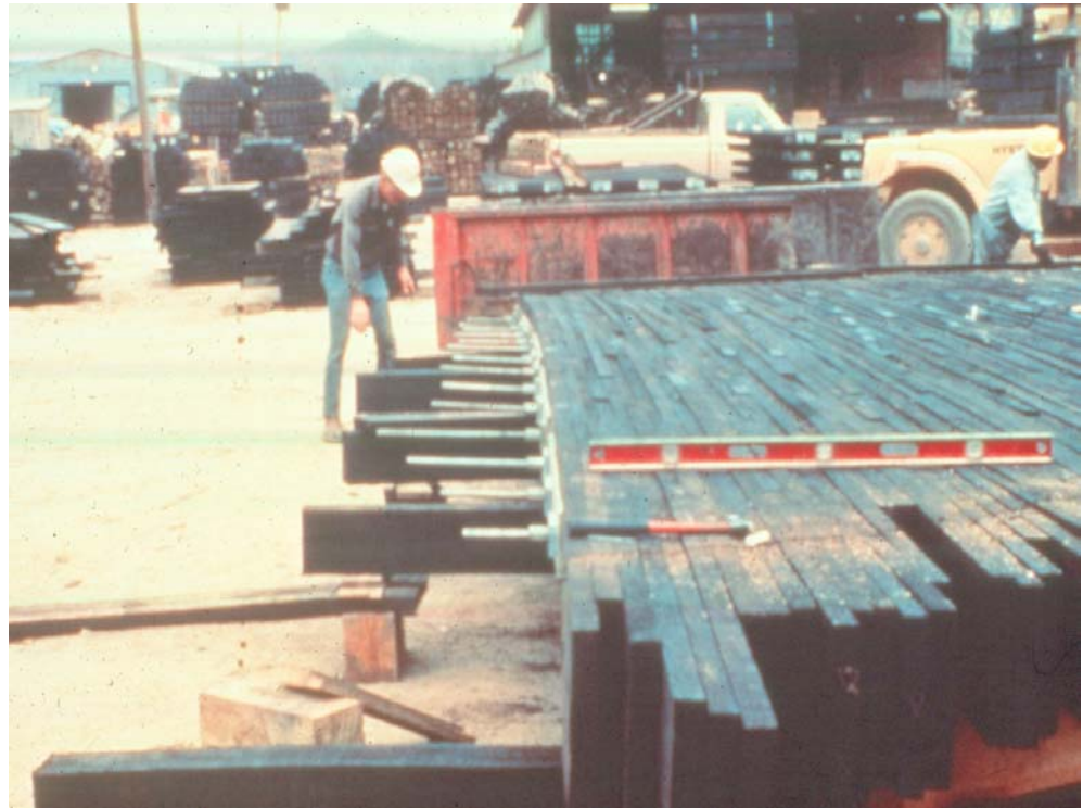
Figure 5.1.4 Stressed-laminated Deck
