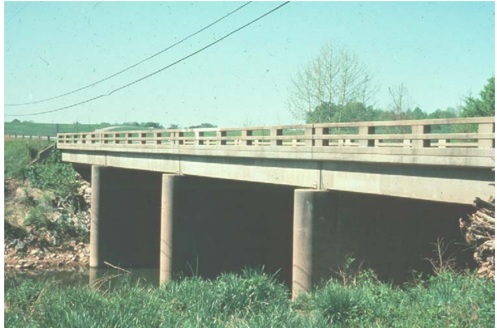
Figure 7.10.1 Typical Box Beam Bridge
