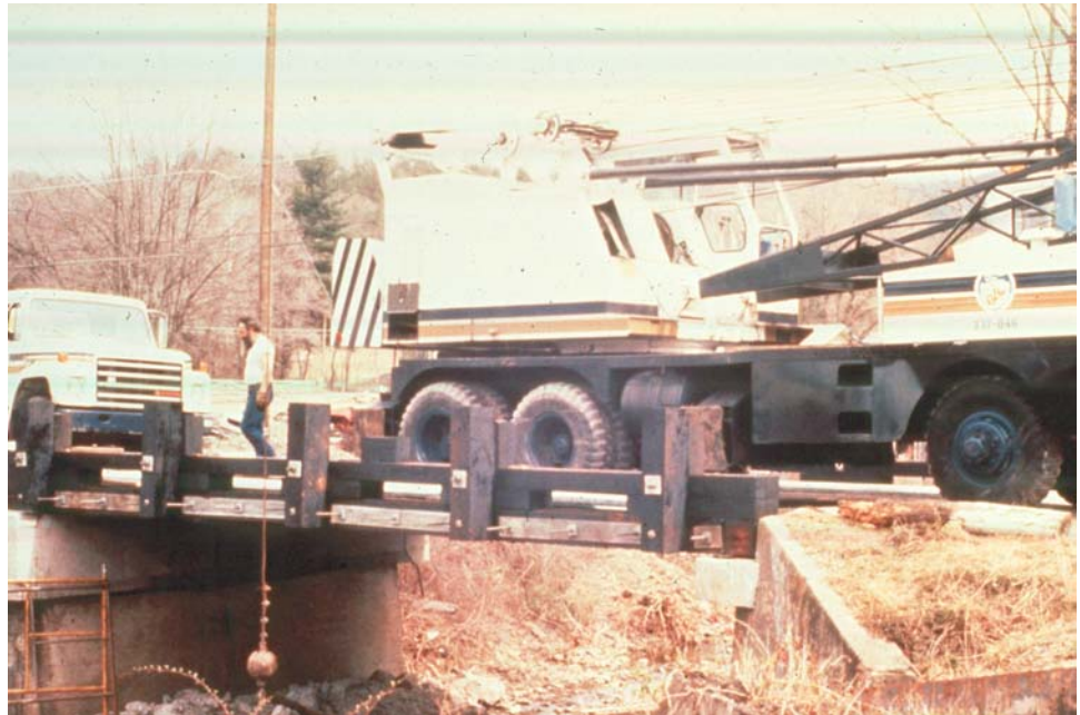
Figure 6.3.3 Solid Sawn Stress-Laminated Deck/Slab Bridge
