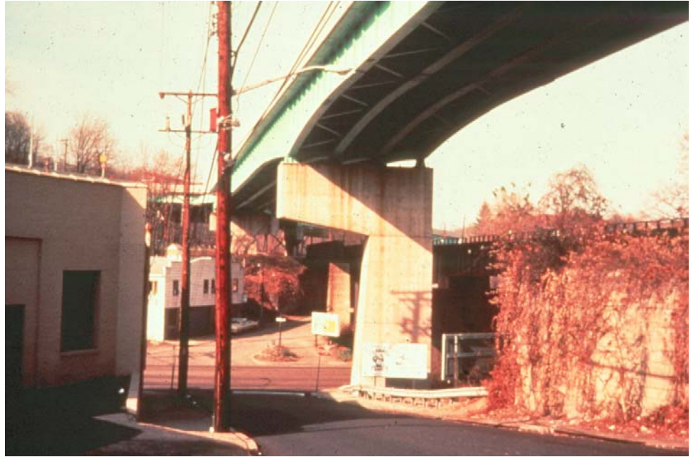
Figure P.2.5 Unusual Concrete Shapes
