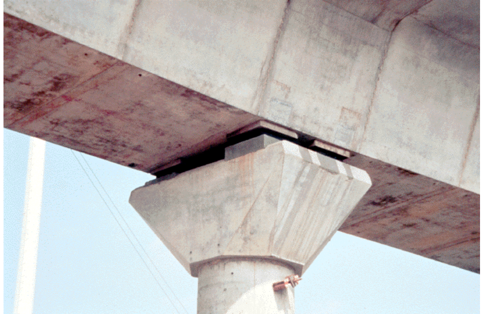
Figure 7.11.32 Box Girder Bearings at Intermediate Pier
