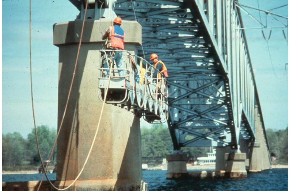
Figure 3.5.3 Rigging for Substructure Inspection
