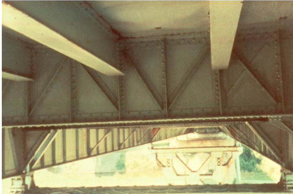
Figure 5.3.2 Underside View of Buckle Plate Deck
