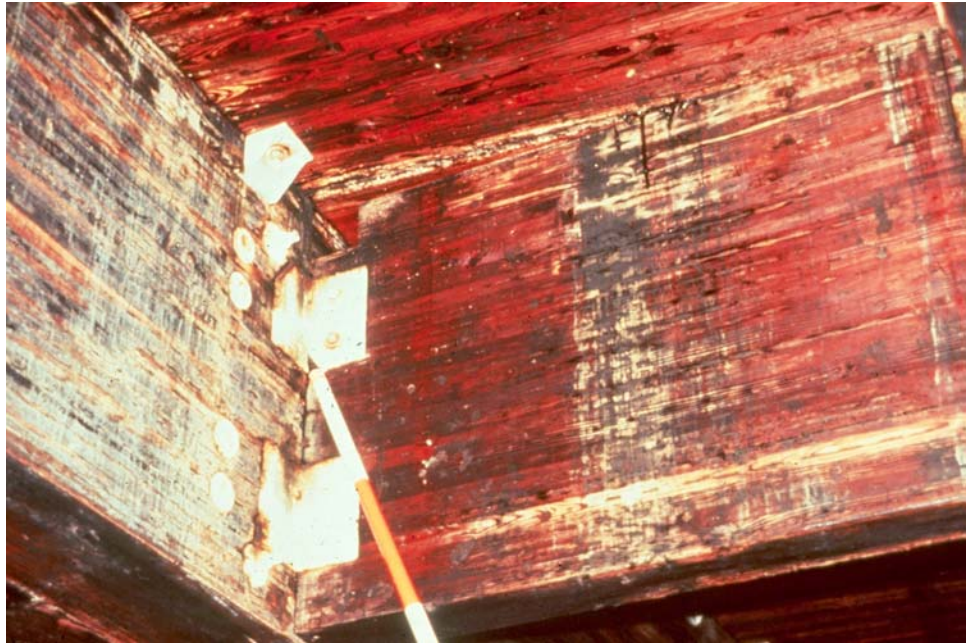
Figure 6.2.16 Typical Diaphragm for a Glulam Multi-beam Bridge
