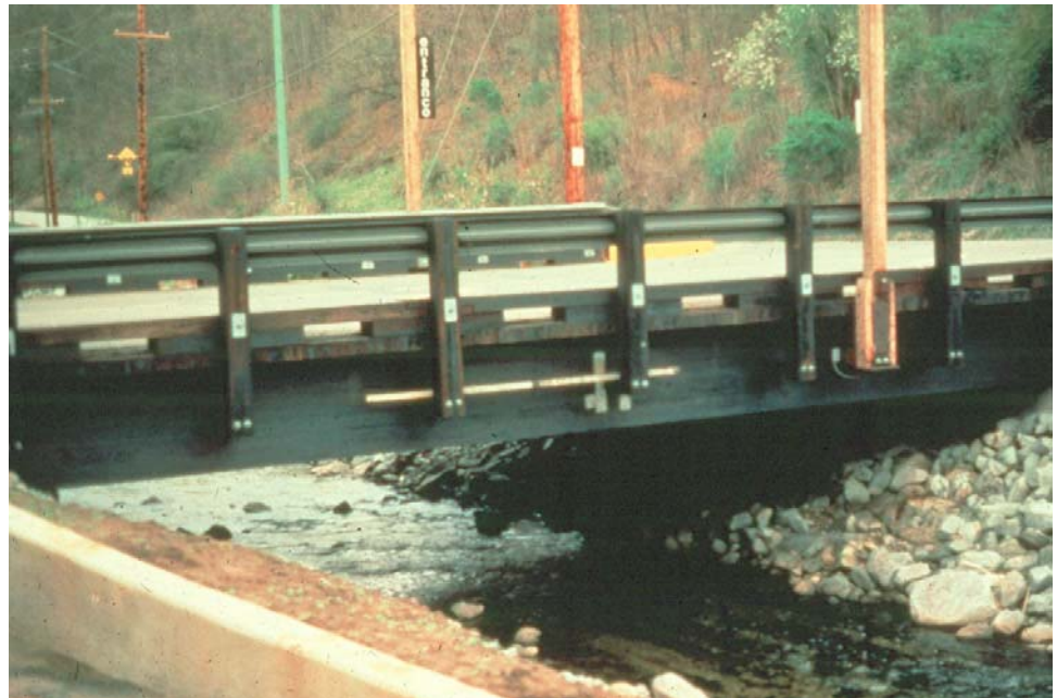
Figure 2.1.1 Glued-laminated Modern Timber Bridge
