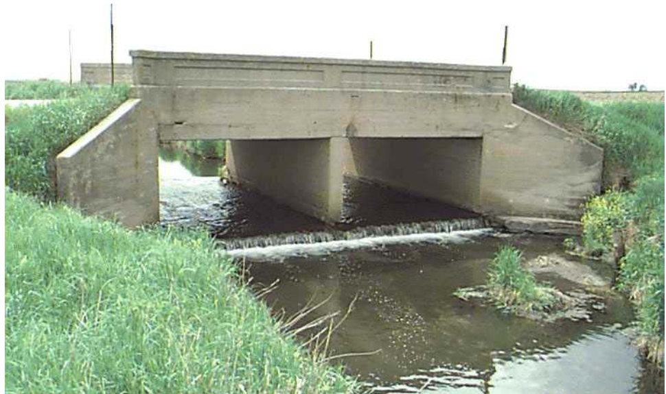
Figure P.3.1 Culvert Structure
