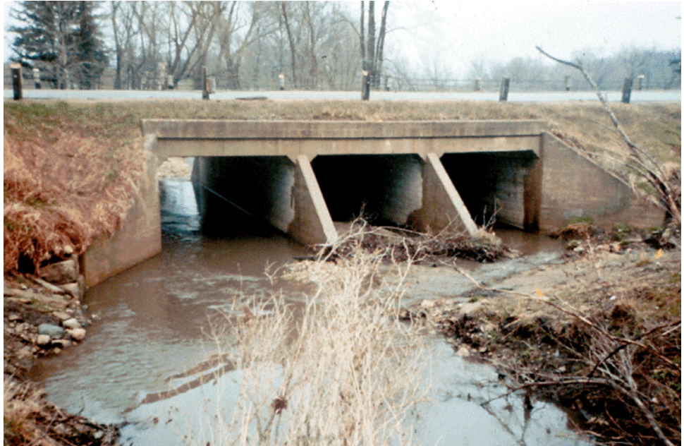
Figure 7.12.1 Concrete Box Culvert
