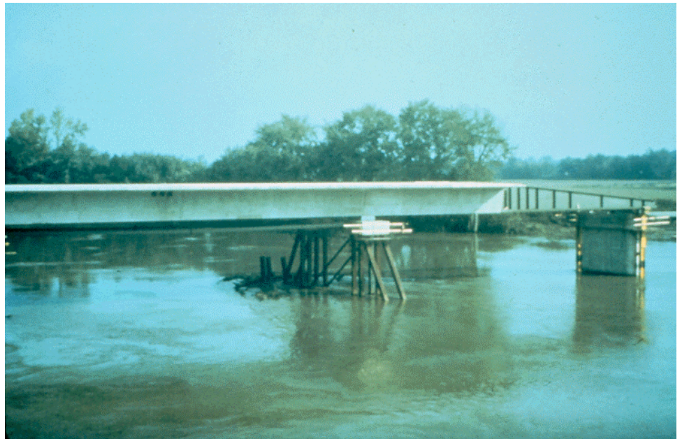
Figure 7.11.24 Incremental Launching Overview (Note Temporary Pile Bent)
