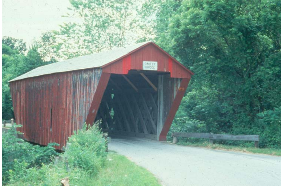
Figure 6.1.5 Town Truss Covered Bridge
