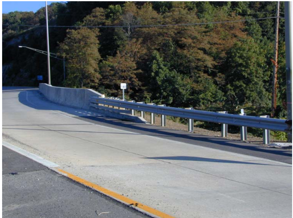
Figure 5.5.3 Approach Guardrail System
