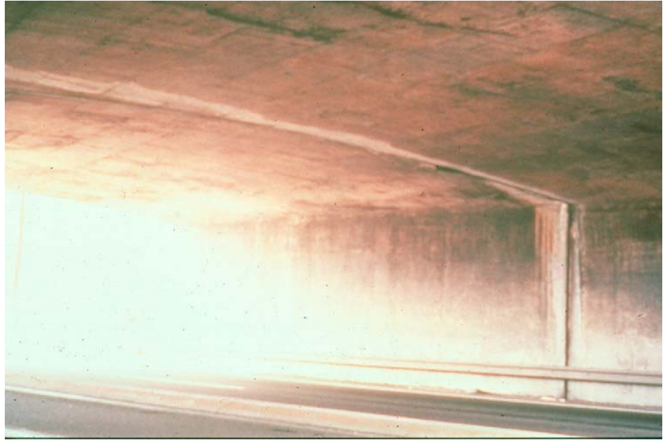
Figure 7.6.16 Longitudinal Joint Between Slab Beam Frames
