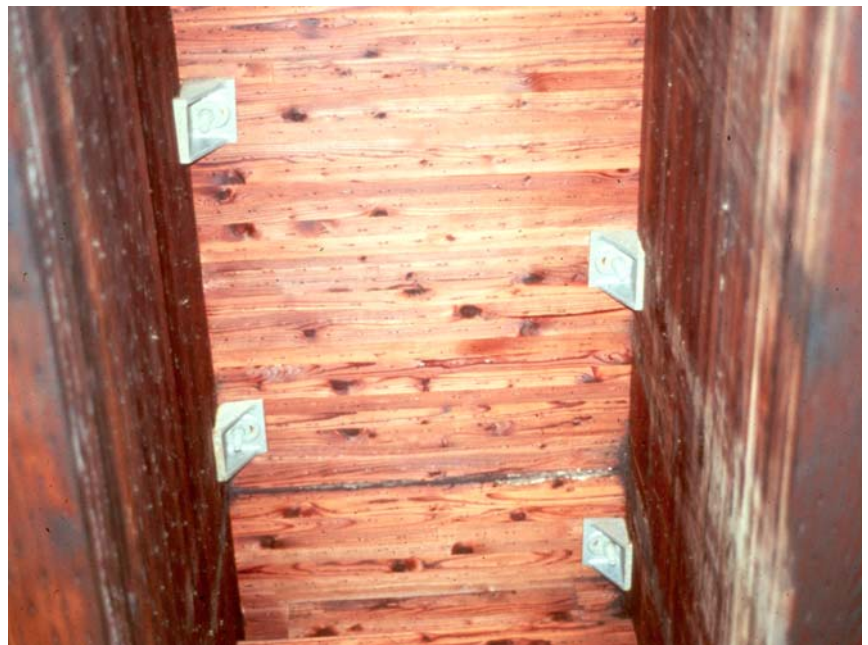
Figure 5.1.3 Glued-laminated Deck Panels
