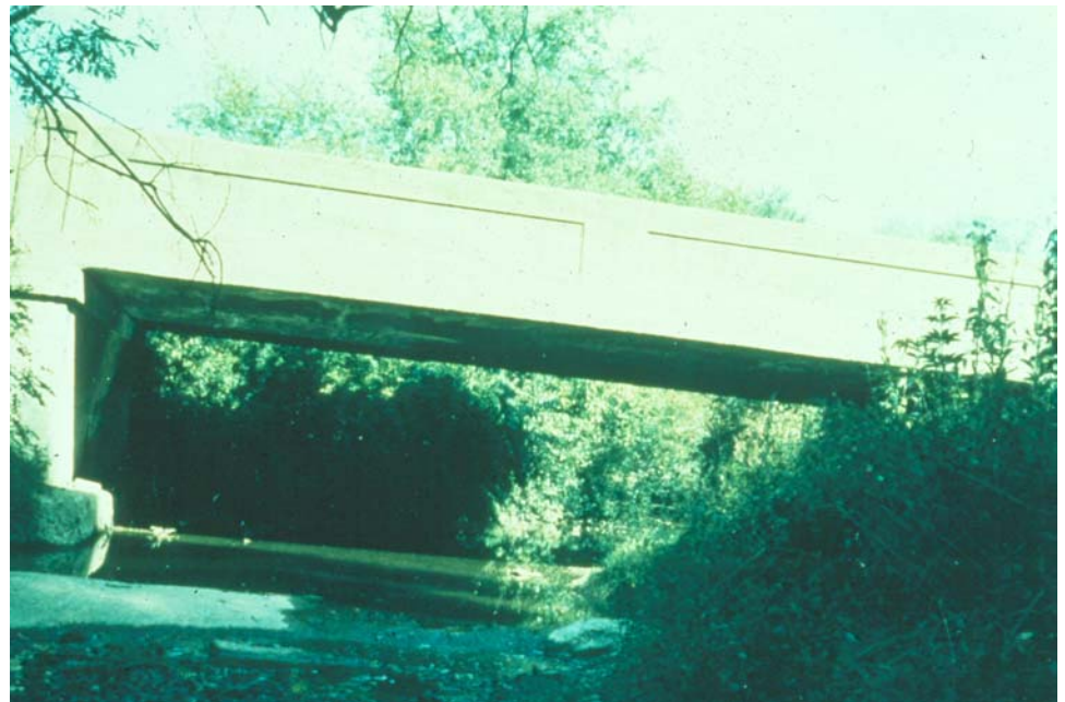
Figure 7.3.4 Concrete Through Girder Elevation View
