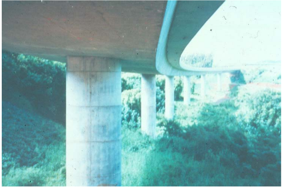
Figure 7.11.2 Typical Cast-in-place Concrete Box Girder Bridge
