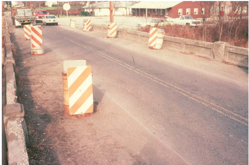
Figure 3.3.8 Vertical Panels – Note panels attached to drums
