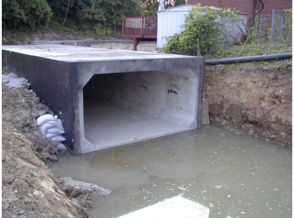
Figure 7.12.6 Precast Concrete Box Culvert
