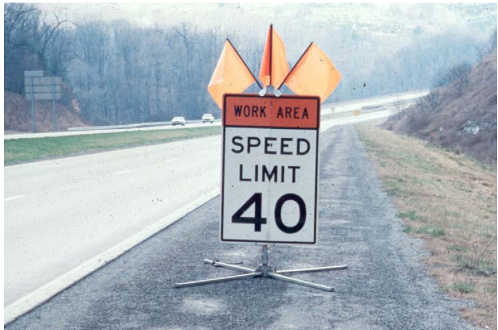
Figure 3.3.5 Work Area Speed Limit Sign (Regulatory)
