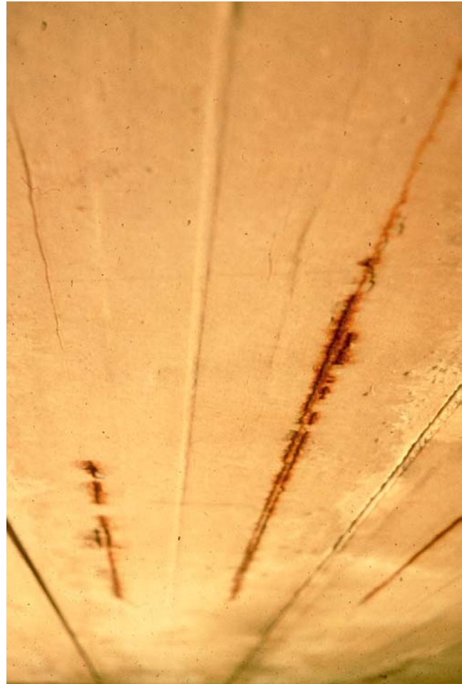
Figure 7.10.17 Burlap Fold Depressions in an Early 1950's P/S Box Beam
