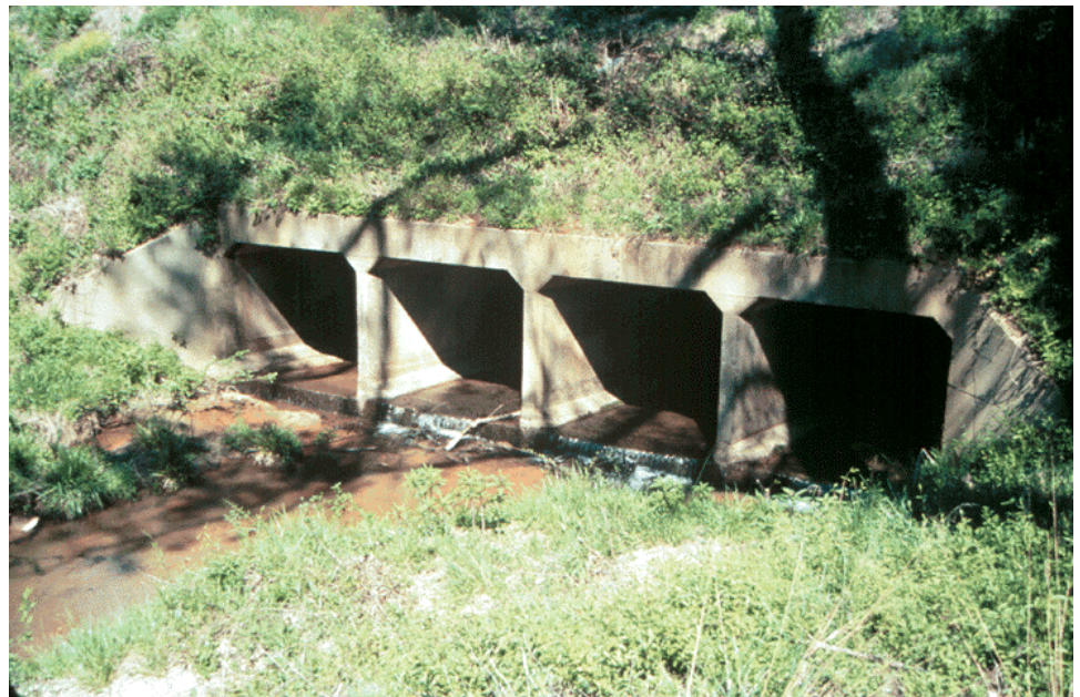
Figure P.3.10 Multiple Cell Concrete Culvert
