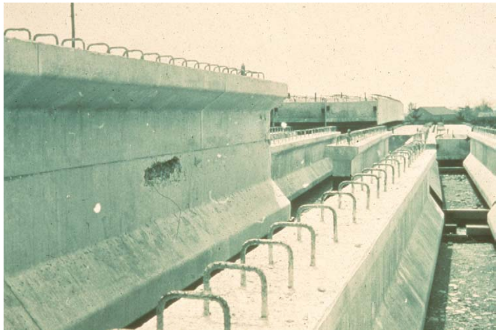
Figure 7.9.5 Cast-In-Place Stirrups
