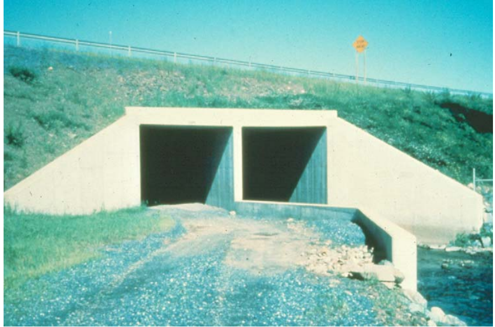
Figure 7.6.4 Typical Concrete Frame Culvert
