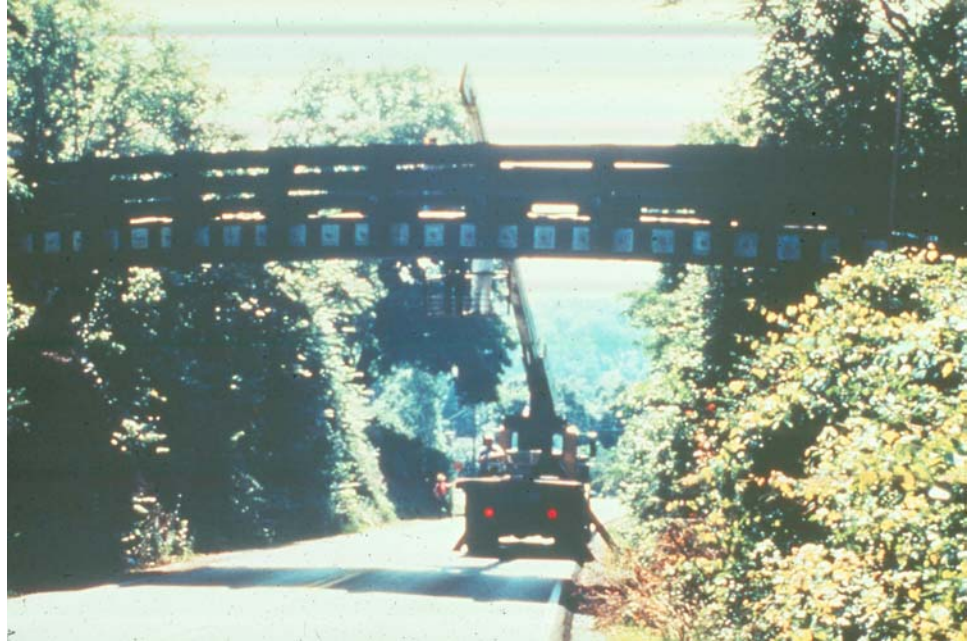
Figure 6.3.4 Glulam Stress-Laminated Deck/Slab Bridge
