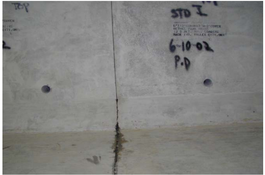
Figure 7.12.8 Precast Concrete Box Culvert Joint
