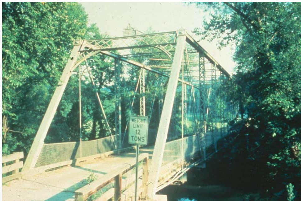
Figure P.2.43 Sway Bracing
