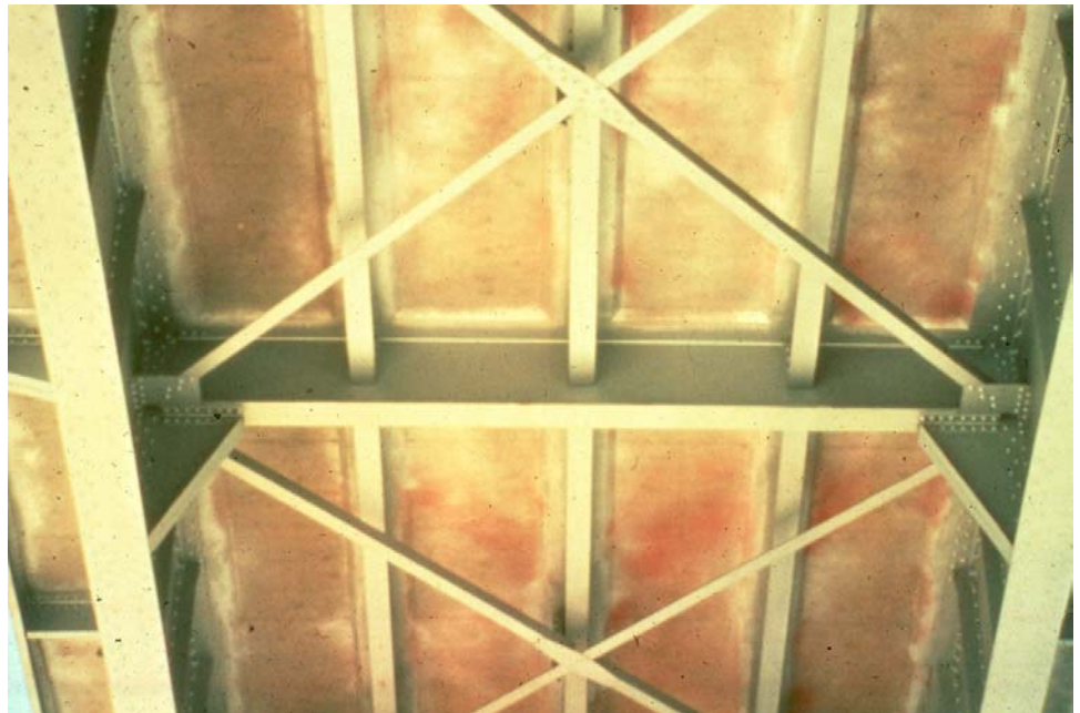
Figure P.2.39 Floor System
