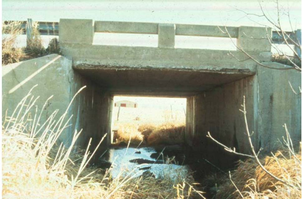
Figure 7.1.1 Typical Simple Span Cast-in-Place Slab Bridge
