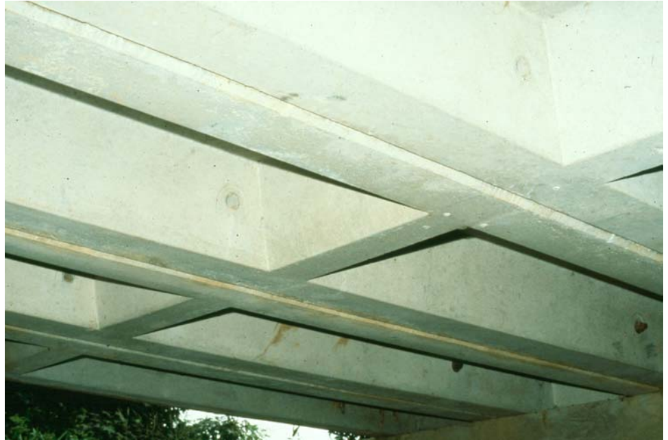
Figure 7.4.1 Underside View of Precast Channel Beam Bridge
