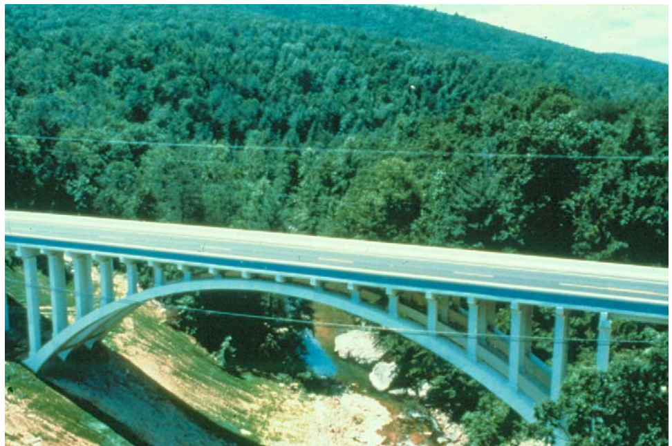
Figure 7.5.1 Open Spandrel Arch Bridge
