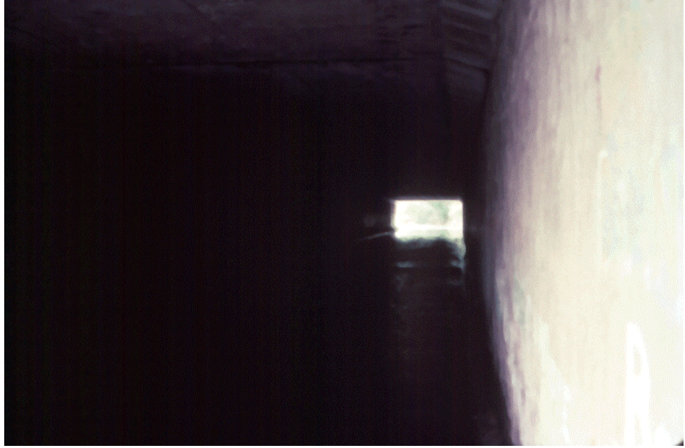
Figure 7.12.7 Sighting Along Culvert Sidewall to Check Horizontal Alignment
