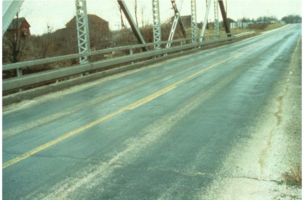
Figure P.2.32 Asphalt Wearing Surface on a Concrete Deck
