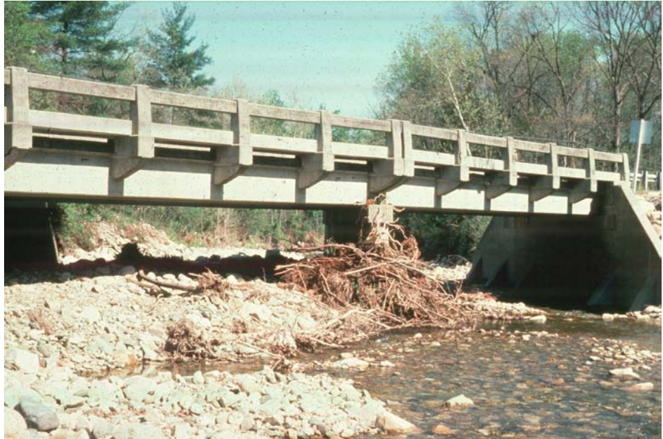
Figure 7.2.1 Multi-span, Simply Supported Tee Beam Bridge
