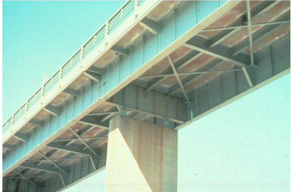
Figure P.2.48 Girder Floorbeam Stringer Bridge
