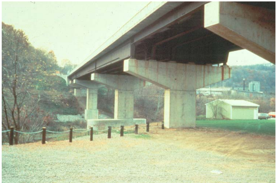
Figure P.2.73 Cantilever or Hammerhead Pier
