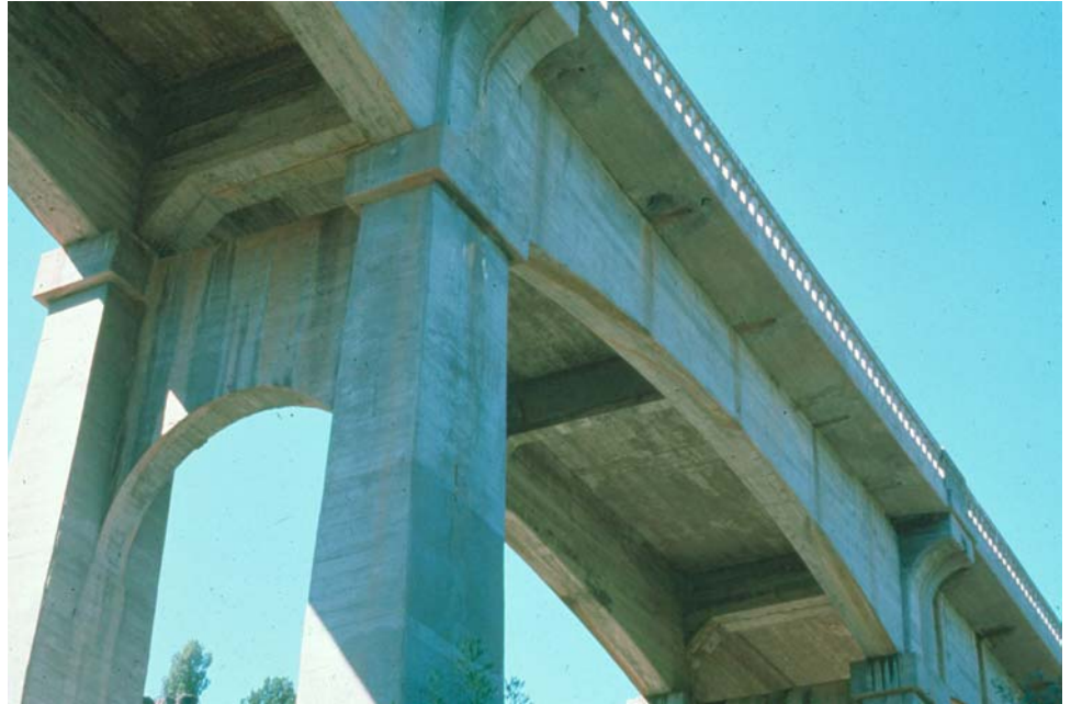
Figure 7.3.3 Concrete Deck Girder, Underside View
