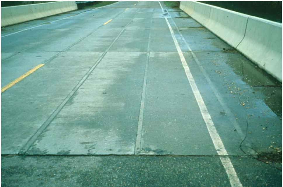
Figure 7.4.8 Top of Slab View of Precast Channel Beam Bridge
