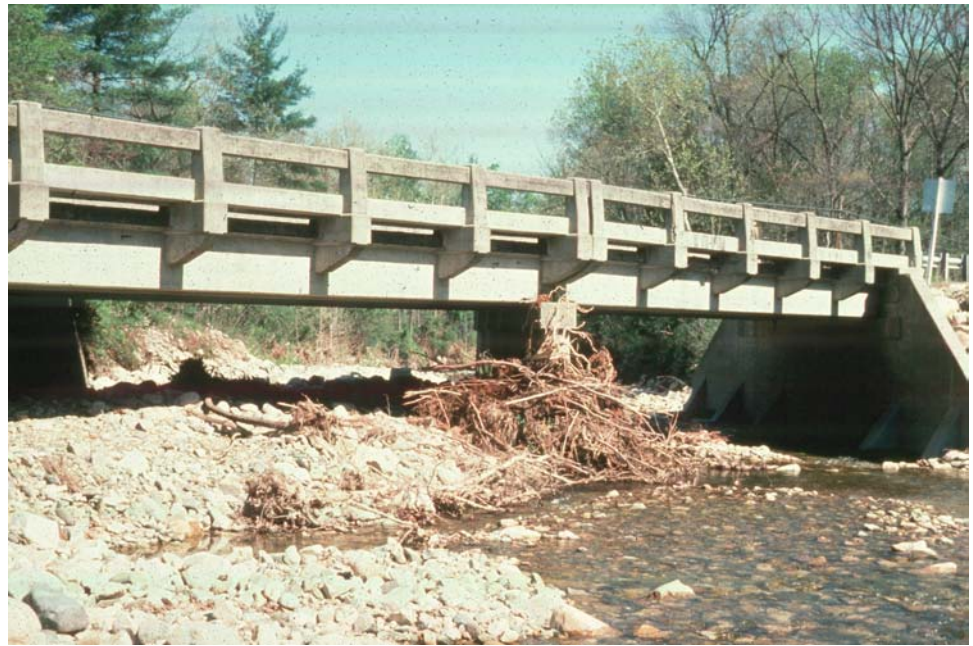
Figure P.1.26 Integral Bridge Deck
