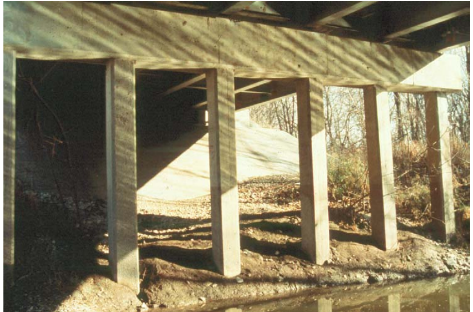
Figure P.2.9 Concrete Pile Bent
