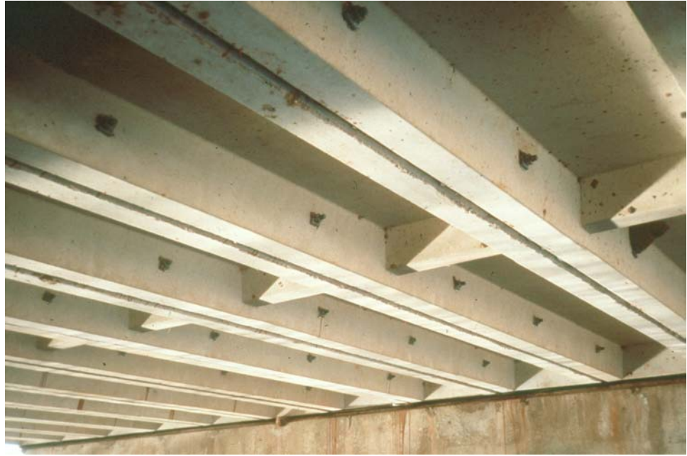
Figure 7.4.2 General Underside View of Channel Beam Bridge
