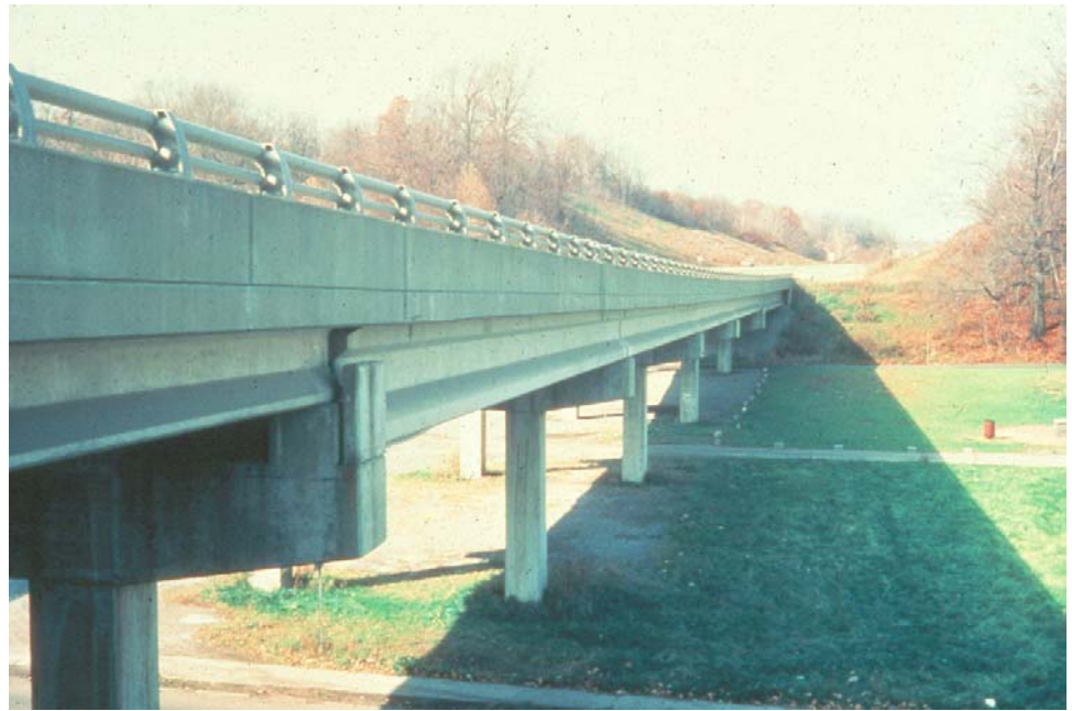
Figure 7.9.1 Prestressed I-Beam Superstructure
