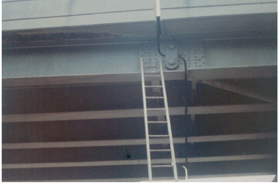
Figure P.2.23 Pin and Hanger Connection
