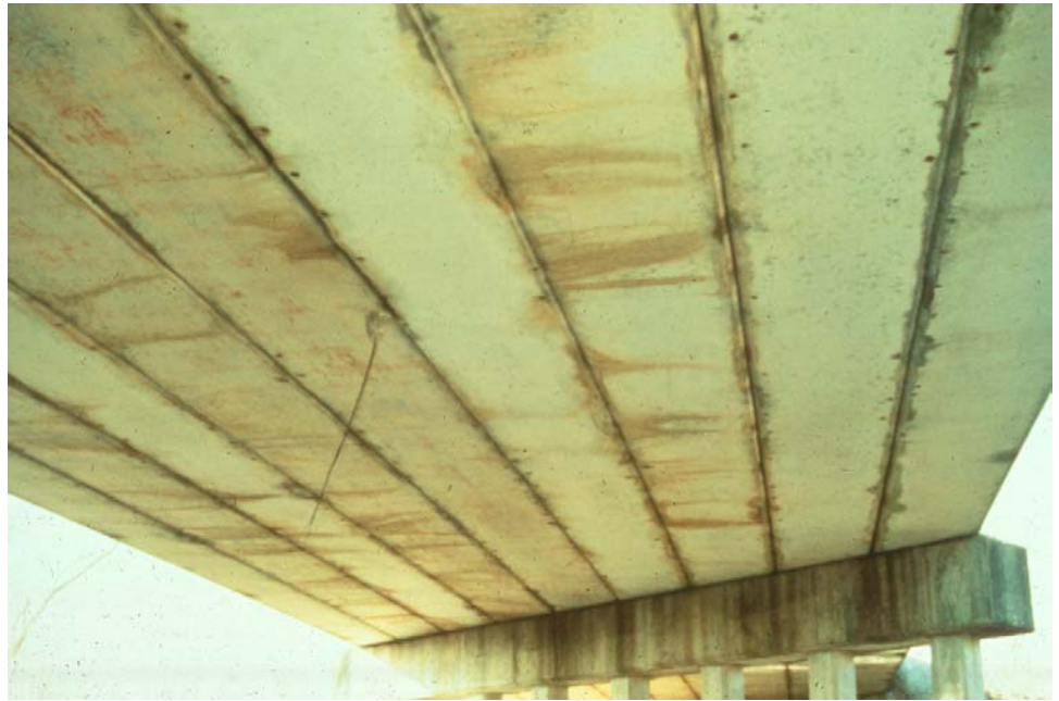
Figure P.2.51 Adjacent Box Beam Bridge
