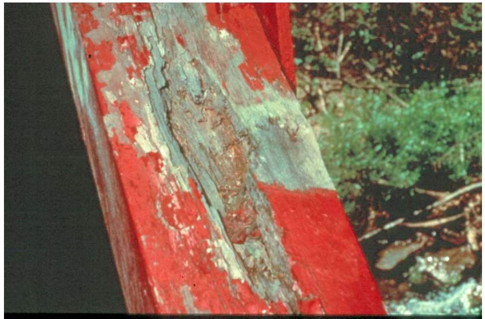
Figure 2.1.7 Decay of Wood by Fungi
