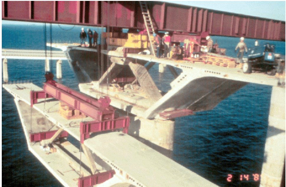
Figure 7.11.17 Balanced Cantilever Construction
