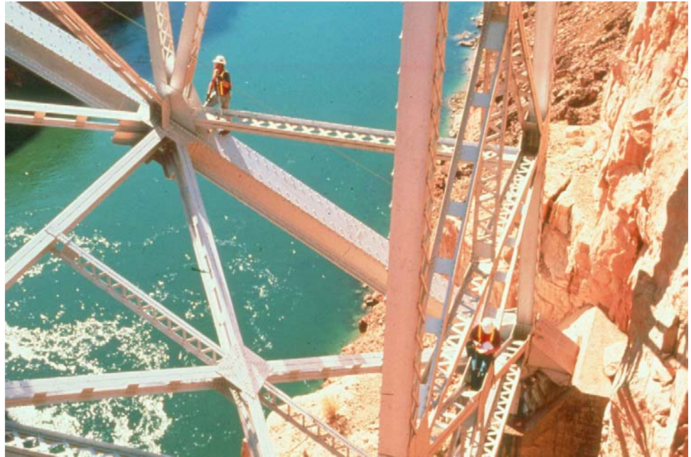
Figure 3.2.7 Inspection Involving Extensive Climbing
