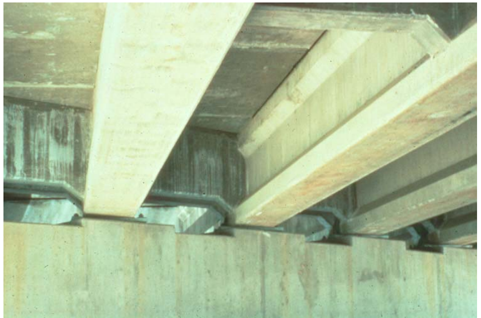
Figure P.2.47 Prestressed Concrete Multi-beam Bridge
