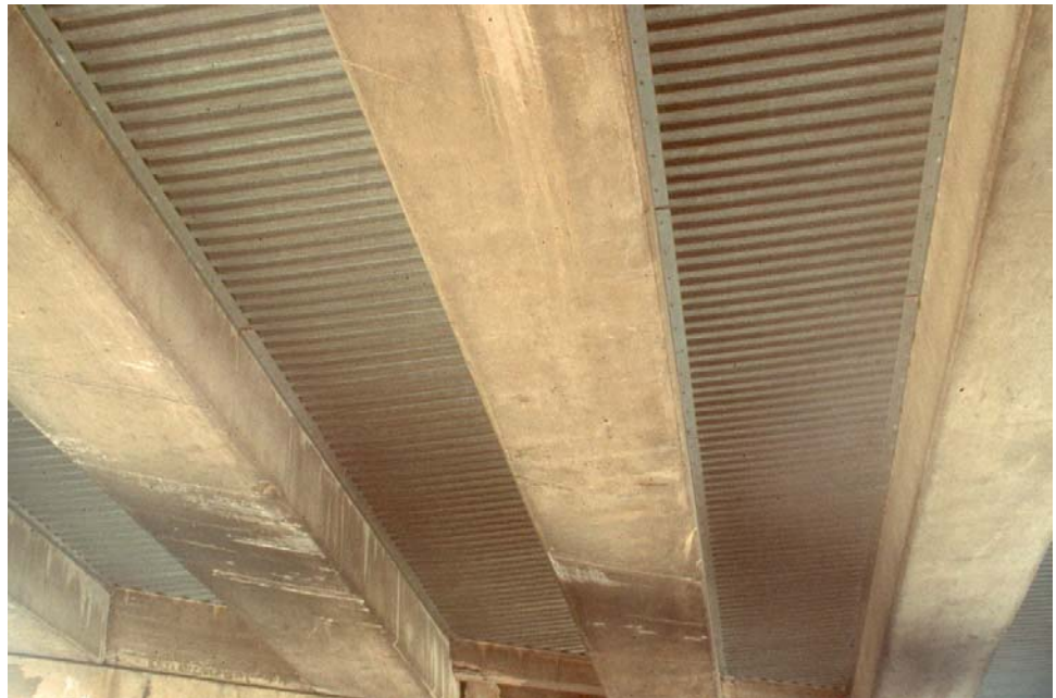
Figure 7.10.7 Underside of a Typical Spread Box Beam
