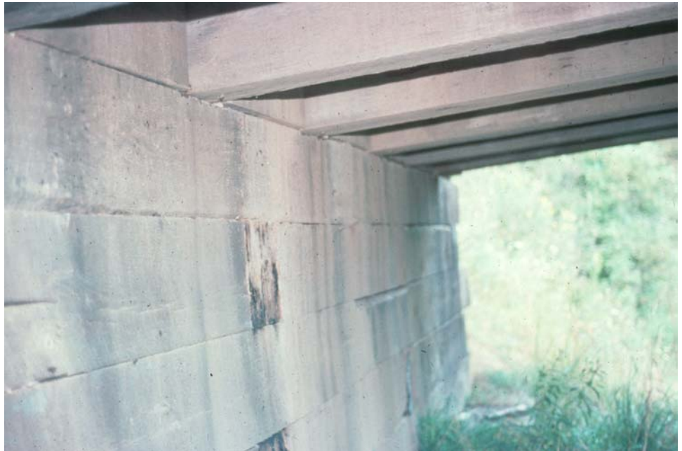
Figure 6.1.11 Bearing Area of Typical Solid Sawn Beam
