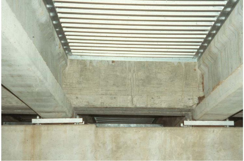
Figure 7.9.11 Typical Concrete Diaphragm
