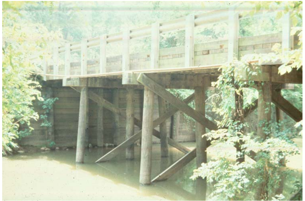
Figure P.2.46 Timber Beam Bridge
