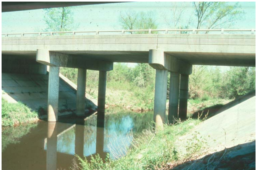
Figure 7.1.2 Typical Multi-span Cast-in-Place Slab Bridge
