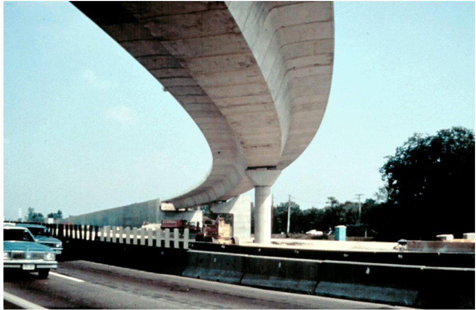
Figure 7.11.12 Segmental Concrete Bridge
