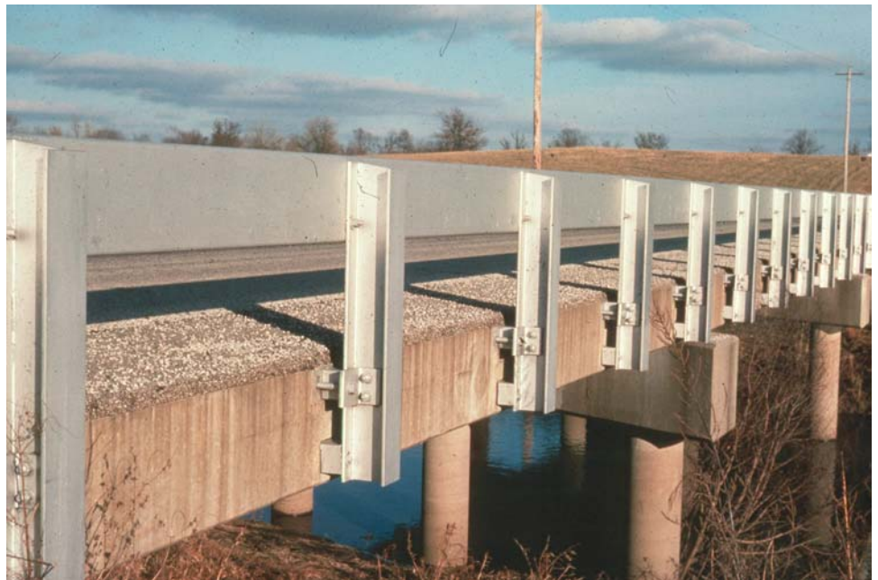
Figure 7.7.1 Typical Prestressed Slab Beam Bridge
