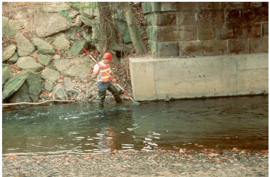
Figure 3.1.5 Inspection for Scour and Undermining
