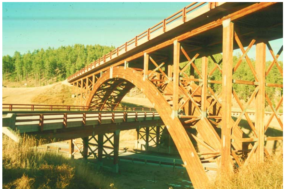
Figure 6.2.8 Glulam Arch Bridge over Glulam Multi-beam Bridge (Keystone Wye interchange, South Dakota)
