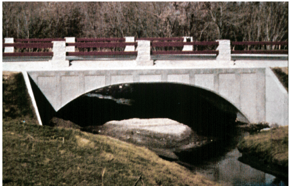
Figure P.3.8 Arch Culvert
