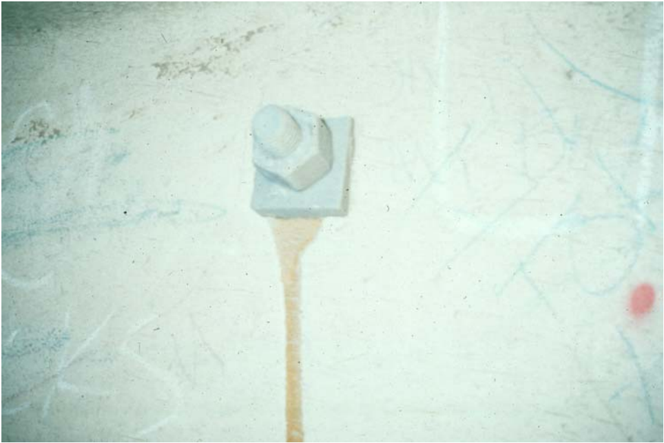
Figure 7.4.10 Close-up of Stem Tie-bolt
