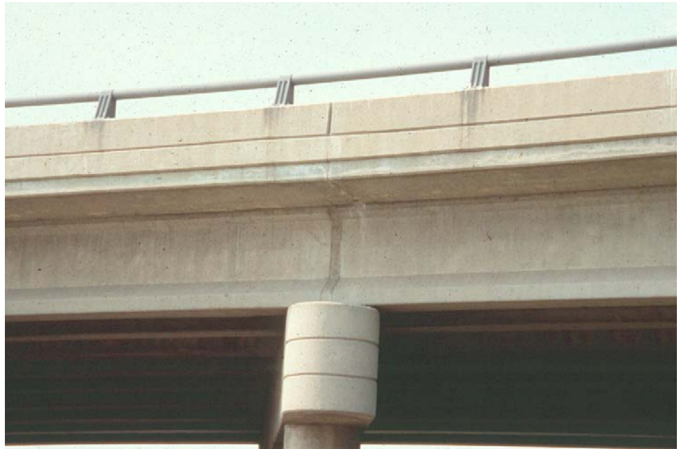
Figure 7.9.4 Continuous Prestressed I-Beam Bridge
