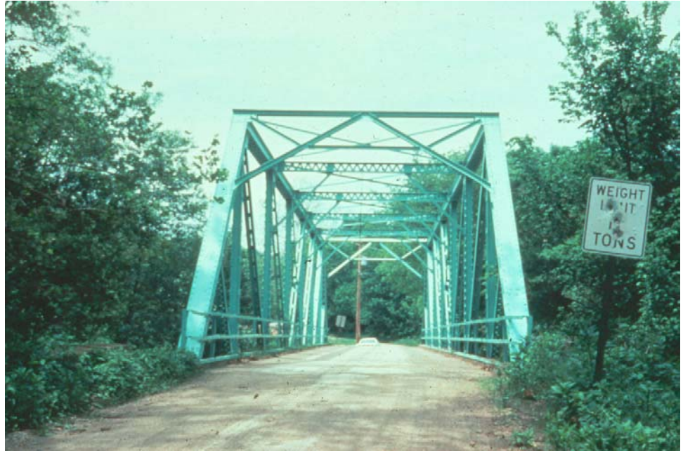
Figure P.2.54 Through Truss Bridge
