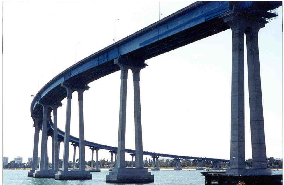
Figure P.2.49 Curved Girder Bridge
