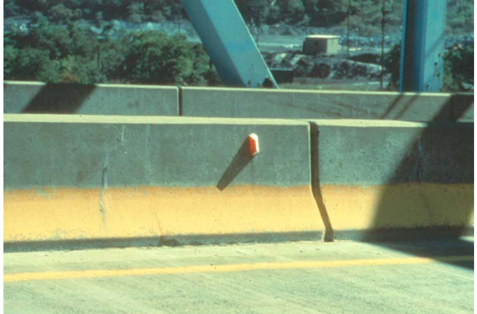
Figure P.2.36 New Jersey Barrier
