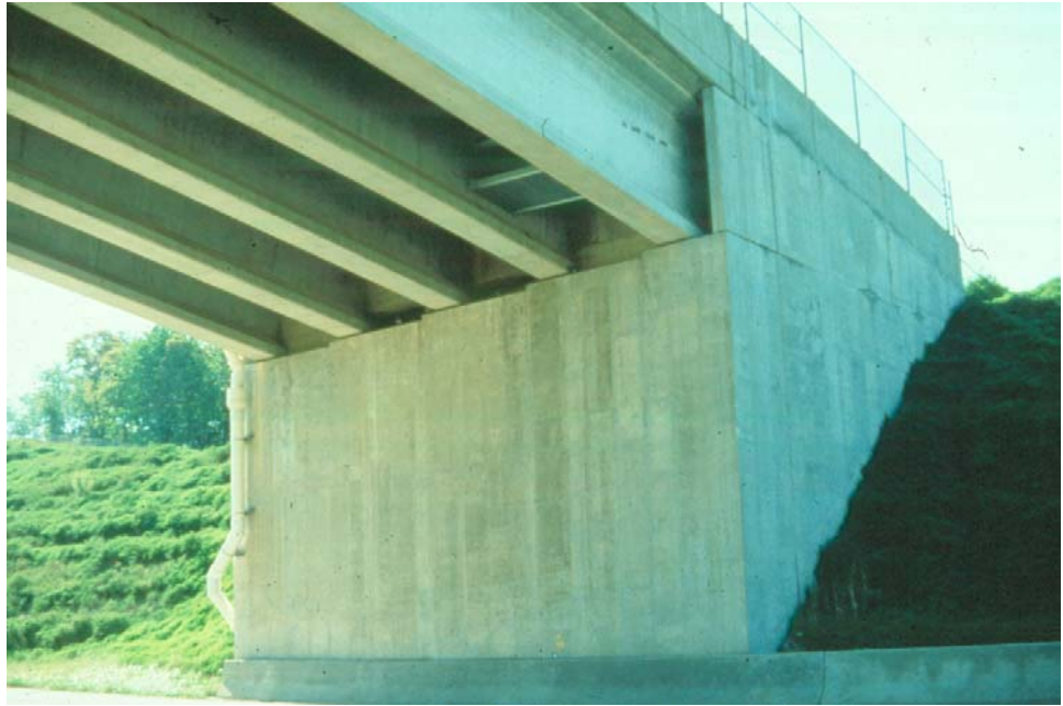
Figure P.2.65 Concrete Abutment
