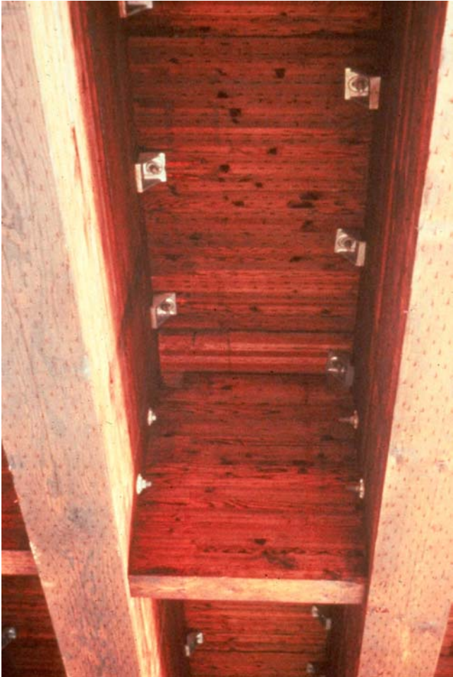
Figure 6.2.11 Typical Glulam Diaphragm
