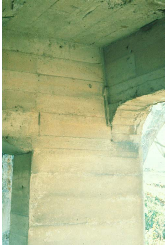
Figure 7.5.13 Spandrel Column Cap Interface
