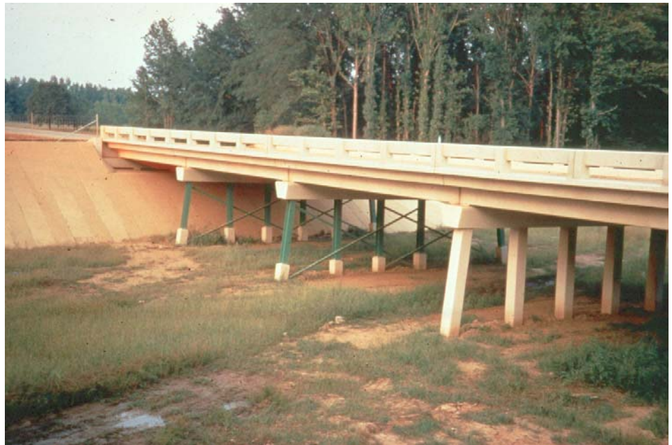
Figure P.2.75 Pile Bent
