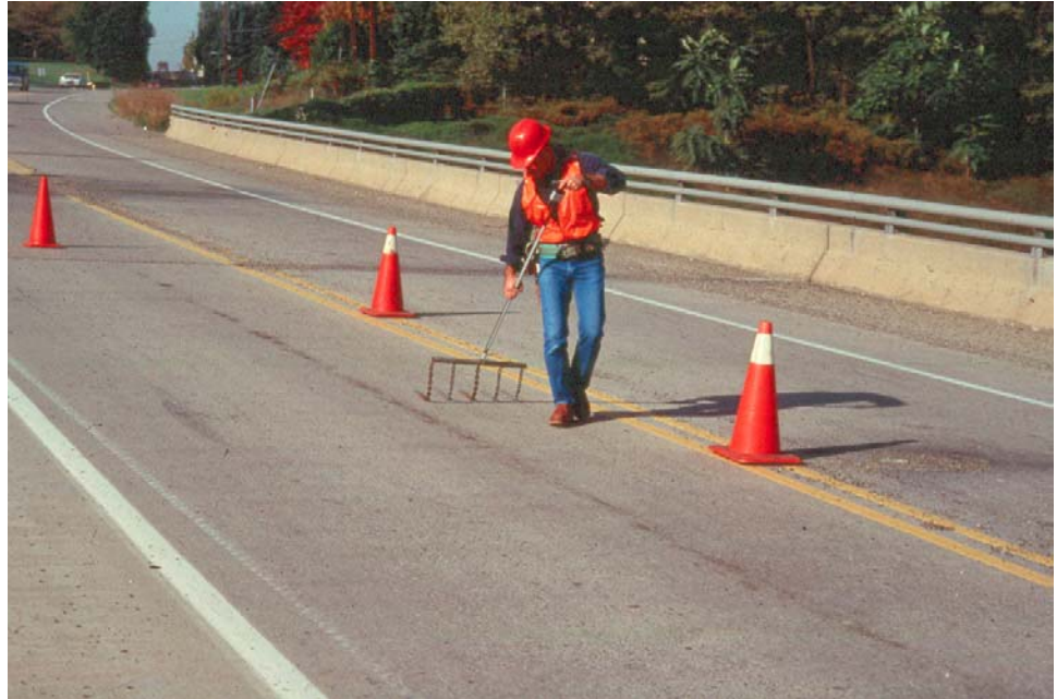
Figure 5.2.6 Inspector Using a Chain Drag
