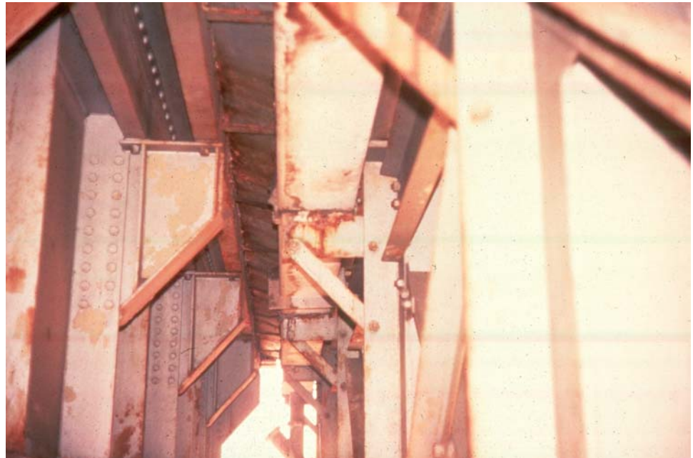
Figure 5.4.20 Support System under a Finger Plate Joint
