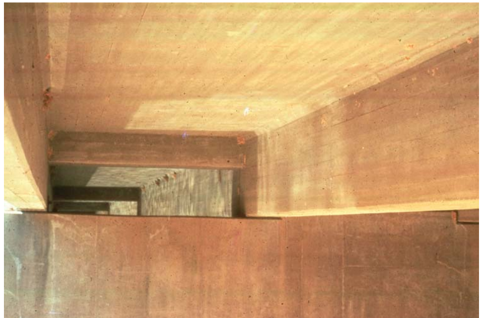
Figure 7.2.6 Tee Beam Diaphragms
