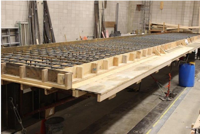
a) Formwork and reinforcement
