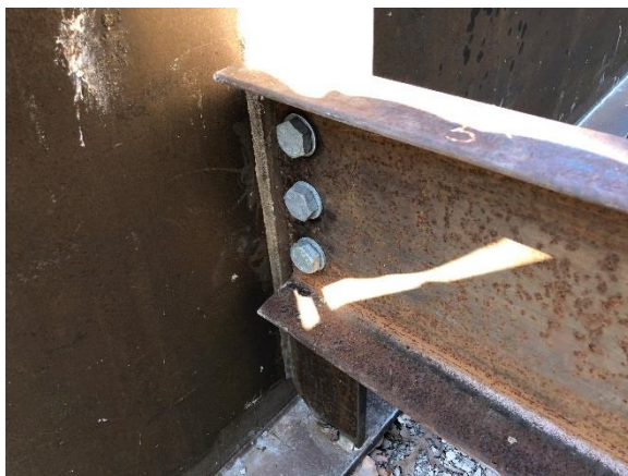
b) Galvanized steel bolted connection
