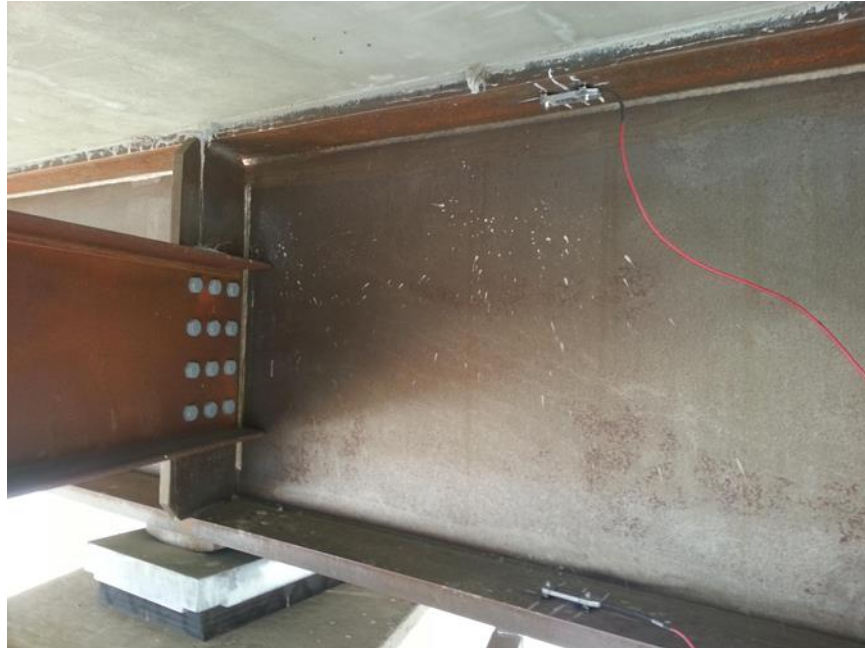
a) Strain gauge setup on A1010 steel girder
