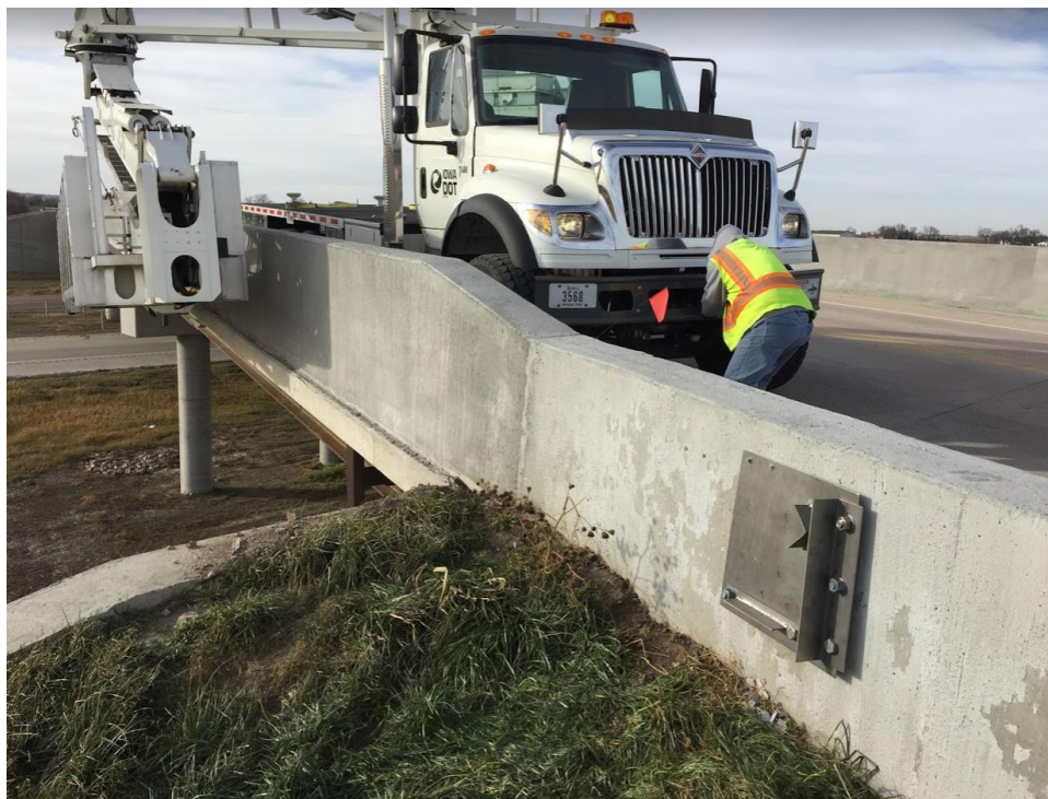
Figure 54. A1010 plate mounting in the field (December 2017)
