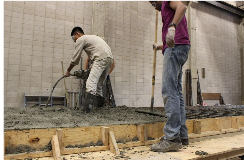
b) Concrete placement
