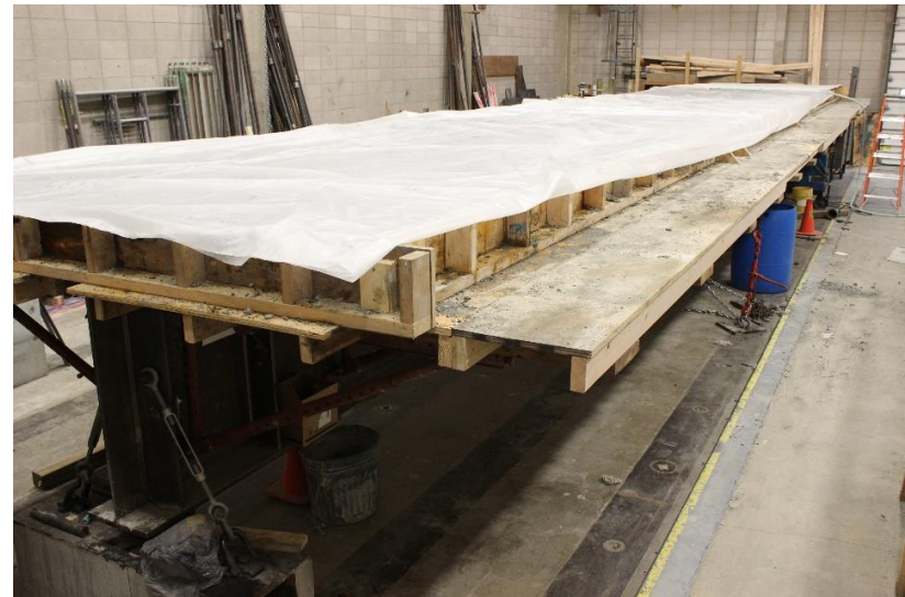
d) Deck concrete curing
