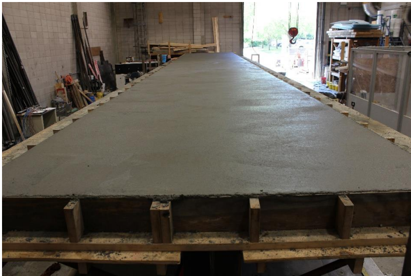
c) Deck finishing
