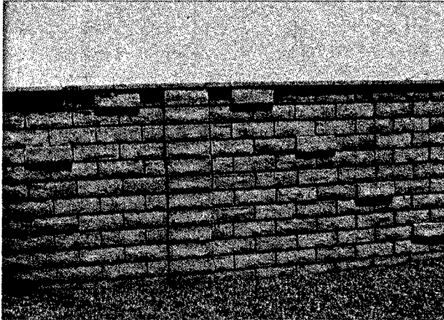
Slump blocks offset to create shadows.
