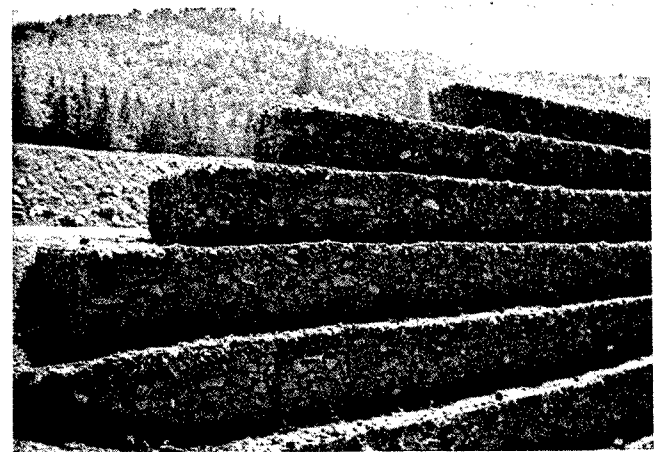
Gabions may be stacked in a variety of ways to construct a wall.
