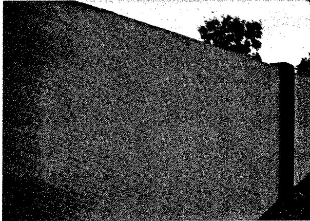
A fine textured broom finish is difficult to see at a distance.
