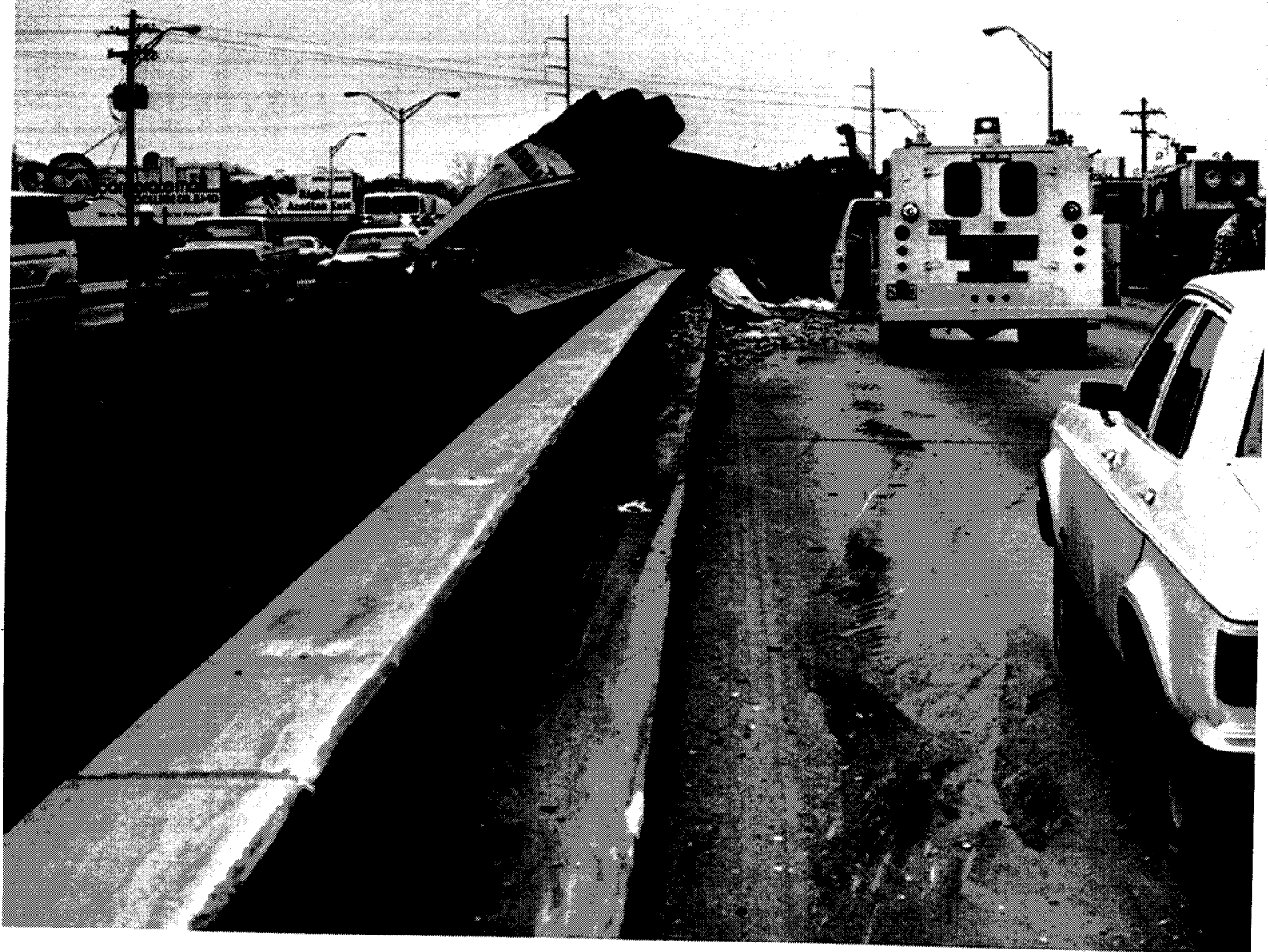
TRUCK STRUCK BRIDGE - OVERTURNED
