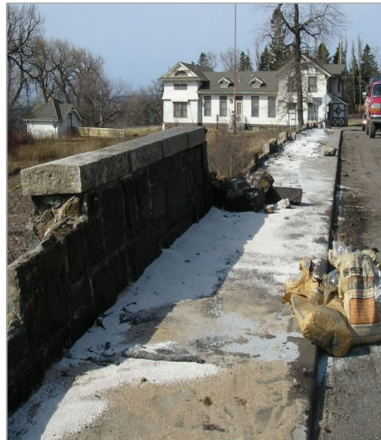
Figure 9. Photos. MnDOT Examples of Superstructure and Railing Damage Due to Truck Impact.
