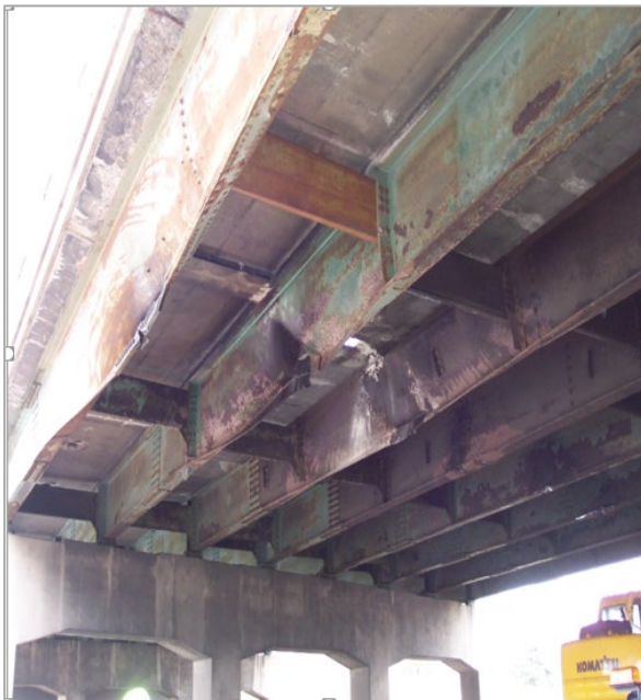
Figure 9. Photos. MnDOT Examples of Superstructure and Railing Damage Due to Truck Impact.
