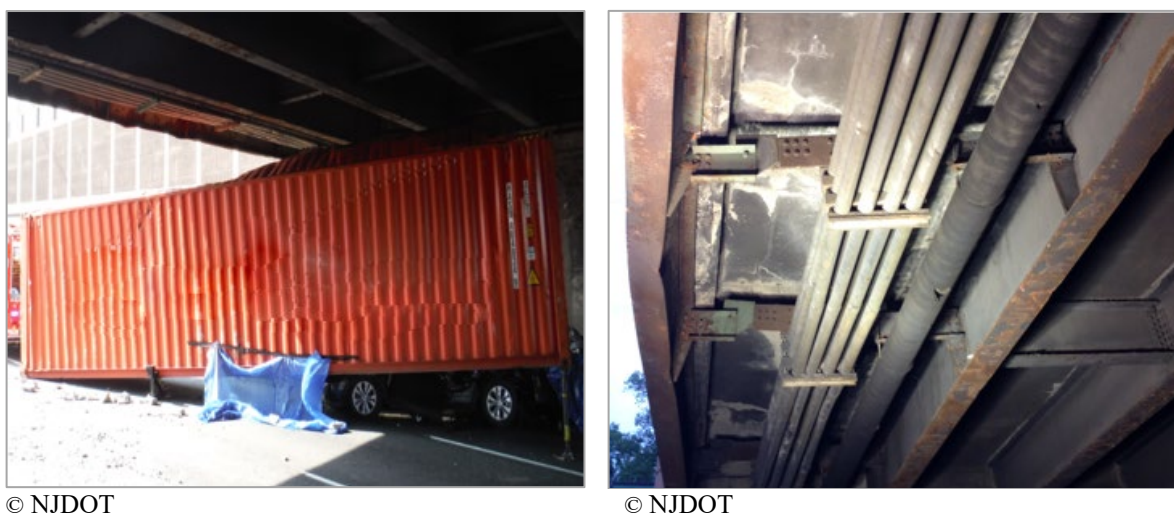
Figure 13. Photos. NJDOT Examples of Superstructure Damage Due to Truck Impact.
