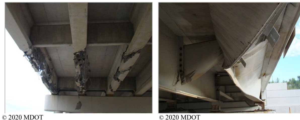
Figure 6. Photos. MDOT Examples of Typical Type III Damage.
