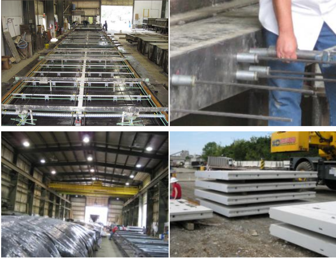
Figure 29. PPCP formwork set up at precast plant, curing, and yard storage.
