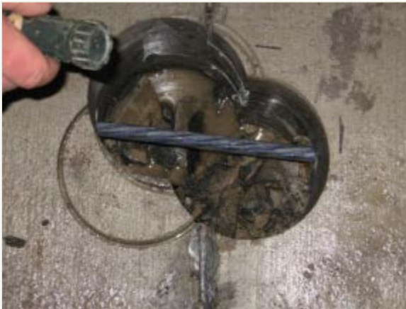
a) Top view across the transverse joint
