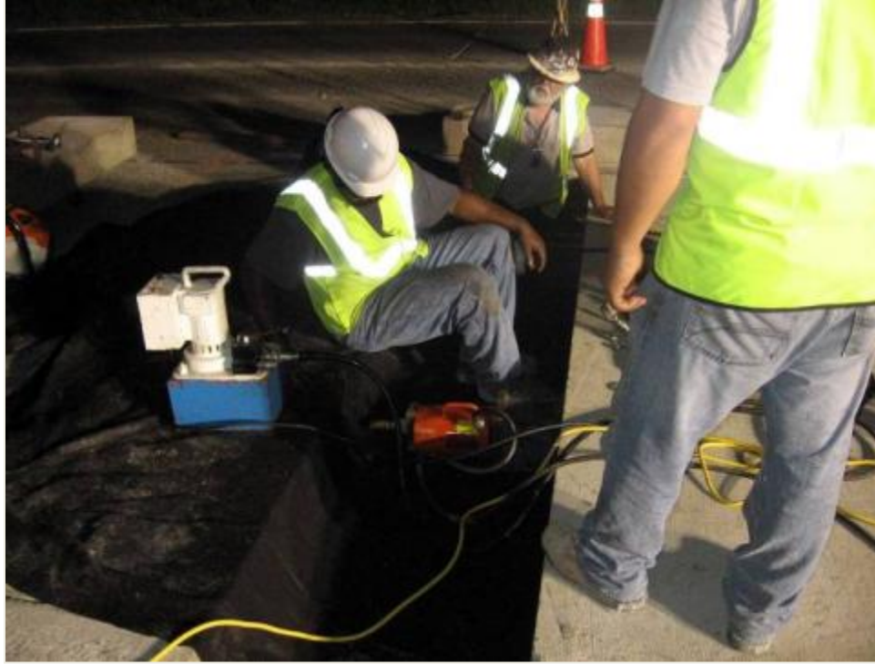
Figure 45. Initial post-tensioning.
