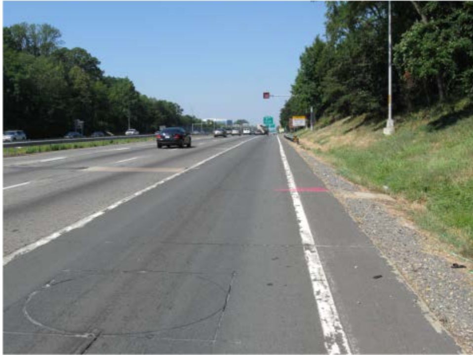
Figure 2. Westbound I-66 mainline with three lanes and an auxiliary shoulder.
