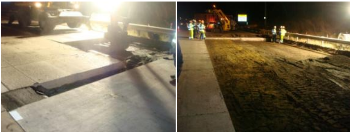
Figure 41. Removal of existing slabs.
