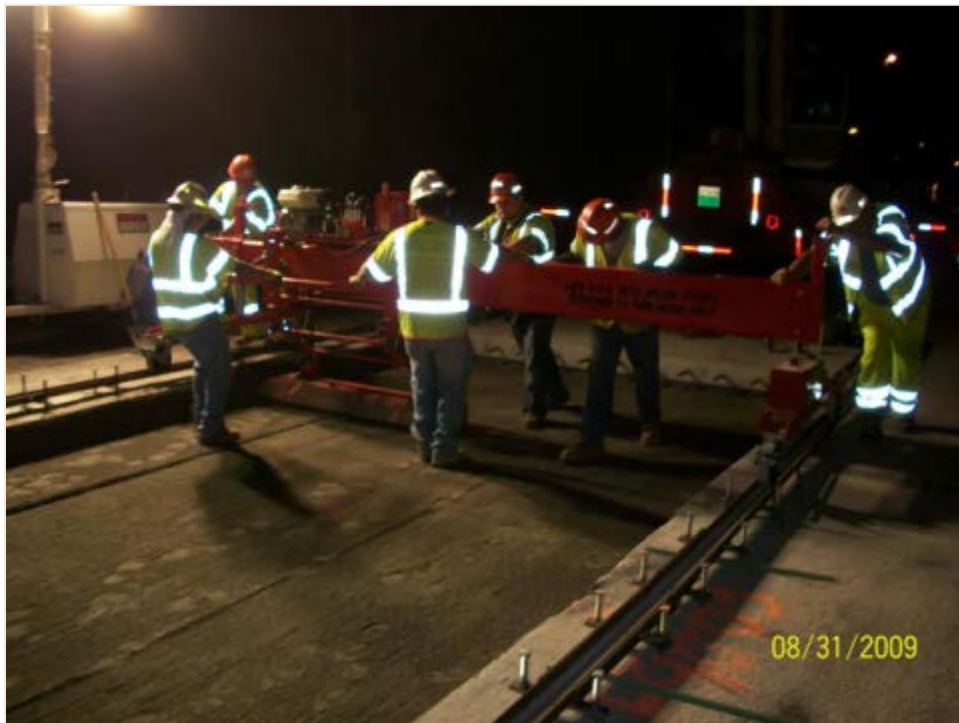
Figure 55. Fine grading of subbase material.
