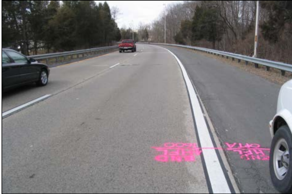
Figure 3. Ramp from I-66 to US 50 West with two lanes and a shoulder.
