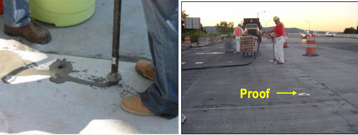
Figure 23. Verification of dowel grout and bedding grout distribution for uniform support (image from project in New York State, 2002).
