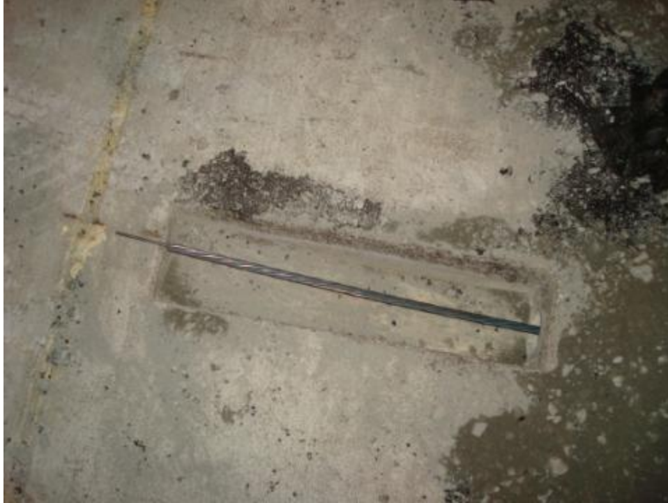
a) Tendon inserted in anchor panel blockouts
