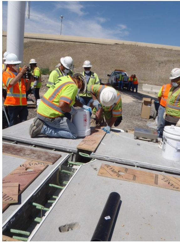
Figure 4. Photo. Mock Up UHPC during Field Demonstration. (courtesy: UDOT)
