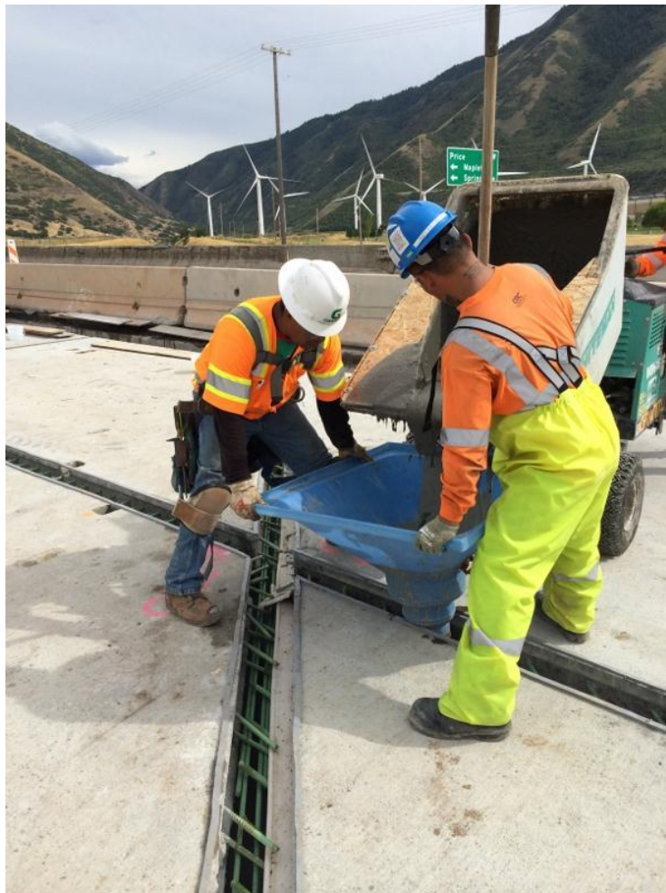
Figure 5. Photo. UHPC placement (courtesy: UDOT).
