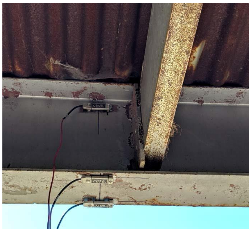
Figure 67. Instrumentation near Midspan for Yutan Bridge Load Test 1
