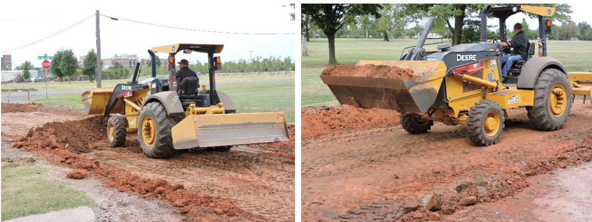
Figure 10-3. Excavation and Preparation of Subbase for Pavement Construction
