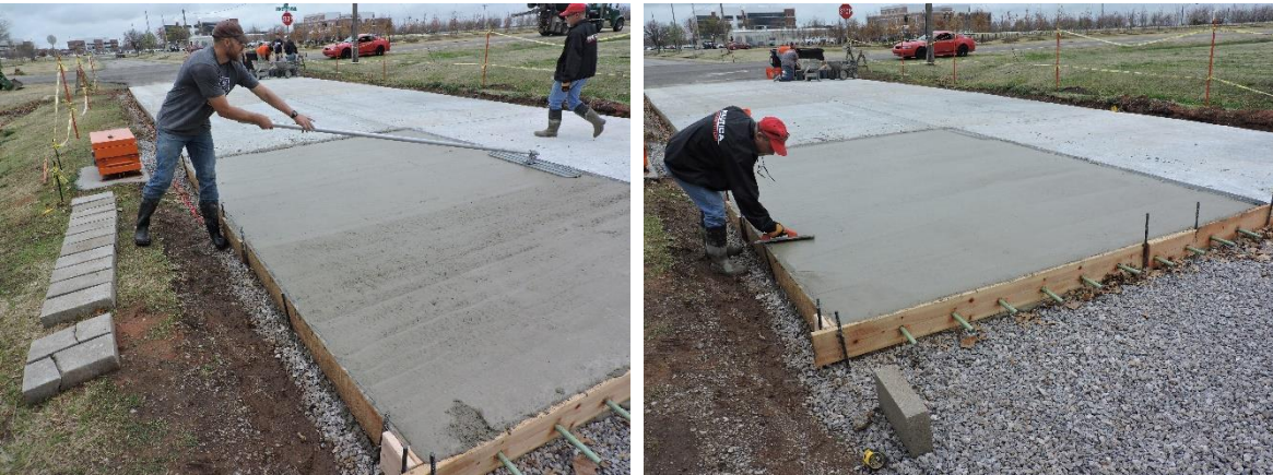
Figure 10-13. Concrete Floating (l) and Finishing (r)
