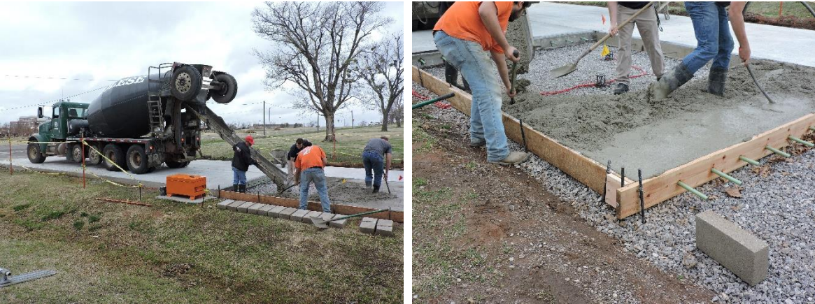
Figure 10-12. Concrete Placement (l) and Consolidation (r)
