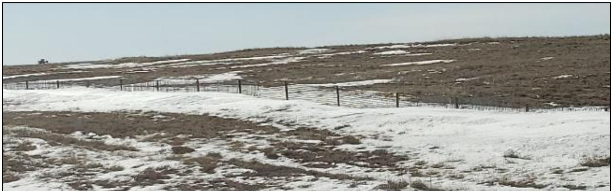
Figure 4.5 - Example of Lath Snow Fences on I-80 (Taken: 2019)
