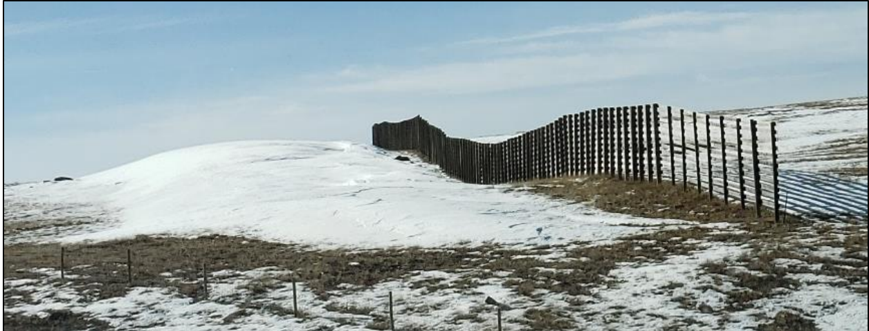
Figure 4.7 Examples of Upright/Vertical Snow Fences on I-80 (Taken: 2019)
