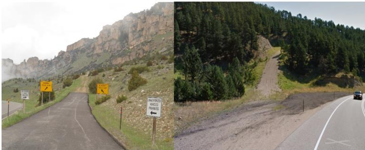
(D) Escape Ramps at Ten Sleep Canyon and Mosier Gulch (US-16) Respectively.
