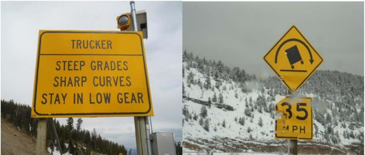
(B) Truck Warning Sign with flasher and Curve Warning Sign (US-14).
