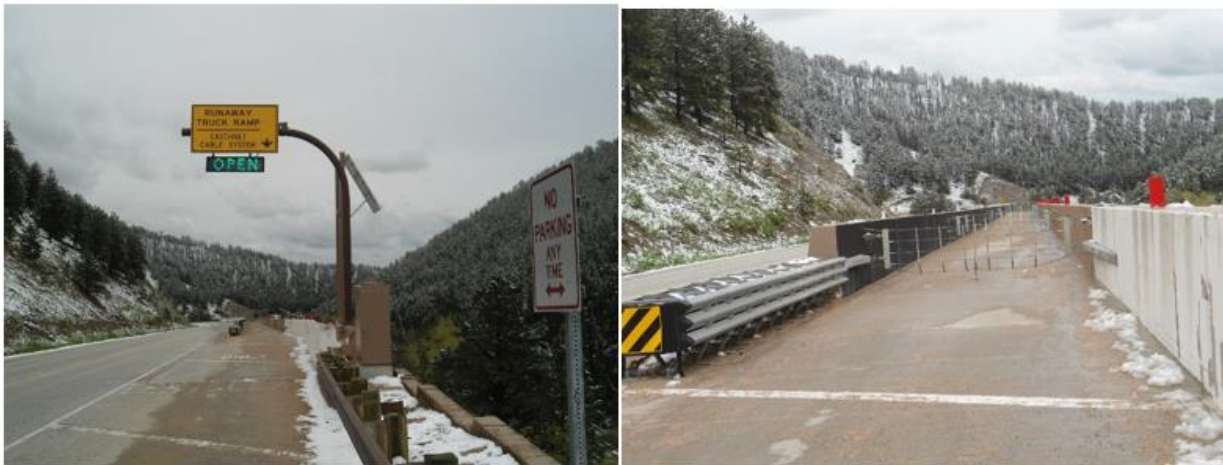
(B) Cable Catch-Net System at Mosier Gulch (US-16).
