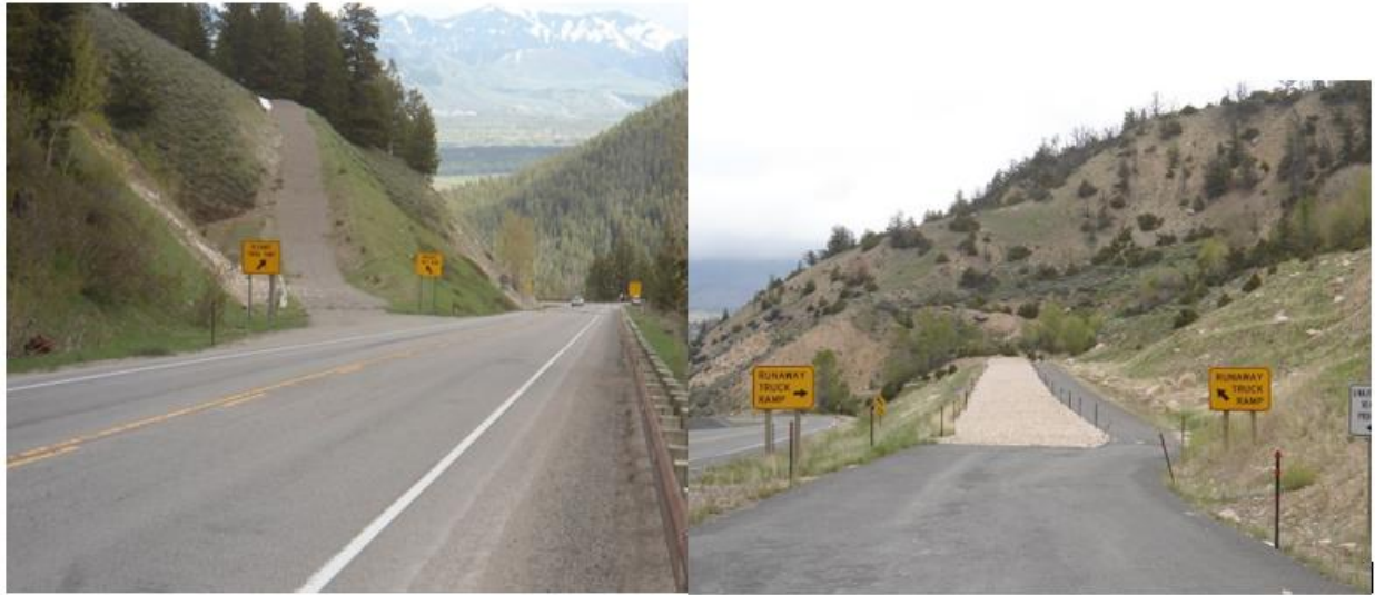
(C) Escape Ramps at Teton Pass (WY-22) and Shell Creek (US-14) Respectively.
