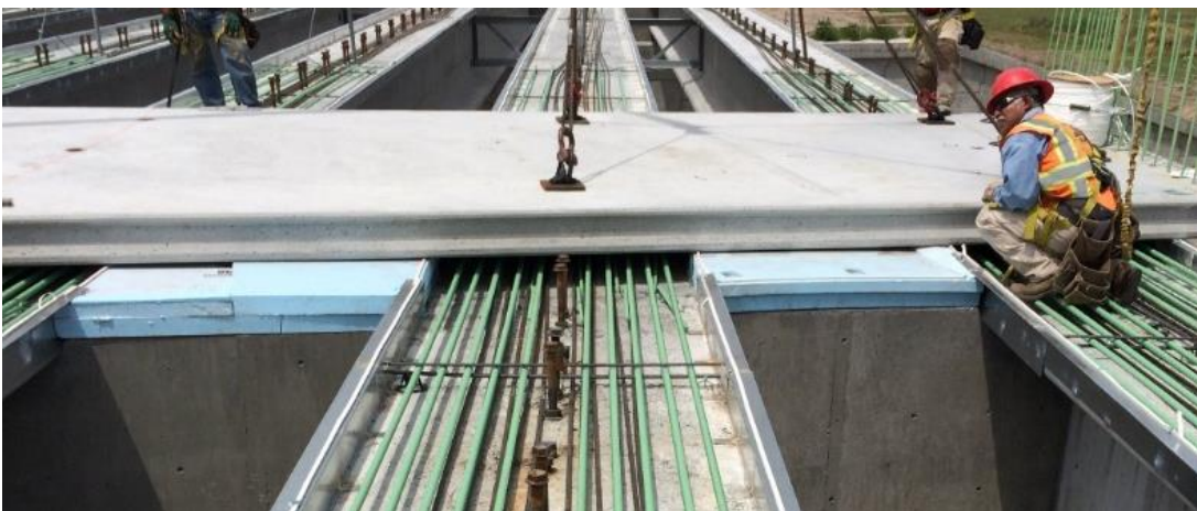
FIGURE 1.4 Deck panel erection
