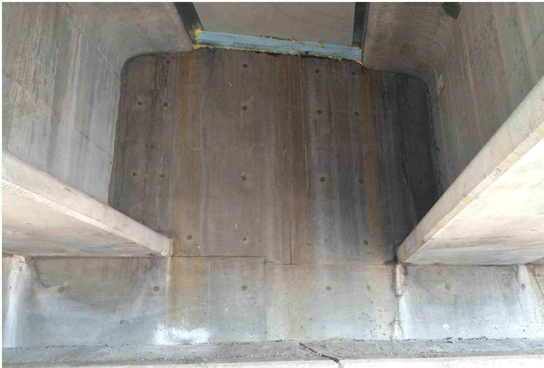
FIGURE 2.5 Girder ends and deck soffit at end diaphragm
