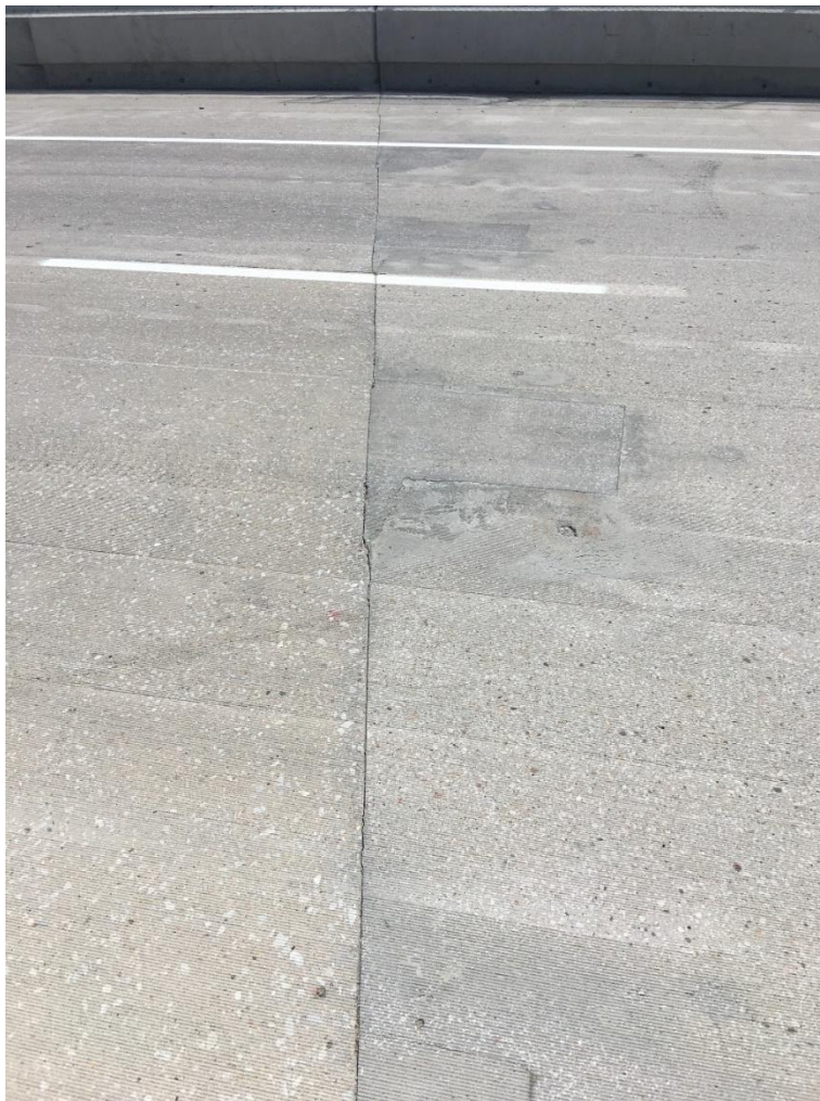
FIGURE 2.17 End panel joint with the approach slab and south anchorage blocks
