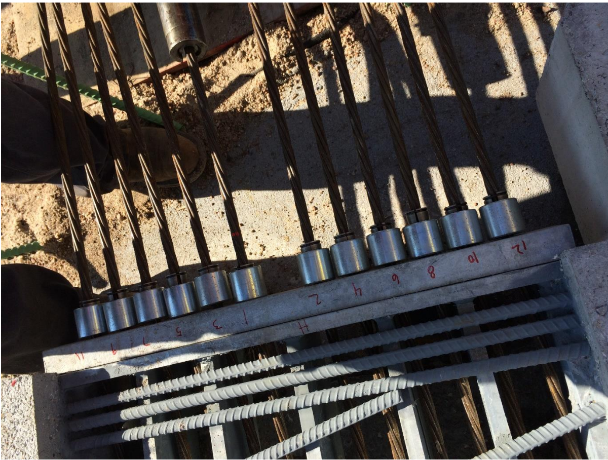
FIGURE 1.6 Post-tensioning the deck panels longitudinally using a new system
