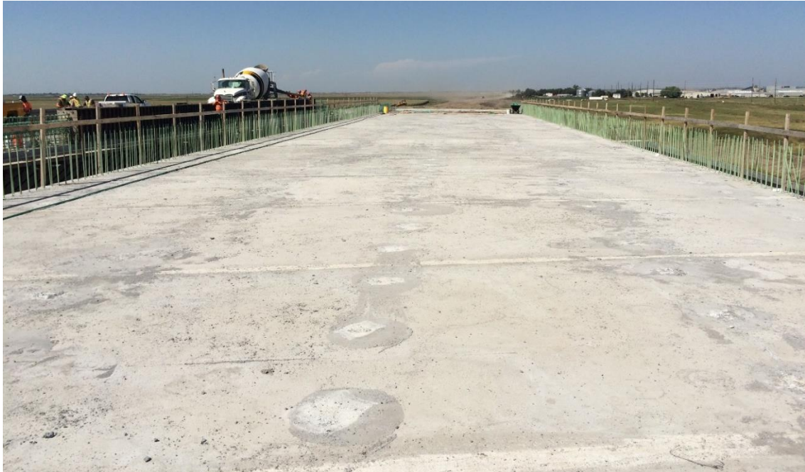
FIGURE 1.7 Precast concrete deck during and after grouting shear pockets and haunches
