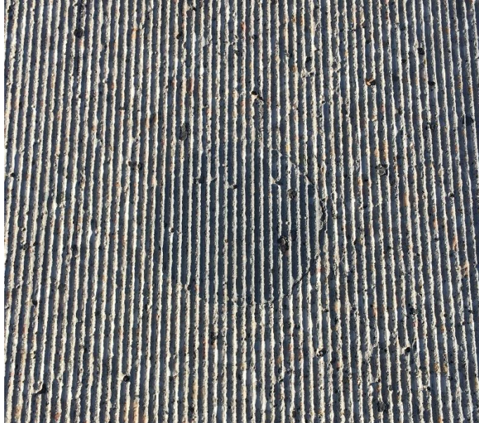
FIGURE 2.8 Grouting hole with fine pour line at its circumference
