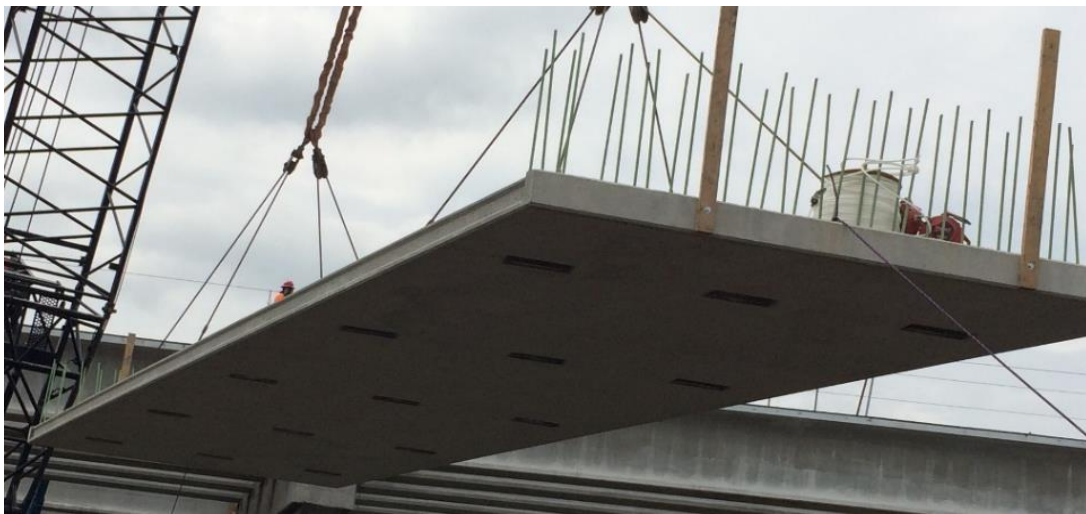
FIGURE 1.3 Deck support system, shear connectors, and PT deviators
