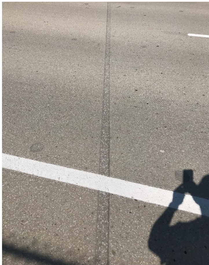
FIGURE 2.27 Pier section transverse joint in precast deck
