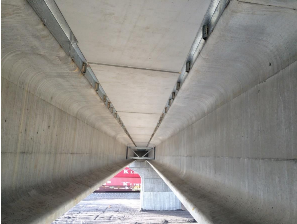
FIGURE 2.4 Underside of the precast concrete deck panels and intermediate diaphragm
