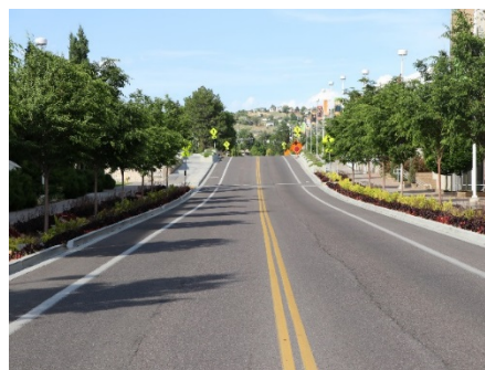
Figure 6: BTPO worked closely with partners to implement improvements through “proof of concept” projects, such as MLK Way above.
