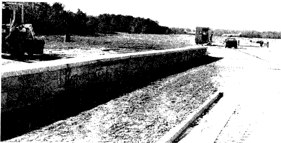
Figure 65. Posttest photographs of median barrier system, test 1818-7-88.
