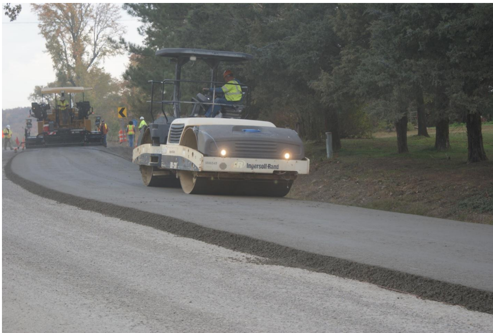
Figure 18. Photo. Larger steel wheel roller (replacing initial light roller) resulting in better compaction and smoother surface.
