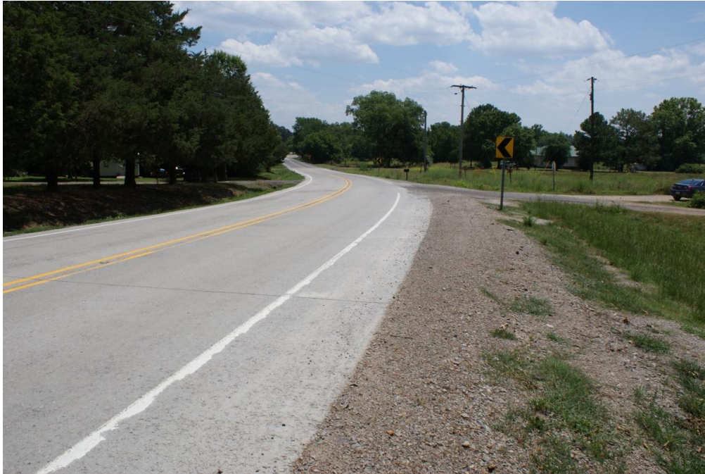
Figure 23. Photo. Completed safety edge after project completion.
