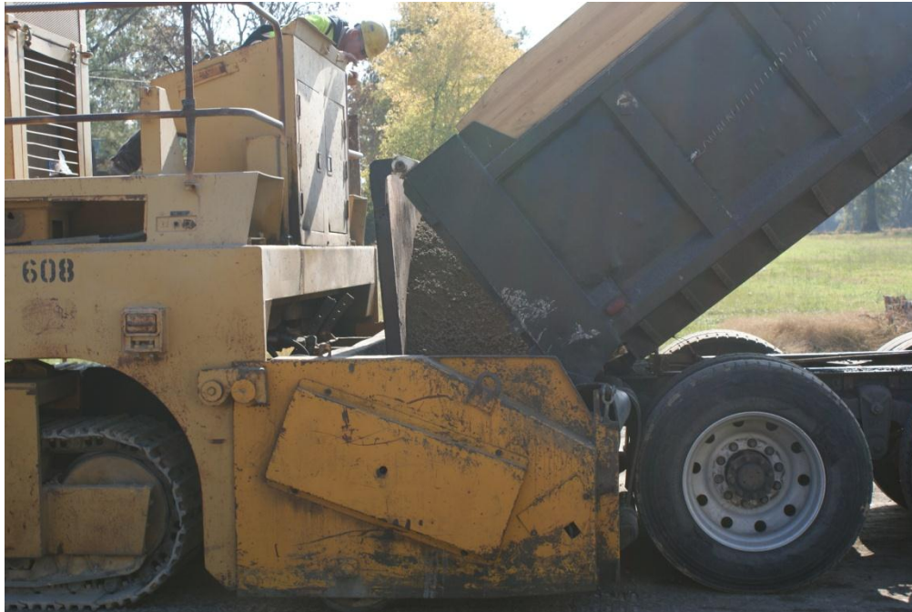
Figure 14. Photo. RCC mix emptied into transfer vehicle.
