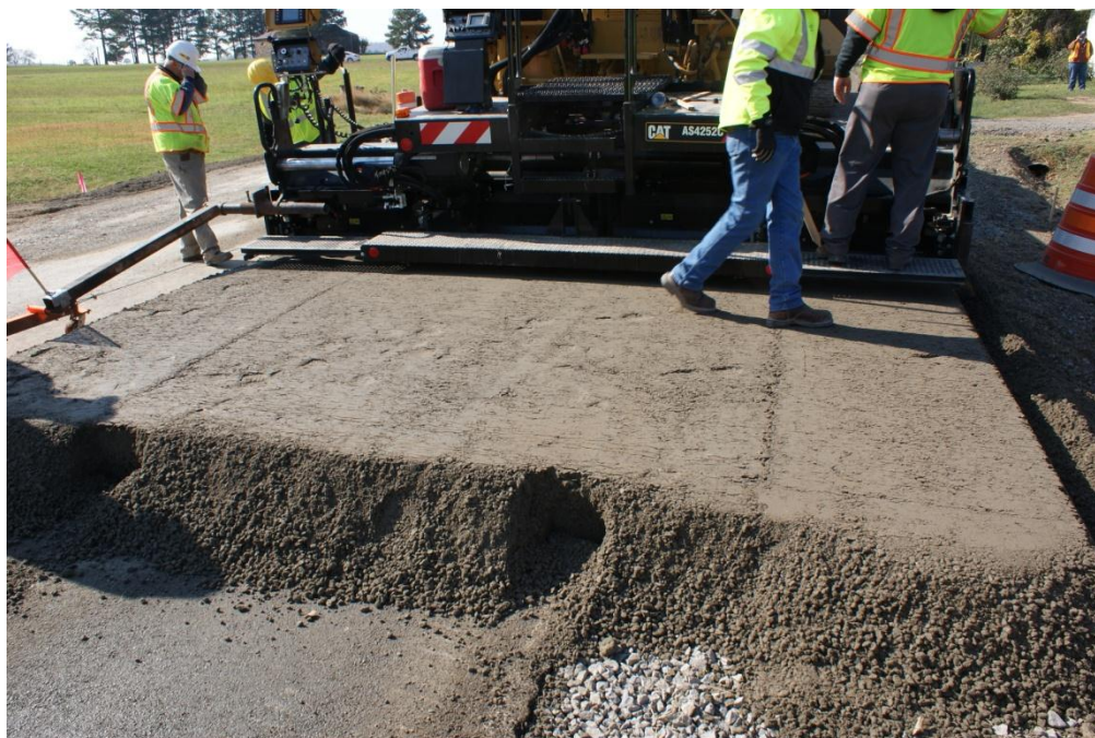
Figure 16. Photo. RCC construction behind paver.
