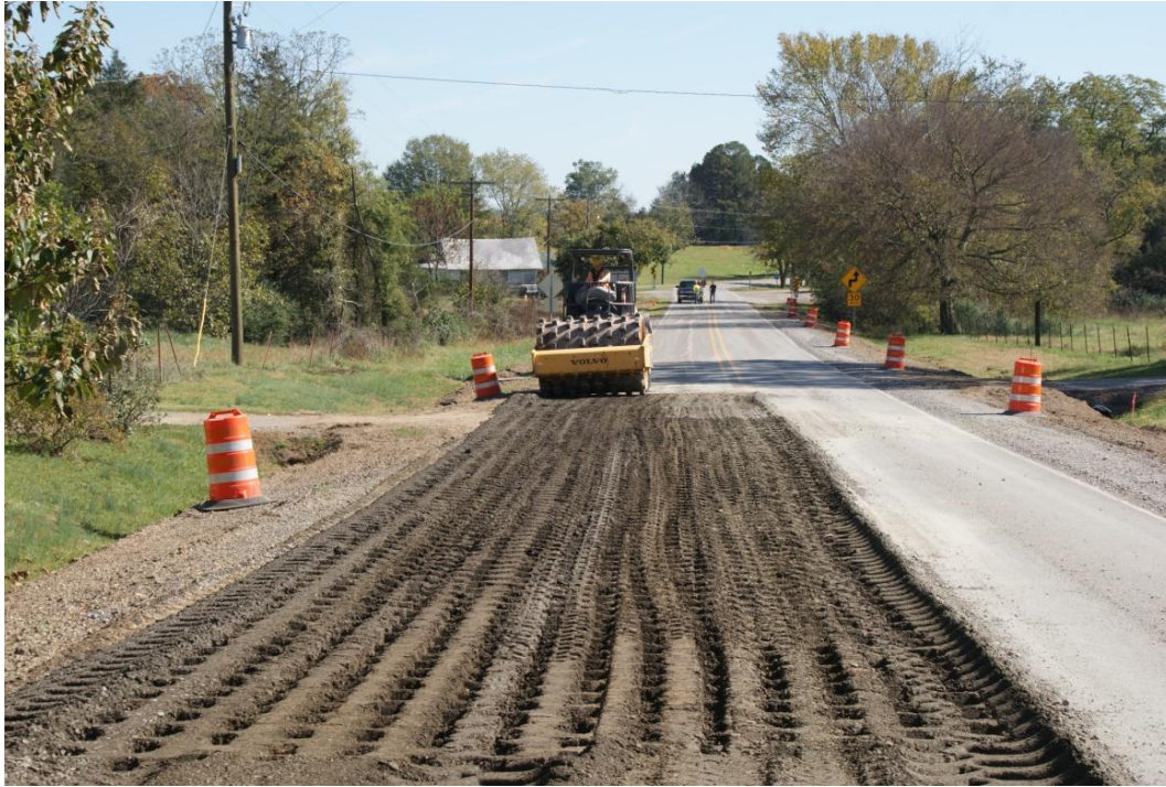
Figure 13. Photo. Cement stabilized material during compaction process.
