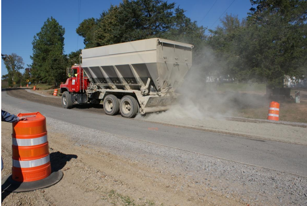
Figure 9. Photo. Application of cement to milled surface.
