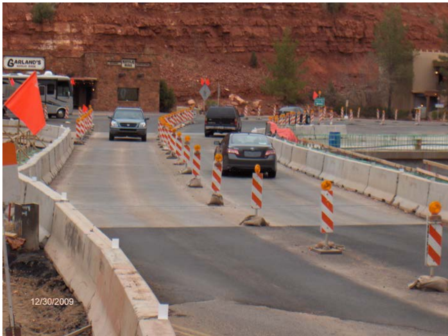
Figure 18. Existing Oak Creek Bridge during construction.
