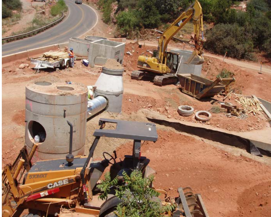
Figure 14. Stormceptors before installation.
