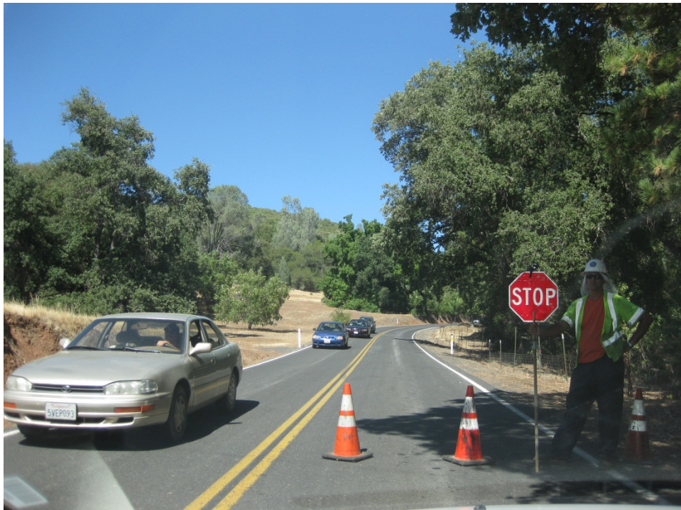
Figure 38. Flaggers halting traffic at the west end of the construction zone.
