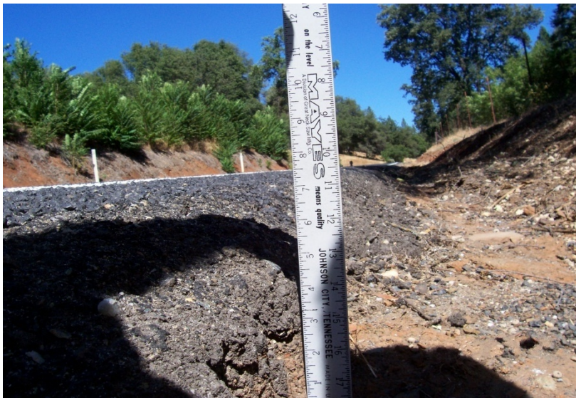
Figure 5. Typical edge-shoulder dropoff on Mountain Ranch Road.
