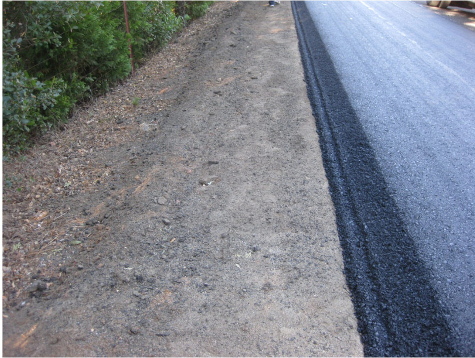
Figure 29. In some locations, the Safety Edge angle was not uniform because of the HMA thickness between the shoulder material and top of the mat compared to the vertical thickness of the Safety Edge shoe.
