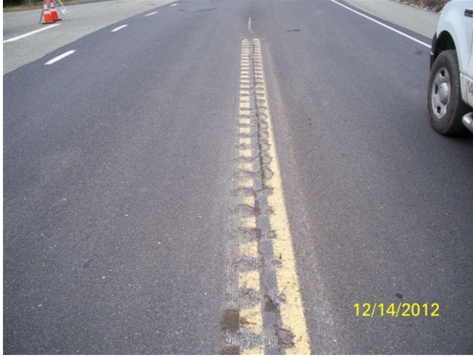
Figure 37. Ground centerline rumble strips.
