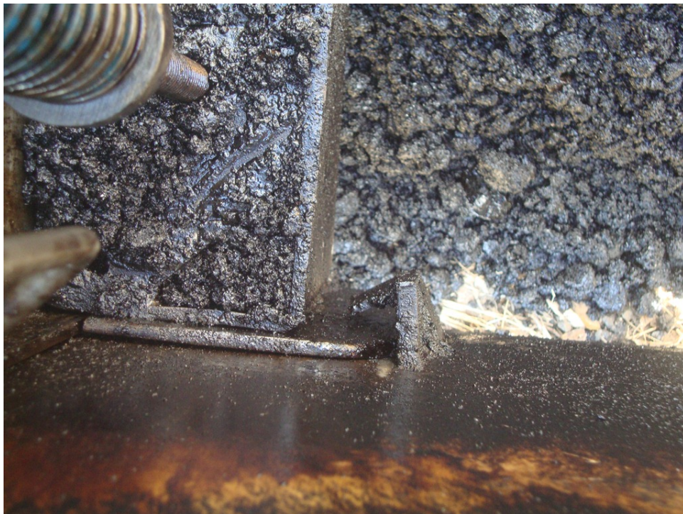
Figure 19. Contractor welded a piece of metal to the Safety Edge shoe and an angled piece to the end gate to prevent HMA from getting between the shoe and the end gate.
