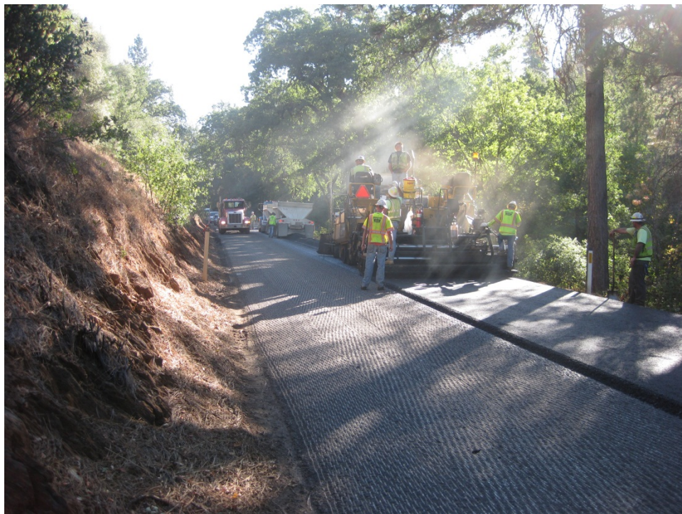
Figure 13. Paving Mountain Ranch Road.
