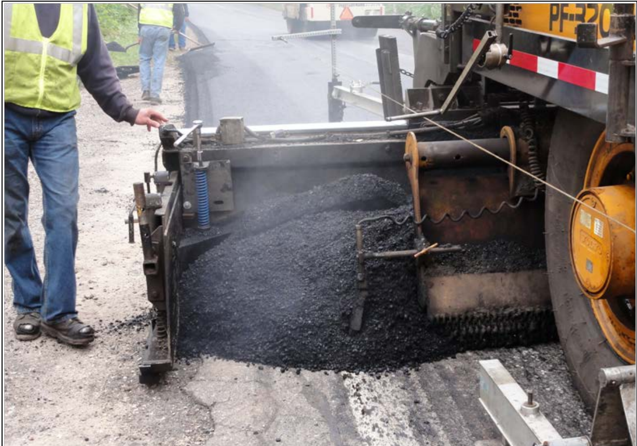
Figure 8. Paving with the Carlson prototype #2 device with the TransTech device is still attached but raised and out of the way.
