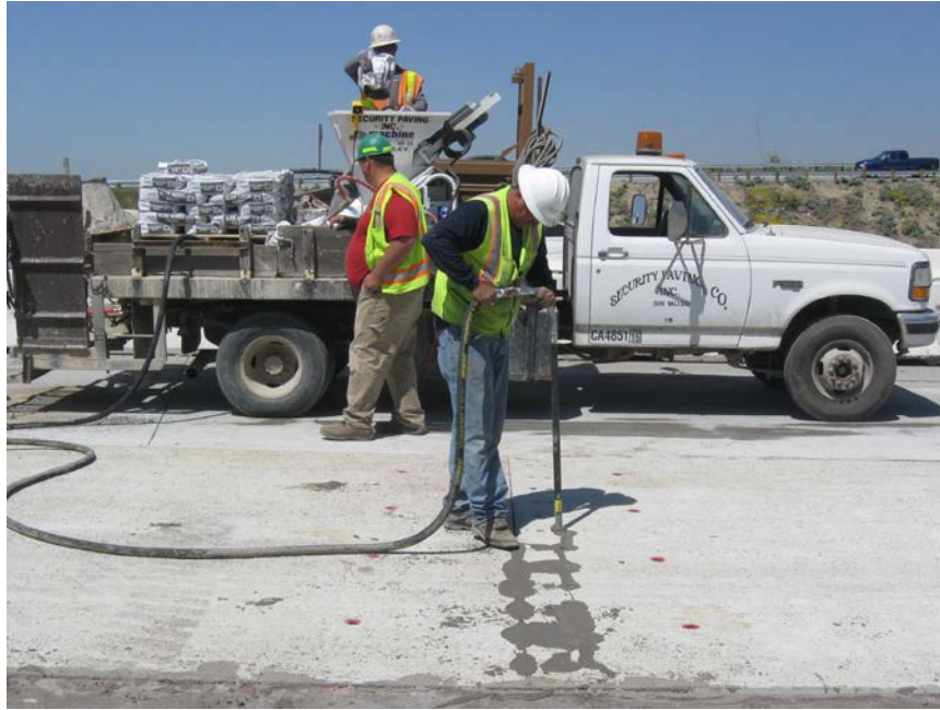
Figure 18. Grouting operation.
