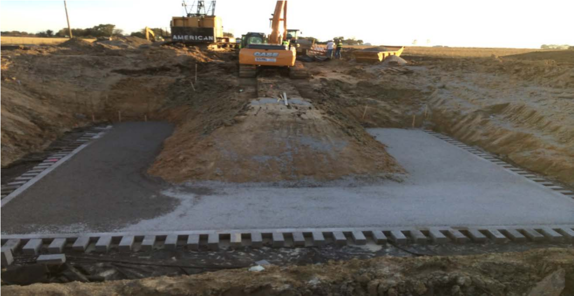
Figure 12. Photo. First row of blocks completed (courtesy: LADOTD).
