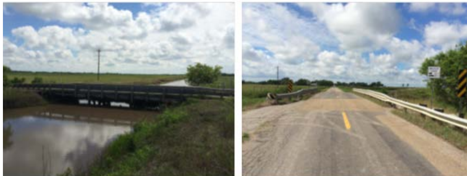
Site 2 Bridge over Maree Michel Creek
