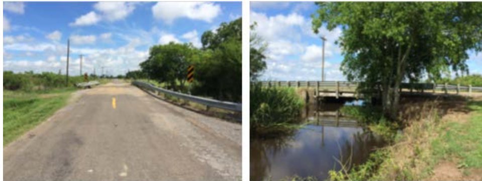
Site 1 Bridge over Unnamed Creek
