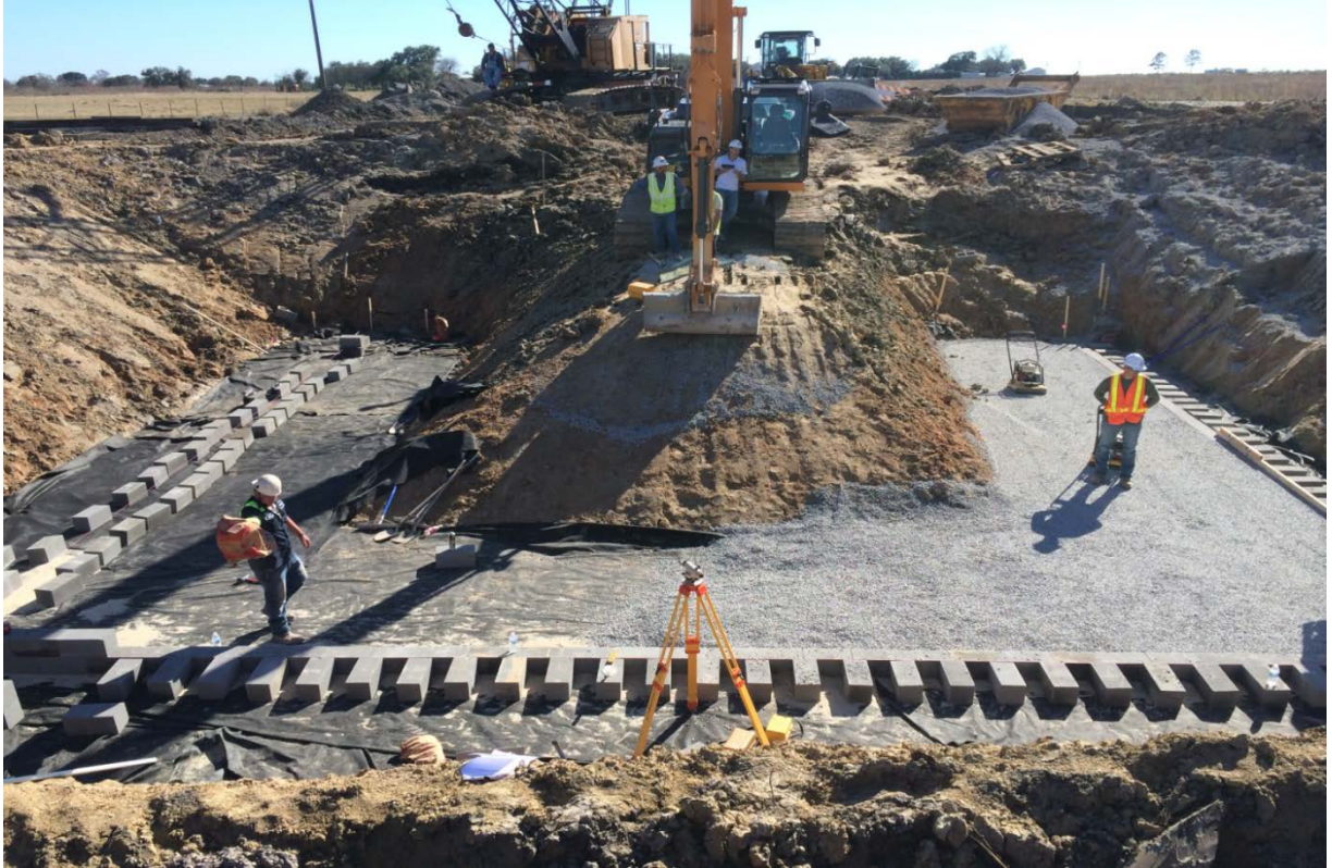
Figure 11. Photo. Installation of first row of blocks (courtesy: LADOTD).
