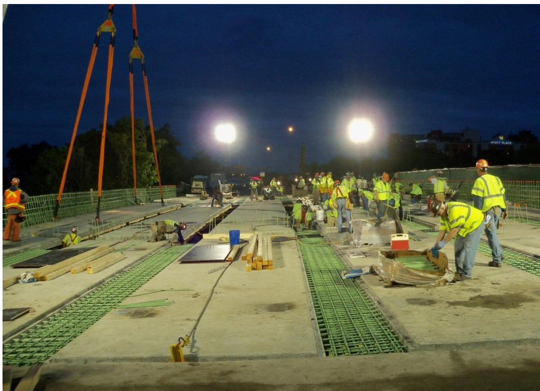
Figure 5. Photo. Wider closure pour for bridge decks.
