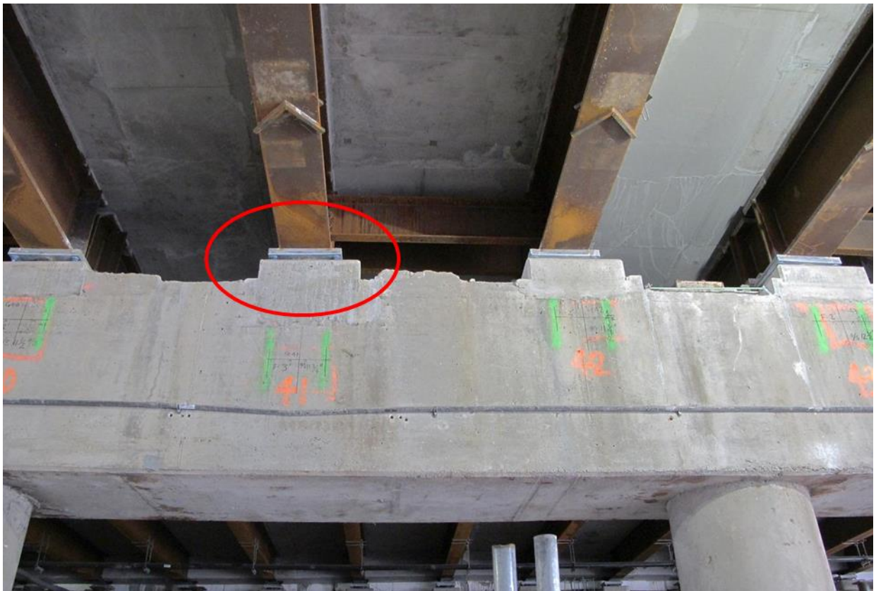
Figure 17. Photo. Pedestal placement for beam seats.
