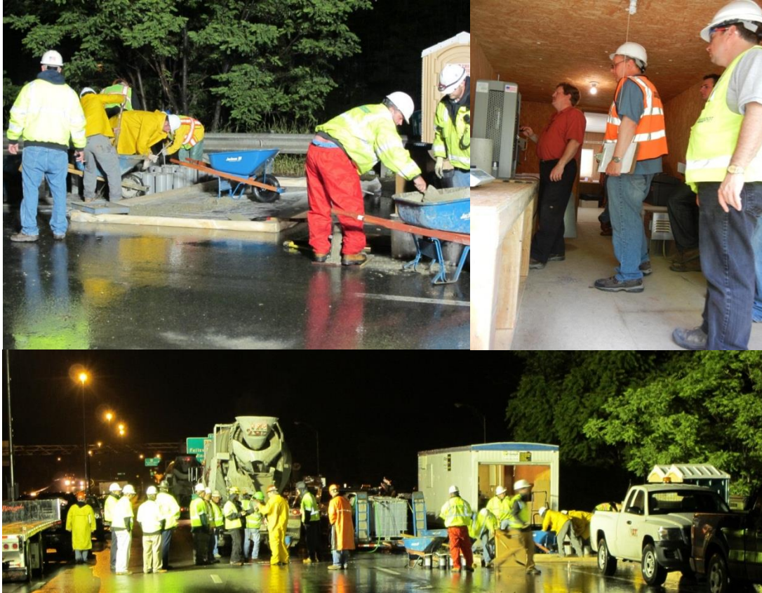
Figure 42. Photo. Mobile laboratory at project site.
