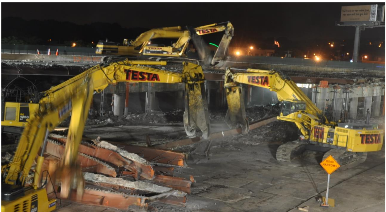
Figure 18. Photo. Demolition of existing bridge superstructure.
