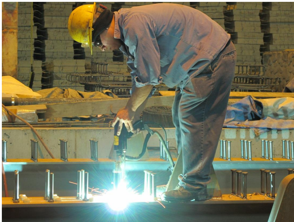
Figure 10. Photo. Shear stud welding.
