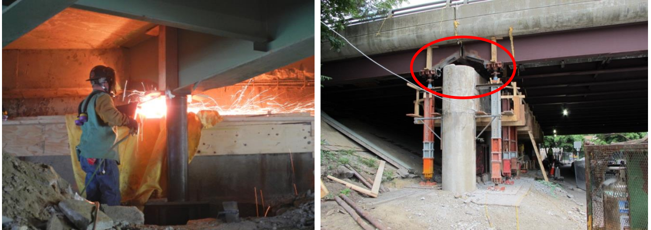
Figure 16. Photo. Shoring and coping of beam ends.
