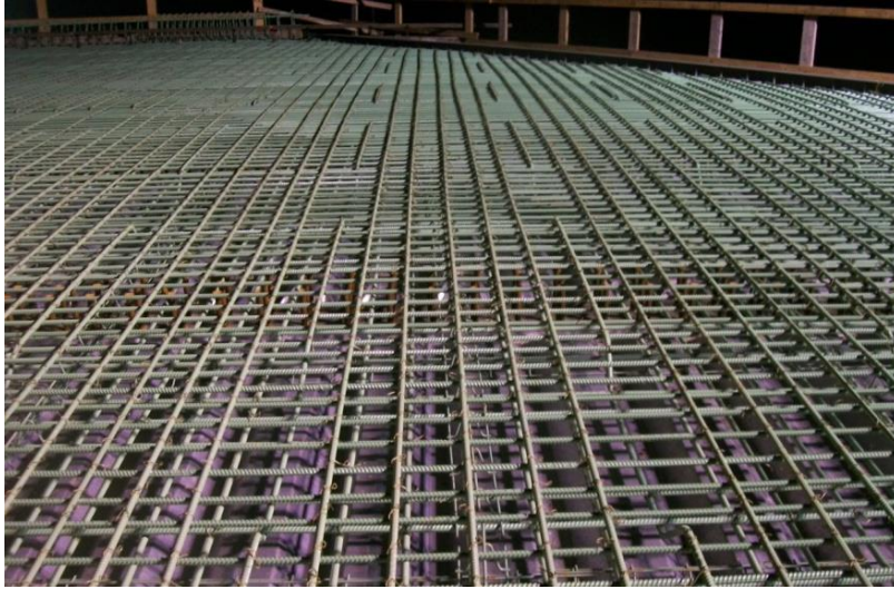
Figure 26. Deck reinforcement.
