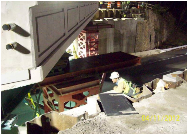
Figure 33. New superstructure being maneuvered into place on abutment.
