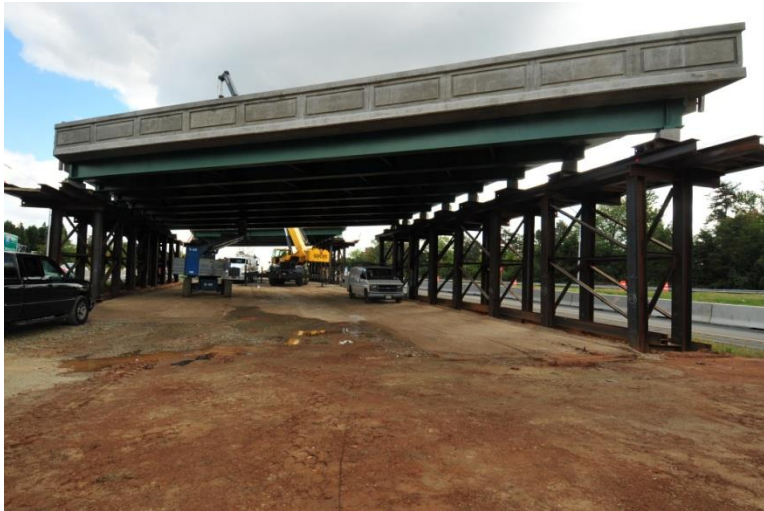
Figure 32. Completed new superstructure in median.
