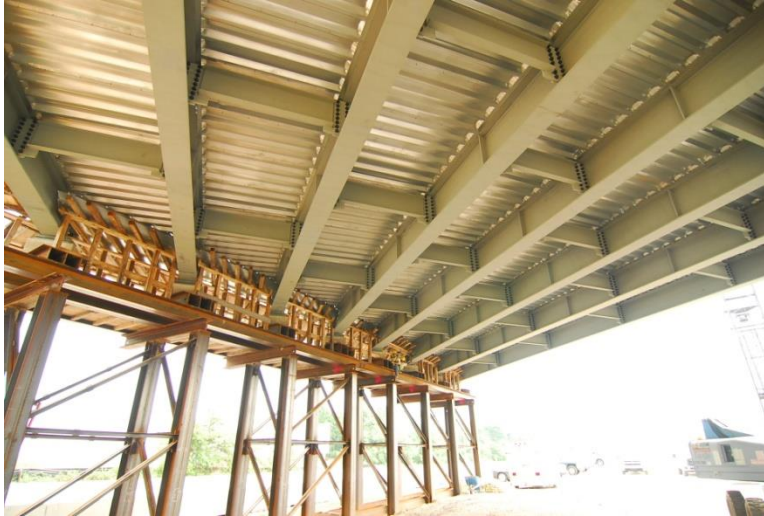
Figure 22. Superstructure in median before placement of deck concrete.
