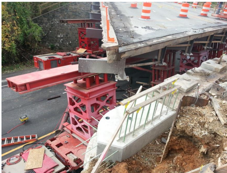
Figure 17. SPMT supporting old superstructure.
