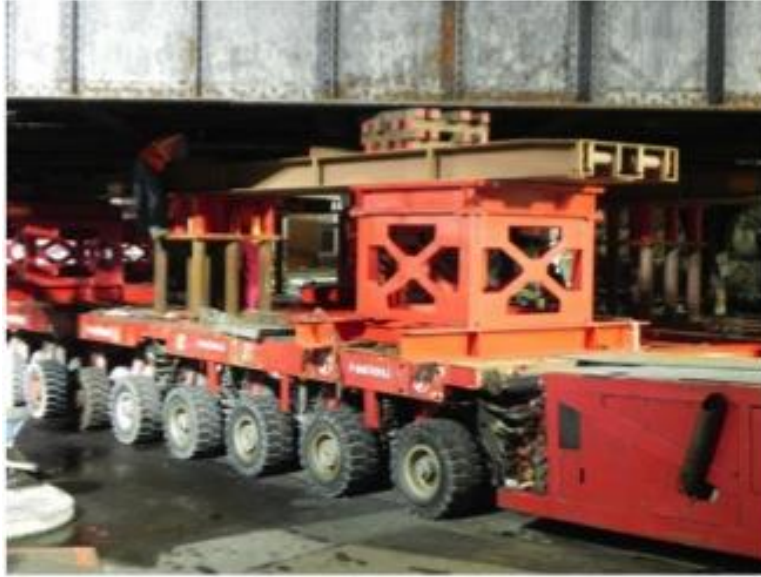
Figure 16. SPMT with multiple wheels supporting structure.
