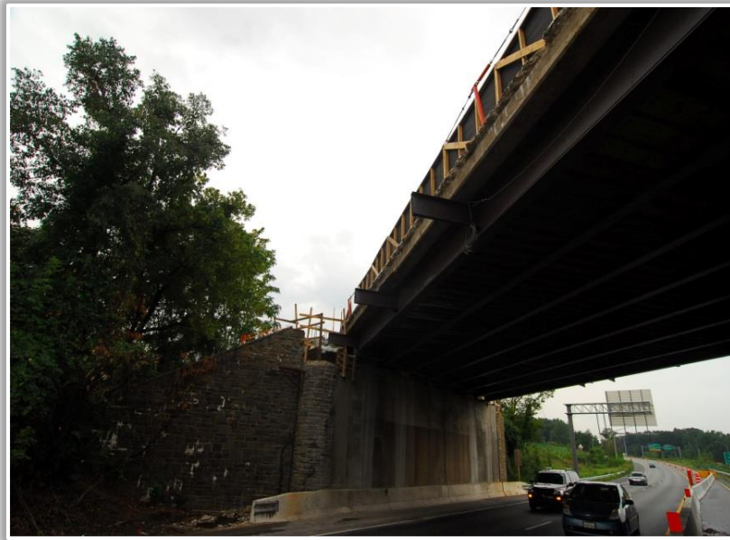
Figure 13. Modification of pilasters and end posts in process.
