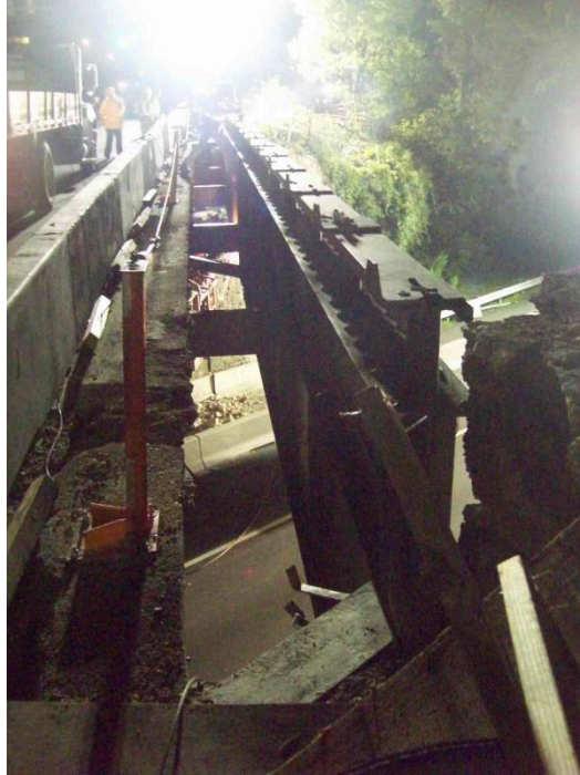
Figure 24. Fascia beam ready for removal.
