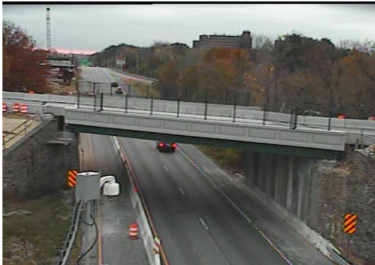
Figure 34. New superstructure in place on abutment.
