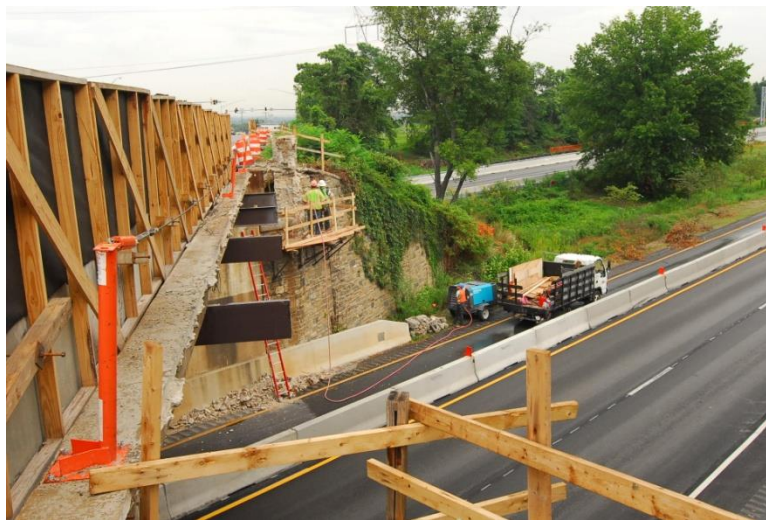
Figure 29. Existing superstructure with fascia beams removed.
