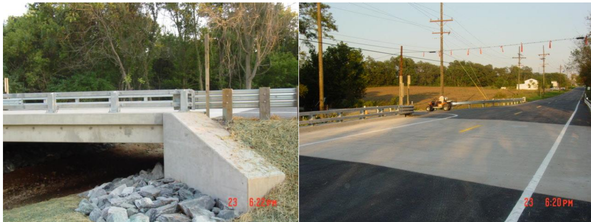
Figure 20. New condition of replaced MD 28 bridge over Washington Run.
