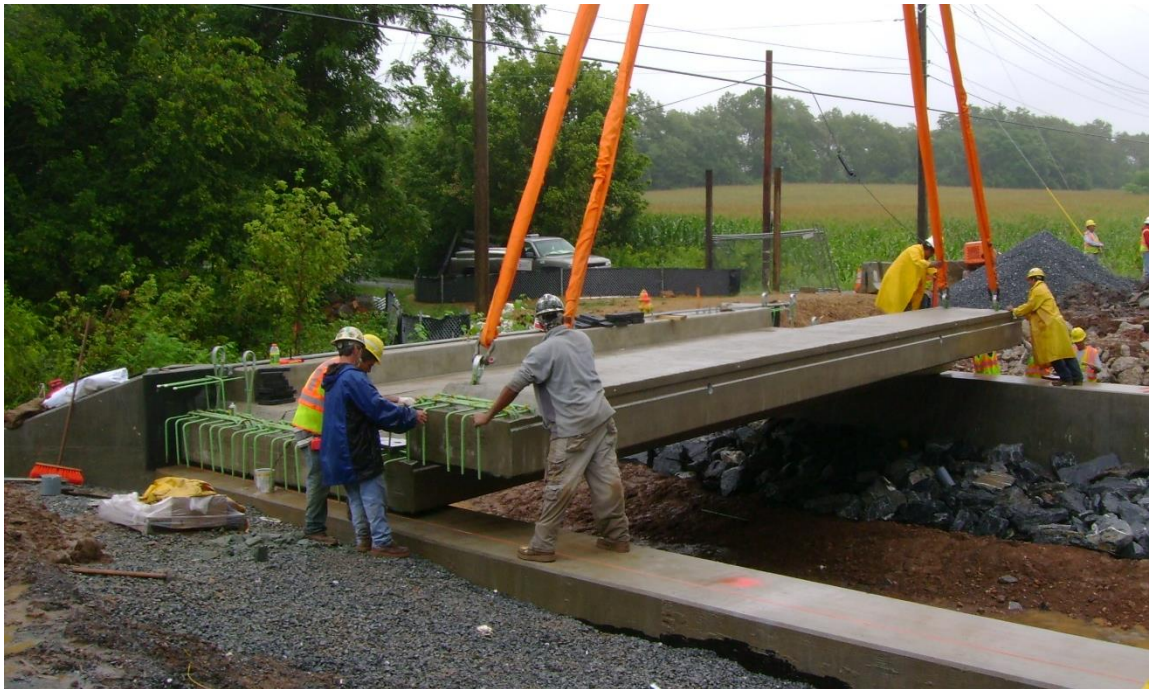
Figure 9. Crane placement of Slab No. 4 at MD 28 project.
