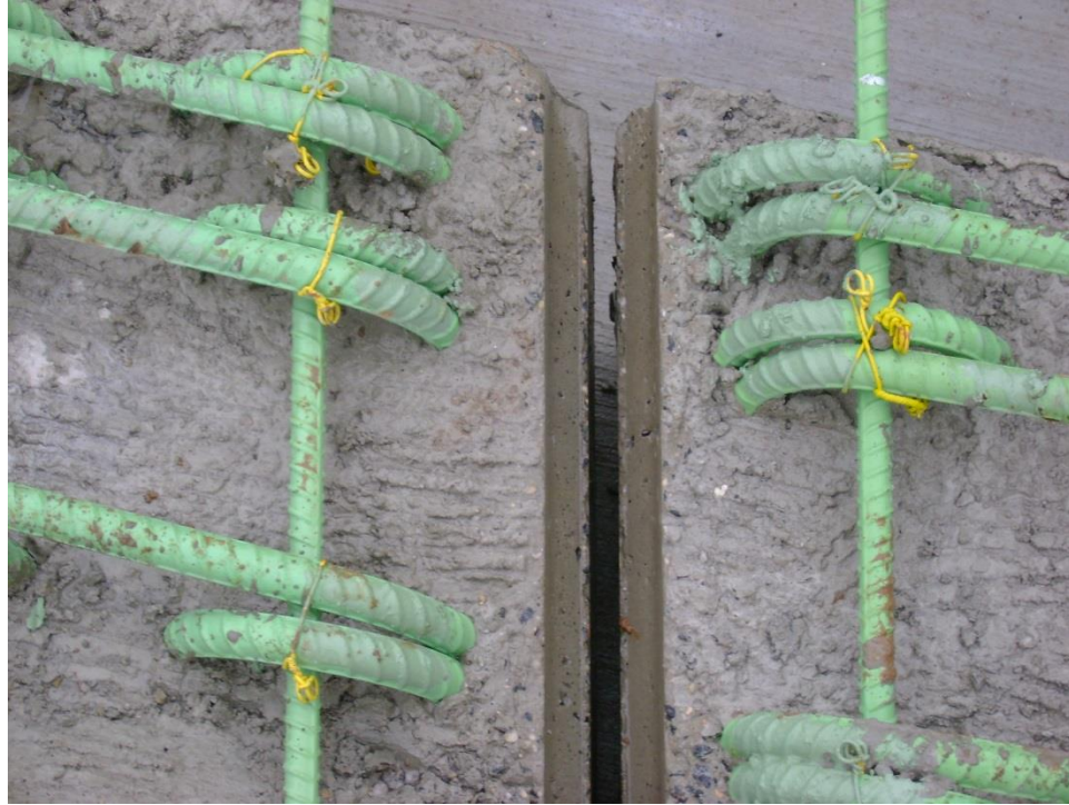
Figure 14. Aerial view of shear key at end of beams.
