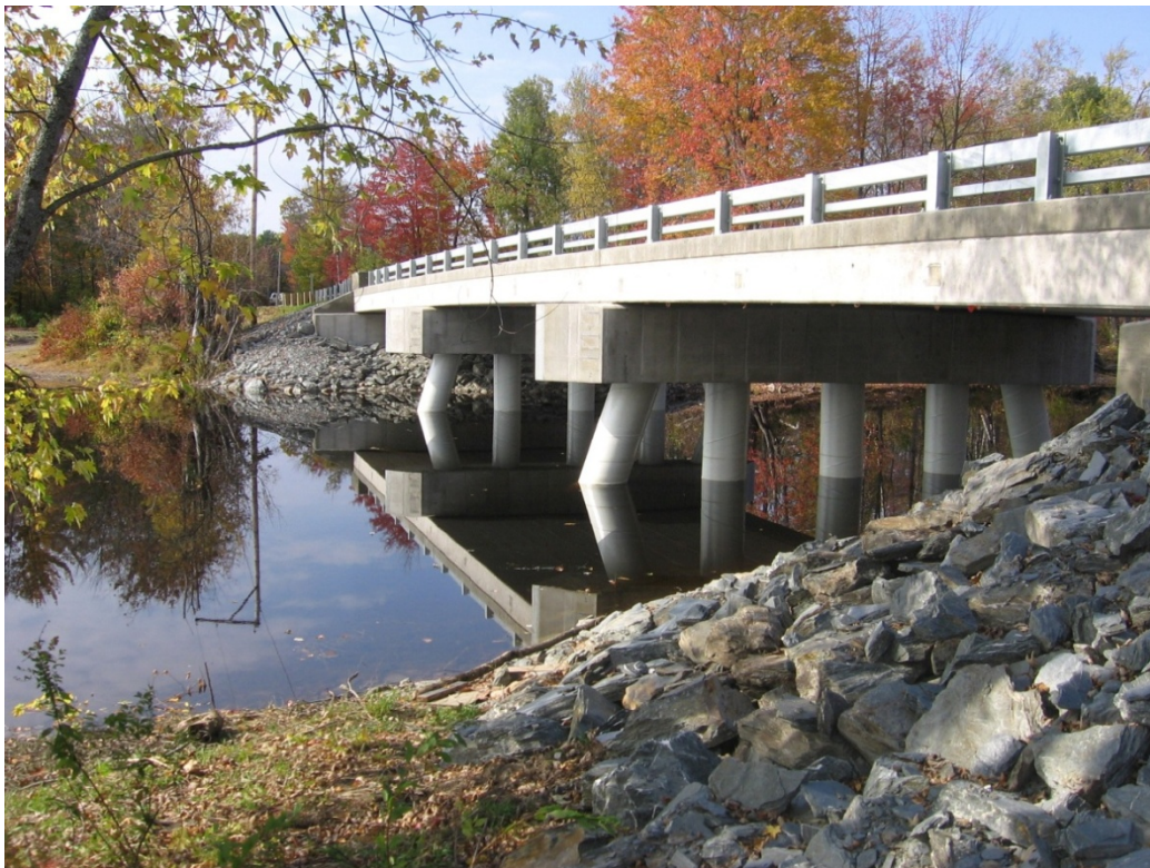
Figure 18. The completed Boom Birch Bridge.
