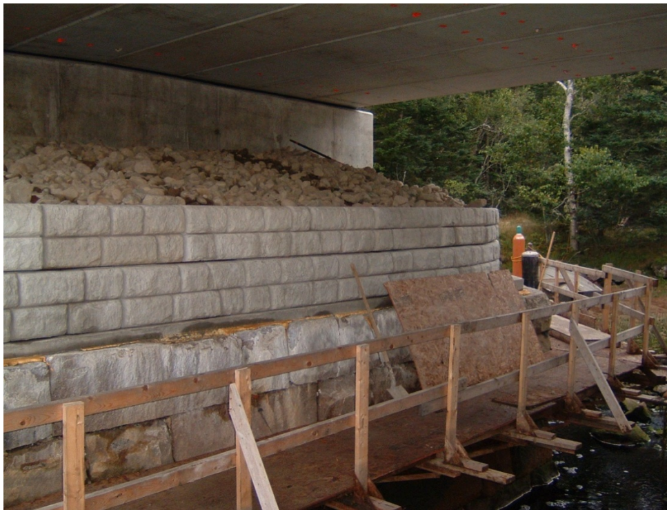
Figure 6. The Lamson Bridge Project maintained and preserved the existing cut stone block wall (on the bottom) for historic and environmental reasons.
