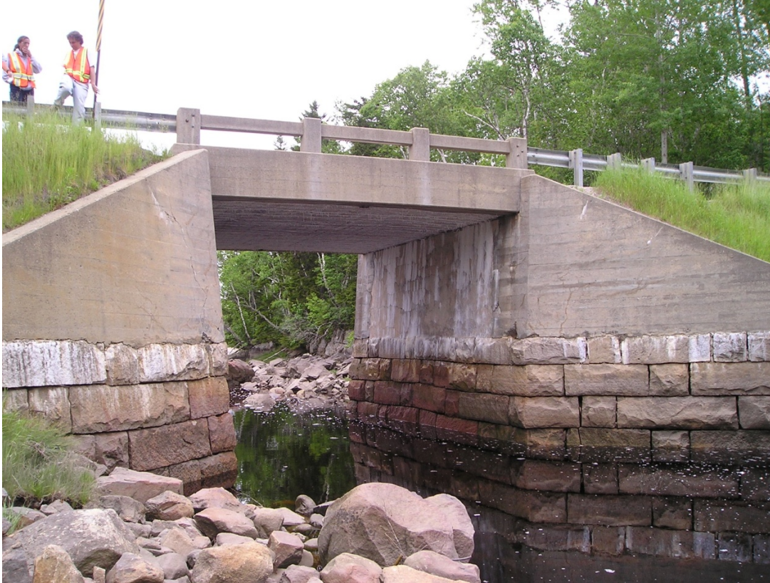
Figure 2. The Lamson Bridge was constructed in the 1930's.
