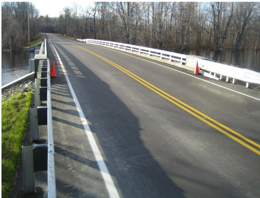
Figure 26. Boom Birch post-construction pavement.
