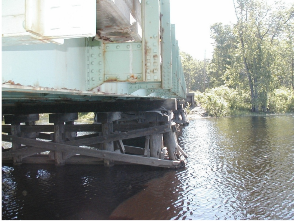
Figure 12. The Boom Birch Bridge was constructed in the late 1930's.
