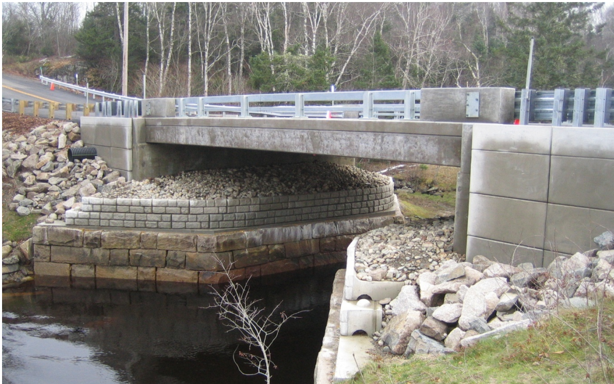
Figure 11. The completed Lamson Bridge Project.
