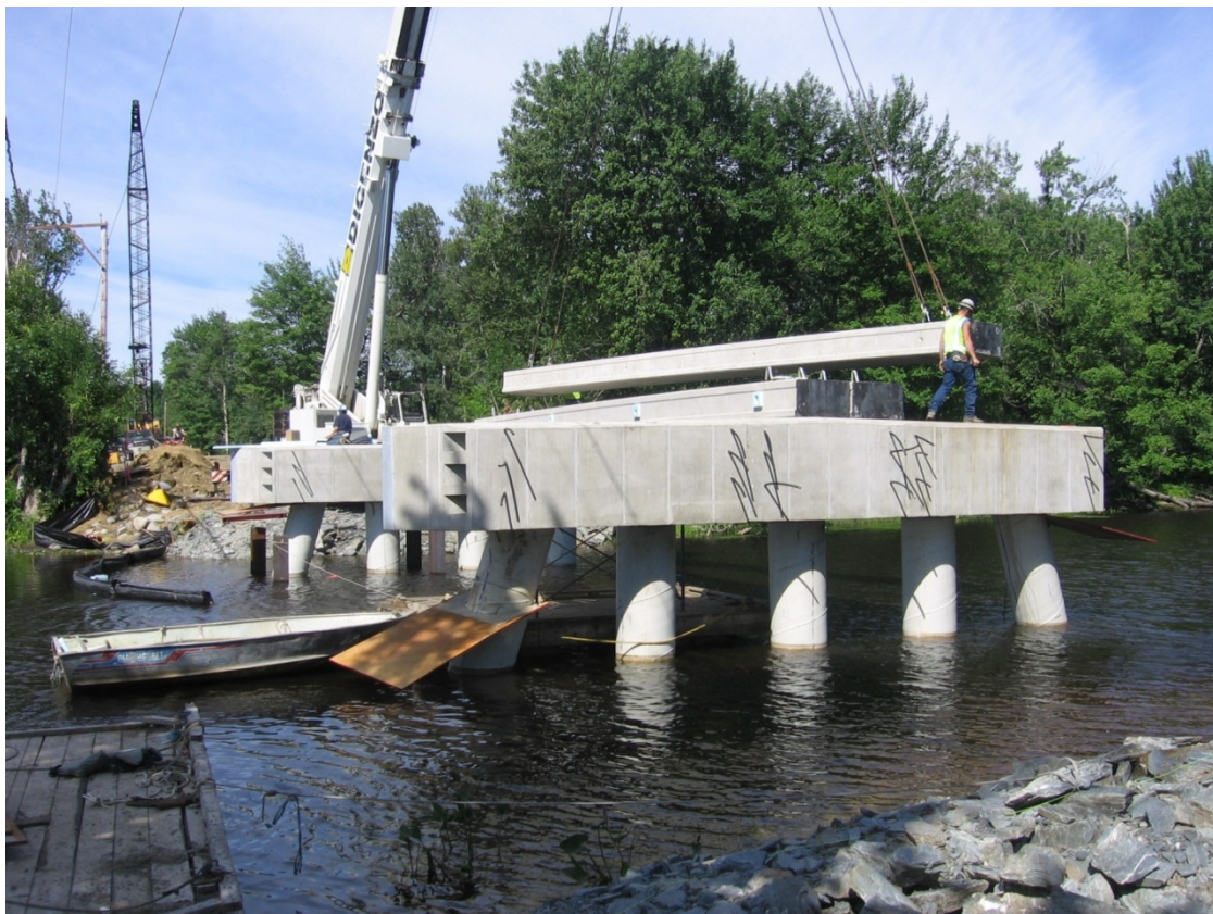
Figure 17. Placement of the superstructure beams.
