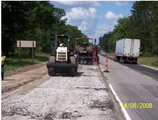
Figure 24. Seating the rubblized pavement.
