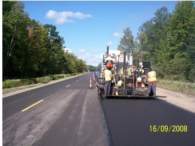
Figure 26. 4E3 leveling application.
