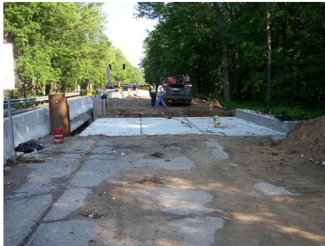
Figure 16. Bridge elements set to grade.
