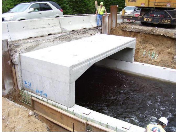
Figure 15. Final placement of a precast bridge element.
