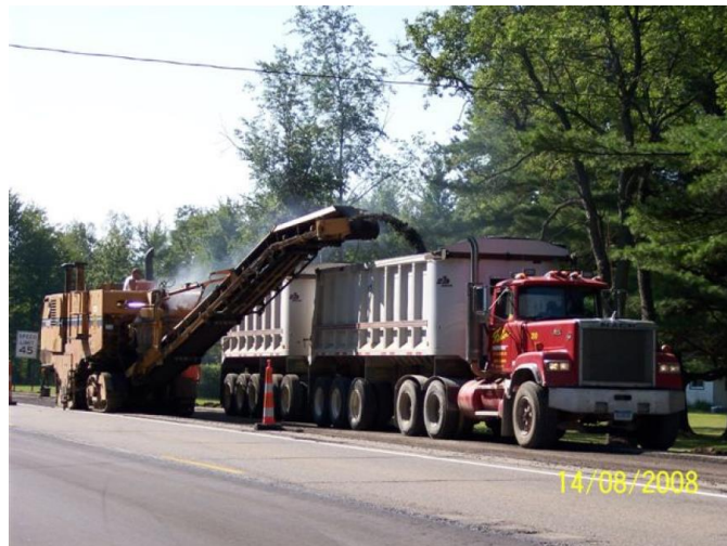
Figure 22. Milling the existing HMA.
