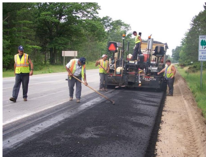
Figure 19. Widening of shoulders to provide two-way temporary lanes.
