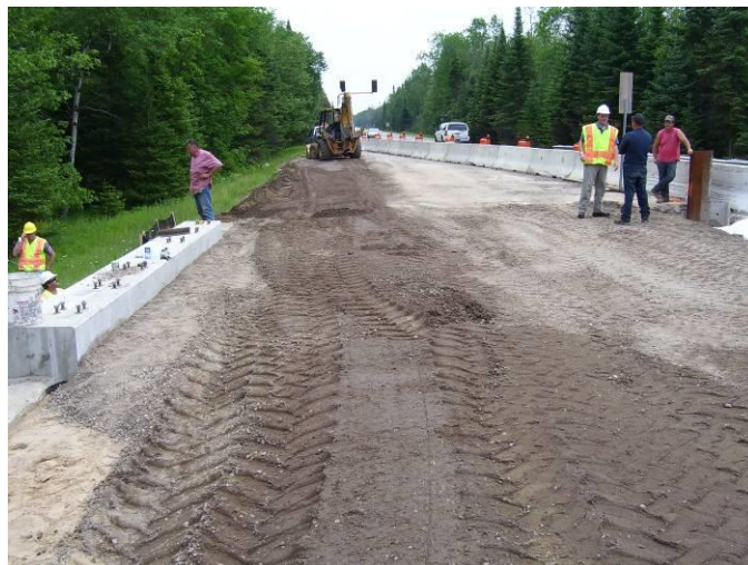
Figure 17. Grading the bridge elements in preparation for placing the HMA layers.
