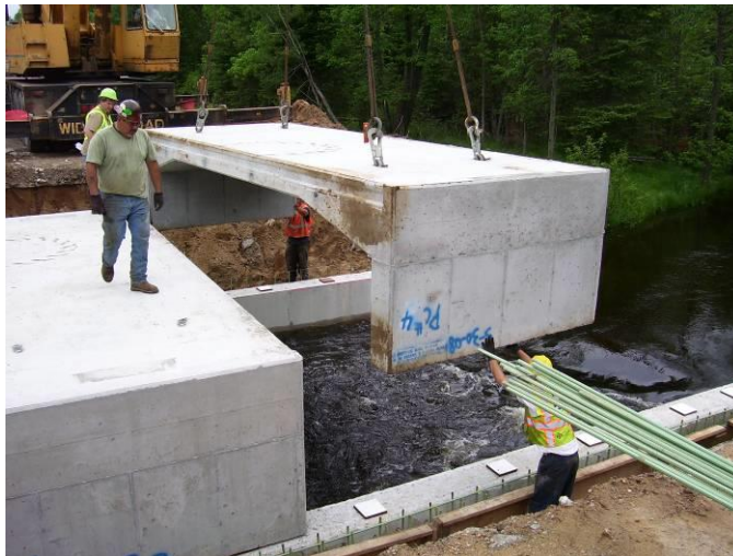
Figure 13. Moving the precast bridge element into place.
