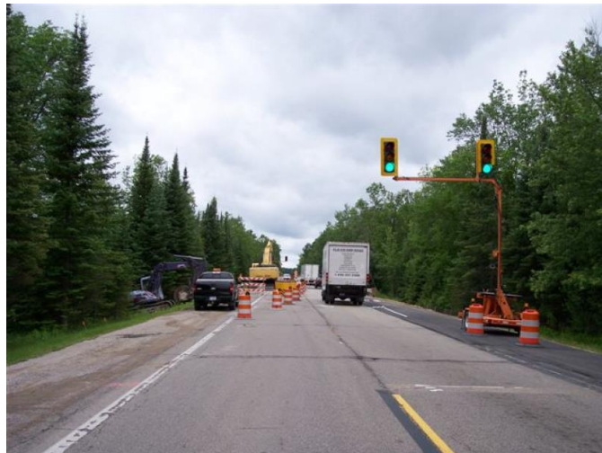
Figure 11. Controlling one-lane traffic using self-adjusting temporary traffic signals.
