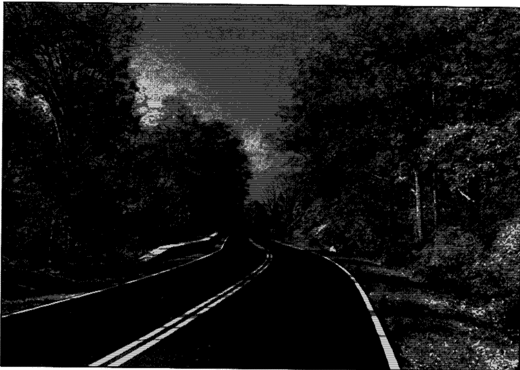
Skyline Drive, Shenandoah National Park, Virginia — Pavement and guardwall reconstruction
