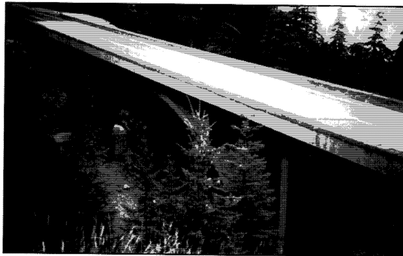
Deadwood Creek Bridge
