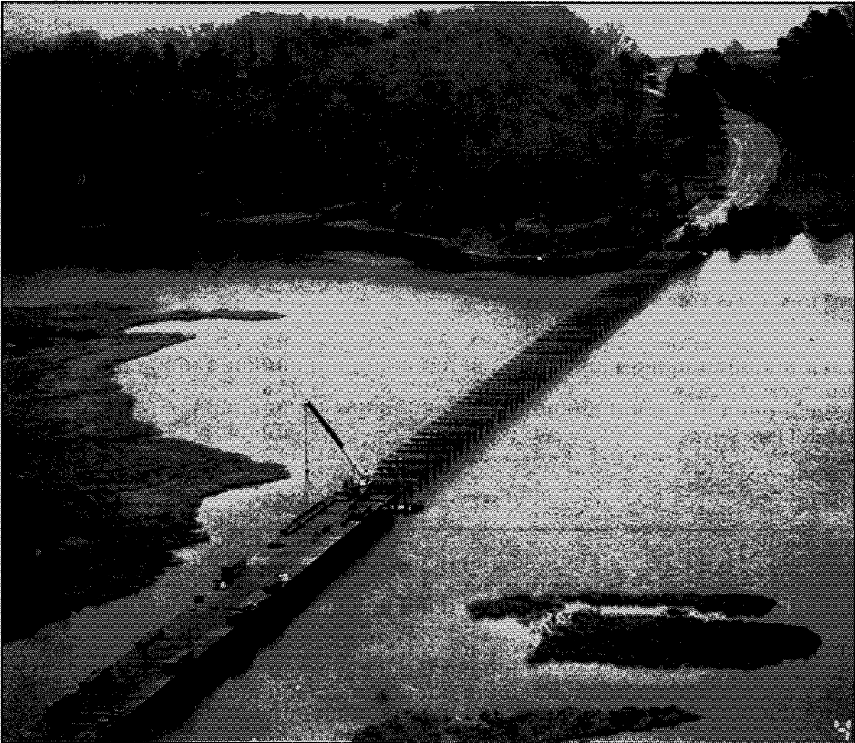
Patuxent Naval Air Station Cedar Point Bridge
