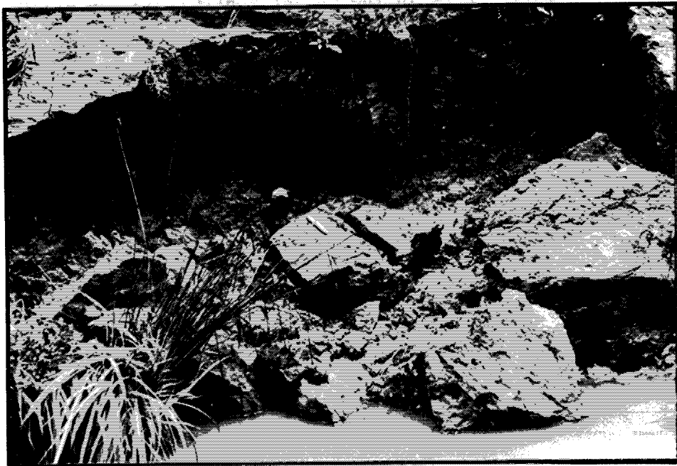
Exhibit 61. Embankment erosion.
