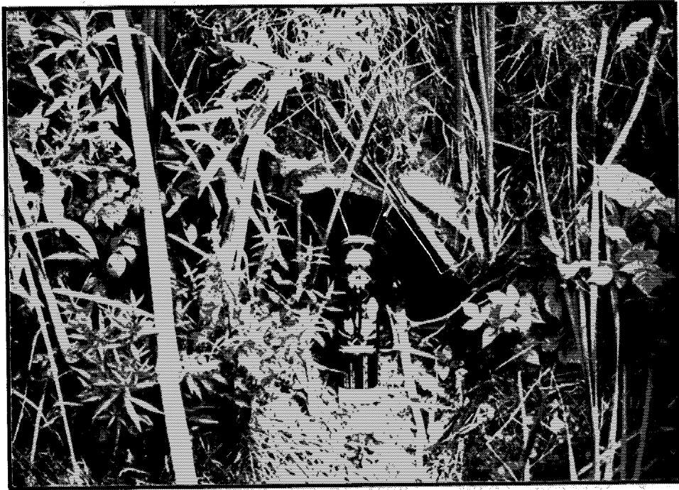
Exhibit 64. Culvert almost completely blocked by sediment accumulation.
