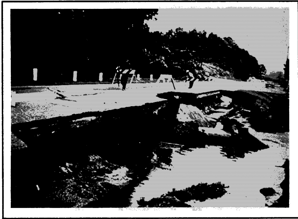
Exhibit 15. Roadway overtopping due to culverts with inadequate capacity may result in extensive damage to the roadway and the embankment.
