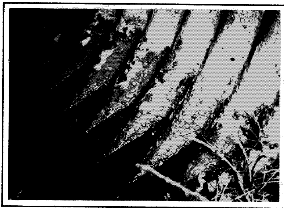
Exhibit 27. Severe corrosion of corrugated steel culvert due to aggressive water.
