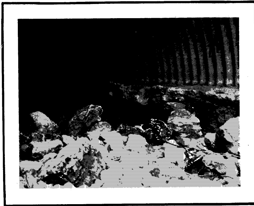
Exhibit 78. Erosion of invert undermining footing of arch.
