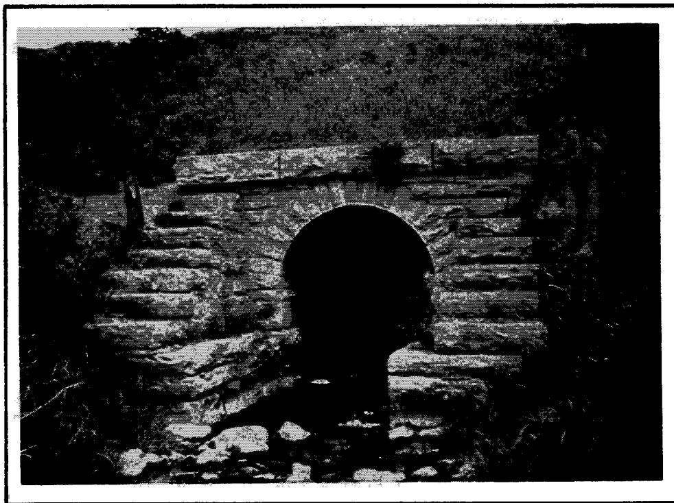
Exhibit 13. Masonry arch culvert. In some areas masonry arches and masonry box culverts are common. With good foundations these culverts have long service lives.
