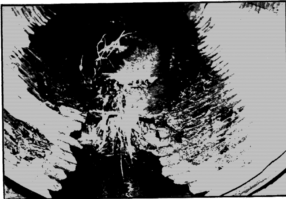
Exhibit 75. Invert deterioration.
