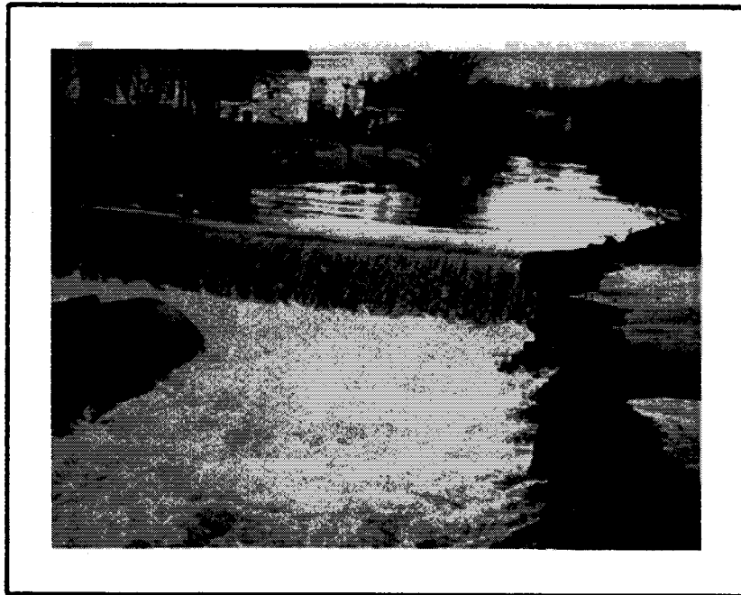
Exhibit 5. Roadway and embankment wash-out.
