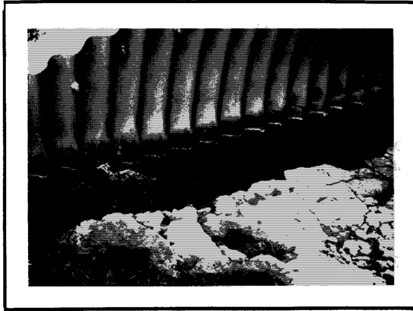
Exhibit 79. Erosion damage to concrete invert.
