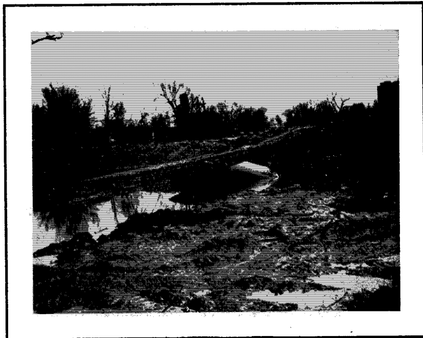
Exhibit 55. Mitered end of culvert turned up due to buoyant forces.
