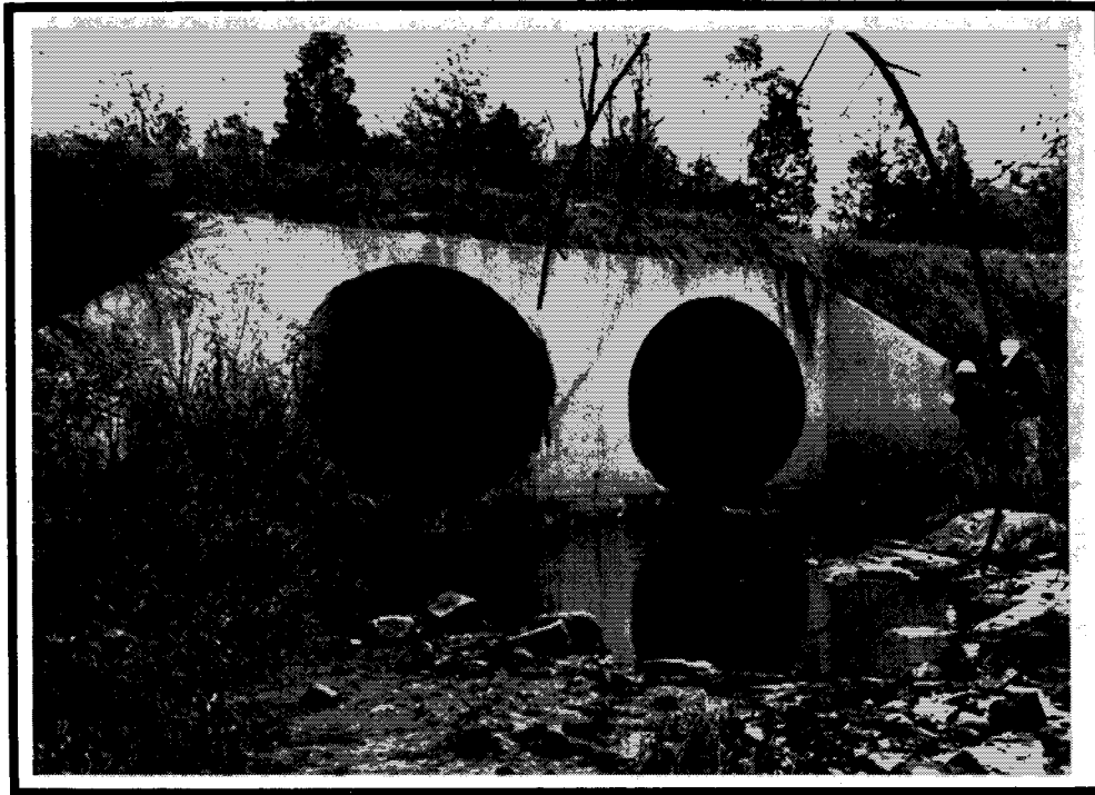
Exhibit 42. Headwall and wingwall end treatment.
