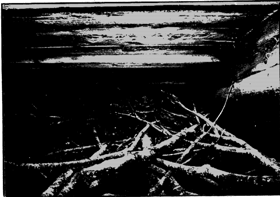
Exhibit 65. Drift and debris inside timber box culvert.
