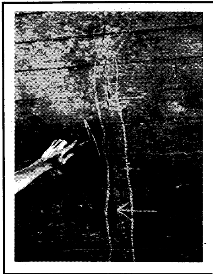
Exhibit 115. Transverse crack in wall of reinforced concrete box culvert.
