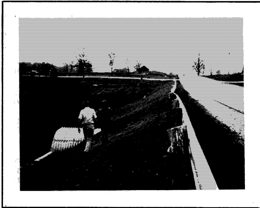
Exhibit 44. A dip in the guardrail or approach roadway may be due to excessive deflection in culvert.
