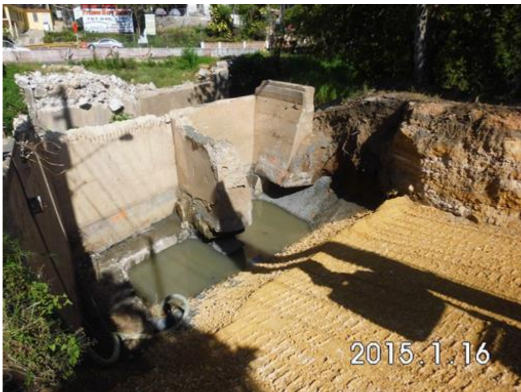
Figure 6. Photo. Excavation of east abutment.
