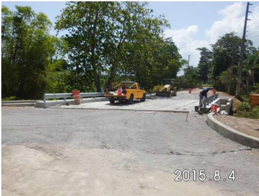
Figure 11. Photo. New Bridge No. 1828 after completion of void slab install.
