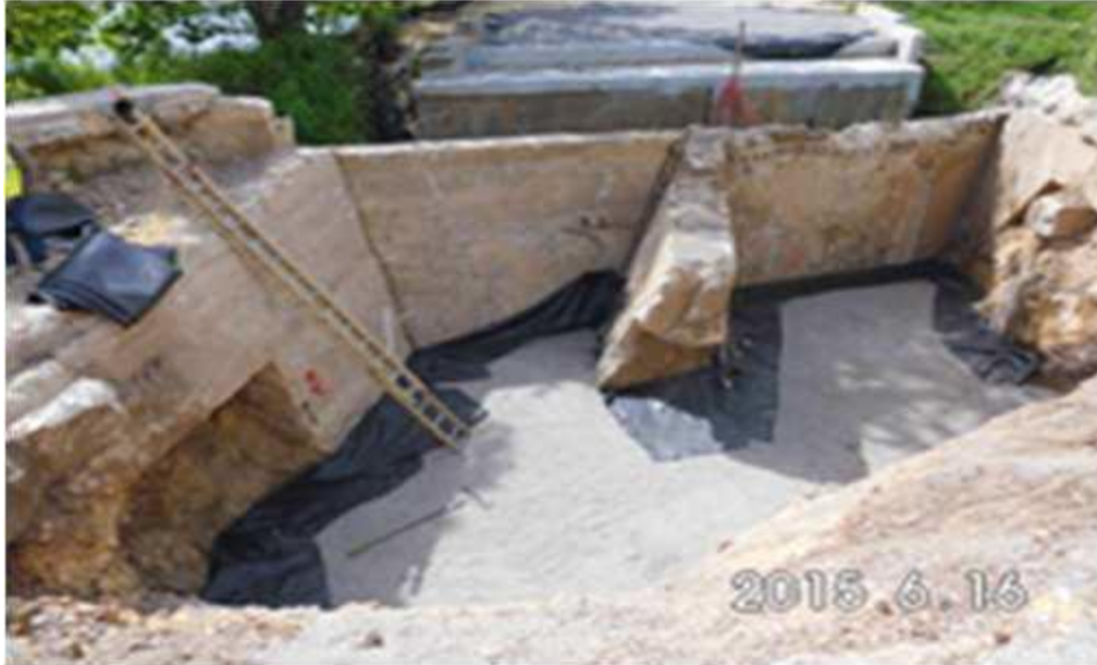
Figure 9. Photo. Construction of GRS-IBS on west abutment.
