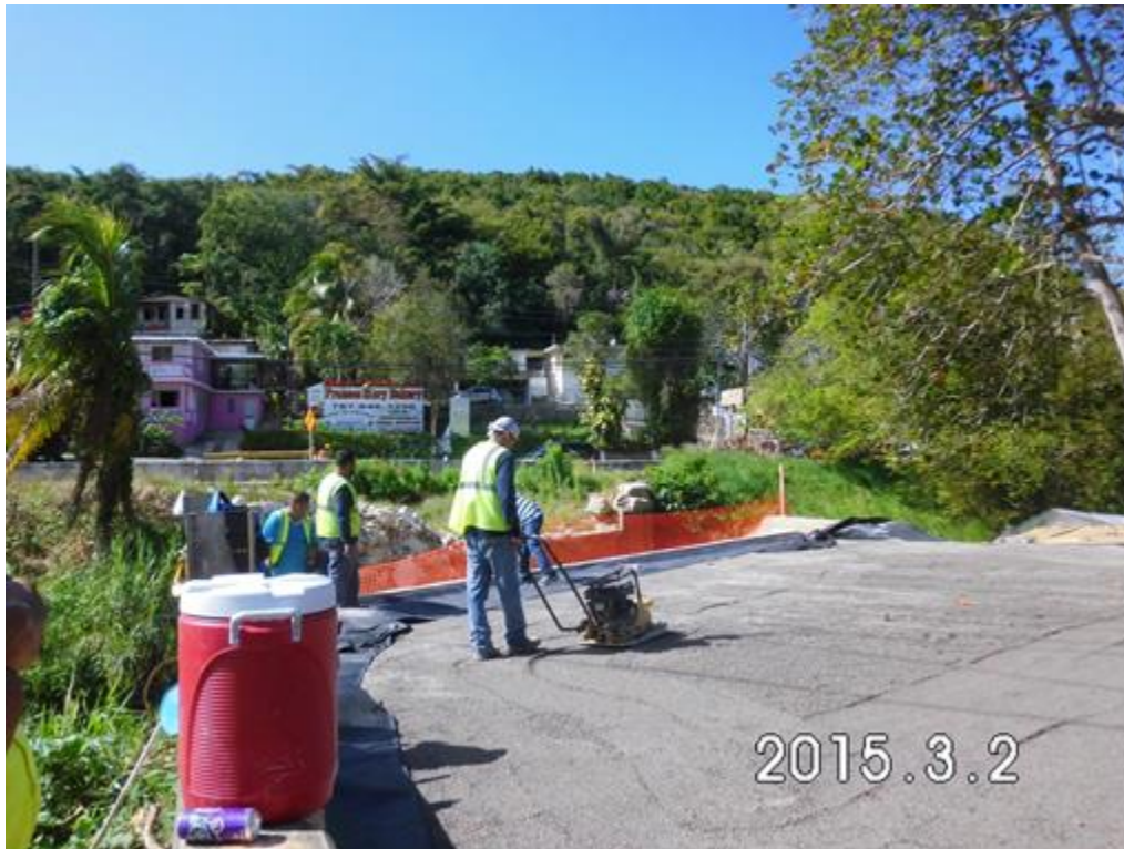
Figure 7. Photo. GRS-IBS installation on east abutment.
