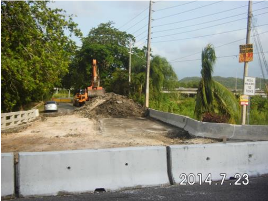
Figure 3. Photo. Existing Bridge No. 1828 on PR-140.
