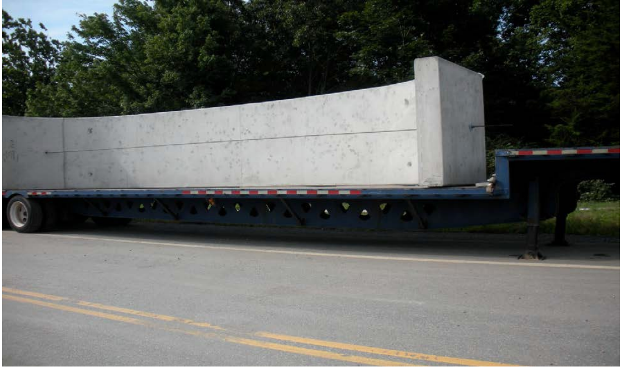
Figure 15. Main bridge element with cable tie on flatbed.
