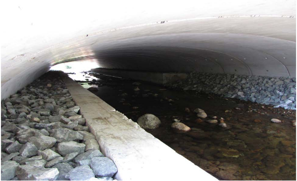
Figure 31. Bridge opening with riprap placed behind old structure abutment walls.
