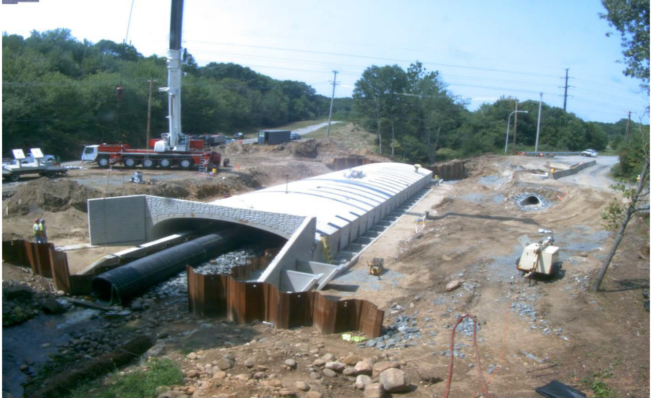
Figure 21. Another wingwall being lowered into place.
