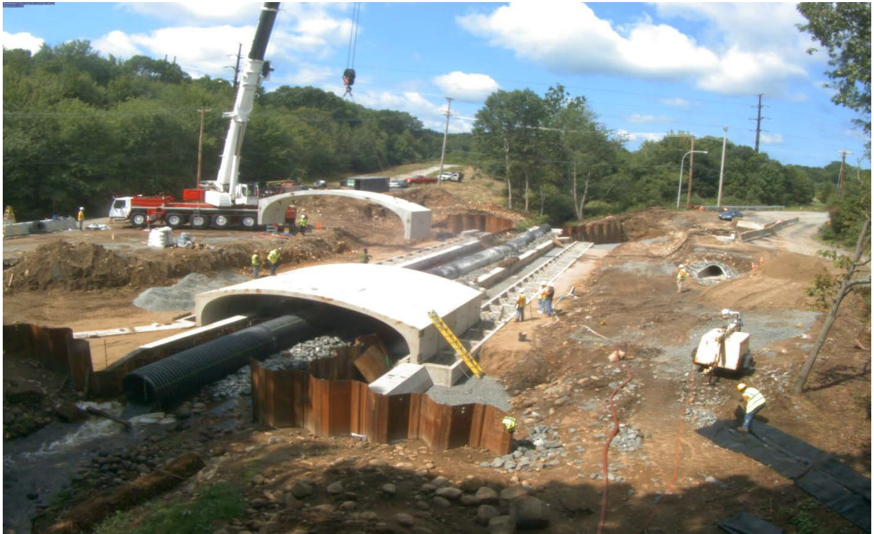
Figure 16. Modular main bridge elements lowered into place.
