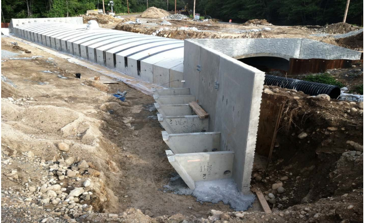
Figure 25. Prefabricated structure showing joints sealed and wrapped.
