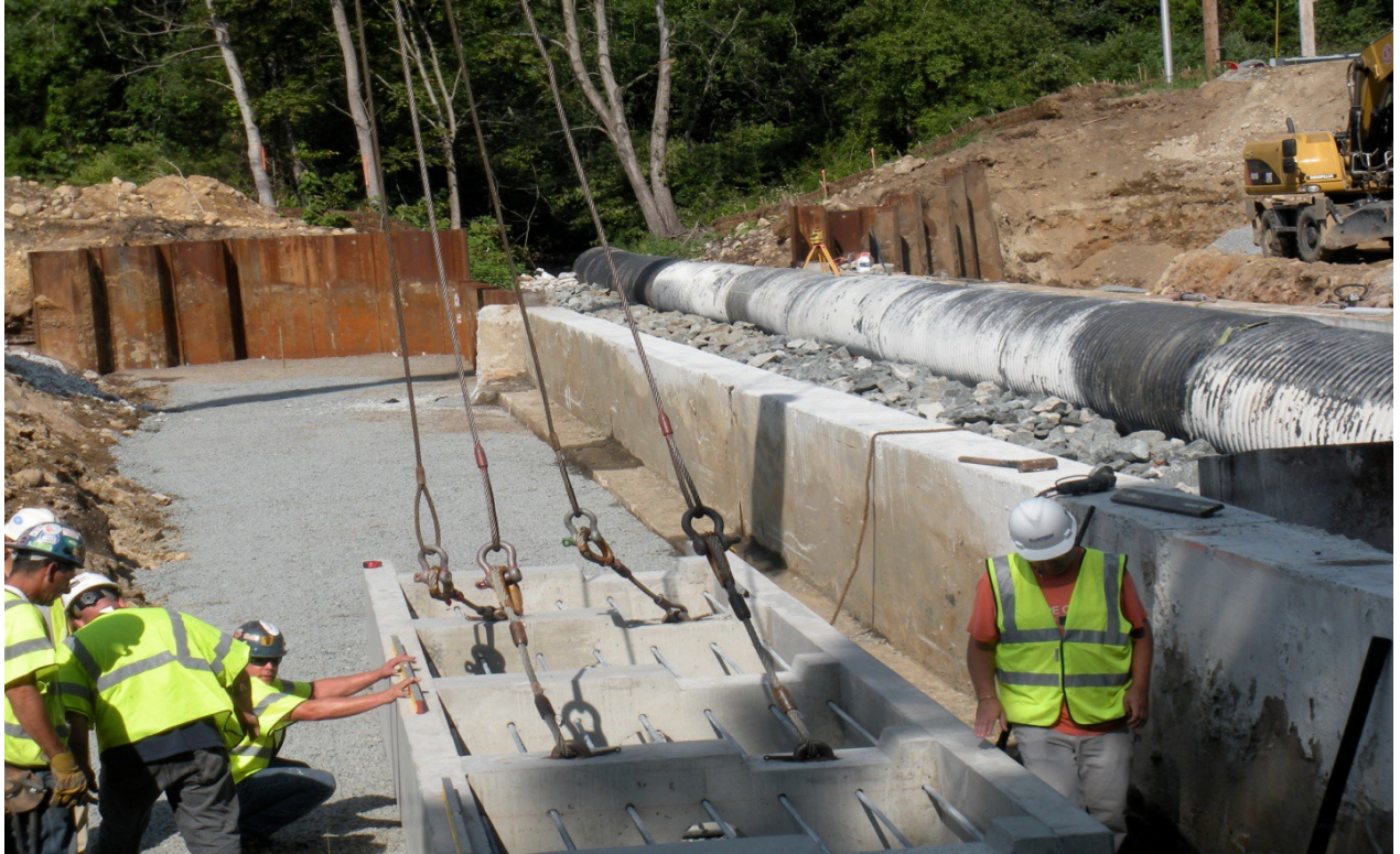
Figure 13. Precast foundation unit being placed on subfooting.
