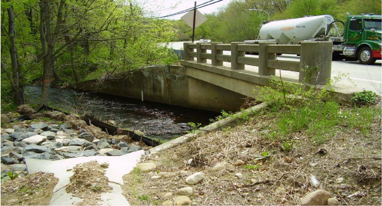
Figure 2. Old Frenchtown Brook Bridge.
