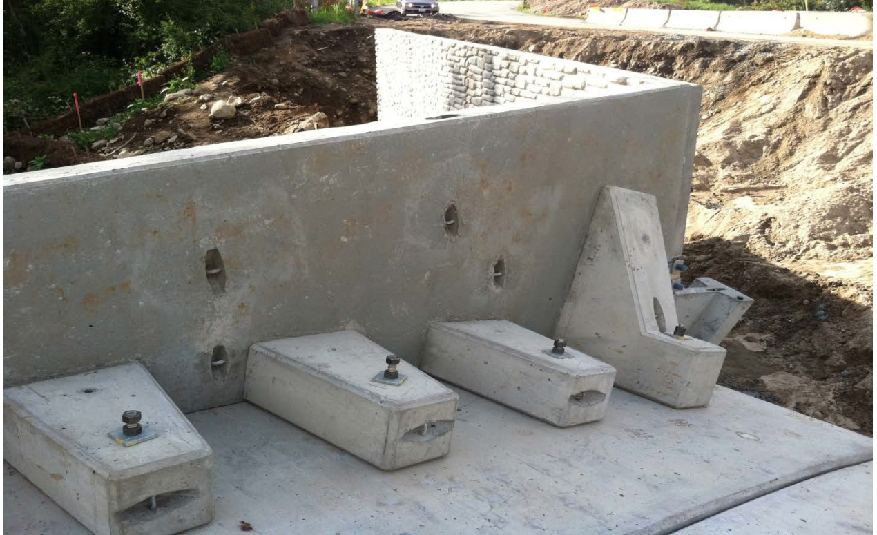
Figure 23. Closeup of headwall anchors.
