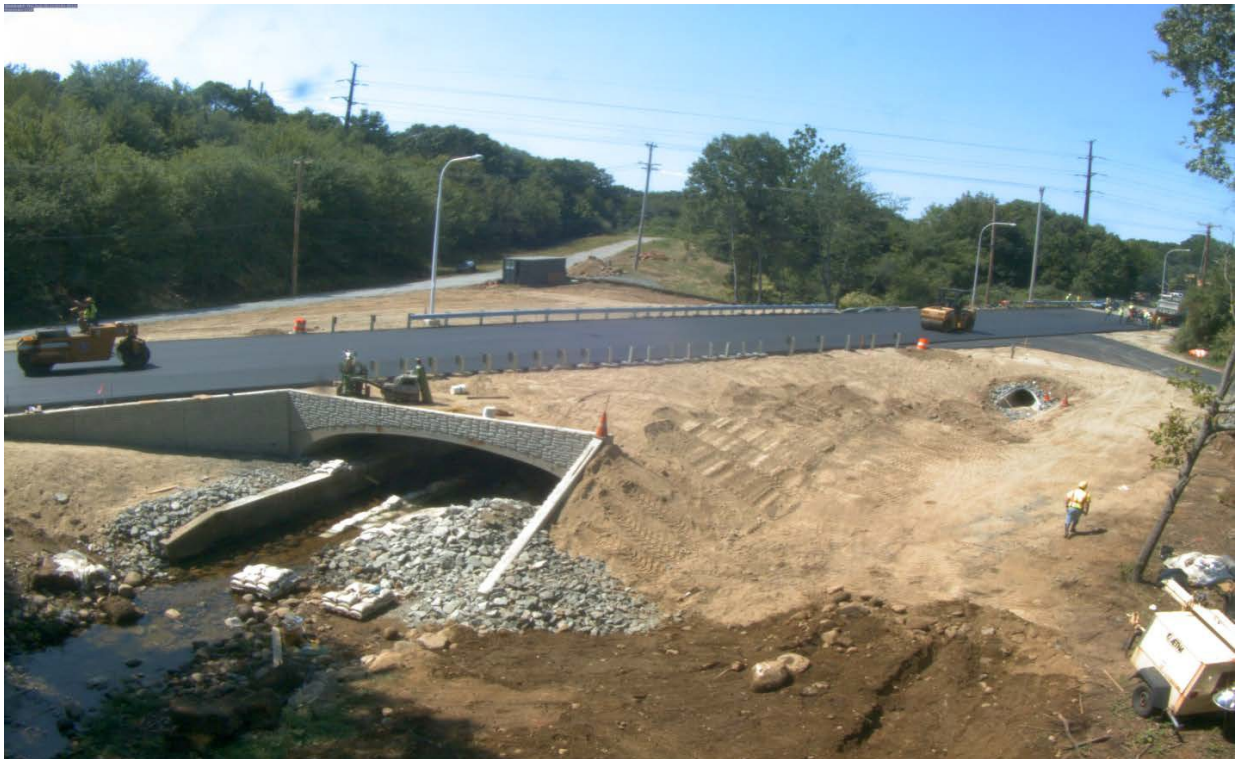
Figure 28. Bituminous material being rolled into place.
