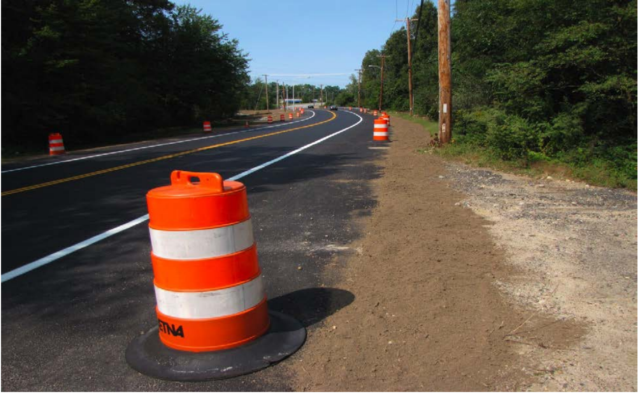
Figure 29. Davisville Road opened to traffic.
