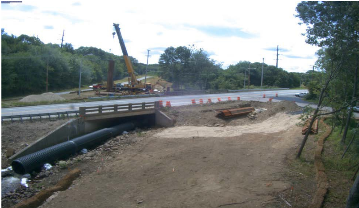
Figure 5. Bridge before closure.
