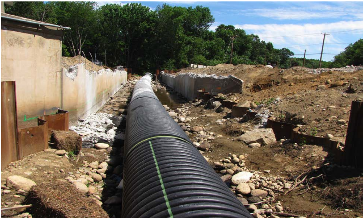
Figure 9. Abutment walls of old bridge left in place so work does not impact stream.
