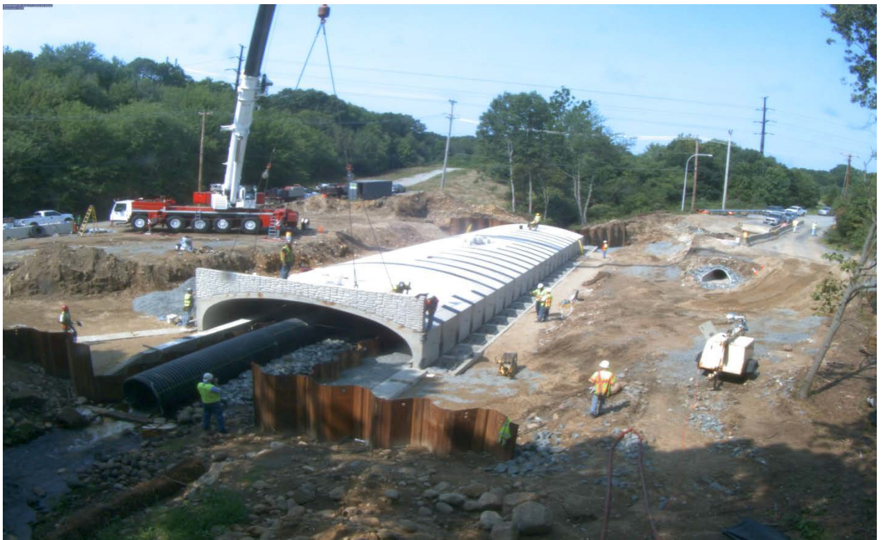
Figure 18. Modular headwall being lowered into place.
