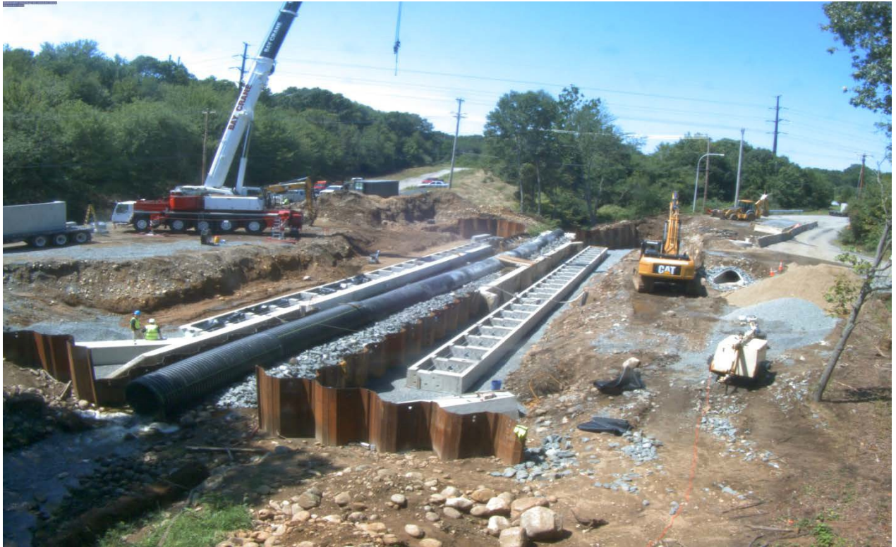
Figure 14. Modular prefabricated footings in place.
