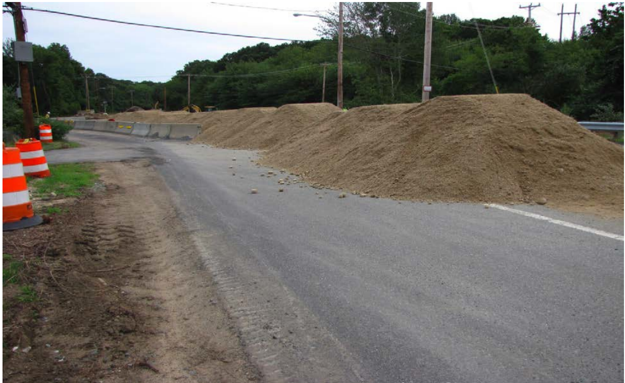
Figure 26. Stockpiled structure backfill.
