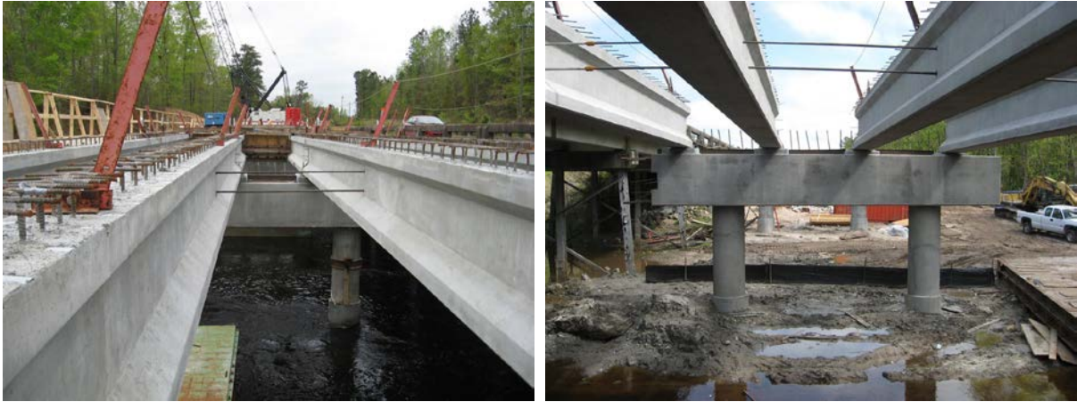
Figure 12. Construction of Black River Bridge (Phase I).
