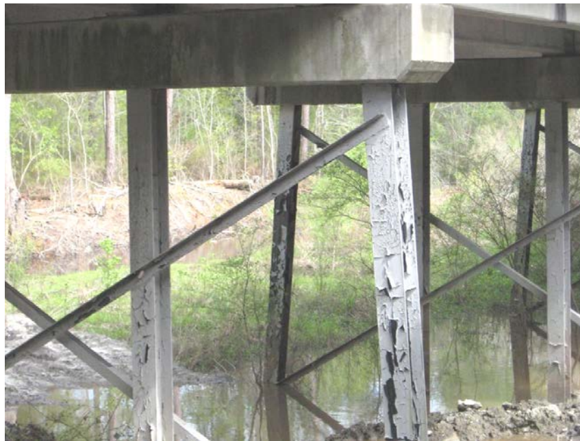
Figure 5. Black River Bridge pile detail.
