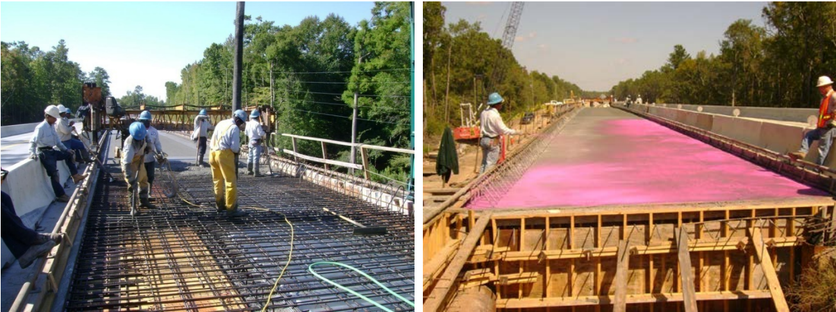
Figure 16. Phase II of construction.
