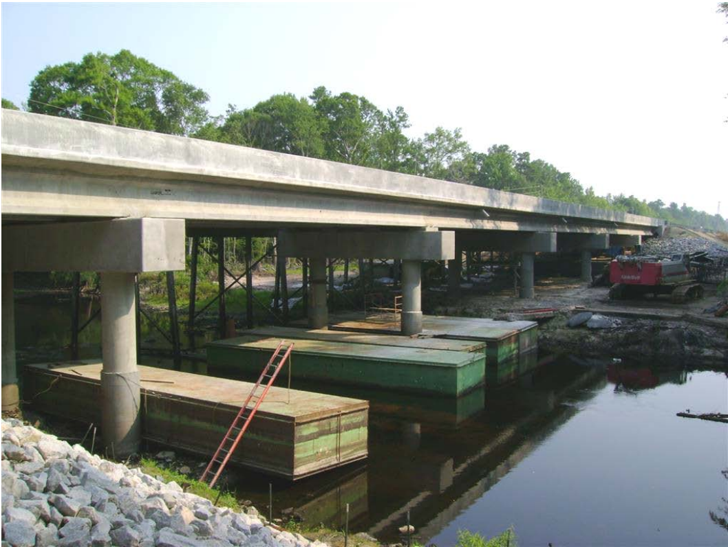
Figure 13. Black River Bridge after phase I of construction.
