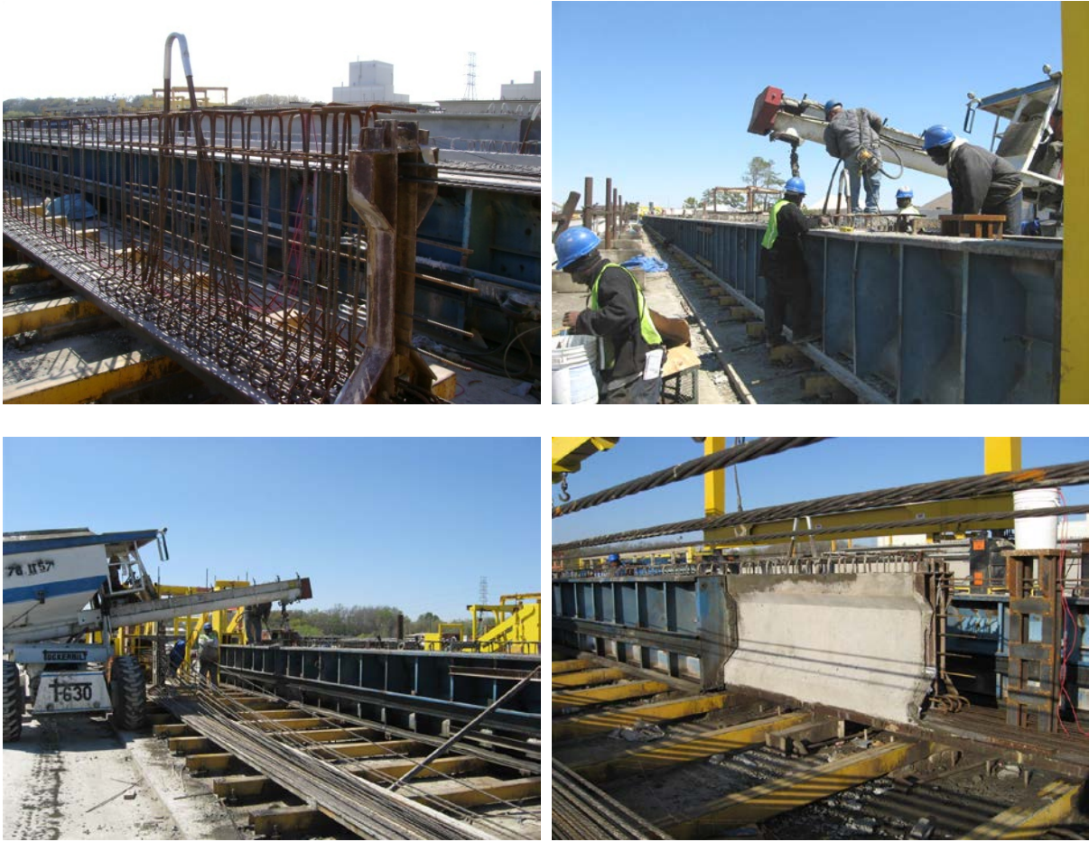
Figure 9. Fabrication of SCC beams.
