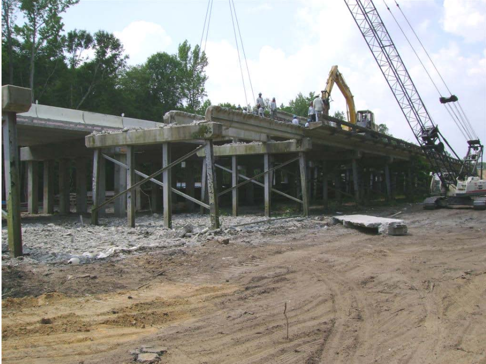
Figure 15. Demolition of the old Black River Bridge.
