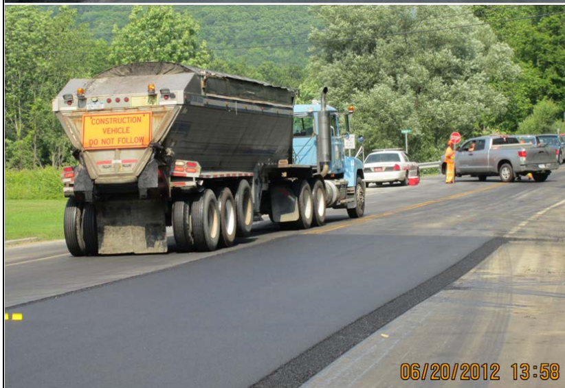
Figure 10. Trucks used to deliver the HMA and WMA mixtures to the paver.
