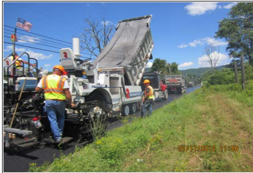
Figure 11. Paver used to place the HMA and WMA mixtures along all three roadway segments.
