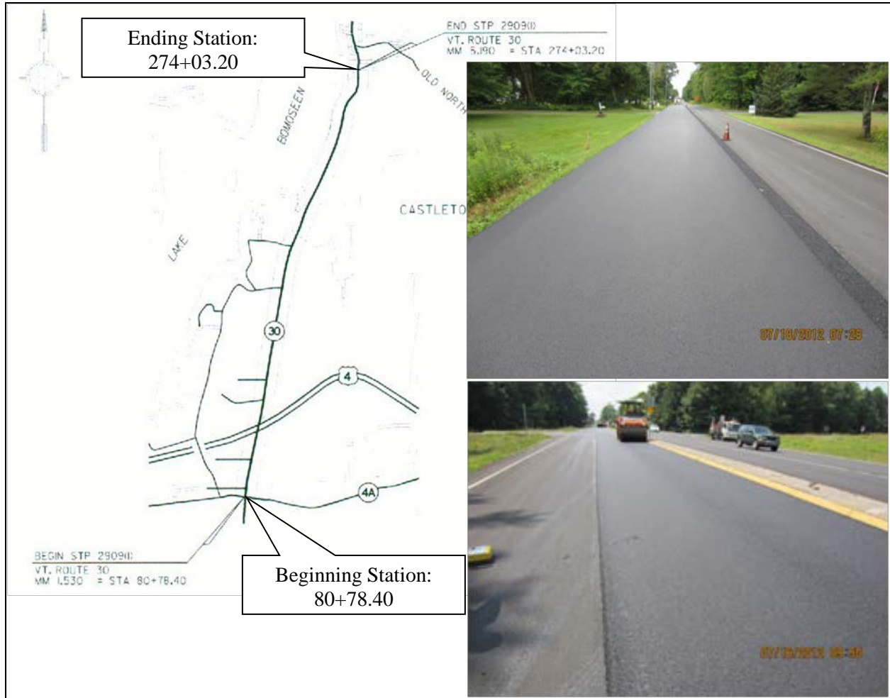
Figure 3. Project #2909—Limits and general view of VT 30 segment north of Castleton.
