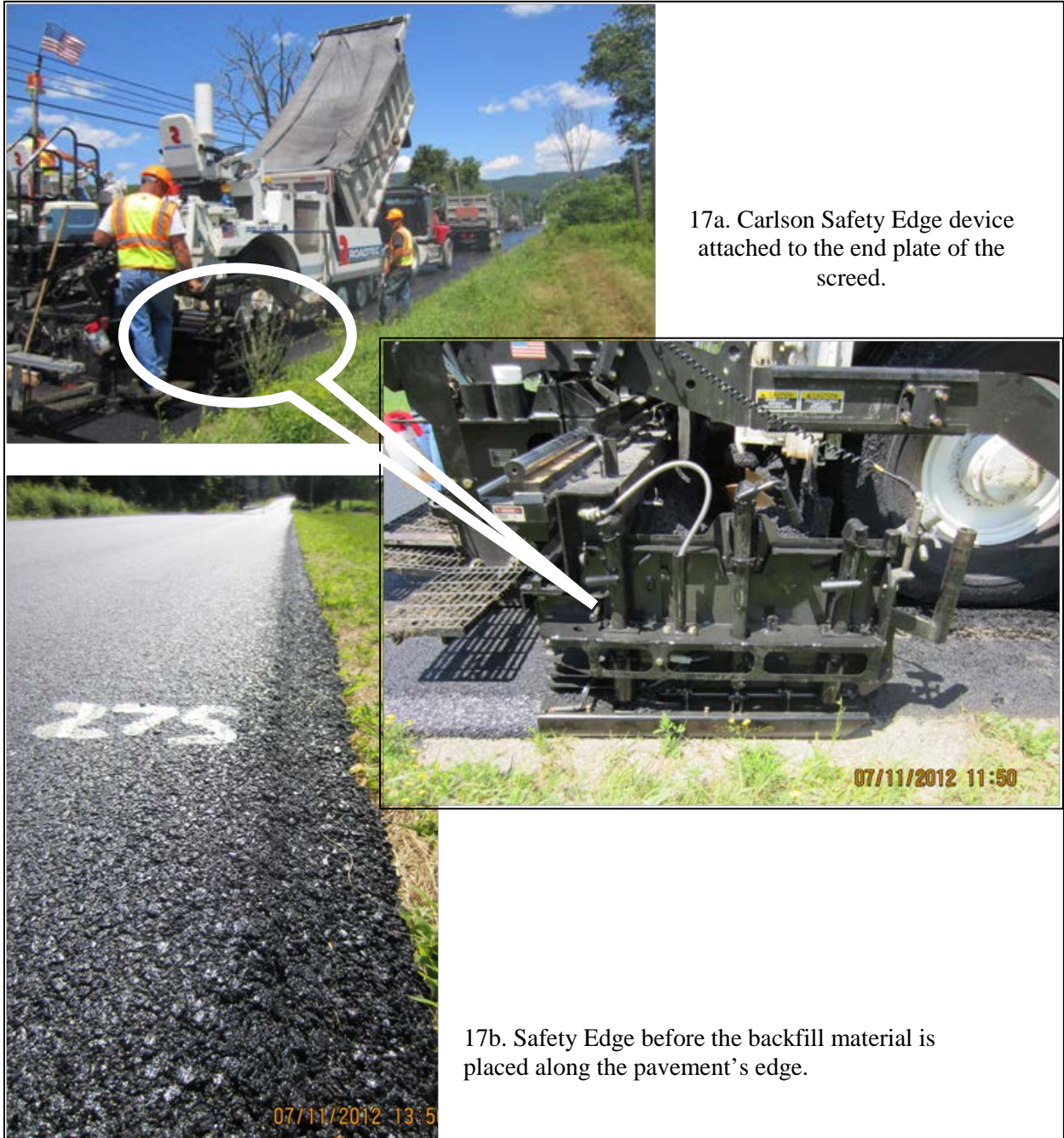
Figure 17. Safety edge placed by the Carlson device.
