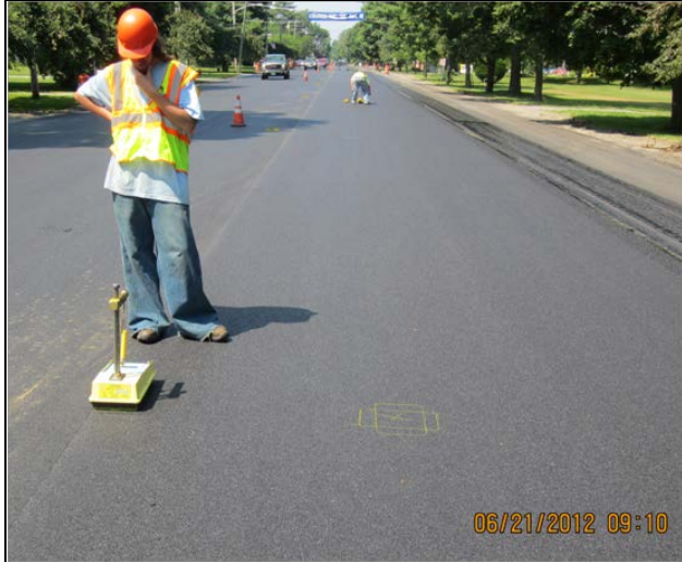
16a. Troxler nuclear density gauge used to monitor the mat density during the rolling operation.
