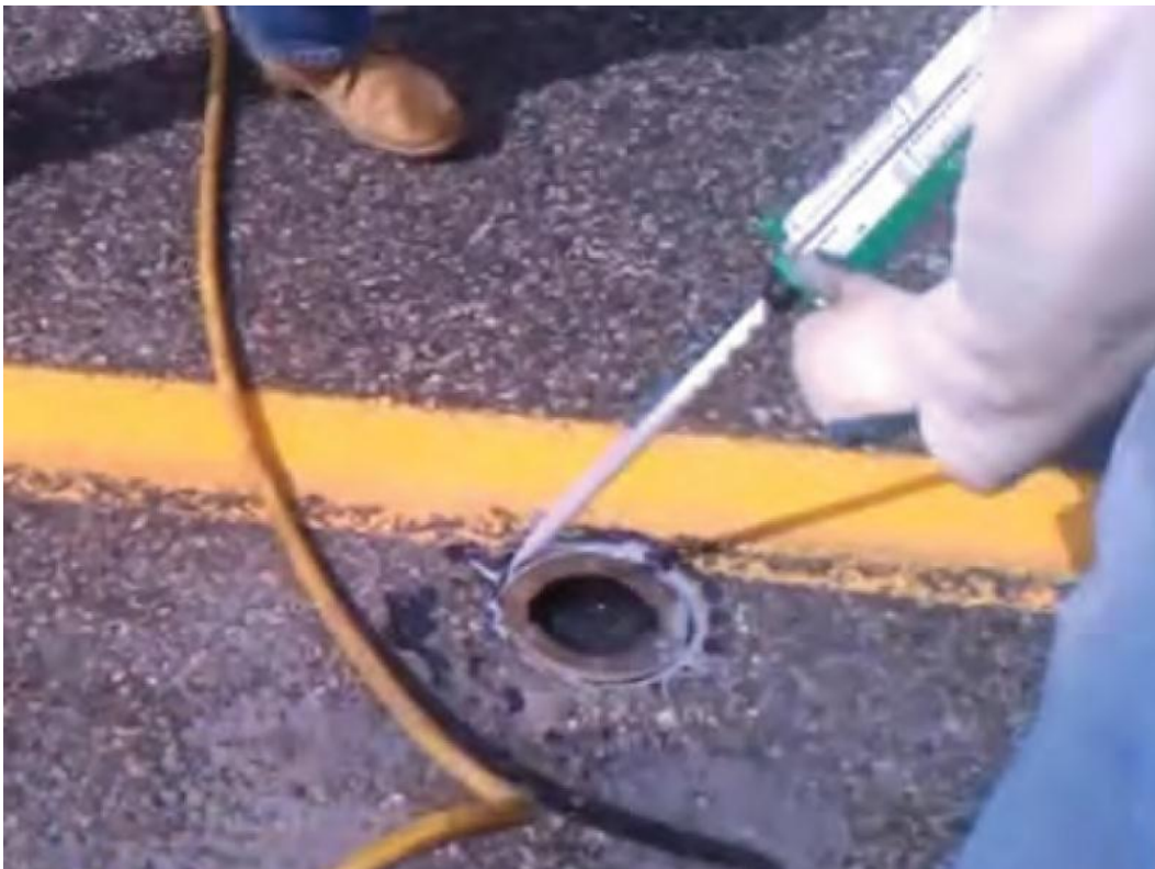
Figure 6. Photo. Application of epoxy to the perimeter of the marker base.
