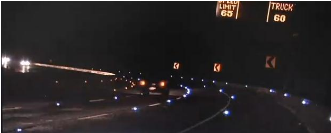
Figure 16. Photo. Nighttime view of I-90 through Snoqualmie Pass with new LED delineators.
