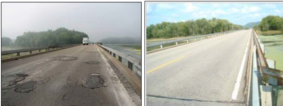
Figure 4. Existing bridge #3 (left) and existing bridge #4 (right).
