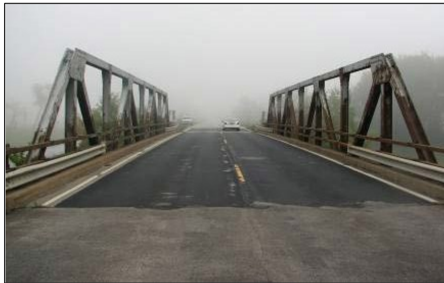
Figure 2. The pony truss bridge #1 prior to reconstruction.
