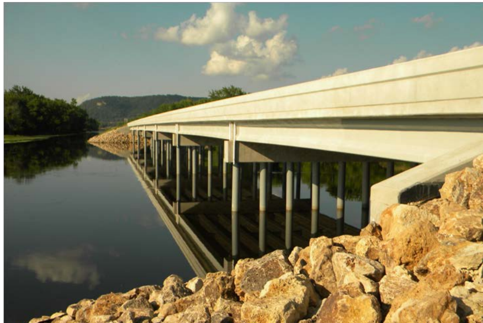
Figure 9. Finished open pile bents at bridge #3.
