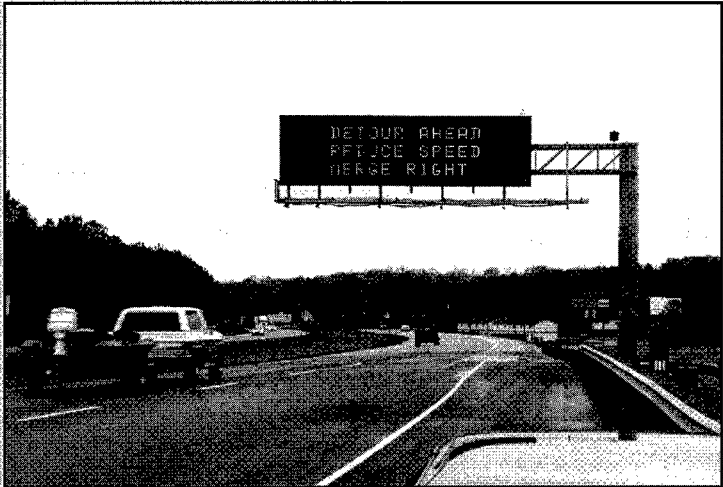
Variable Message Signs (VMSs) warn motorists at strategic locations.
