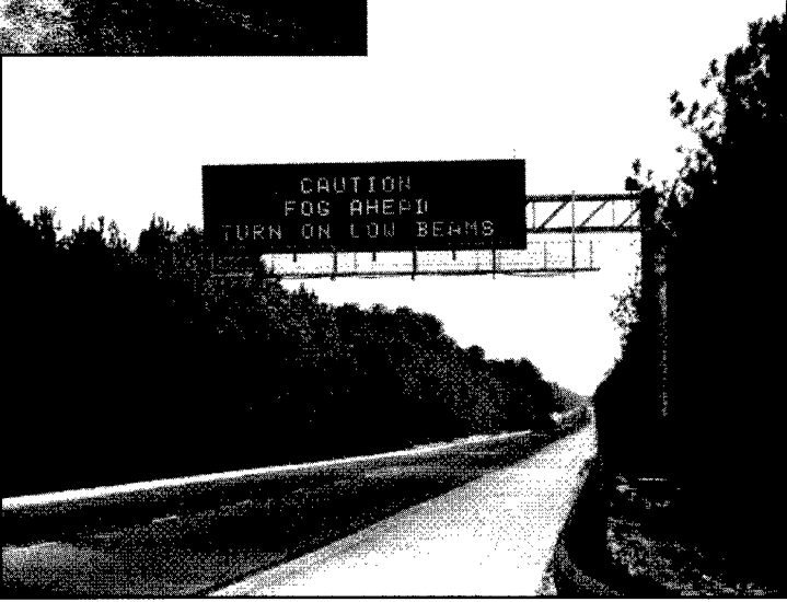
Variable Message Signs (VMSs) displays predetermined messages in accordance with the fog or speed condition scenario in effect.
