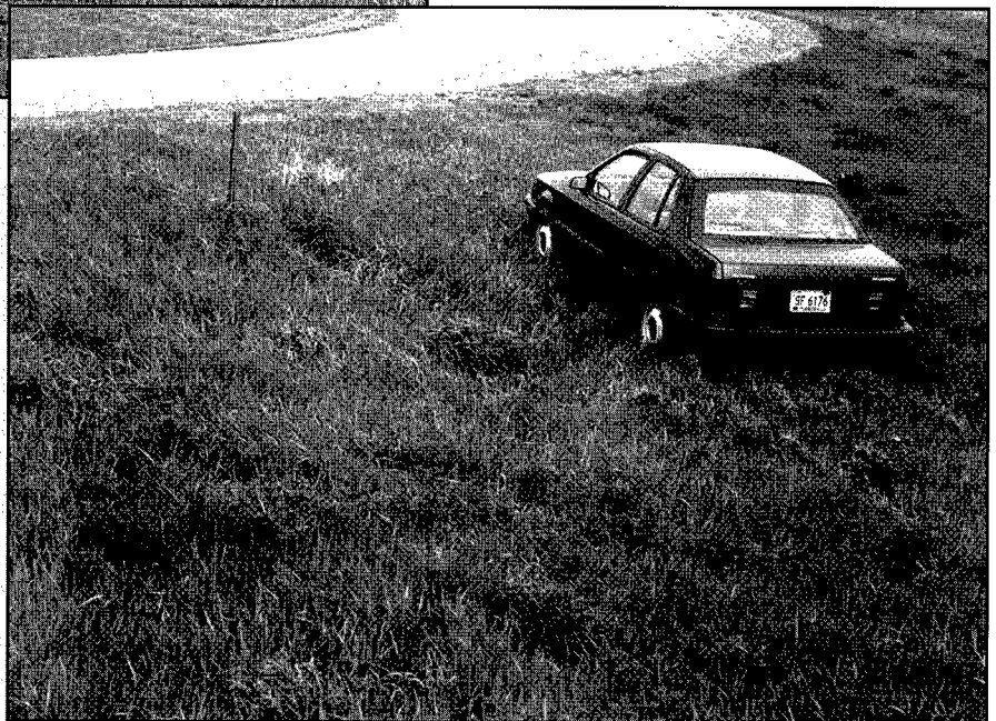
Corrected drive slope 8-to-1 grade.
