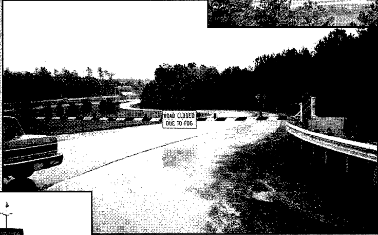
Swing gates control ramp access.
