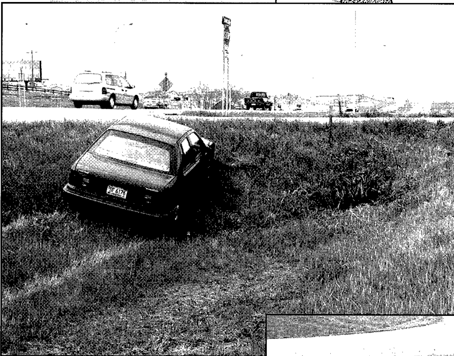
Non-corrected drive slope 4-to-1 grade.
