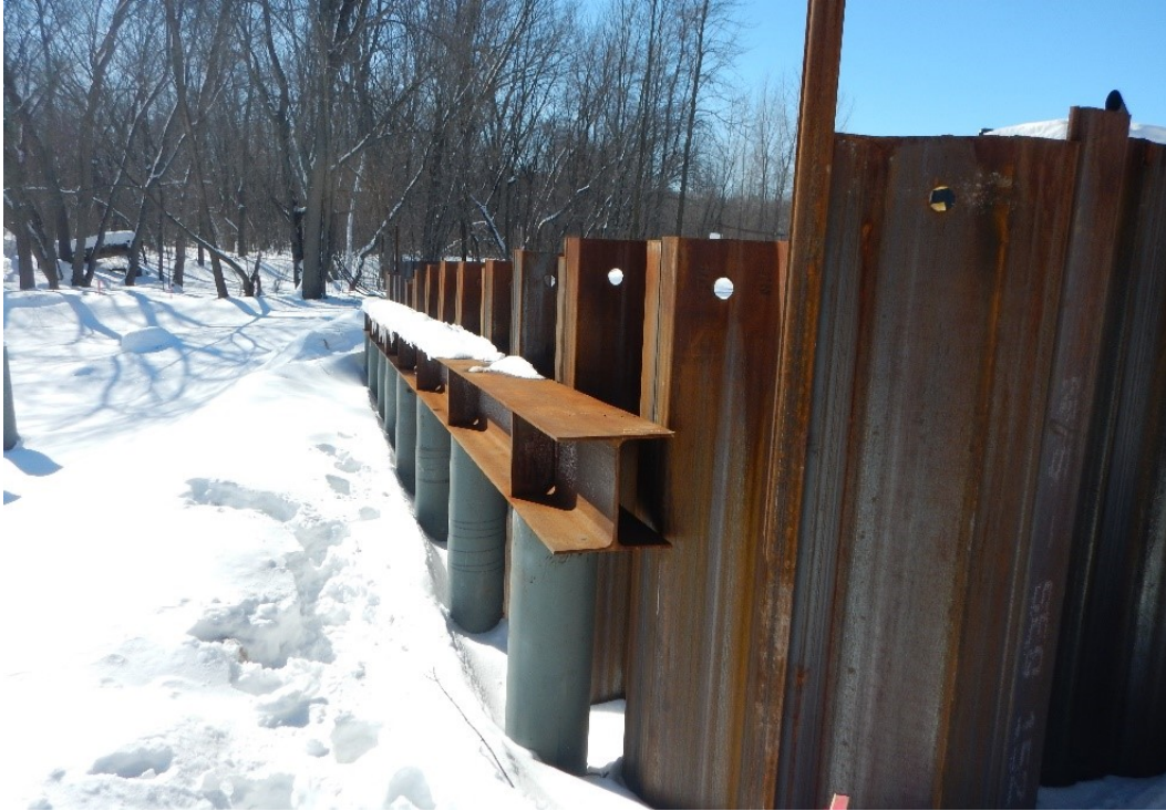
Figure 5.25 Abutment construction with CIP piling, H-beam, and steel sheeting for the abutment and wing wall. Photo credit Hennepin County.
