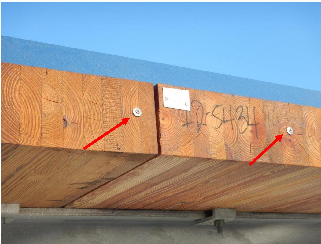
Figure 4.43 Washers attached to panel end-grain to create air space under the flashing.
