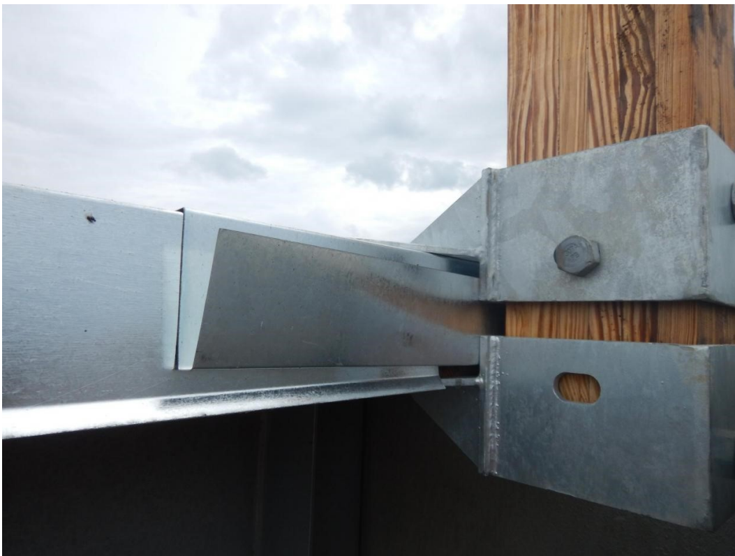
Figure 4.49 Post hardware installed over the flashing.
