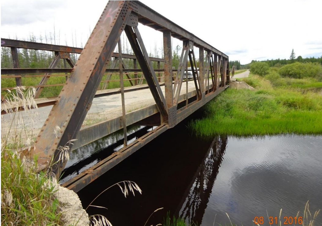
Figure 4.1 Original 1919 steel pony-truss bridge that was replaced during this project.
