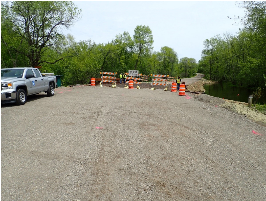
Figure 5.53 Roadway approaches and bridge deck prepared for final bituminous paving. Photo credit Hennepin County.
