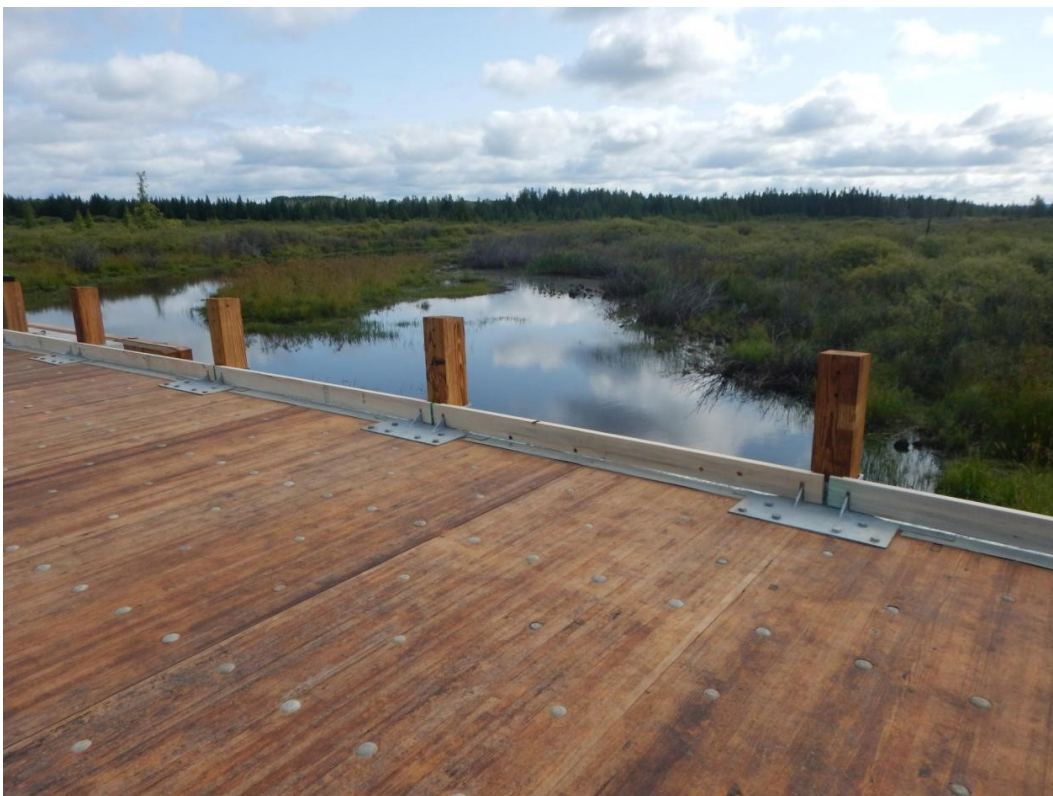
Figure 4.57 A temporary wood paving edge was developed and installed prior to overlay.
