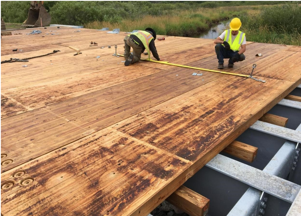
Figure 4.40 A ratchet tightening system was used to ensure tight edge-to-edge.
