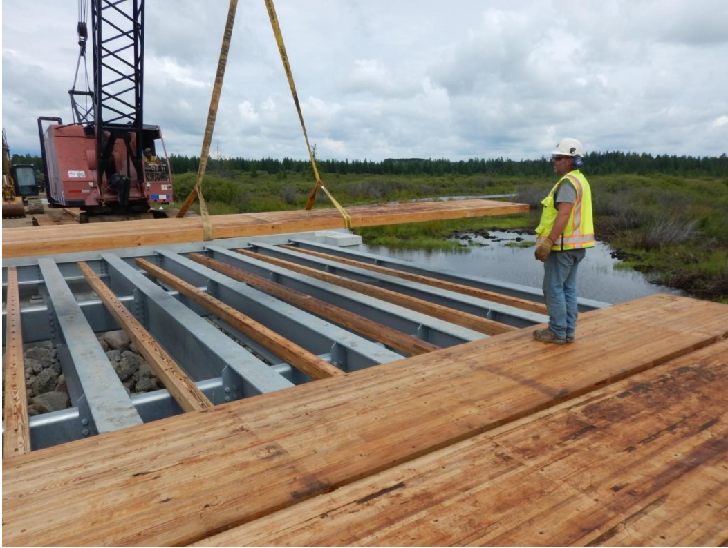
Figure 4.35 Panels were lifted using straps.
