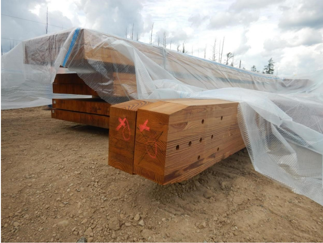
Figure 4.25 Wood materials were covered with a plastic tarp to protect from rain.
