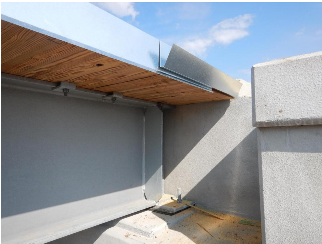
Figure 4.47 Short flashing sections were installed at the bridge corners.
