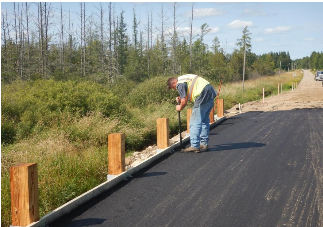
Figure 4.65 Hand tamping of bituminous along paving edge.
