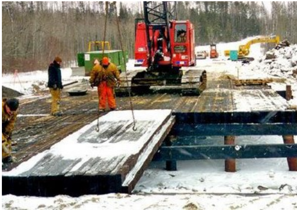
Figure 3.1 Winter construction of a longitudinal spike-laminated timber deck.
