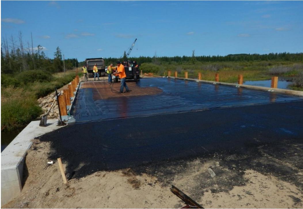
Figure 4.62 A tack coat was applied to the timber deck surface and the bituminous wedge.
