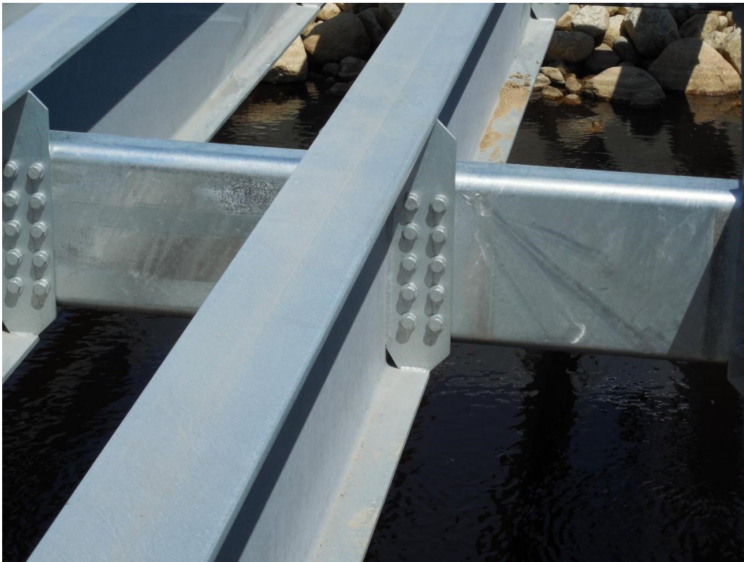
Figure 4.21 Steel diaphragm installation.
