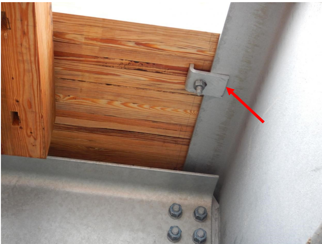
Figure 4.32 Close-up of galvanized clip connection between panel and steel beam.
