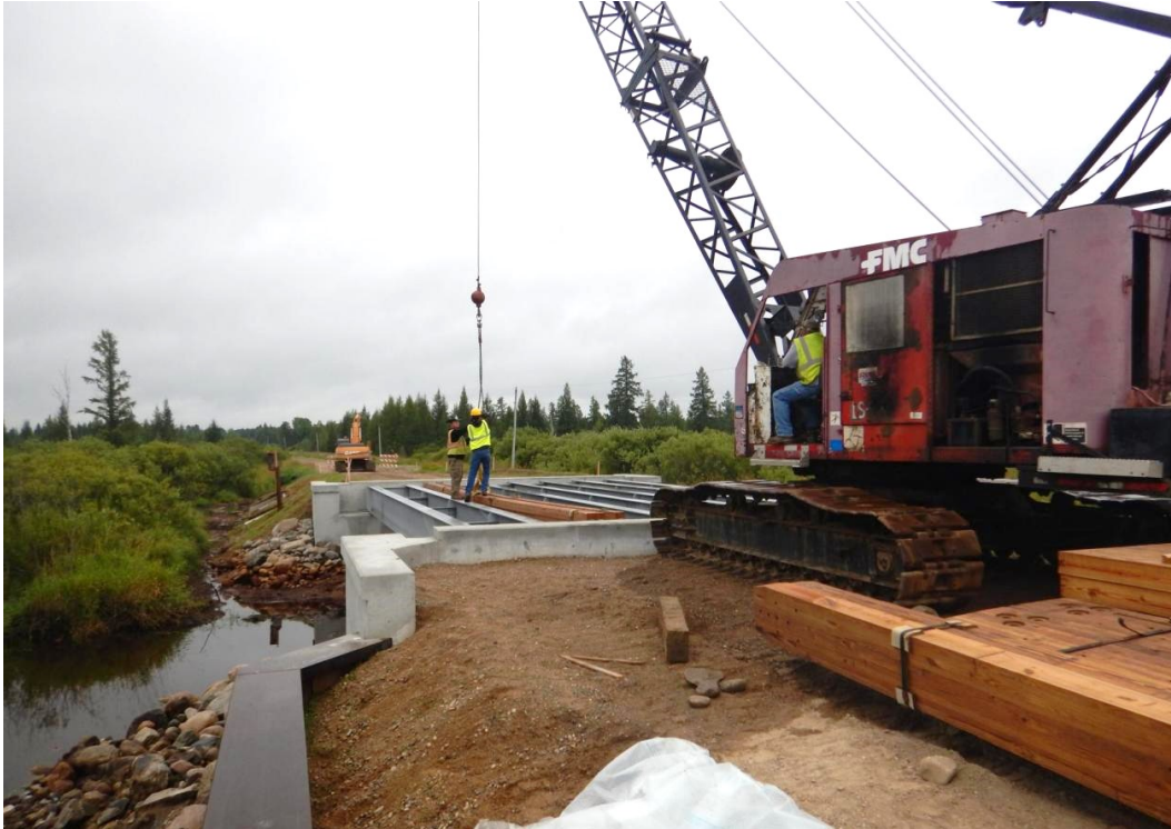
Figure 4.26 Stiffeners were moved to the bridge deck using a crane.
