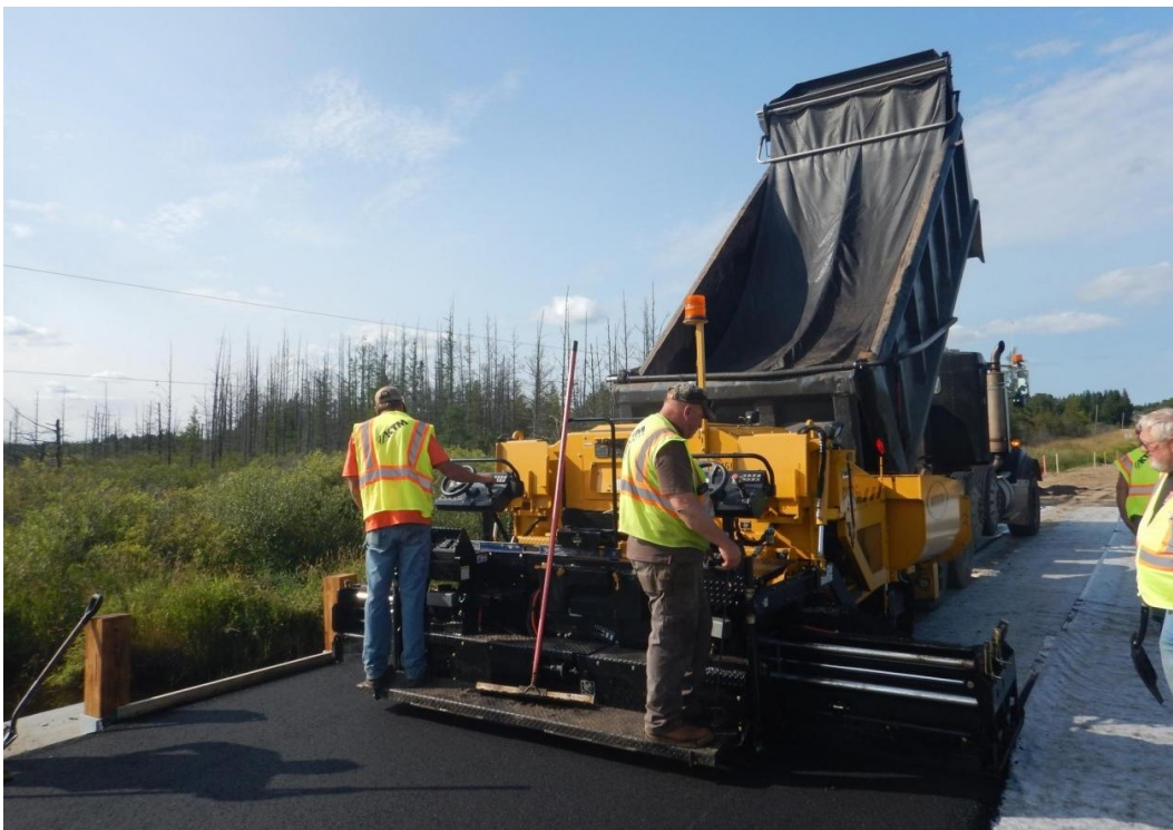
Figure 4.69 A second layer of bituminous overlay was added on top of the membrane.
