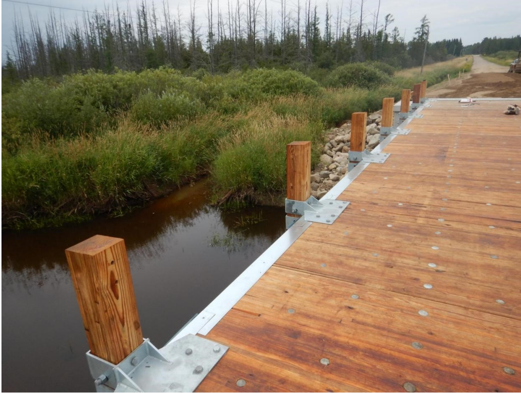
Figure 4.50 Fully installed flashing and rail posts.
