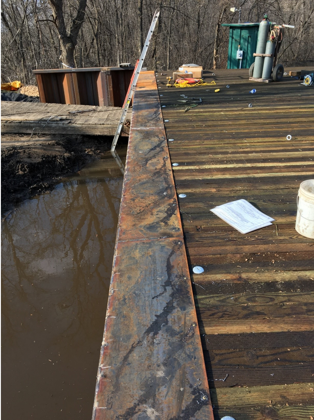
Figure 5.38 Steel plate installed over the end of the abutment cap and the end of the timber panels covering the end gap (Figure 5.32). Photo credit Hennepin County.
