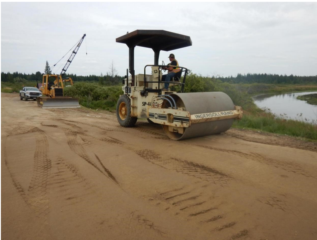
Figure 4.55 Vibratory compaction of the approach prior to bituminous installation.
