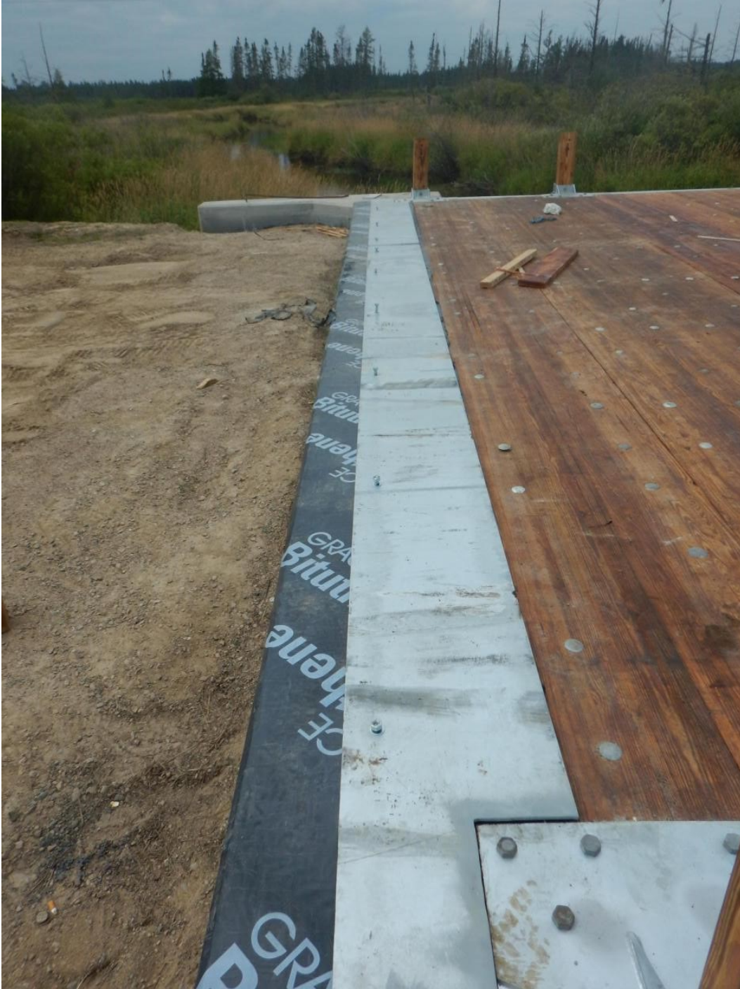
Figure 4.51 Waterproofing membrane and steel cover plate.
