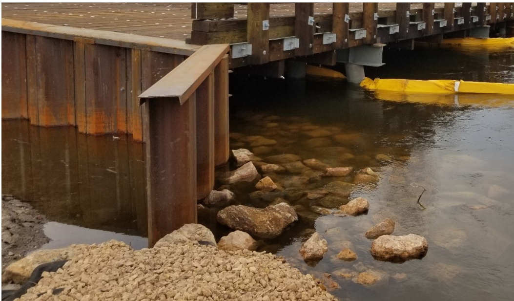
Figure 5.28 Completed west abutment showing sheet pile, end wing wall and steel channel cap. Photo credit Hennepin County.
