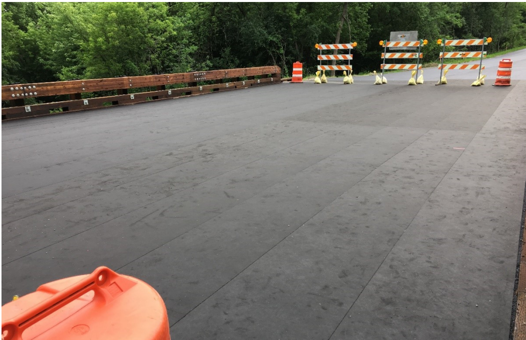
Figure 5.57 Waterproof membrane installed on top of the (base course) bituminous layer in multiple rows. Each row of waterproof membrane was overlapped by 4 inches according to the manufacturers' specifications. Photo credit Hennepin County.
