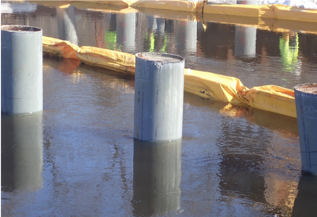
Figure 5.26 CIP piling that has been driven and filled. Photo credit Hennepin County.
