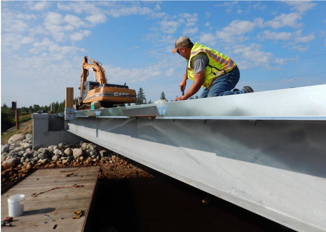
Figure 4.46 Installed flashing to protect timber deck edge.
