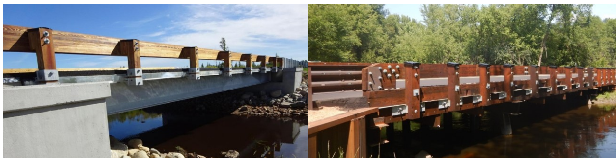
Modern Minnesota Timber Bridges. The left bridge photo is a galvanized steel girder with transverse glued-laminated timber deck panels built by St. Louis County. The right bridge photo is a longitudinal dowel-laminated timber deck with metal spikes panelized bridge built by Hennepin County.
