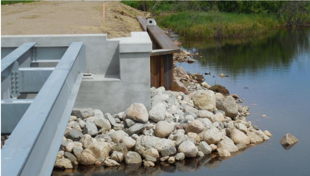
Figure 4.16 Concrete abutment, sheet pile wing wall and riprap to protect the roadway and bridge.
