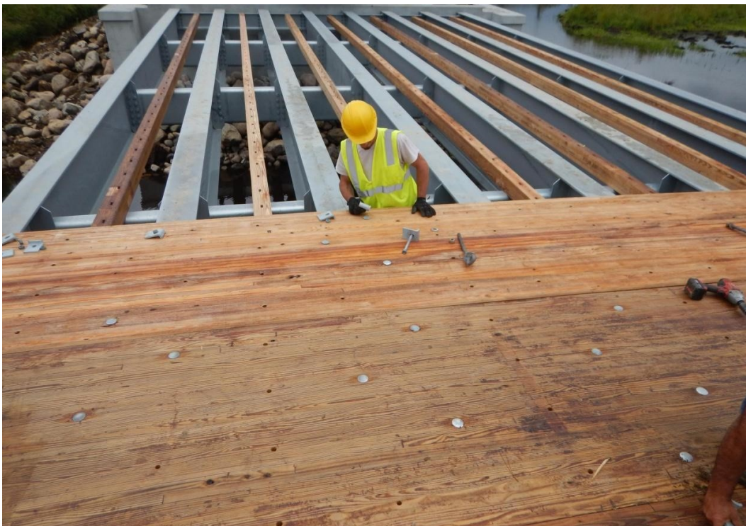
Figure 4.34 Stiffener bolts were also installed during placement of the panels.
