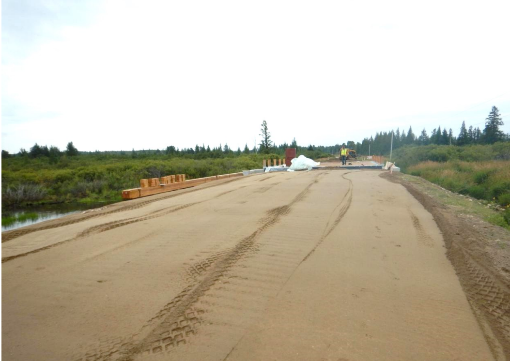
Figure 4.56 Prepared approach prior to paving.
