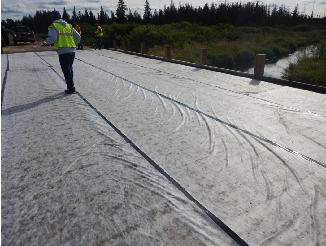
Figure 4.68 Multiple rows of waterproof membrane installed on top of the bituminous layer.
