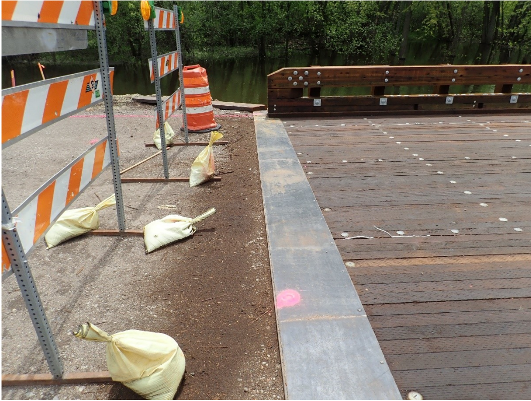
Figure 5.39 Steel plate at bridge transition after backfill and railings. Photo credit Hennepin County.
