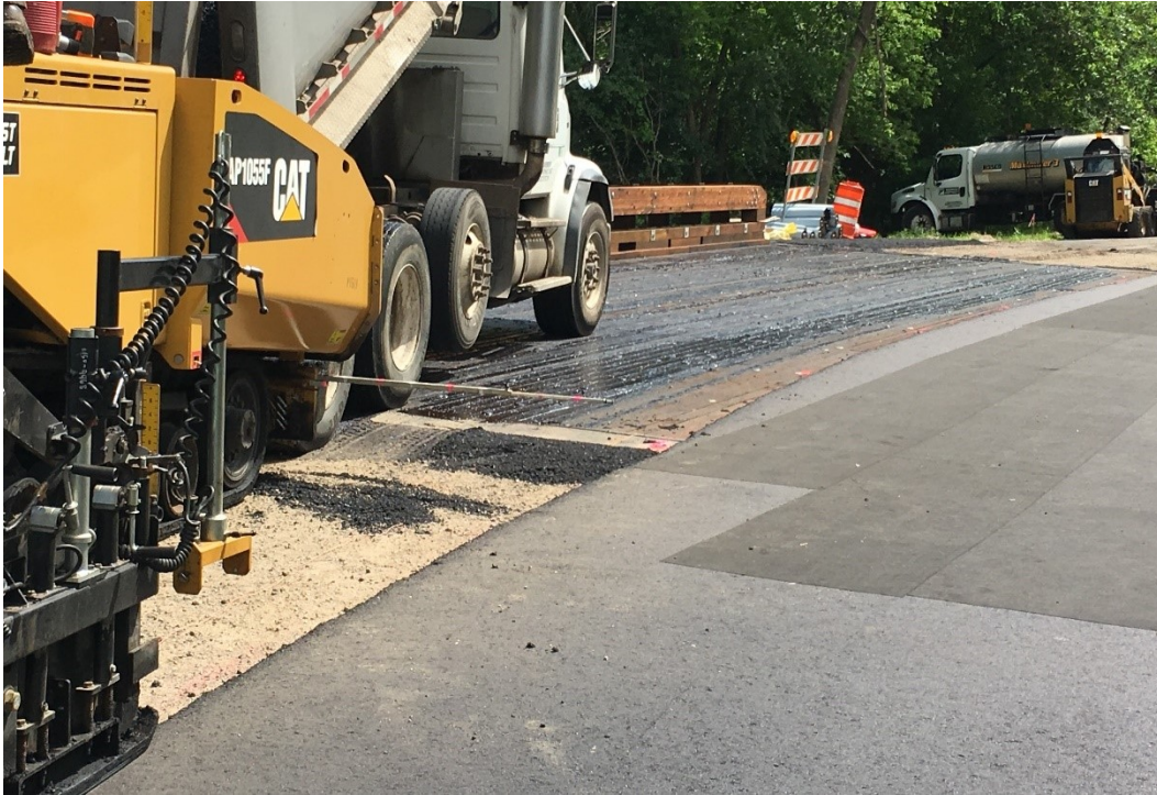
Figure 5.56 Tack coat application prior to first layer of bituminous. Photo credit Hennepin County.
