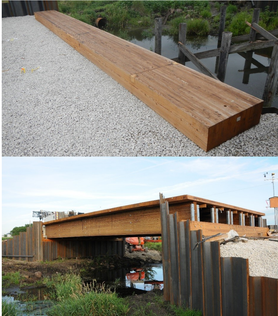
Figure 3.4 GRS abutment construction and bridge deck installation in Buchanan County, Iowa.
