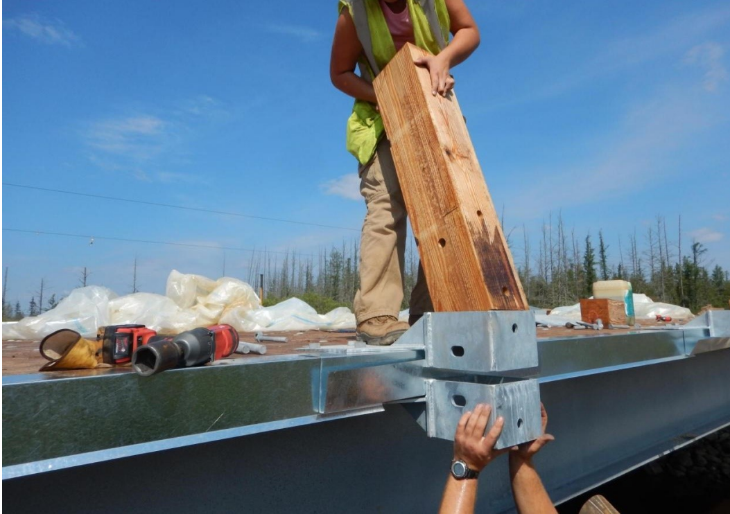
Figure 4.48 Post hardware plates were installed prior to post installation.
