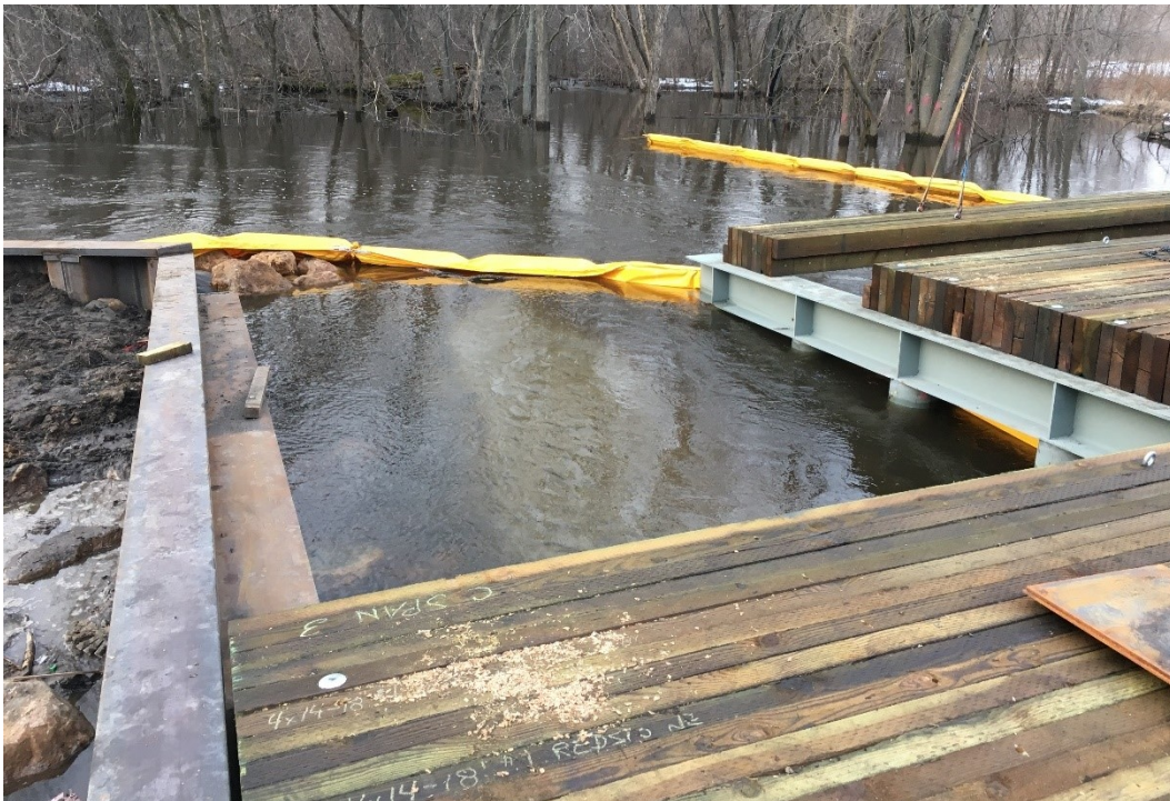
Figure 5.37 Extreme high stream level during deck installation. Design details ensured strong connections between the CIP, pier caps, and timber panels. Photo credit Hennepin County.
