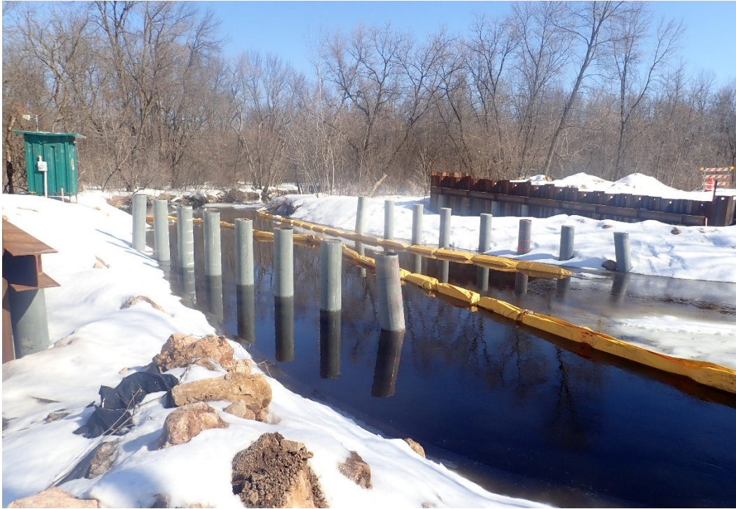
Figure 5.23 Sheet metal abutment, CIP piling and pier supports after installation.
