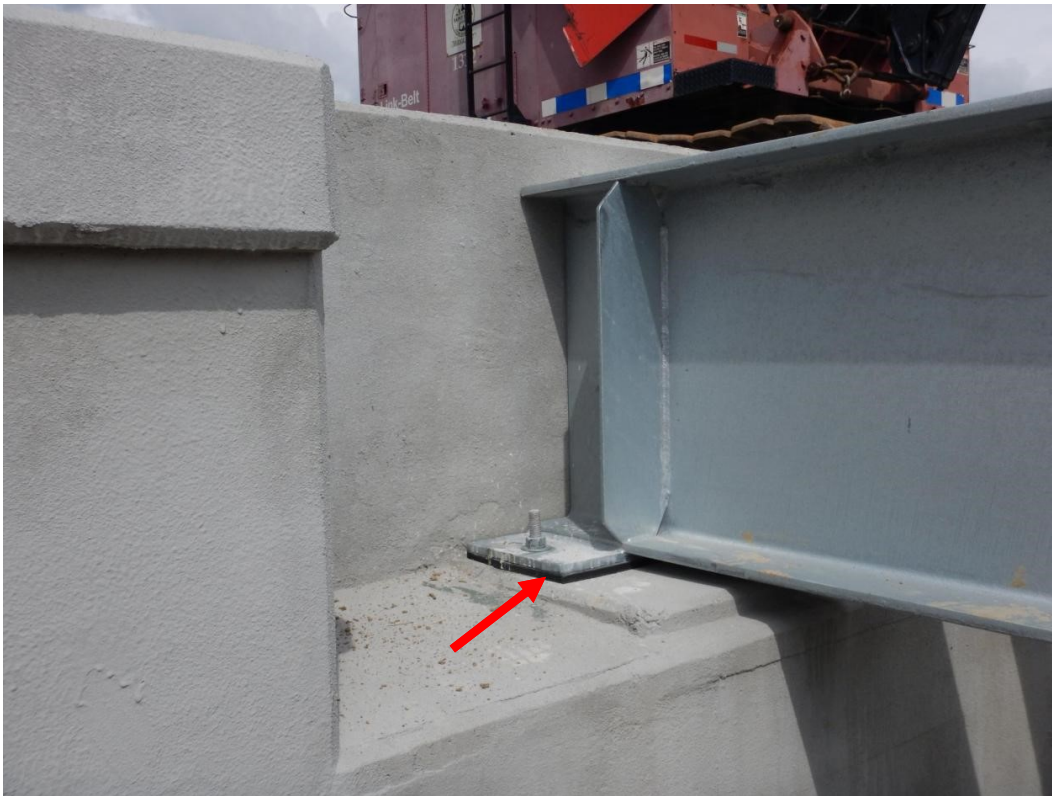
Figure 4.19 Steel beams installed onto steel bearing plates with neoprene pads.
