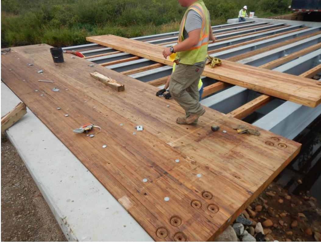
Figure 4.33 Additional panels were placed and connected to the steel beams.
