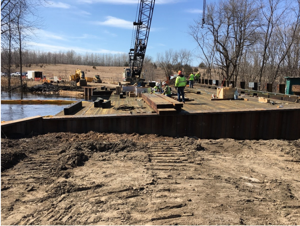
Figure 5.40 North edge of railing being installed prior to deck completion. Photo credit Hennepin County.
