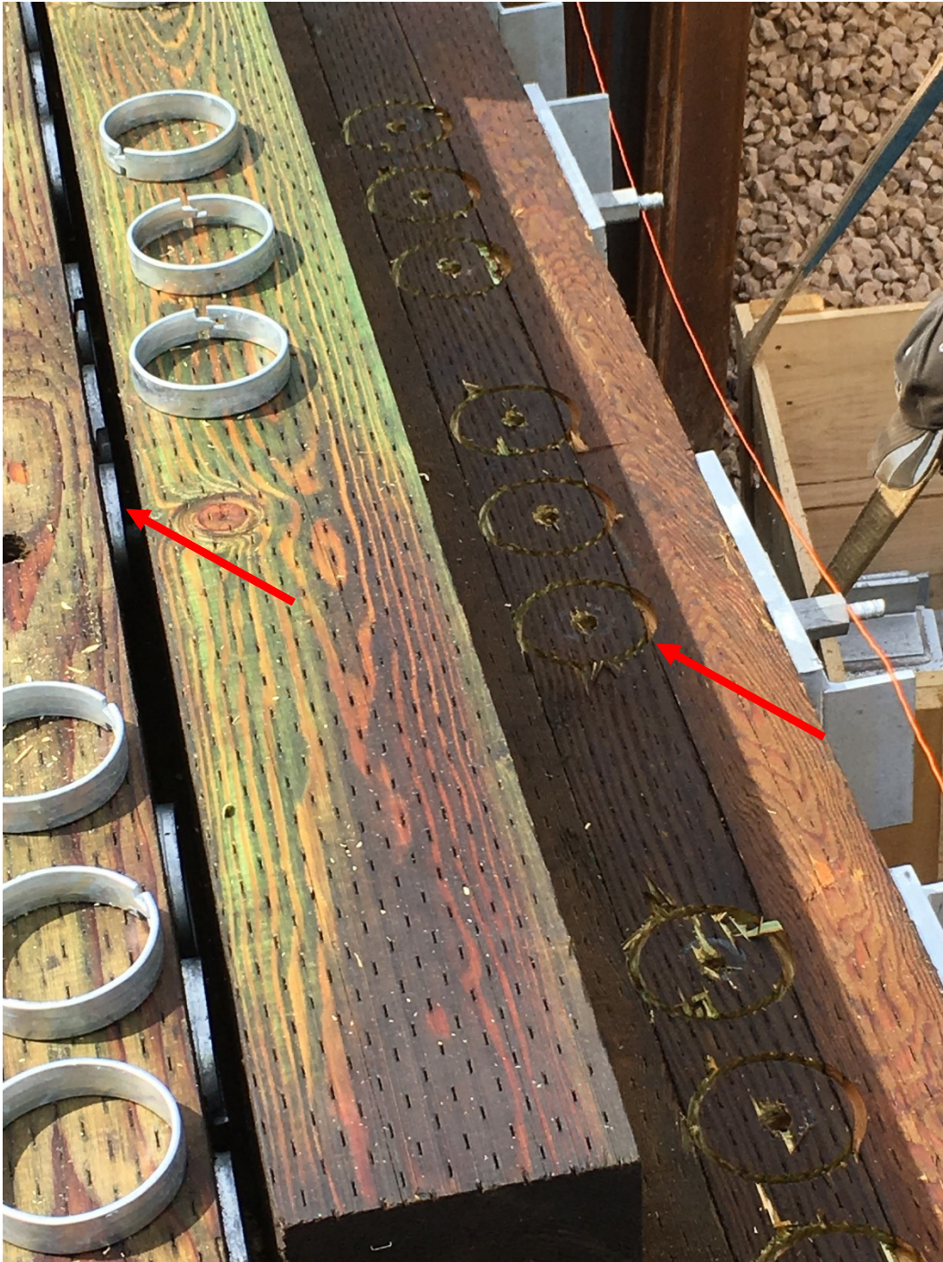
Figure 5.43 Predrilling and inserting split ring connectors at the interface of the timber deck and between the scupper blocks. Photo credit Hennepin County.
