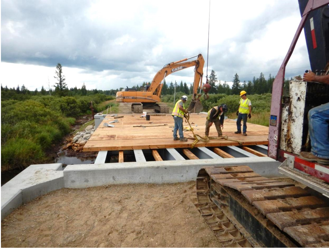
Figure 4.41 Ongoing panel placement during day 1 of panel installation.
