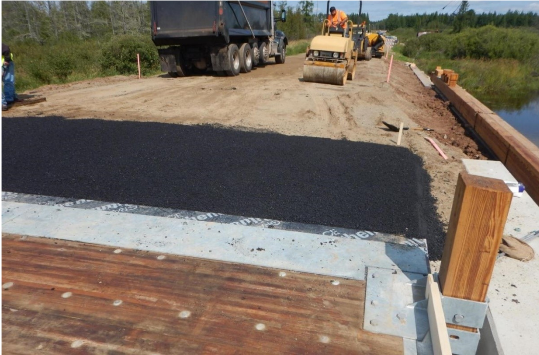
Figure 4.60 Multiple layers of bituminous were placed and compacted to create a wedge before the bridge.
