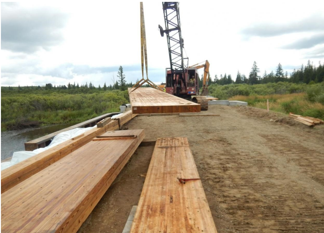
Figure 4.38 Ongoing installation of transverse deck panels
