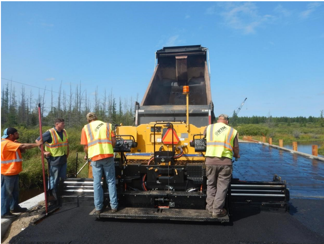
Figure 4.63 First layer of bituminous overlay being deposited onto timber deck.
