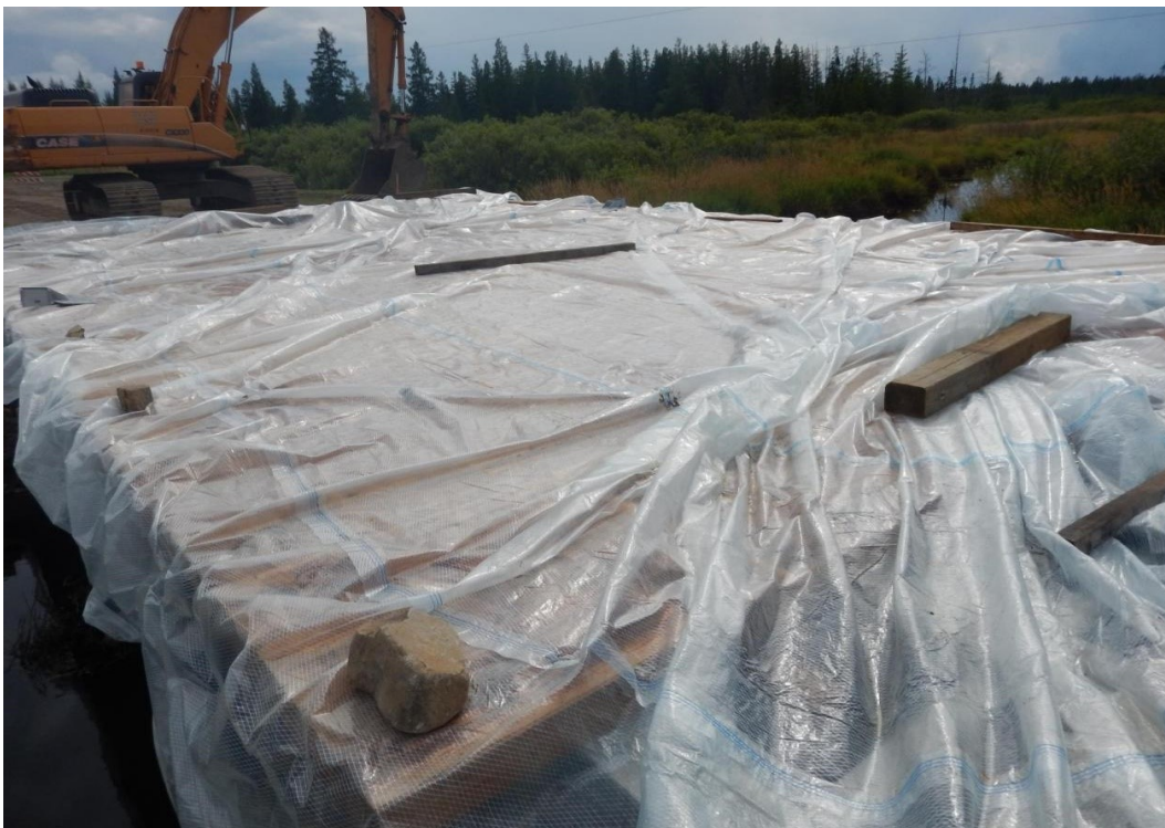
Figure 4.42 A tarp was placed onto the bridge deck to keep panels dry during construction.
