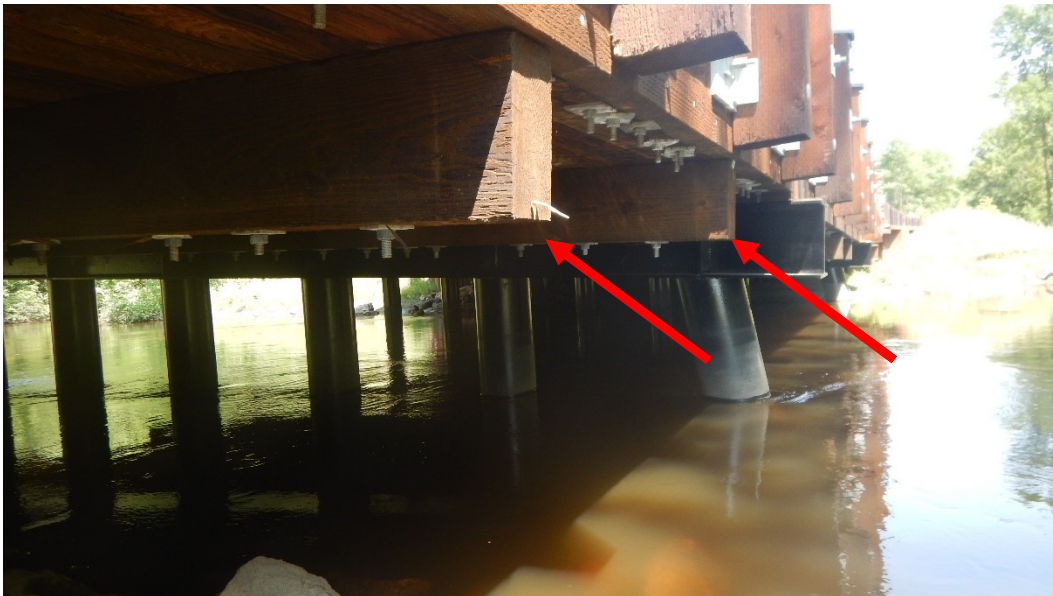
Figure 5.65 Underside view of completed superstructure showing the timber spreader beams (red arrows) at the underside of the timber deck panels.
