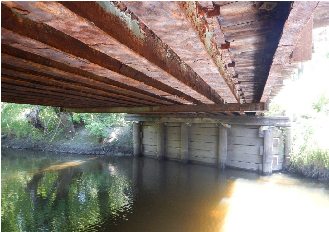
Figure 5.4 Deteriorated steel girders in underside view of the superstructure for Hennepin County Bridge L8081.
