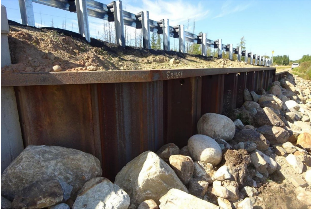
Figure 4.17 Upstream wing wall (driven sheet pile) with riprap to protect the roadway and bridge from scour erosion damages.
