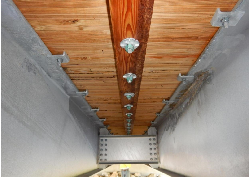
Figure 4.37 Bottom side connections.
