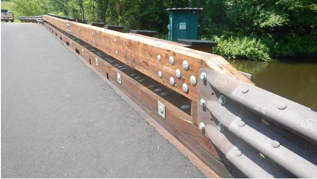
Figure 5.58 Completed installation of the crash-tested bridge railing and curb system.
