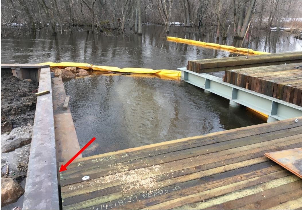
Figure 5.34 Span 3 showing designed gap (identified with red arrow) between panel end and abutment wall. Photo credit Hennepin County.
