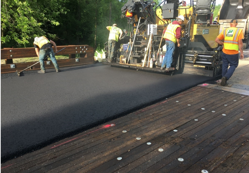
Figure 5.54 First layer (base course) of bituminous overlay being deposited onto timber deck that had a tack coat applied (not shown). Photo credit Hennepin County.
