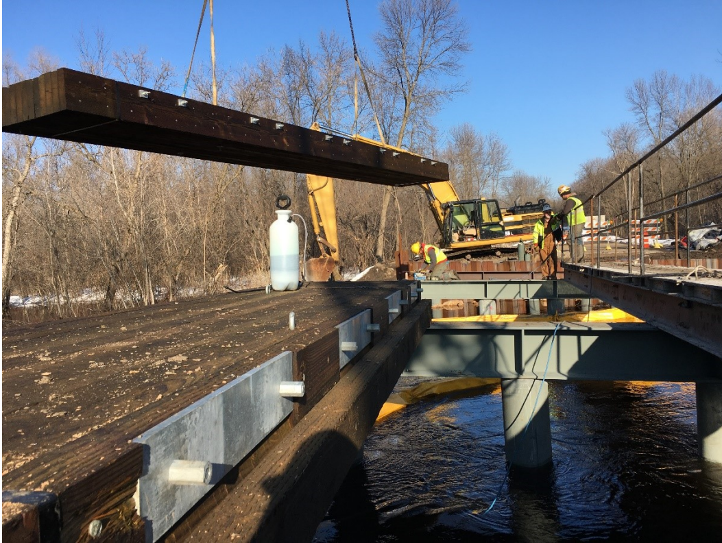
Figure 5.29 Panel C18 being installed using a crane on span 1. Steel plates are recessed into the deck panel outer lamination approximately 3-ft for the crash-tested bridge railing and curb system. Photo credit Hennepin County.
