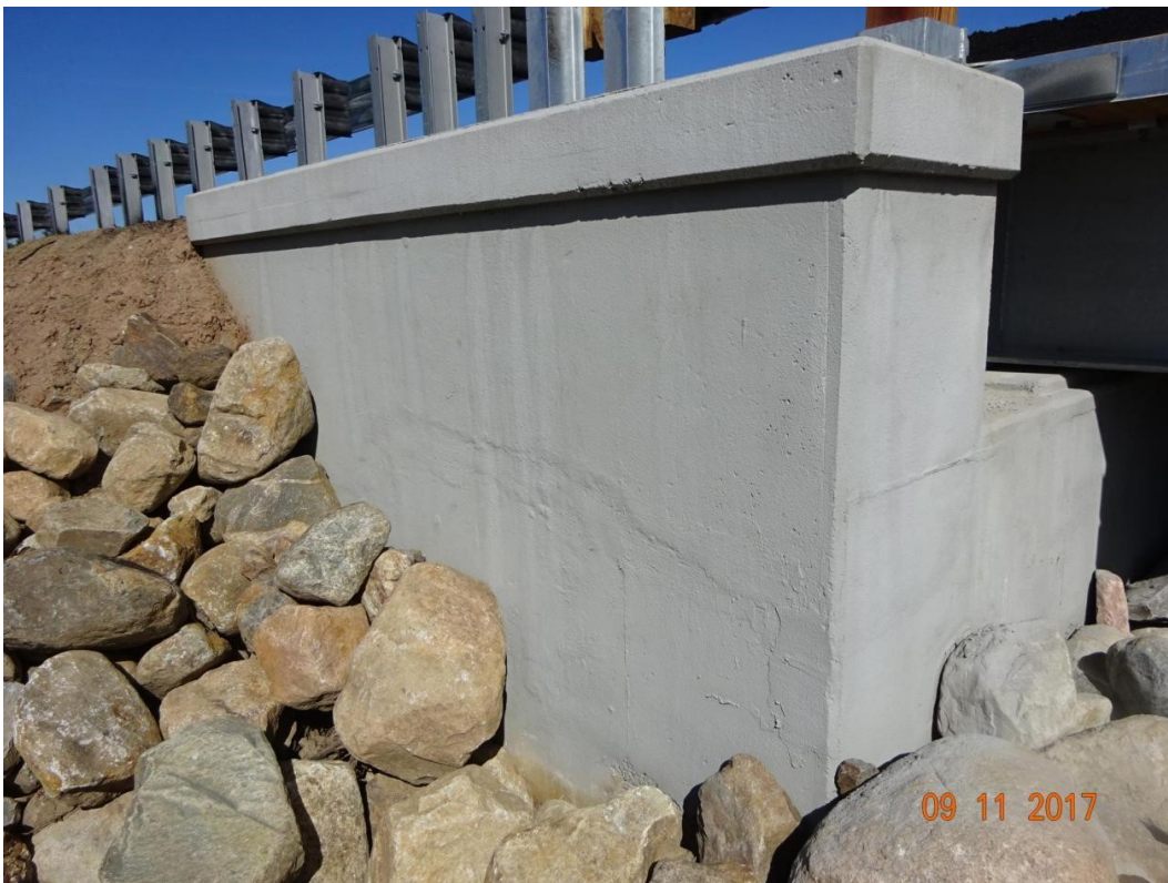
Figure 4.18 Downstream concrete abutment with riprap.
