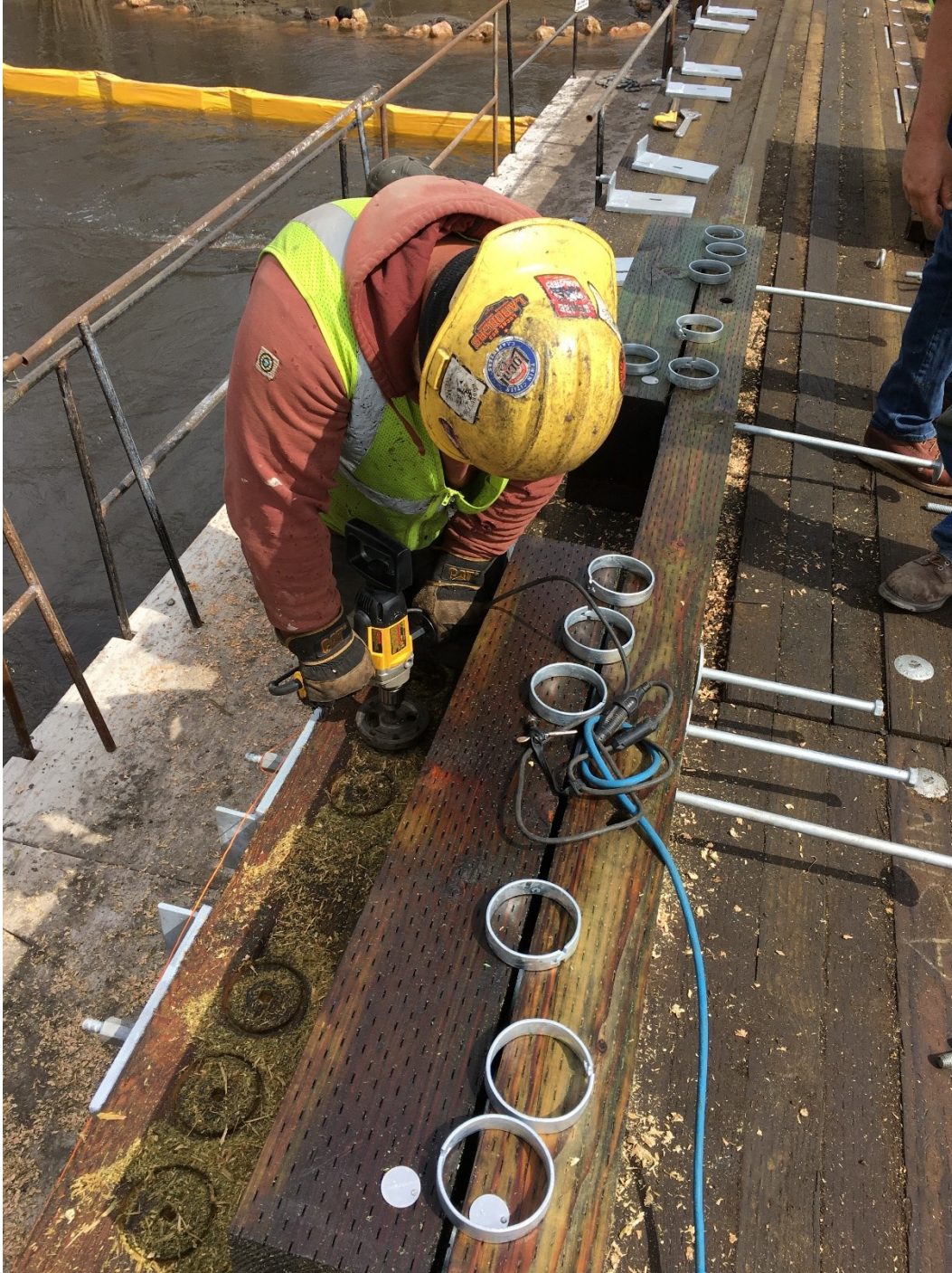
Figure 5.42 Predrilling split ring connectors for scupper to deck connection. Photo credit Hennepin County.
