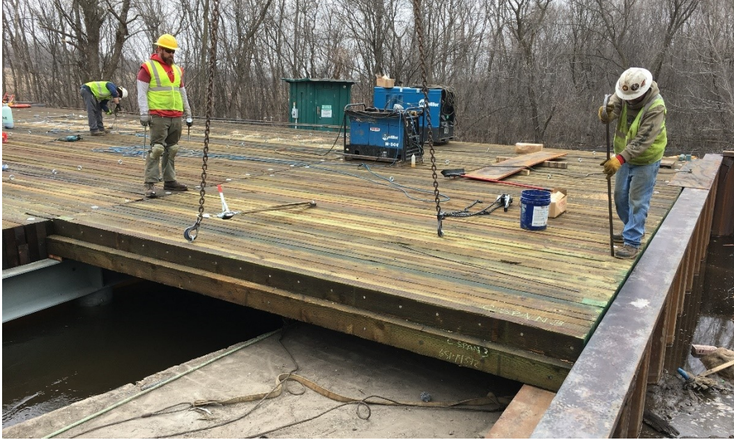
Figure 5.36 Panel installation and lever hoist used to tighten splice edge joints. Photo credit Hennepin County.
