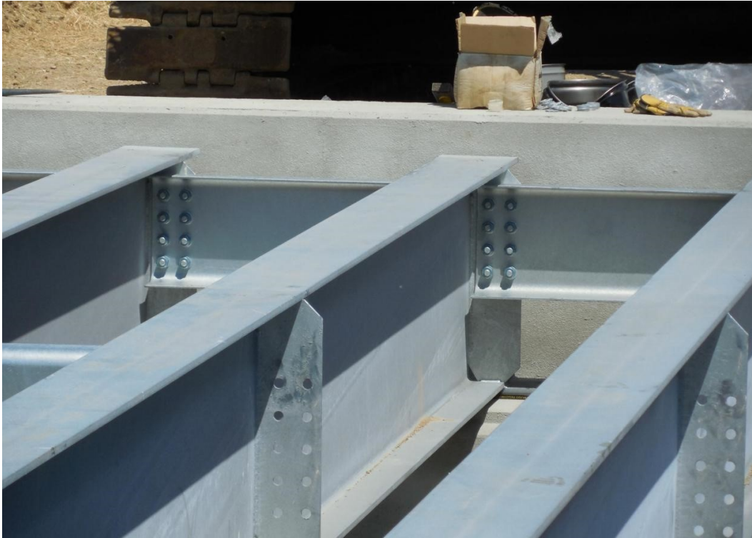
Figure 4.20 Steel diaphragm installation.
