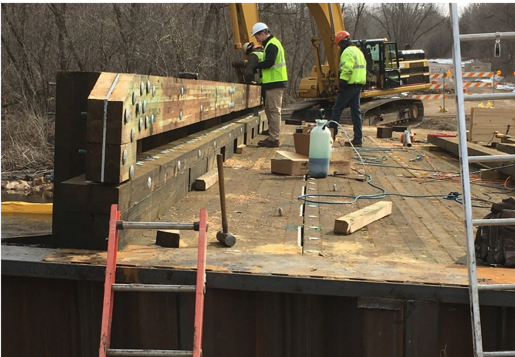
Figure 5.47 Finalizing crash-tested bridge railing and curb system installation on north edge of bridge. Photo credit Hennepin County.
