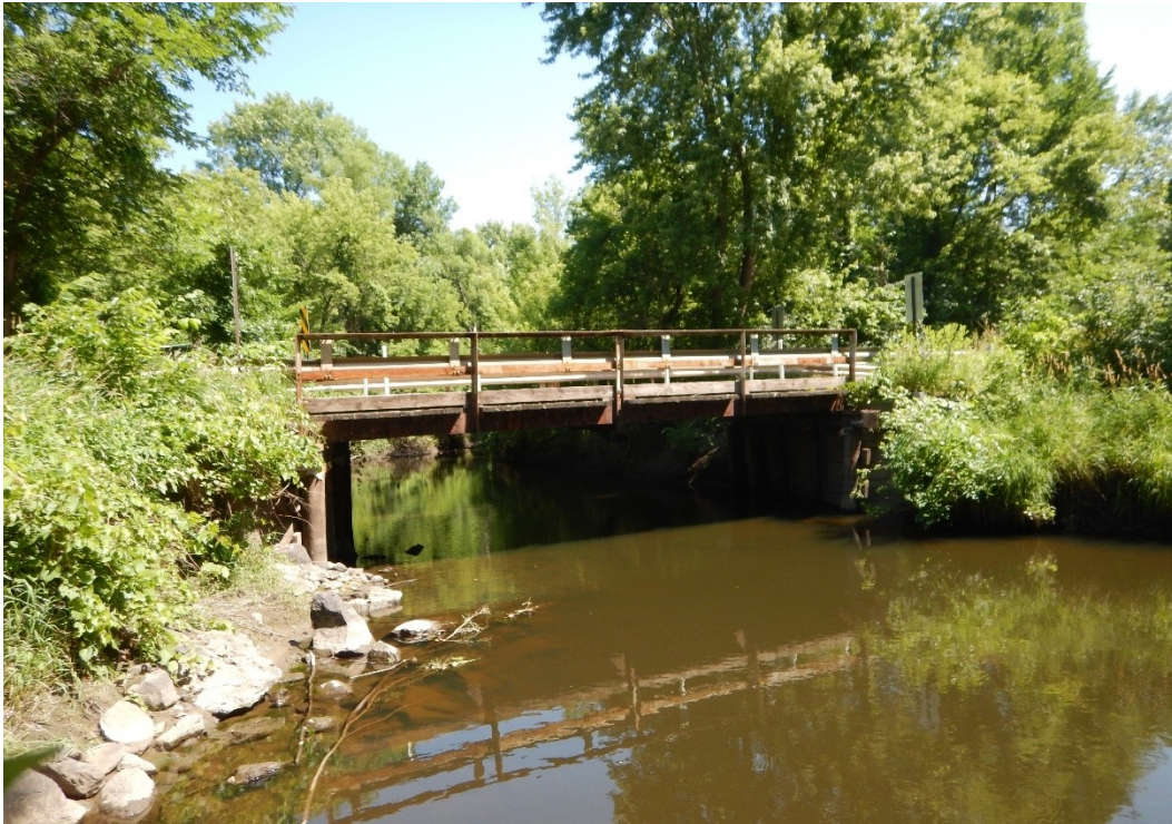
Figure 5.1 Original steel girder bridge (L8081) that was replaced during this project.
