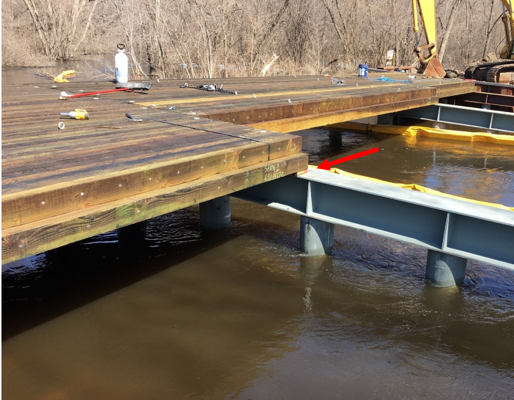
Figure 5.32 Installed panel for span 1 with sleeper blocking (identified with red arrow) at pier support to align top of timber decks. Photo credit Hennepin County.
