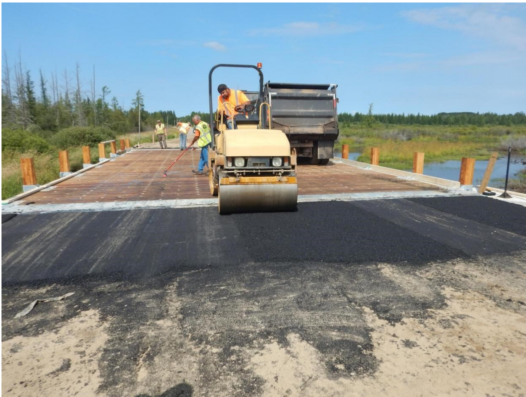
Figure 4.61 Both approaches were prepared with a bituminous wedge.
