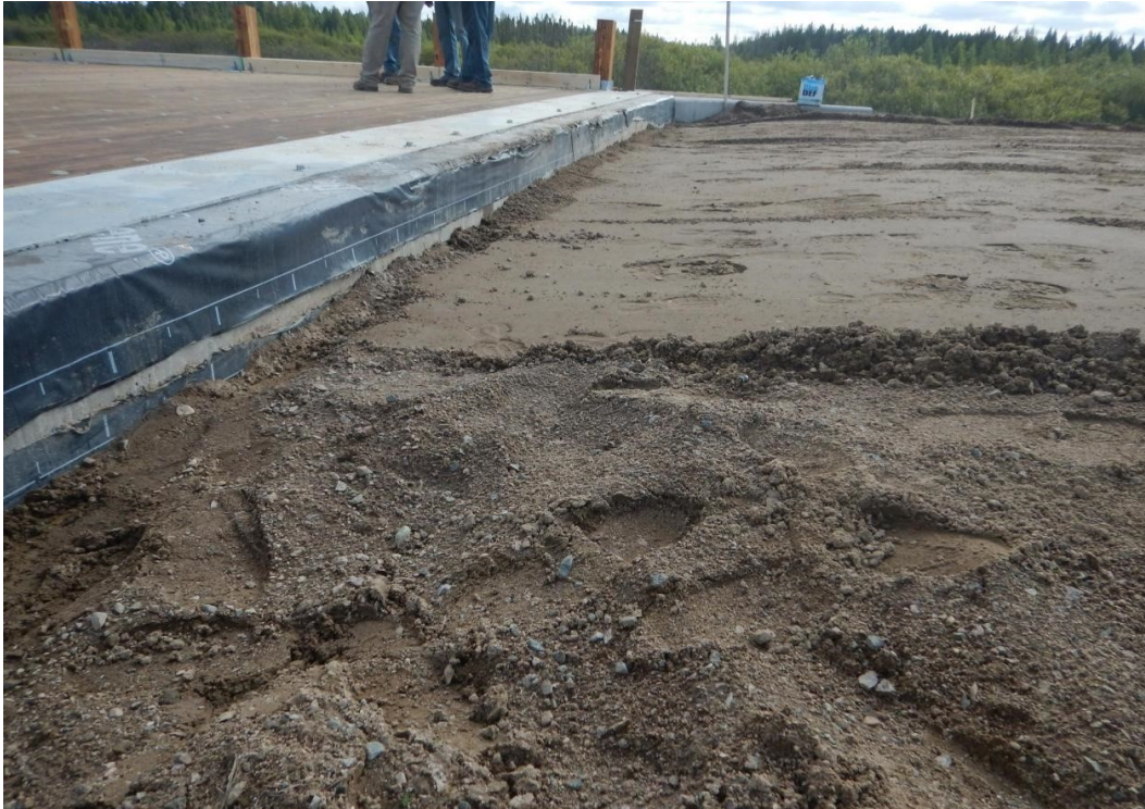
Figure 4.54 Shaping in preparation of the bituminous wedge.
