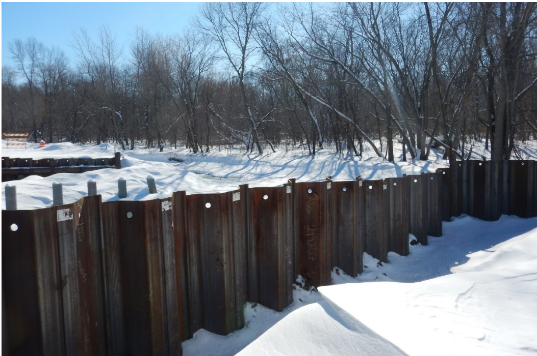
Figure 5.24 Sheet pile abutment wall and wing wall after installation.
