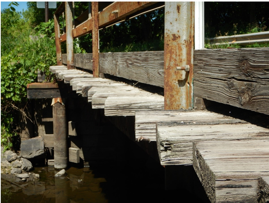
Figure 5.6 Transverse timber plank deck and steel railing system for bridge L8081.
