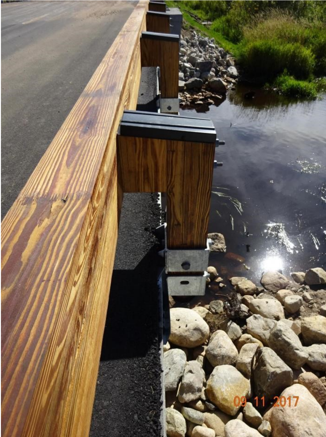
Figure 4.73 Side view showing TL2 curbless rail system used on this bridge and the installed plastic cap for moisture protection.
