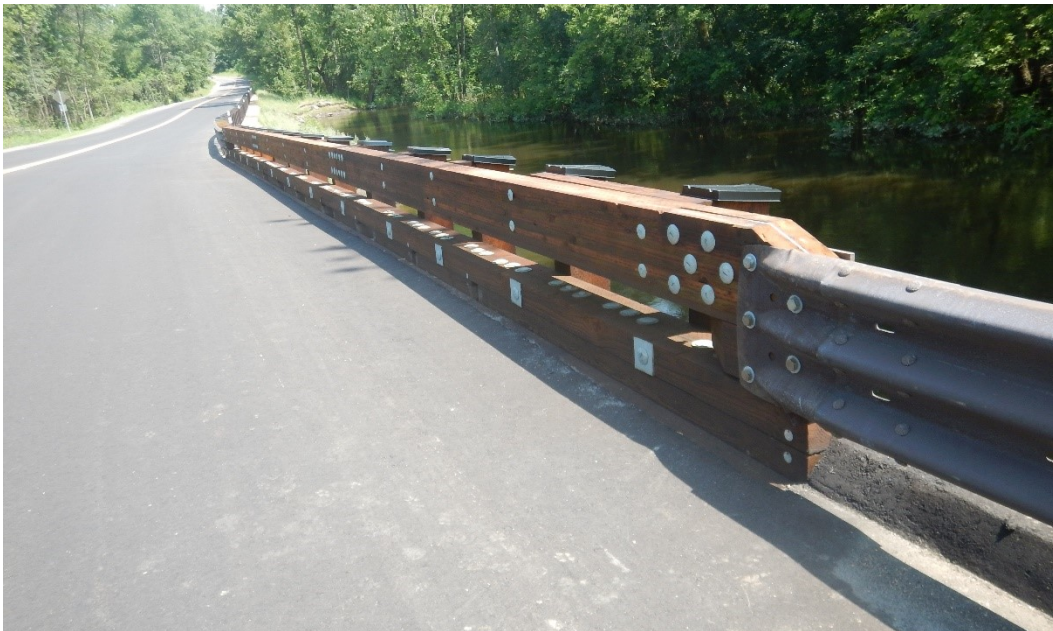
Figure 5.61 View showing TL4 rail system used on this bridge and the installed plastic cap for moisture protection.
