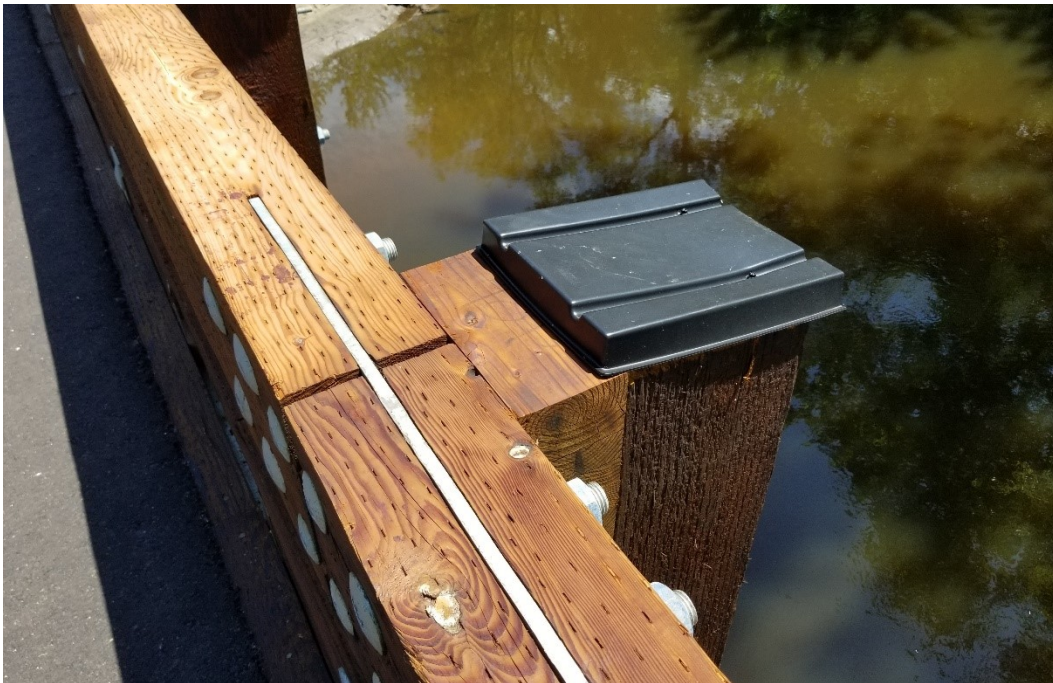
Figure 5.51 Plastic rail post flashing to divert water from rail post end grain. Preferred installation is for the screws to attach through the vertical side of the cap.
