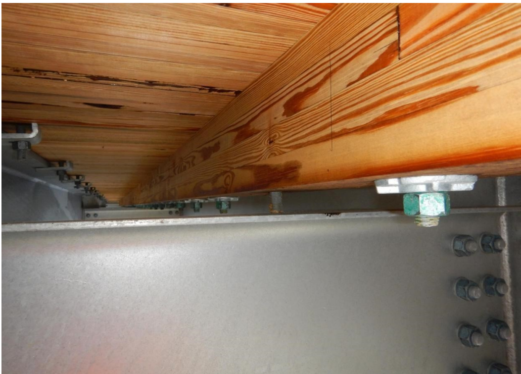
Figure 4.36 Close-up of glulam stiffener bolts, malleable washers and nuts.
