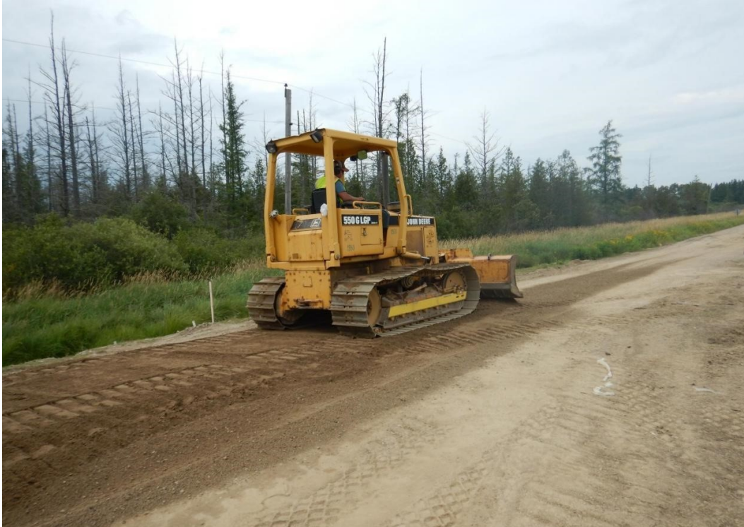
Figure 4.52 Leveling the approach prior to bituminous installation.
