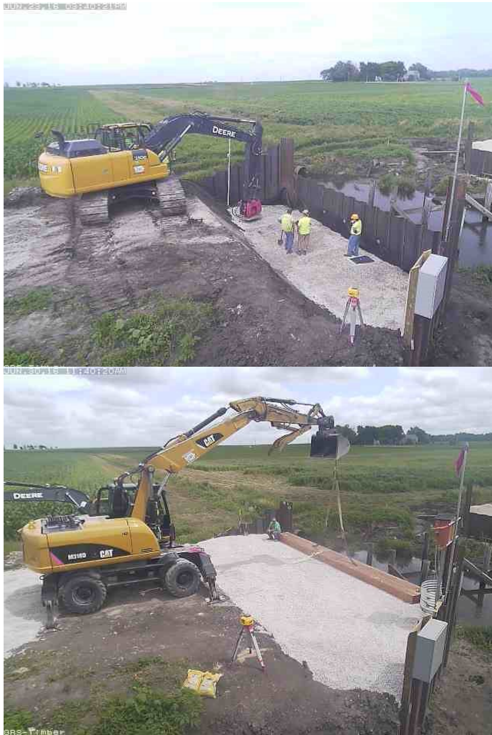
Figure 3.3 GRS abutment during construction in Buchanan County, Iowa (2016).
