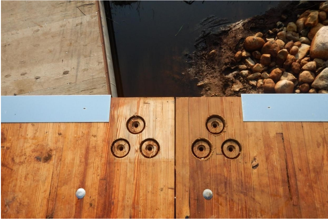
Figure 4.44 Flashing between rail posts was installed first using galvanized roofing nails.
