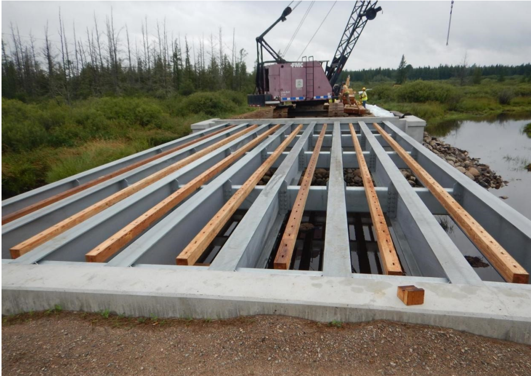
Figure 4.28 Stiffeners in place prior to deck installation.
