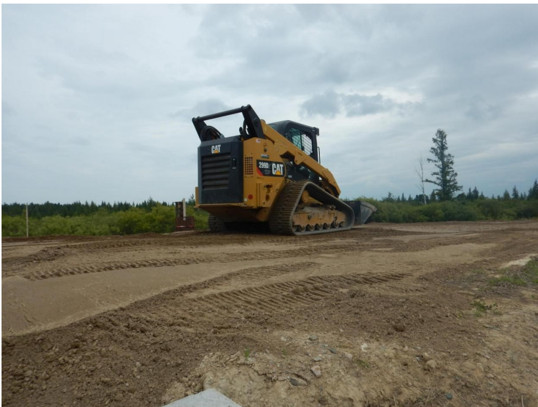
Figure 4.53 Shaping and leveling the approach prior to bituminous installation.
