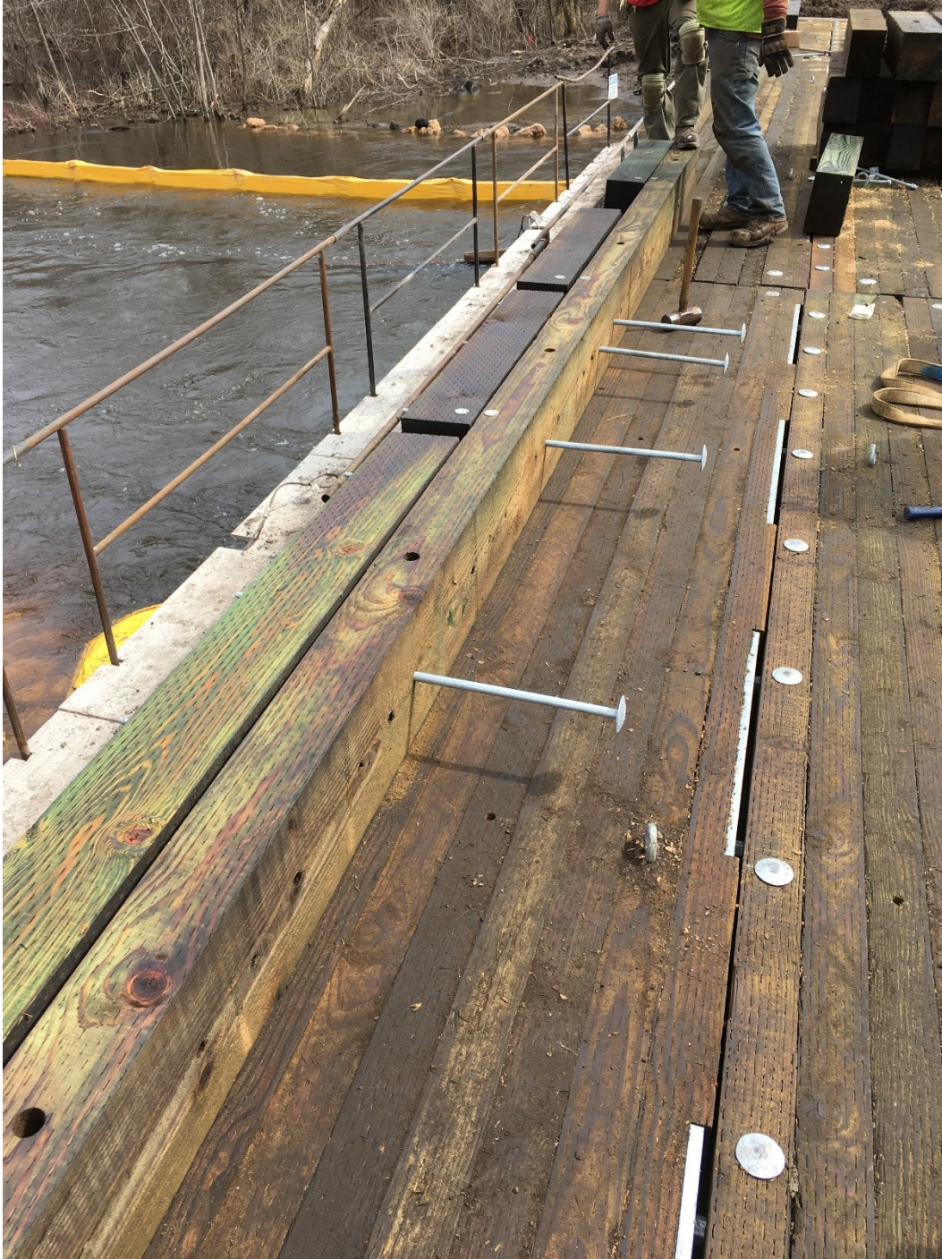
Figure 5.41 Prefabrication of the timber curb and scupper blocks (laid out on their side) prior to connection to the deck panels along the north deck edge. Photo credit Hennepin County.
