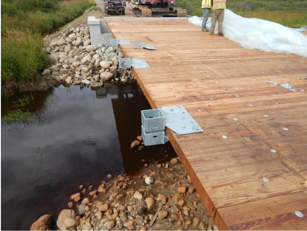
Figure 4.39 Post hardware was test fit to ensure proper panel placement.
