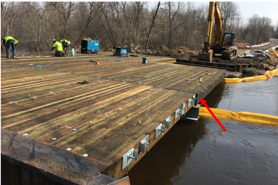
Figure 5.35 Span 2 panels installed indicating excess width due to misalignment on downstream deck edge that required slight modification. Photo credit Hennepin County.
