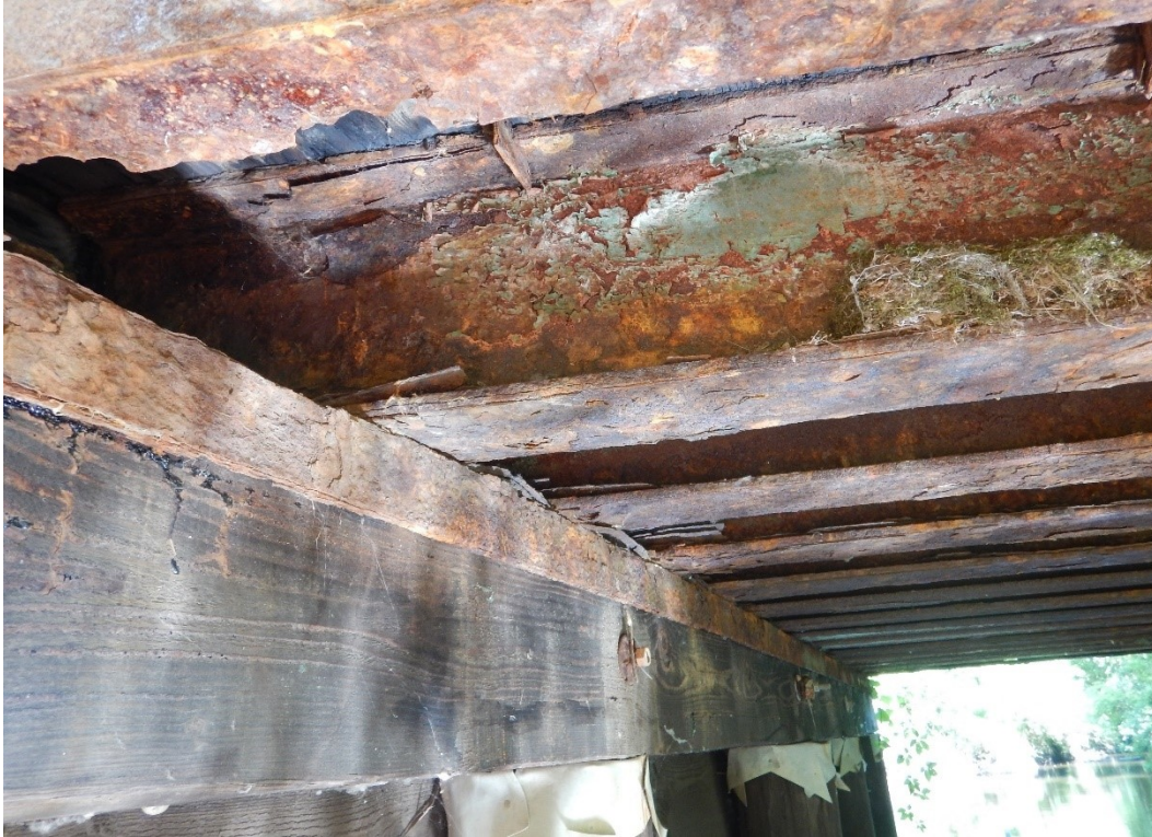
Figure 5.5 Close up of steel girder bearing on timber pile and cap abutment for bridge L8081.
