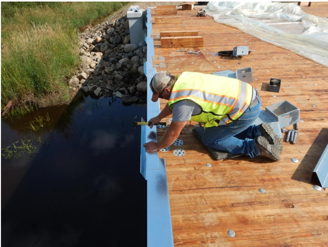
Figure 4.45 Flashing at posts was installed after the between post flashings.
