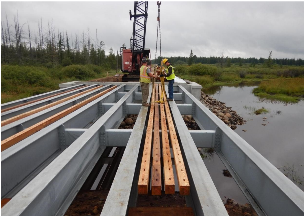
Figure 4.27 Stiffeners were placed between each steel beam.
