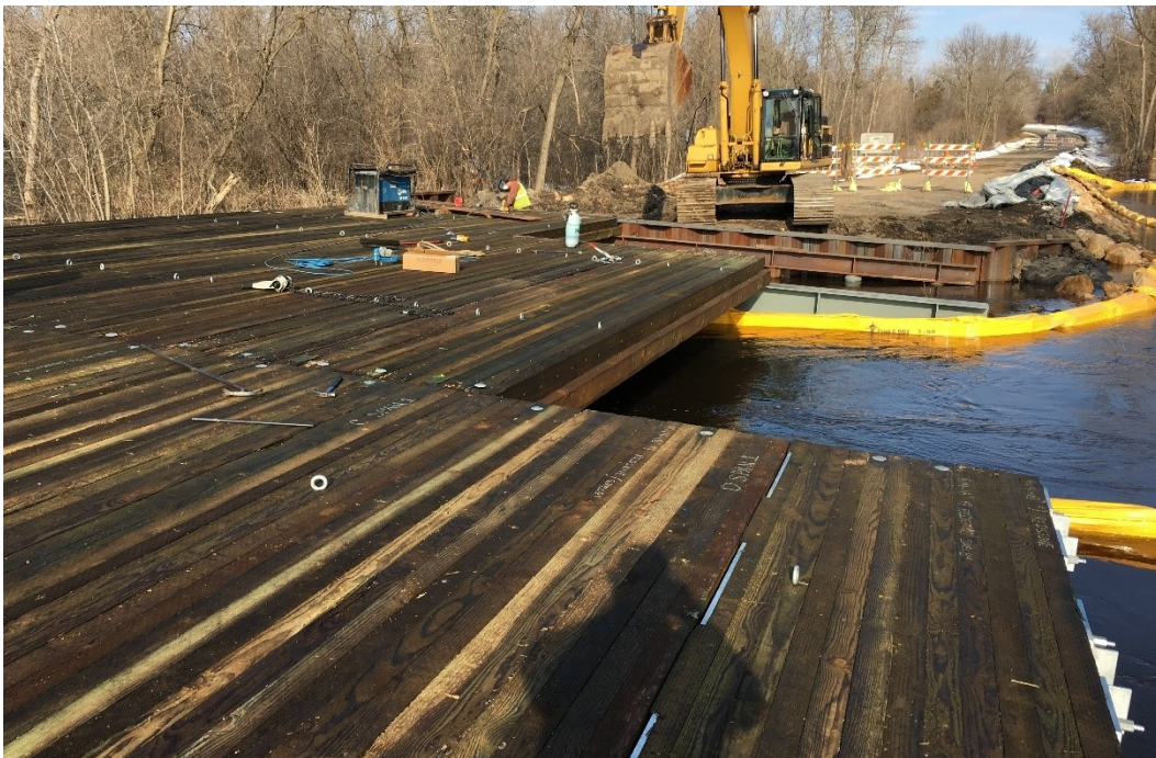
Figure 5.33 Panel installation in progress for spans 1, 2, and 3. Photo credit Hennepin County.
