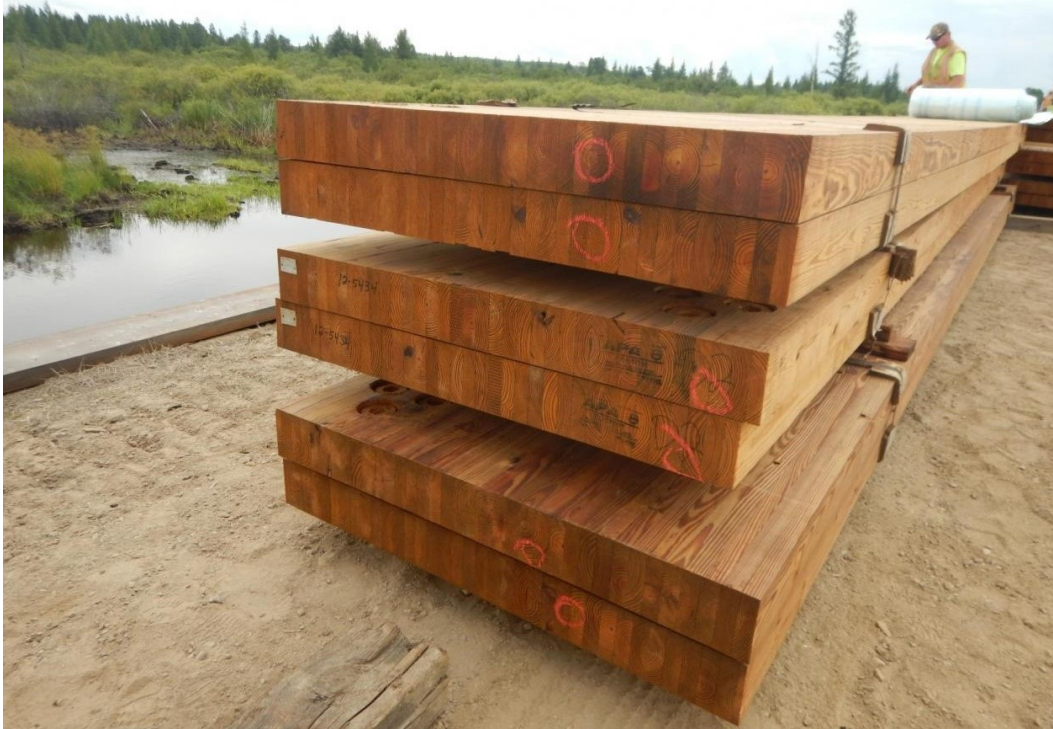
Figure 4.23 Glulam panels after delivery and unloading at the construction site.
