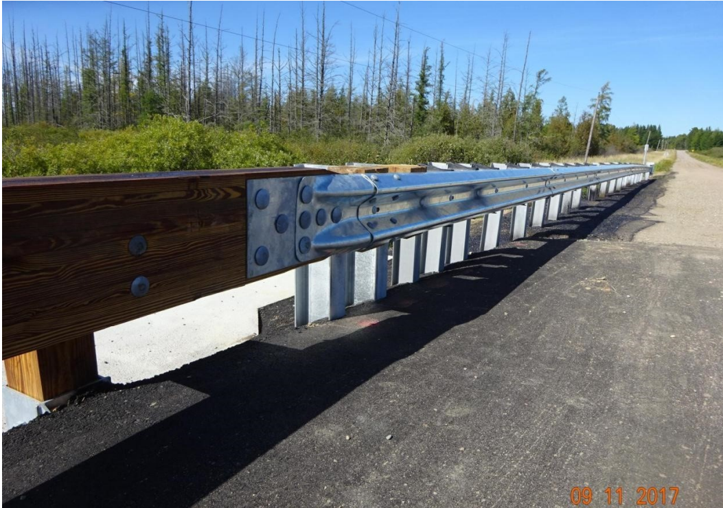
Figure 4.74 Guard rail attached to the glulam rail system.
