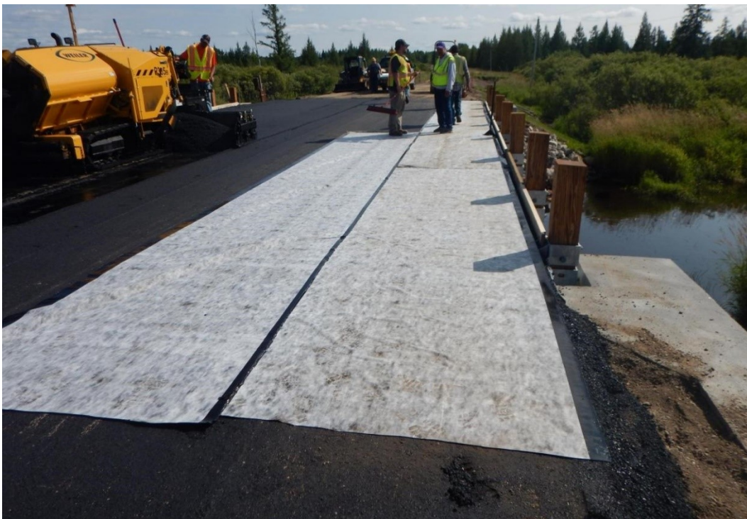
Figure 4.67 Each row of waterproof membrane was overlapped by 4 inches according to specifications.
