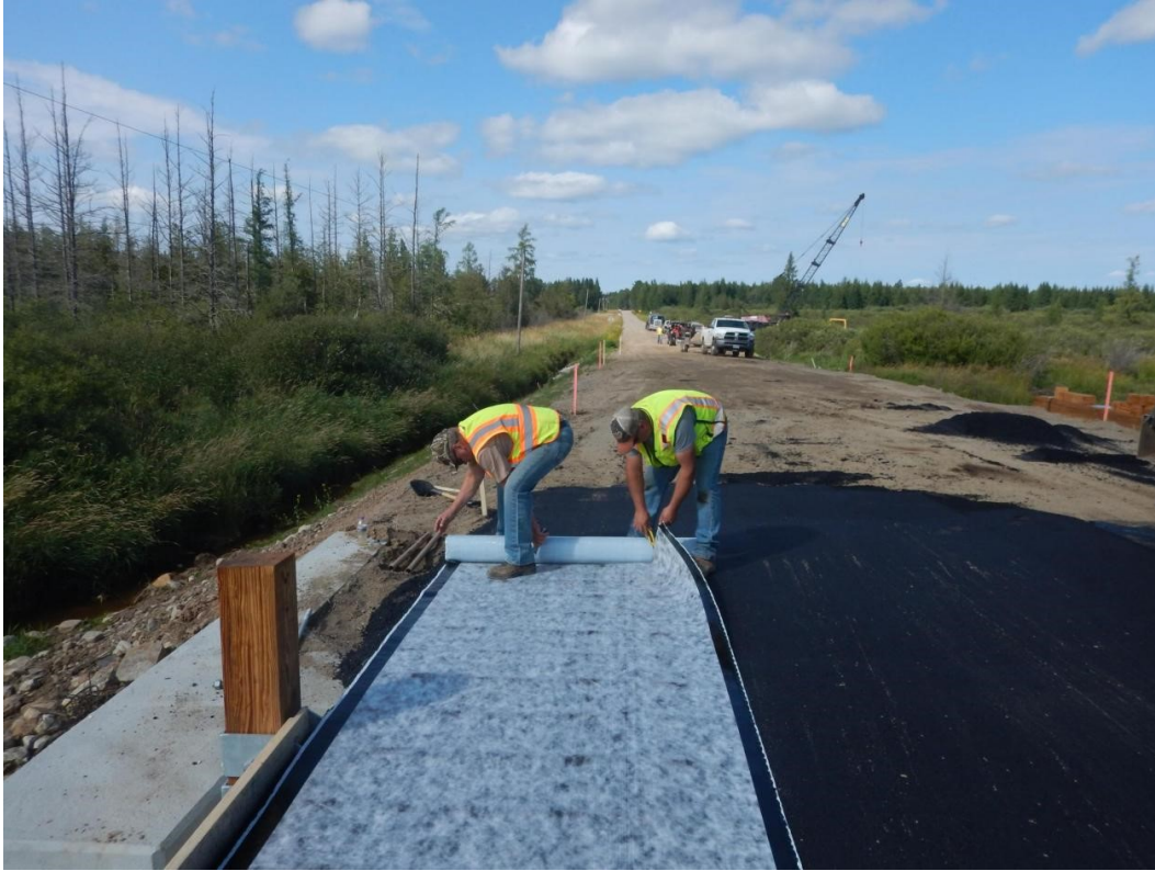
Figure 4.66 Installation of waterproof membrane between layers of bituminous.
