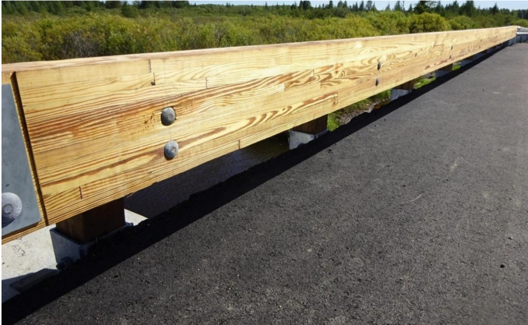
Figure 4.71 Glulam railing installation.
