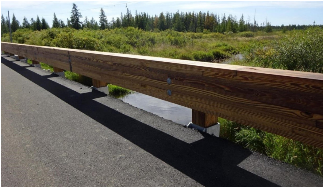
Figure 4.72 Glulam rail installation.
