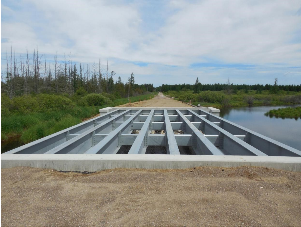
Figure 4.22 Installed steel beams and diaphragm stiffeners.
