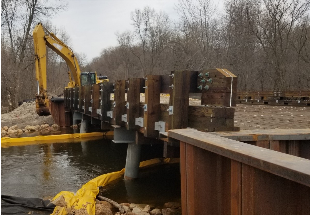
Figure 5.46 Rail posts, spacers and railing installed on north edge of bridge. Photo credit Hennepin County.
