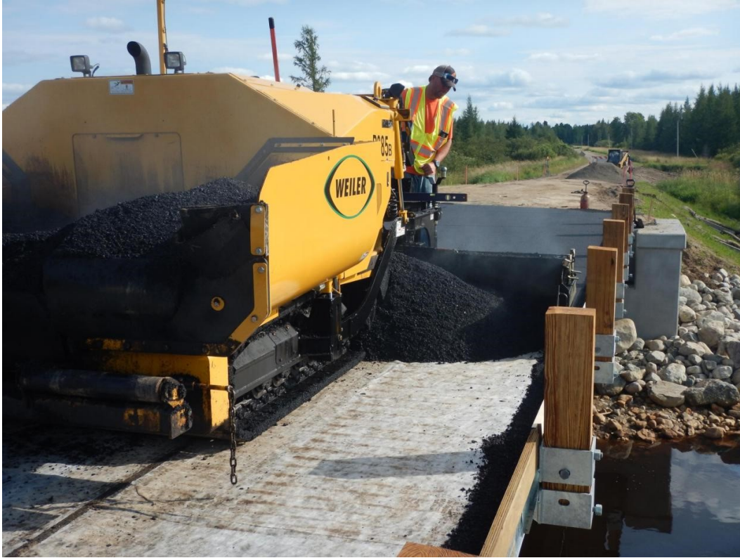
Figure 4.70 Second layer of bituminous added to the membrane.
