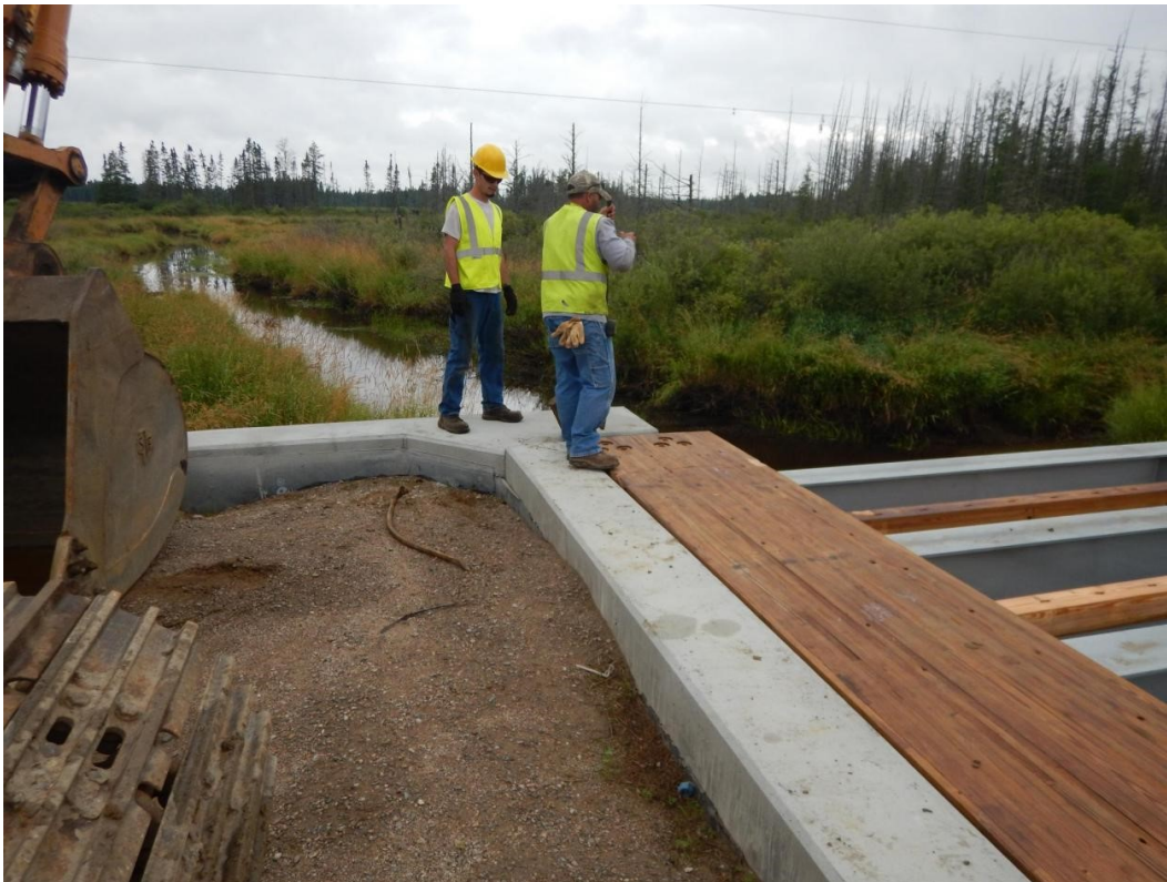
Figure 4.30 The first transverse panel was placed on the south side of the bridge.
