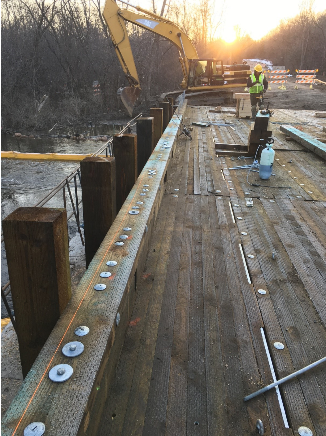
Figure 5.45 Curbs, scupper blocks, and rail posts installed along the north edge of the bridge. Embedded steel plates are to reinforce the bridge railing against vehicle impact forces. Photo credit Hennepin County.
