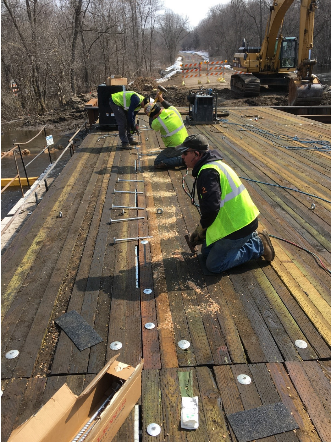
Figure 5.31 Dome head drive spikes being installed into the panel splice joint. Note the embedded steel plates at this location are installed to help anchor the crash-tested bridge railing and curb system. Photo credit Hennepin County.
