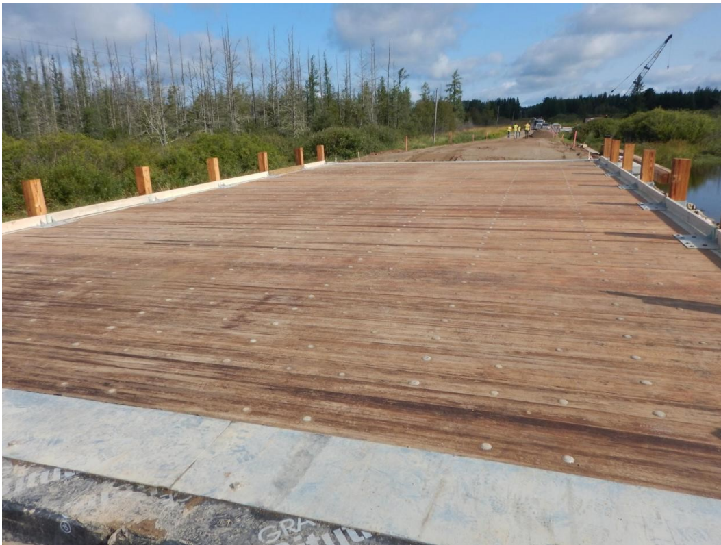
Figure 4.59 The bridge deck was swept clean, paving edge installed and ready for paving.
