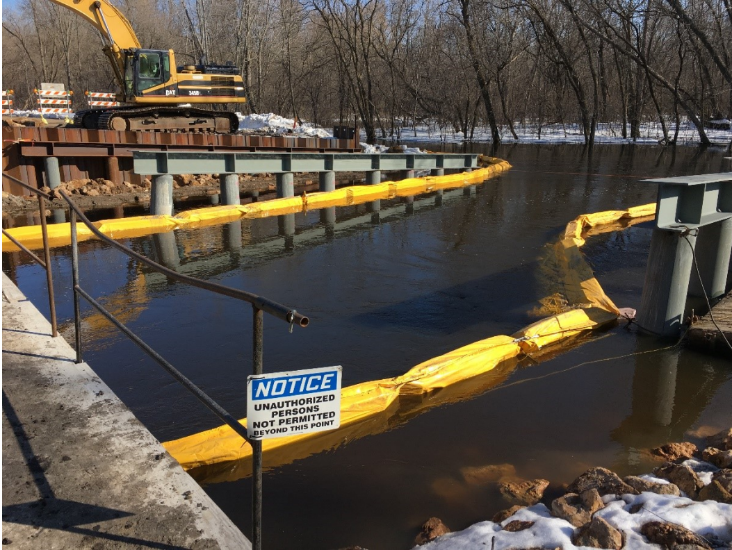
Figure 5.27 Substructure showing completed abutments, piers and pollution prevention flotation prior to timber deck installation. Piles are of different heights to meet required roadway super elevation. Photo credit Hennepin County.
