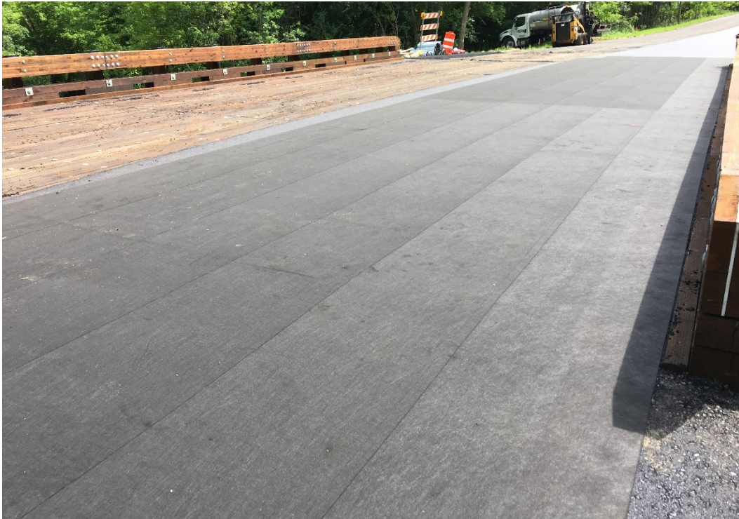
Figure 5.55 Bituminous reinforcing membrane after installation onto the (base course) bituminous layer. Photo credit Hennepin County.
