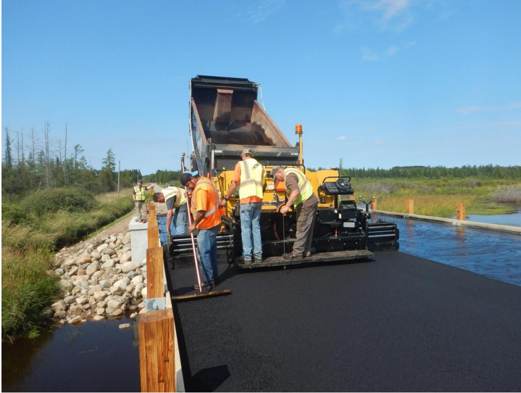
Figure 4.64 Overlay work along paving edge.
