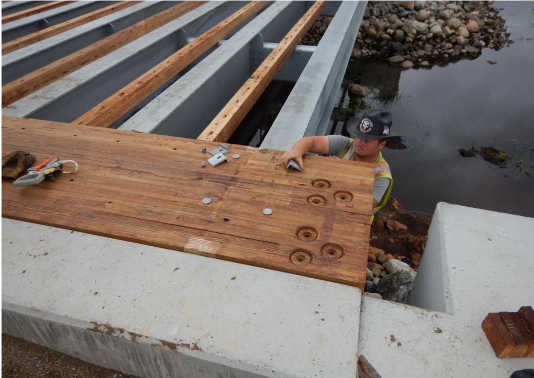
Figure 4.31 A galvanized clip system was used to attach each panel to the steel beam.
