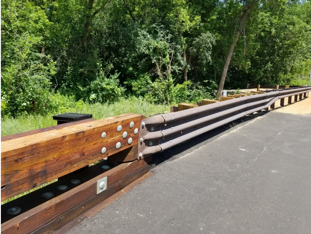
Figure 5.60 Approach semi-rigid guardrail system along north side of roadway.
