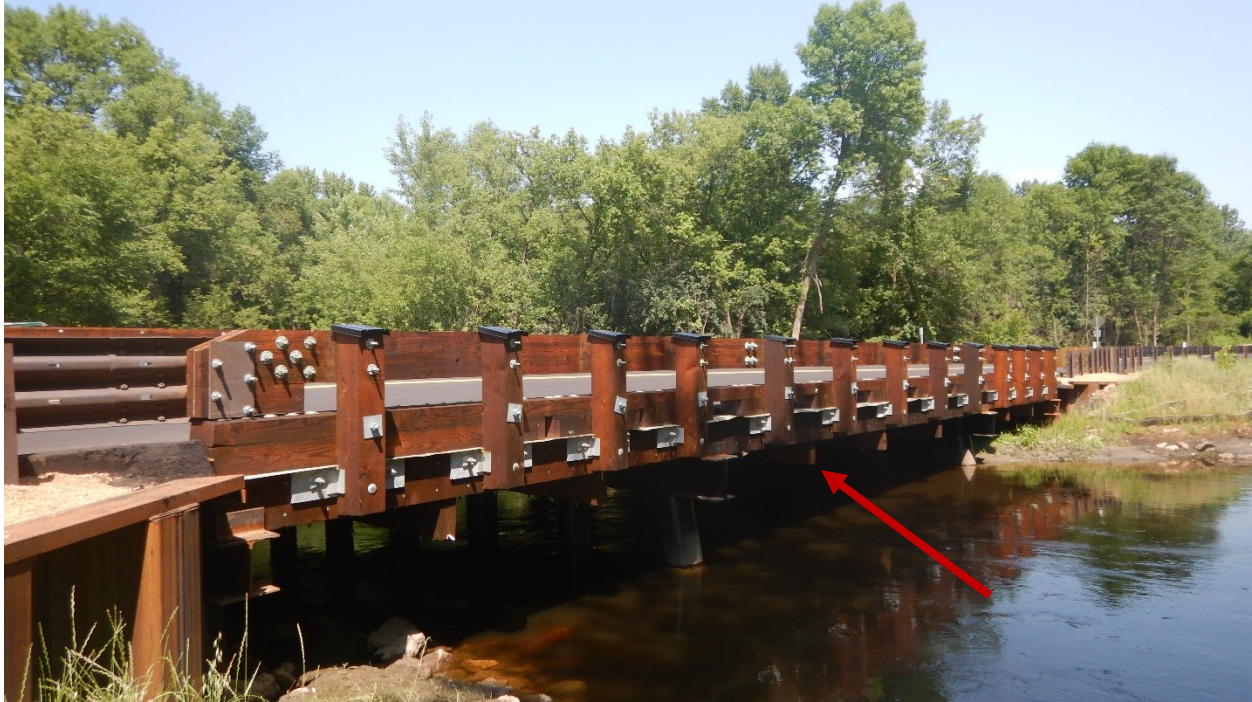
Figure 5.8 Completed picture of dowel-laminated deck with metal spikes, transverse spreader beams (highlighted with red arrow), and railings.
