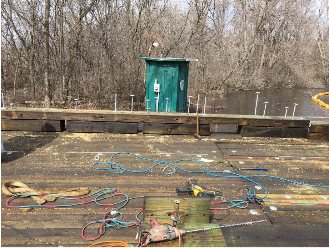
Figure 5.44 Curb and scupper aligned prior to connection to deck panels. Photo credit Hennepin County.
