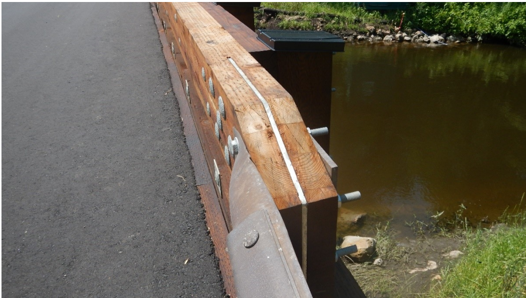
Figure 5.59 Glulam rail splice connection detail with steel approach railing.
