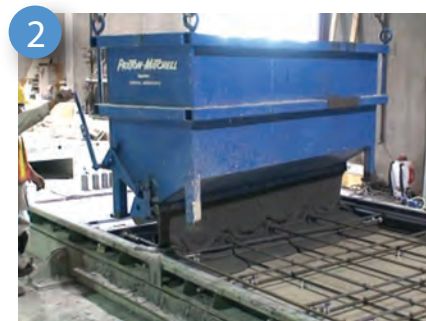
Placing the UHPC
