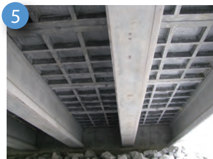
Underside of Bridge
