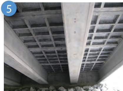
Underside of Bridge
