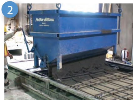
Placing the UHPC
