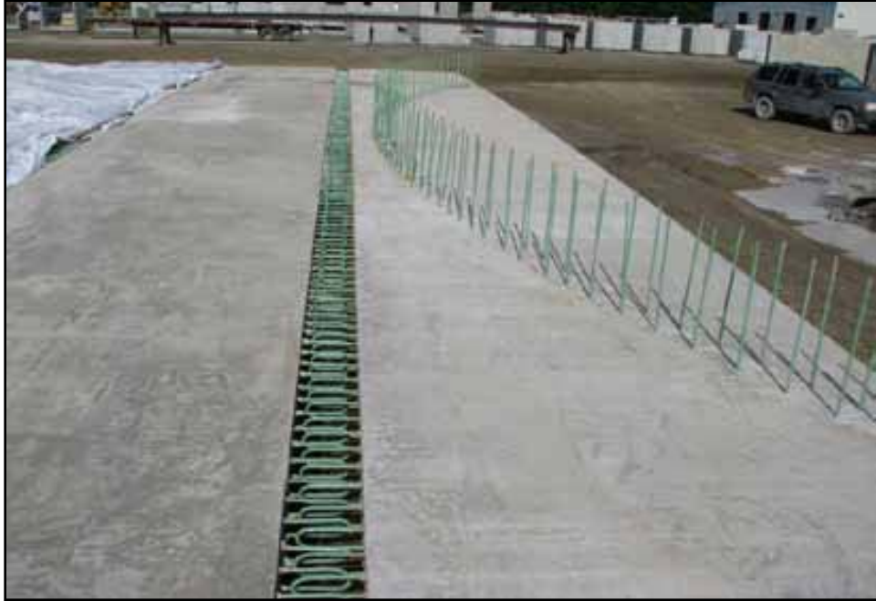
Figure 19. Adjacent superstructure units with connection reinforcement.
