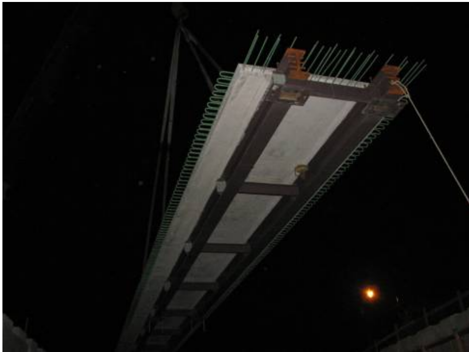
Figure 18. Installation of superstructure unit.
