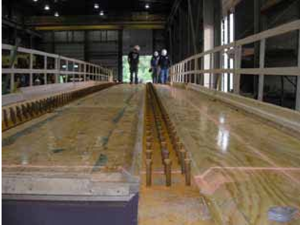
Figure 15. Formwork for a precast superstructure unit.
