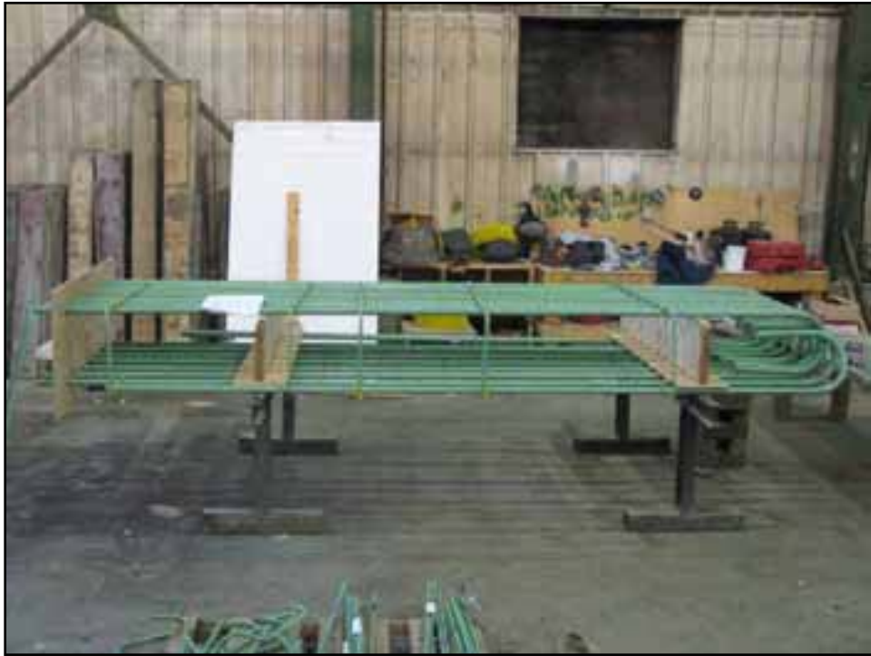
Figure 6. Reinforcement for precast pier unit.
