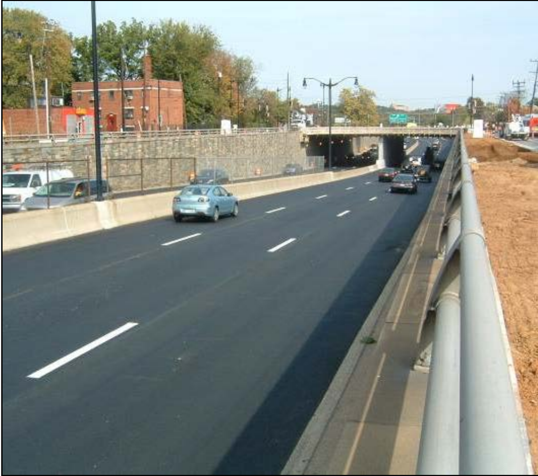
Figure 21. Traffic flow upon completion of work on Kenilworth Avenue.
