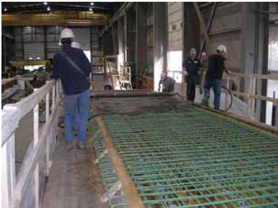
Figure 16. Steel reinforcement for a precast superstructure unit.
