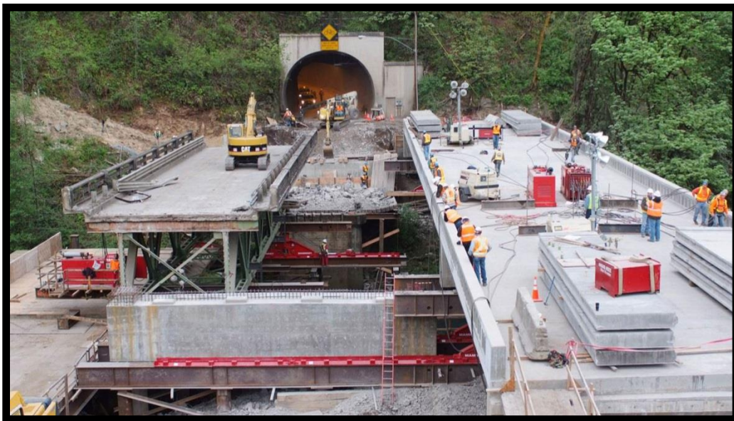
Figure 1-5 SIBC with Constraints Limiting Traffic Control Options at the OR-38 Bridge Project, Oregon
