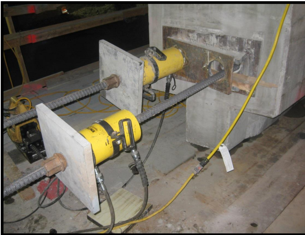
Figure 4-7 PT Jacks on Threaded High-Strength Bars Push Bridge into Place
