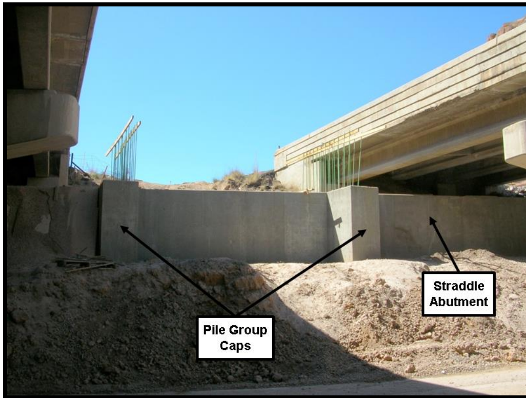
Figure 3-9 Straddle Abutment on the I-80 Echo Road Bridge Project, Utah
