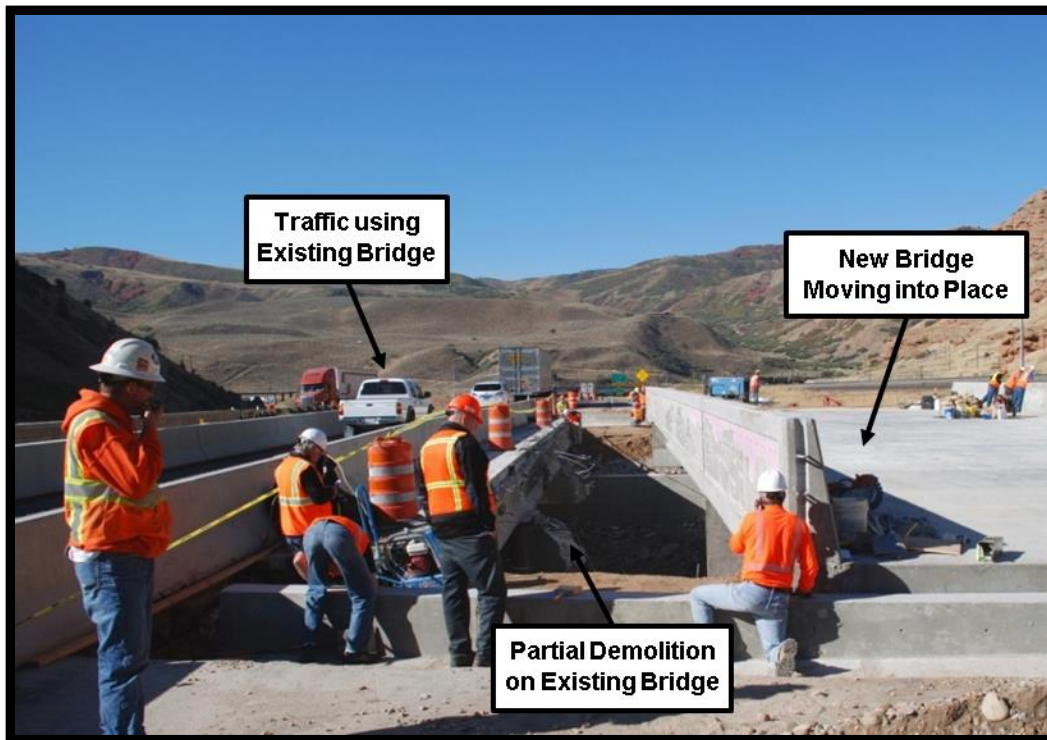
Figure 4-8 SIBC Showing Partial Demolition on the Existing Bridge while Maintaining Traffic
