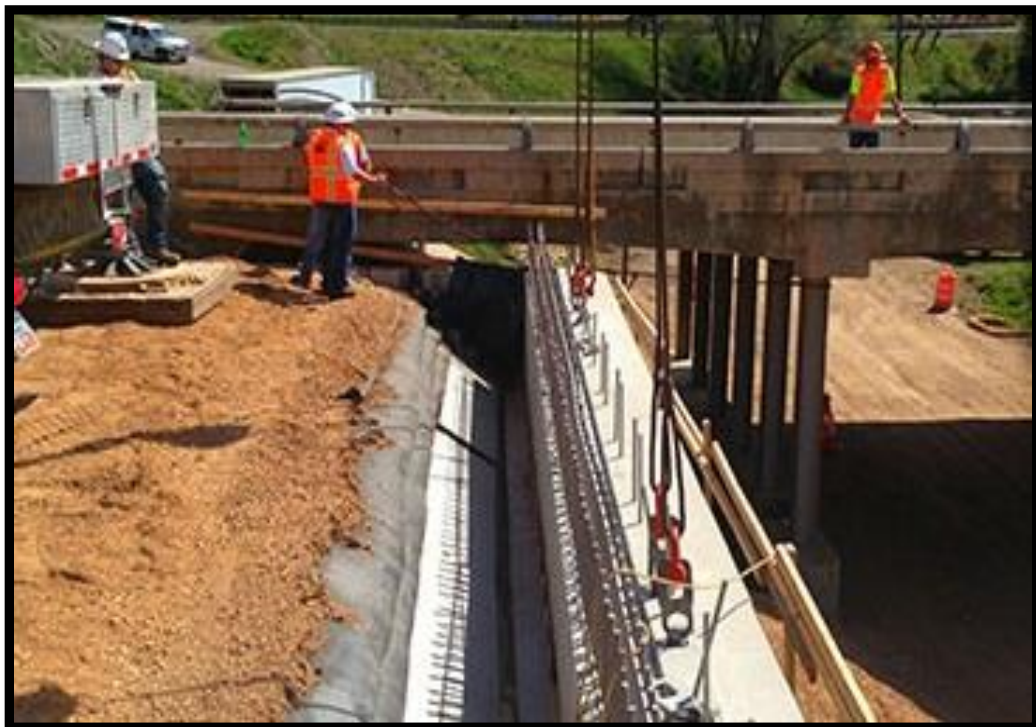
Figure 3-6 GRS System for the I-84 Echo SIBC Project, Utah
