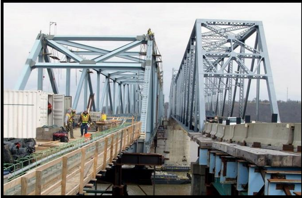
Figure 1-3 SIBC for a Large Truss Bridge on the Milton-Madison Bridge Project, Indiana/Kentucky
