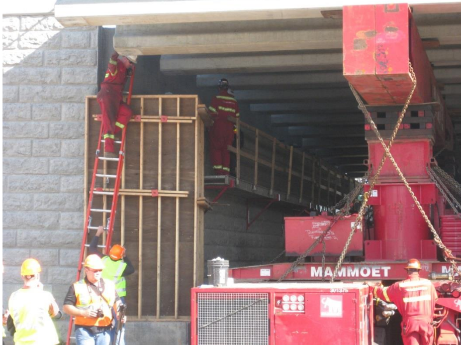
Figure 70. Photo. The vertical and horizontal positions of all girders of the span were carefully monitored from the abutment to ensure that it was lowered uniformly so as to not excessively stress the girders, deck, and pier columns, which could potentially cause cracking or other distresses.
