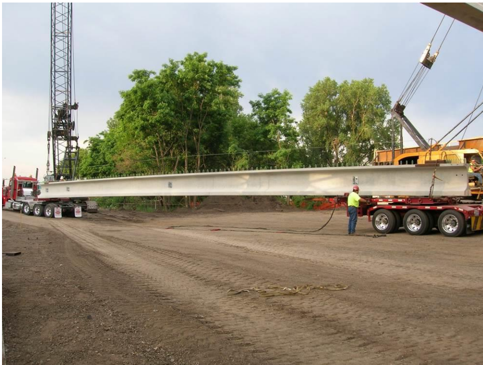
Figure 14. Photo. 103-ft prefabricated concrete girders were shipped one at a time from the fabrication plant to the bridge staging area on trucks equipped with steering trailers.
