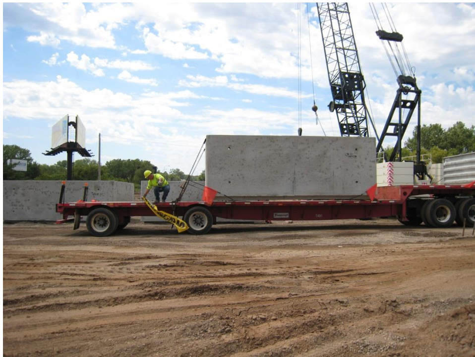
Figure 54. Photo. Shipping the sections on flatbed trucks for the prefabricated elements of the box culvert bridge tunnel beneath Maryland Ave.
