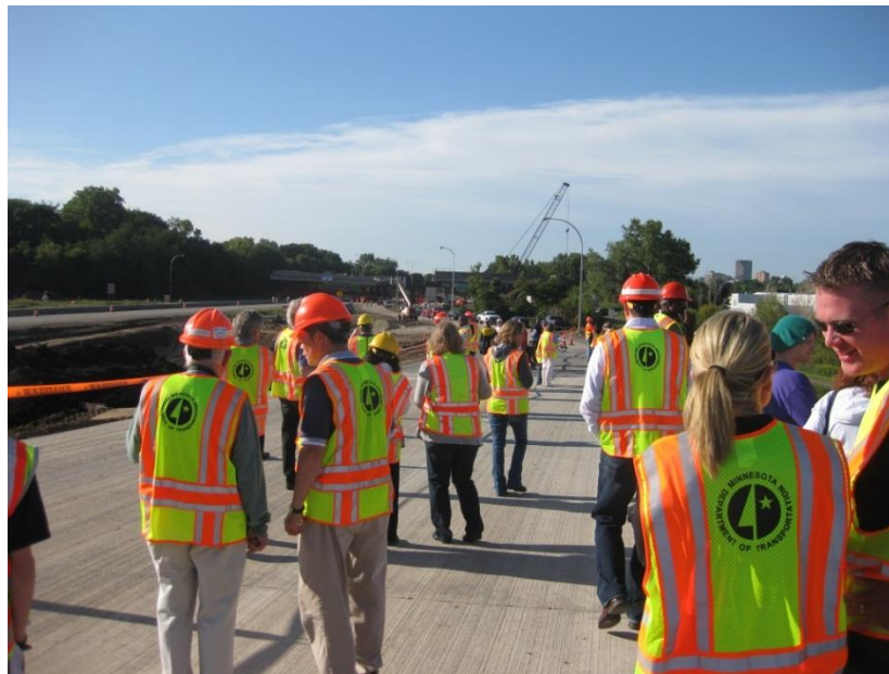
Figure 86. Photo. MnDOT staff observing the moving of the Maryland Ave. bridge using the SPMT.
