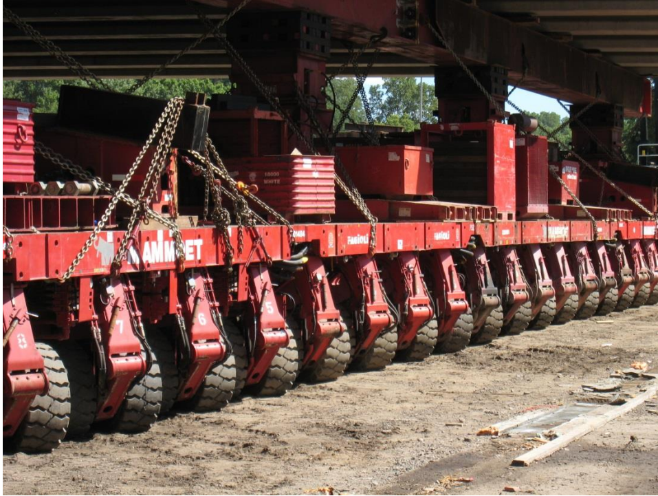
Figure 59. Photo. An SPMT is a computer-controlled platform vehicle with a large array of articulating wheels on the bottom. The SPMT used for this project had a total of 288 wheels on 2 sets of 18 axles.
