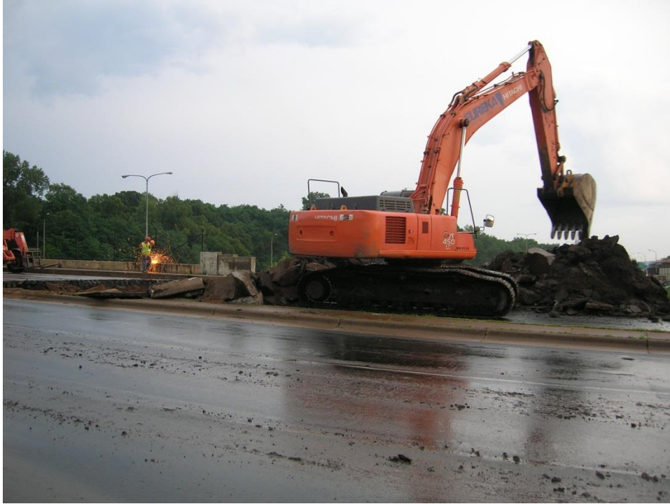
Figure 40. Photo. Demolishing Maryland Ave. bridge 6513.
