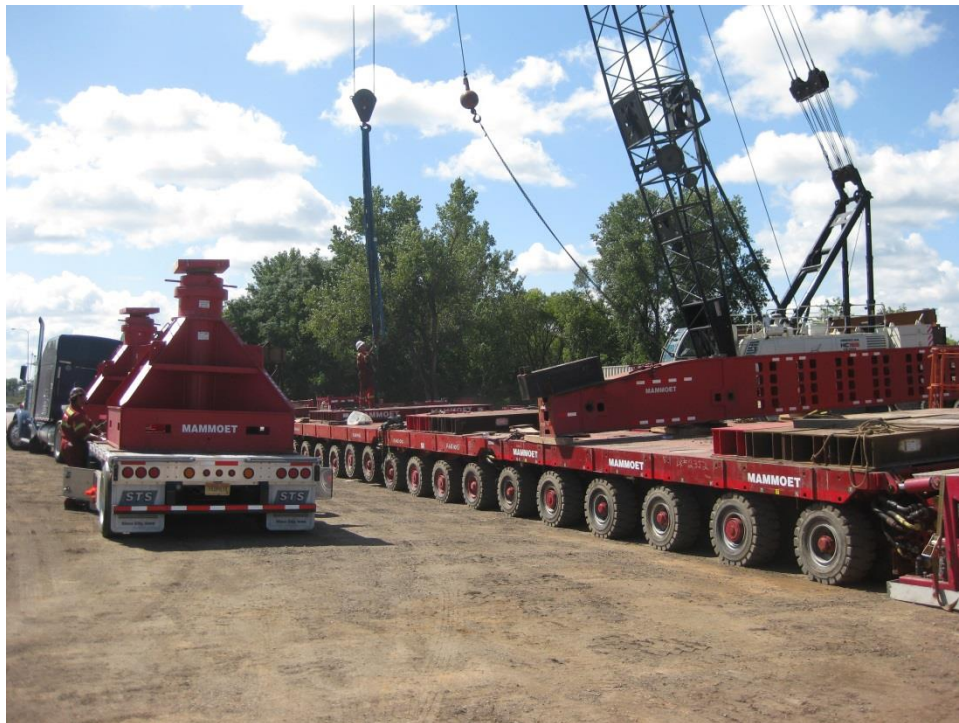
Figure 61. Photo. The SPMT was stripped down and shipped to the job site on a total of 30 flatbed trucks and reassembled at the job site for this project.
