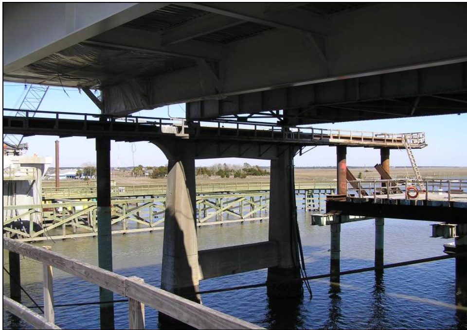
Figure 4. Approach span existing piers.
