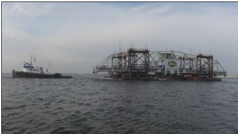
Figure 11. New swing span being transported to the bridge site.
