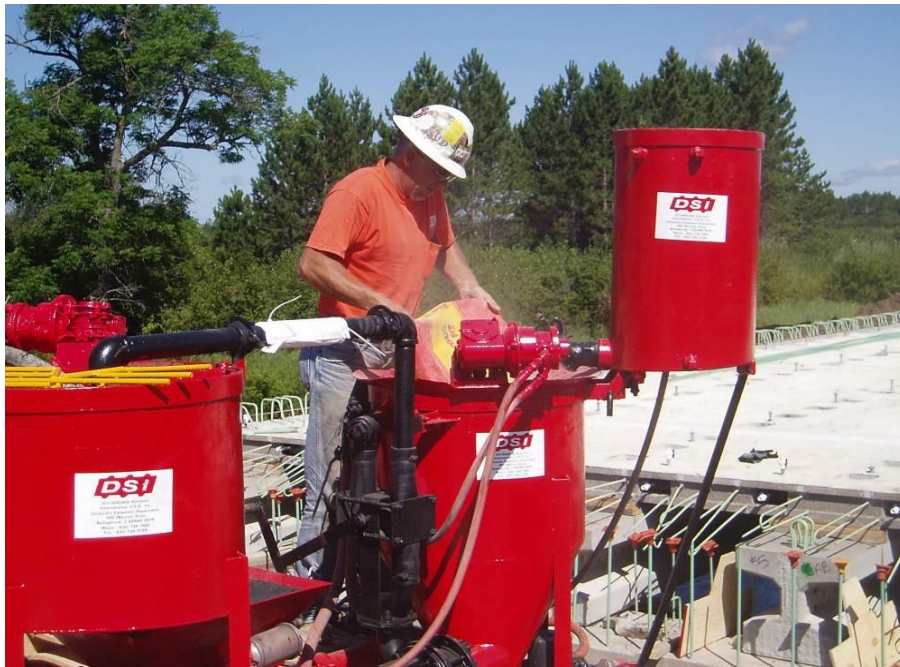
Figure 63. Equipment for mixing and pumping post-tensioning duct grout.
