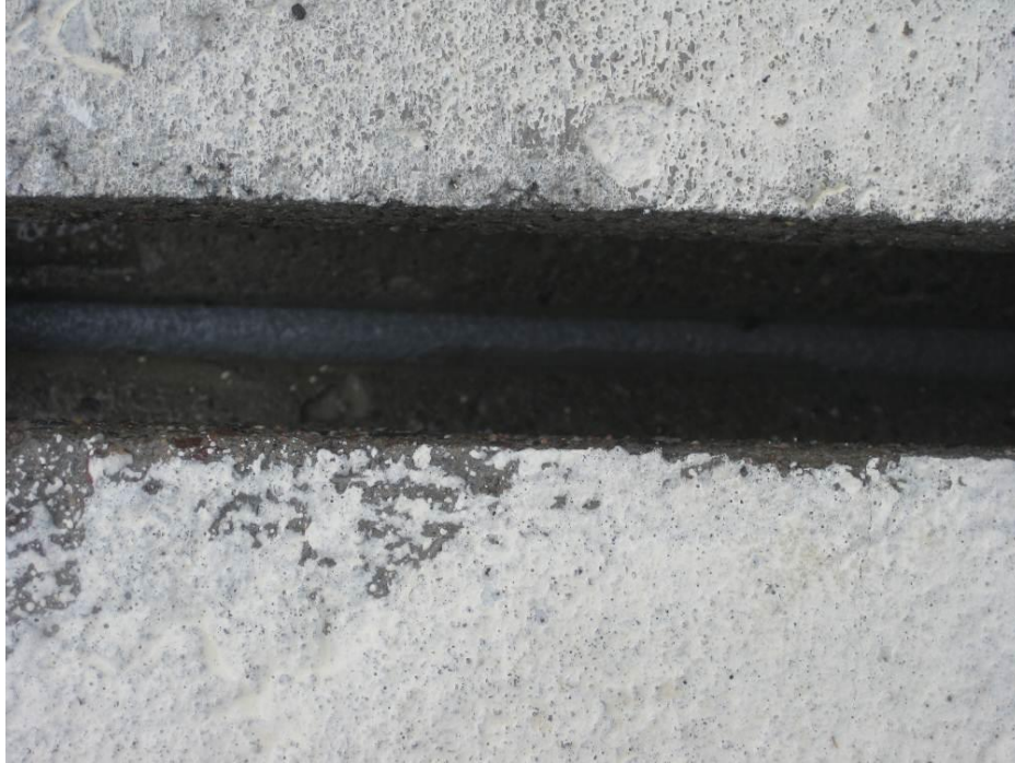
Figure 42. View of the backer rod from the top of the deck panels. The backer rod prevents the grout poured into the transverse joint keyway from escaping.
