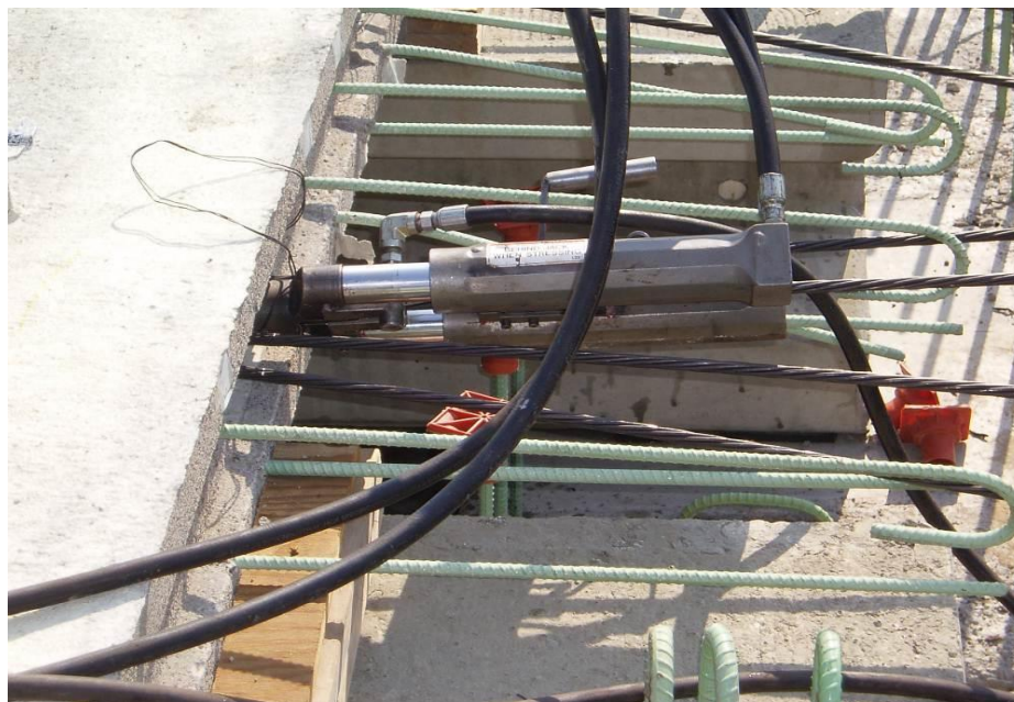
Figure 61. Post-tensioning the steel strands.
