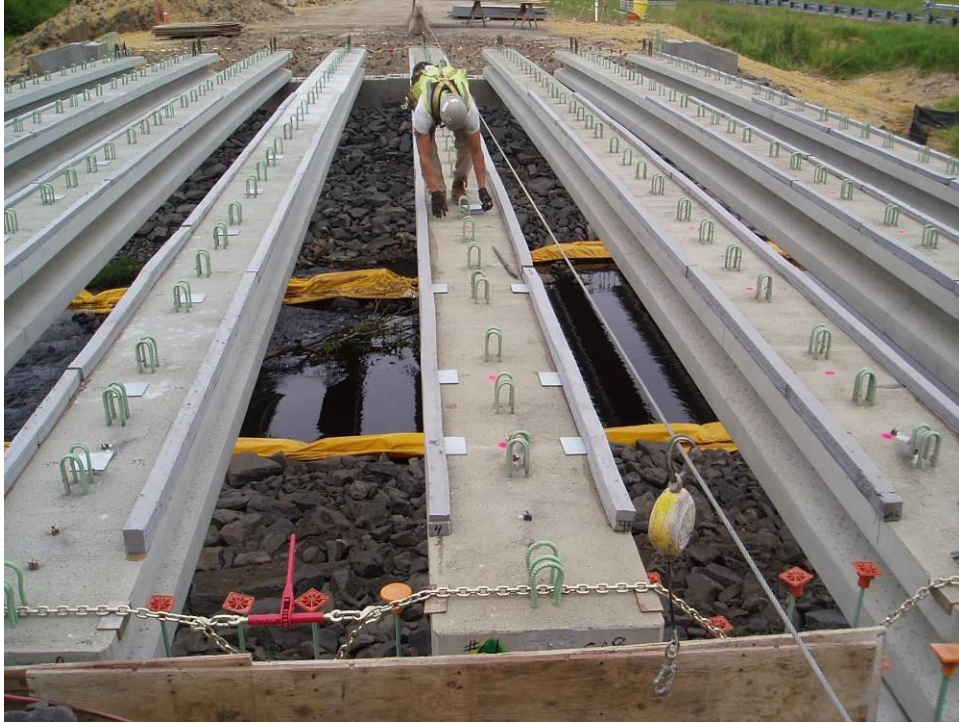
Figure 17. Placement of the leveling plates on top of the concrete girders.
