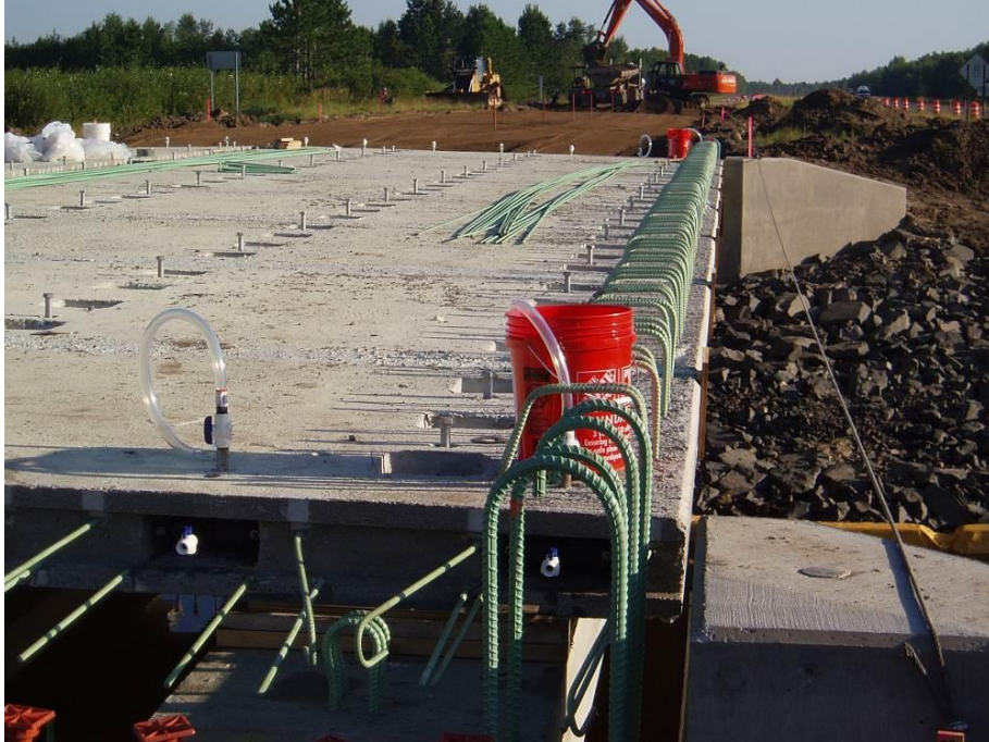
Figure 62. Testing and clearing the corrugated post-tensioning ducts prior to grouting.
