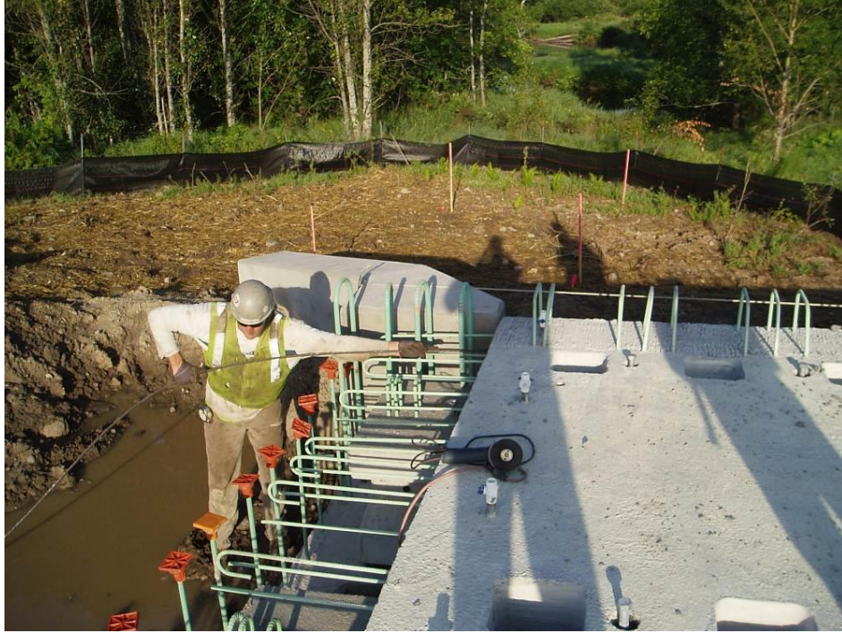
Figure 58. Installing the post-tensioning strands.
