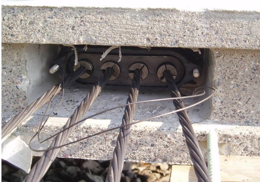
Figure 60. Anchoring the post-tensioning strands.
