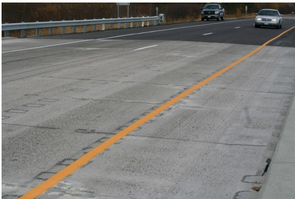
Figure 77. Both inside and outside shoulders of the new bridge are wider, resulting in improved motorist safety.
