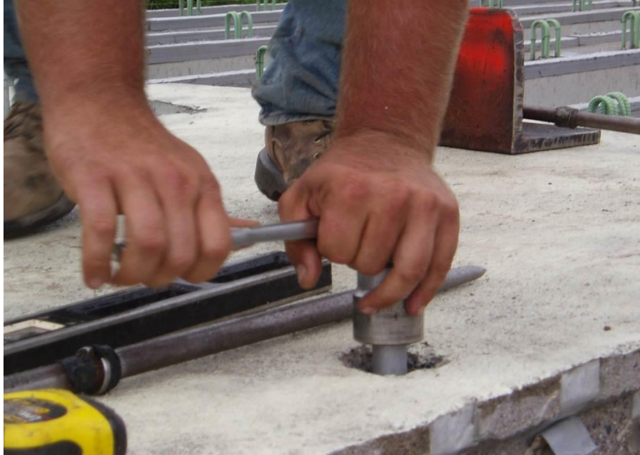
Figure 32. Close-up of torquing the leveling bolts to achieve the proper grade.
