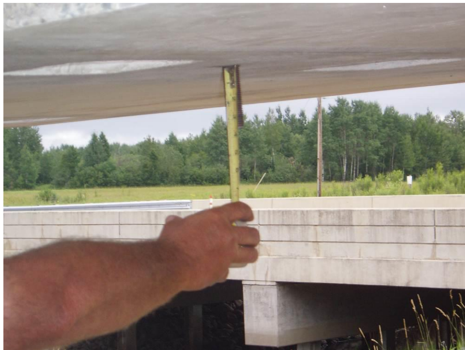
Figure 25. Protusion of the leveling bolt at the bottom of the deck panel to lift the deck panel above the surface of the girder and form the haunches.
