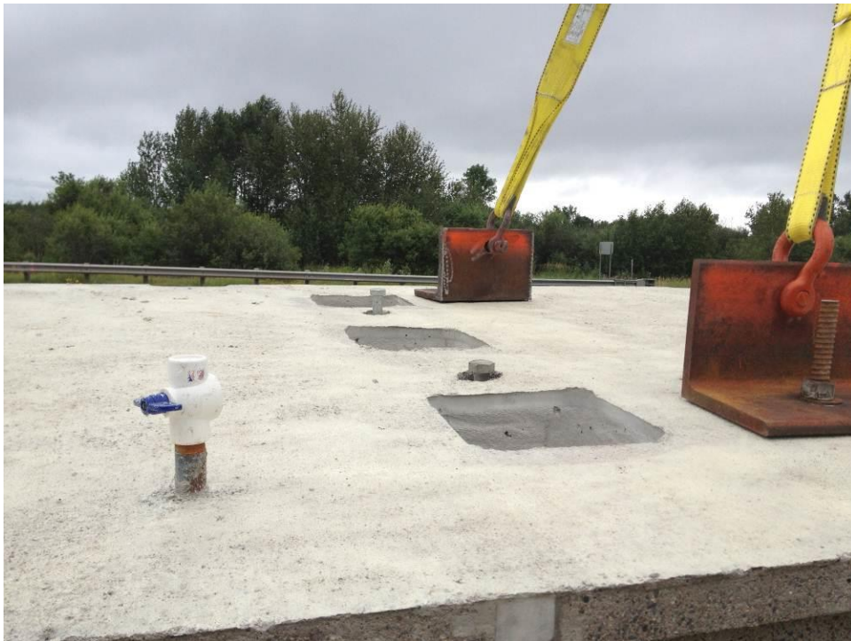
Figure 23. Close-up of the lifting hardware.
