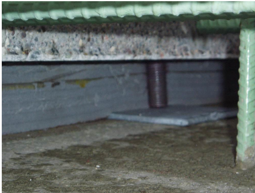
Figure 33. Leveling bolt resting on the steel plate on top of the girder.
