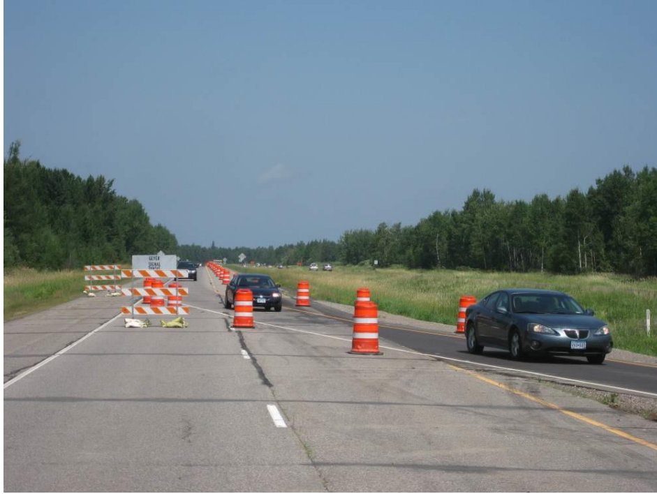
Figure 74. Taper and north bypass due to closure of the southbound lanes.
