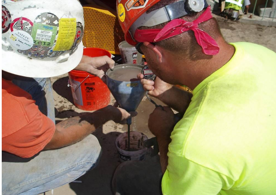
Figure 64. Measuring fluidity of grout using flow cone to meet manufacturer's specifications.
