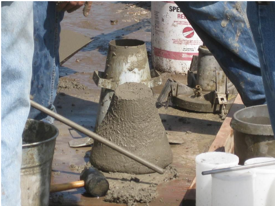
Figure 49. Testing the grout for slump.
