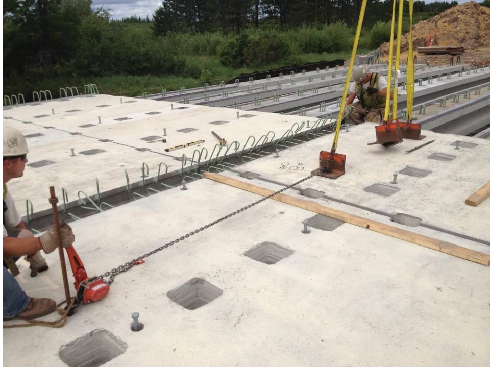
Figure 36. Alignment of deck panels.
