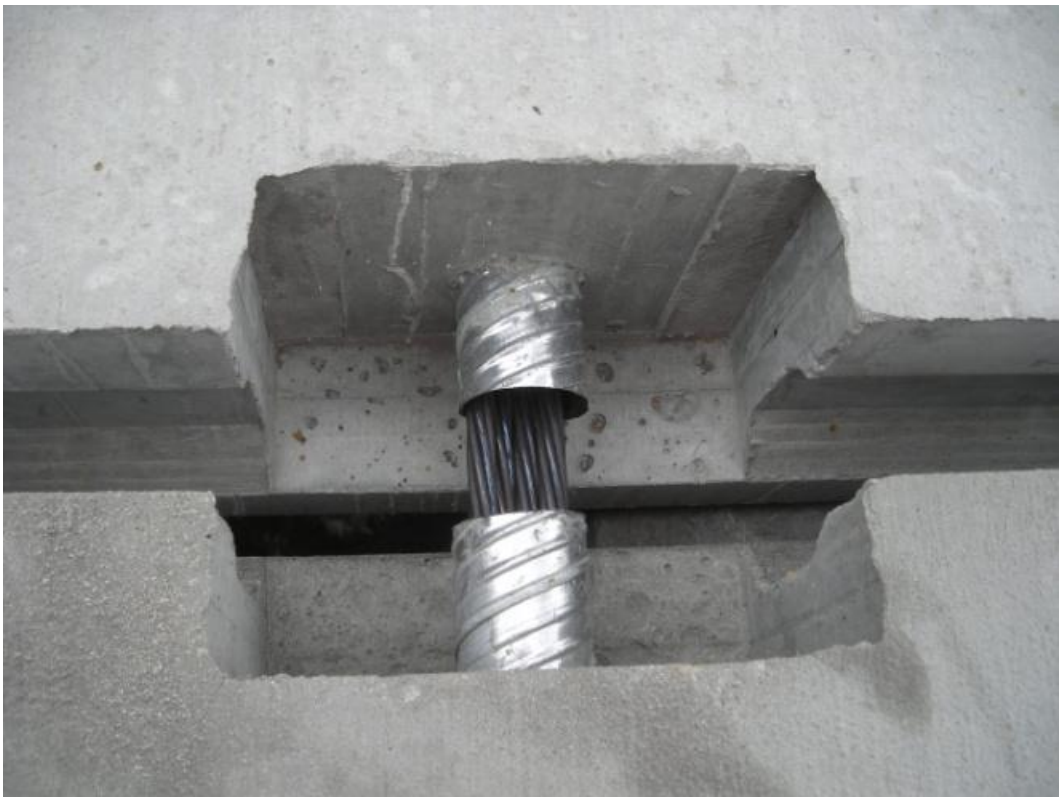
Figure 15. Photo. Posttensioning ducts between deck panels.
