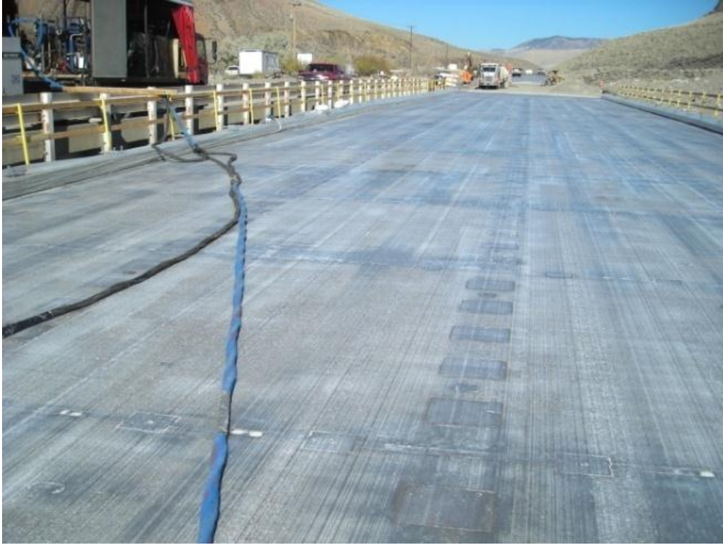
Figure 16. Photo. Finished milled deck.
