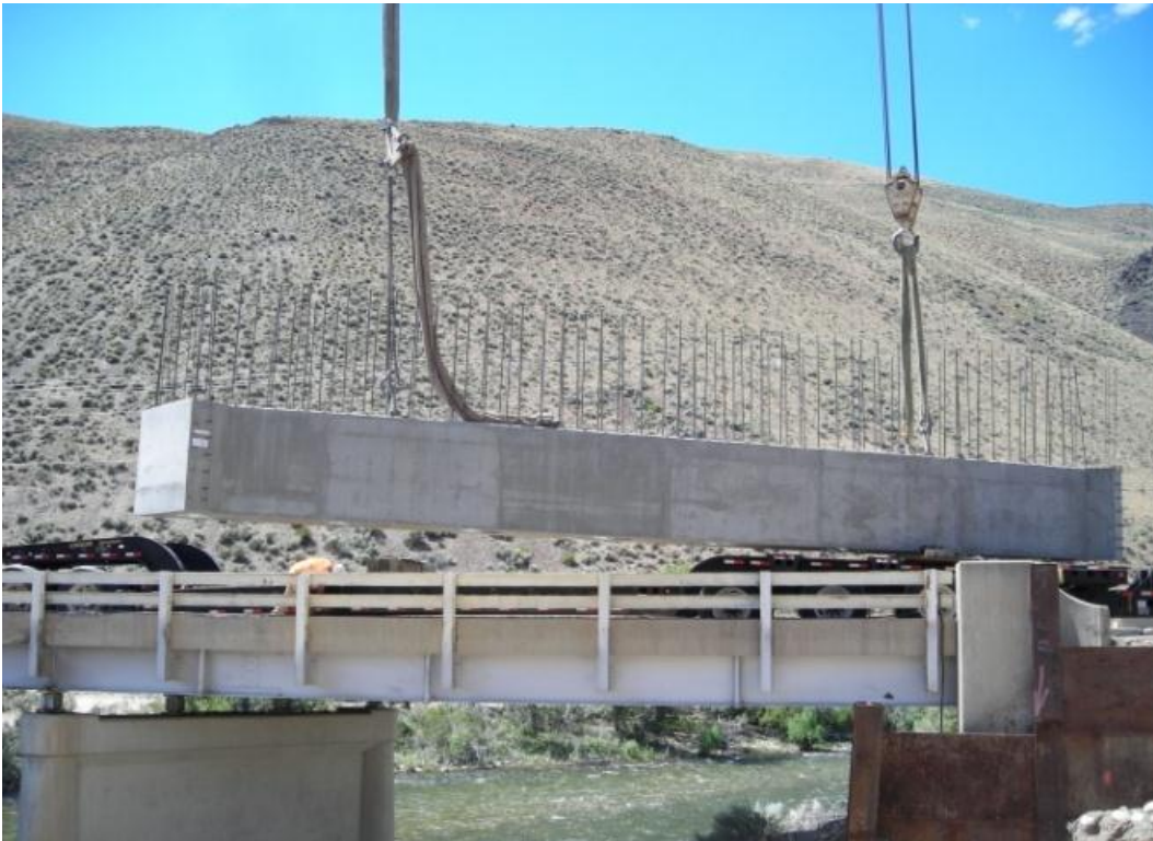
Figure 5. Photo. Precast abutment.
