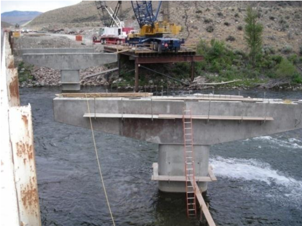
Figure 11. Photo. Completed pier.
