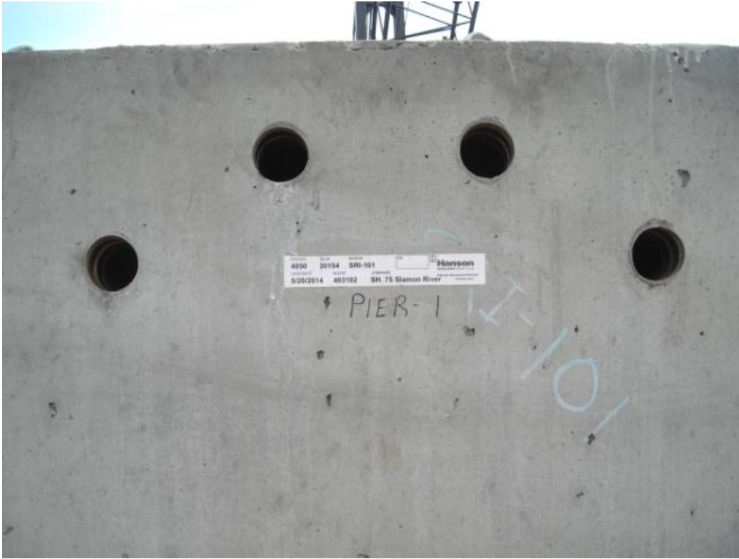
Figure 8. Photo. Pier column sleeves.
