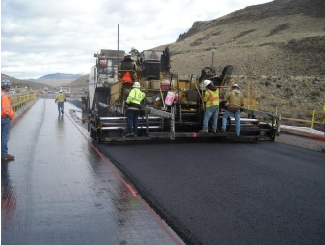
Figure 17. Photo. Paving on deck.
