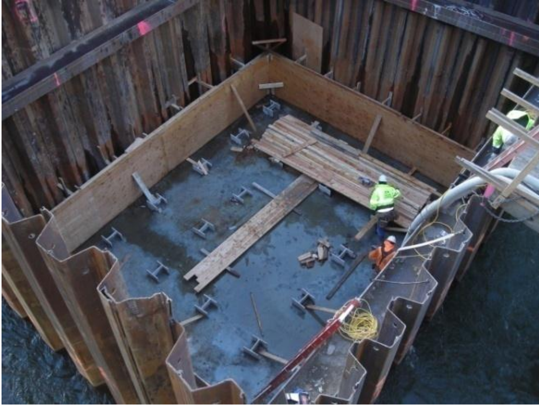
Figure 6. Photo. Pile cap for pier.
