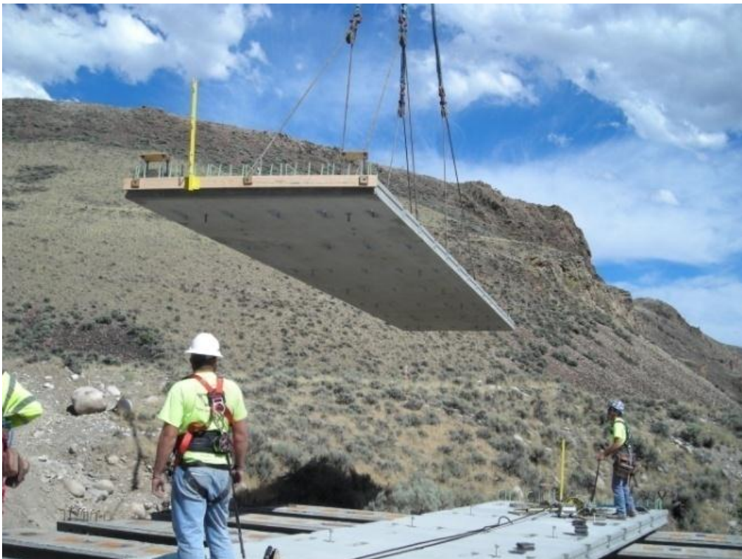
Figure 13. Photo. Deck panel placement.
