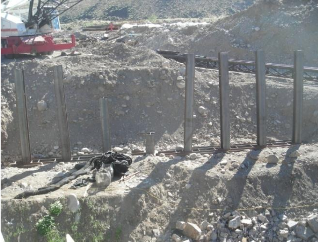
Figure 4. Photo. Piling for abutment.
