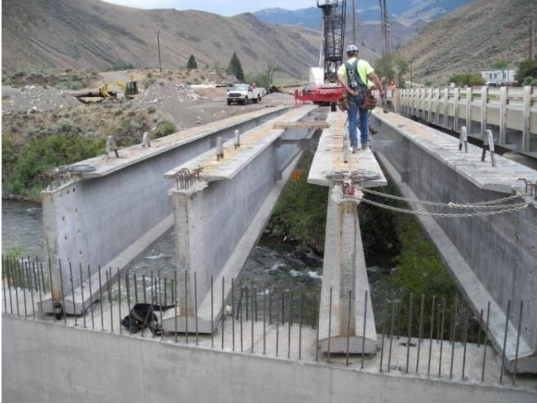
Figure 12. Photo. Girder placement.
