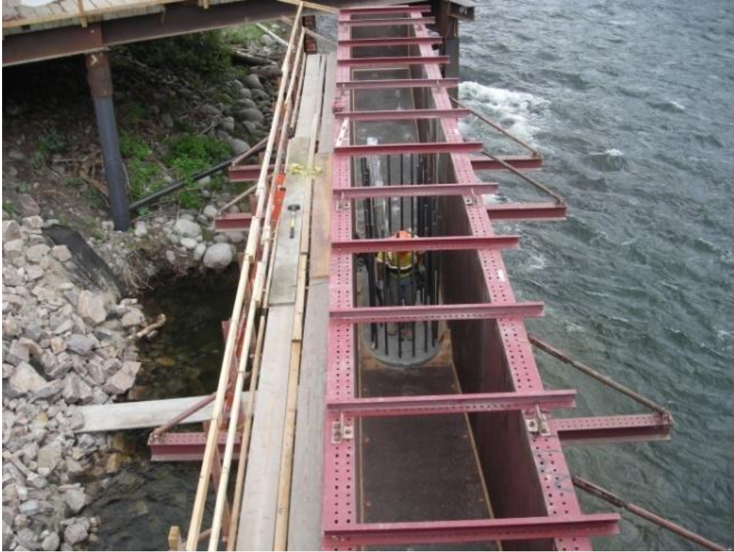
Figure 10. Photo. Pier cap form.
